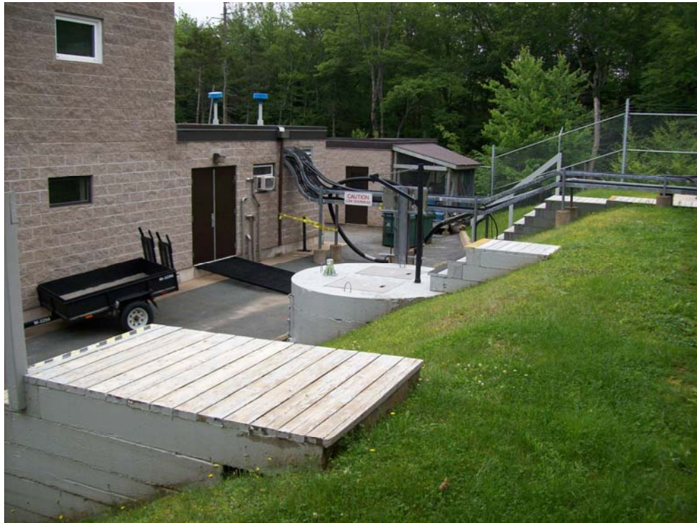
Photo 28 Lockview Effluent Pumping Station
