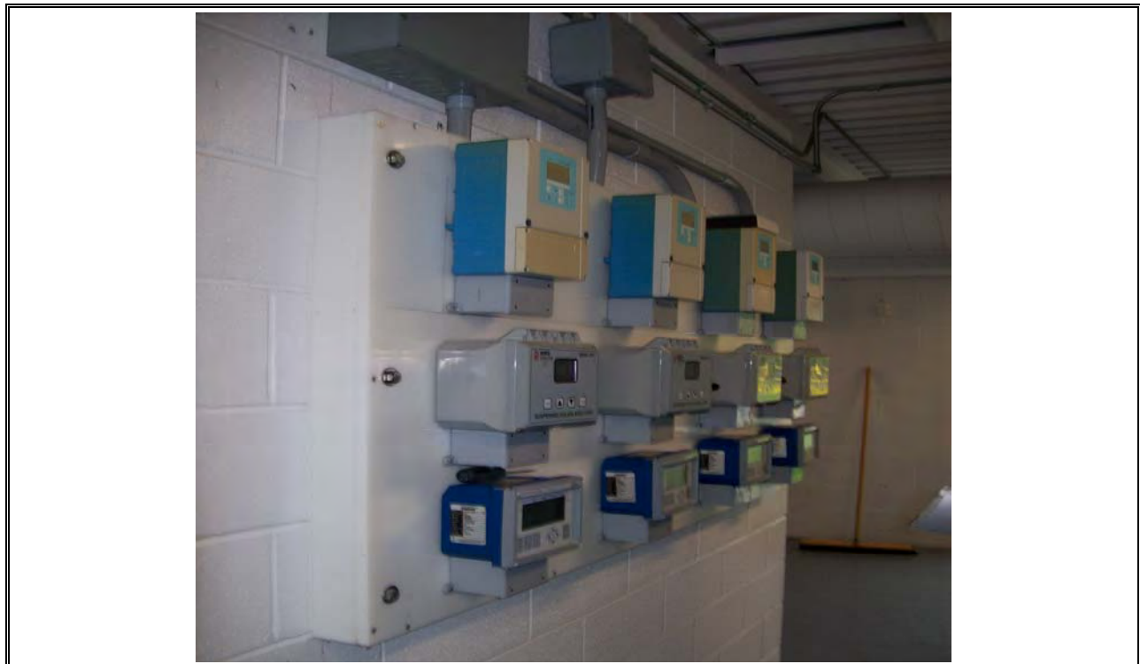
Photo 26 AeroTech SBR Online Analyzer Control Panel
