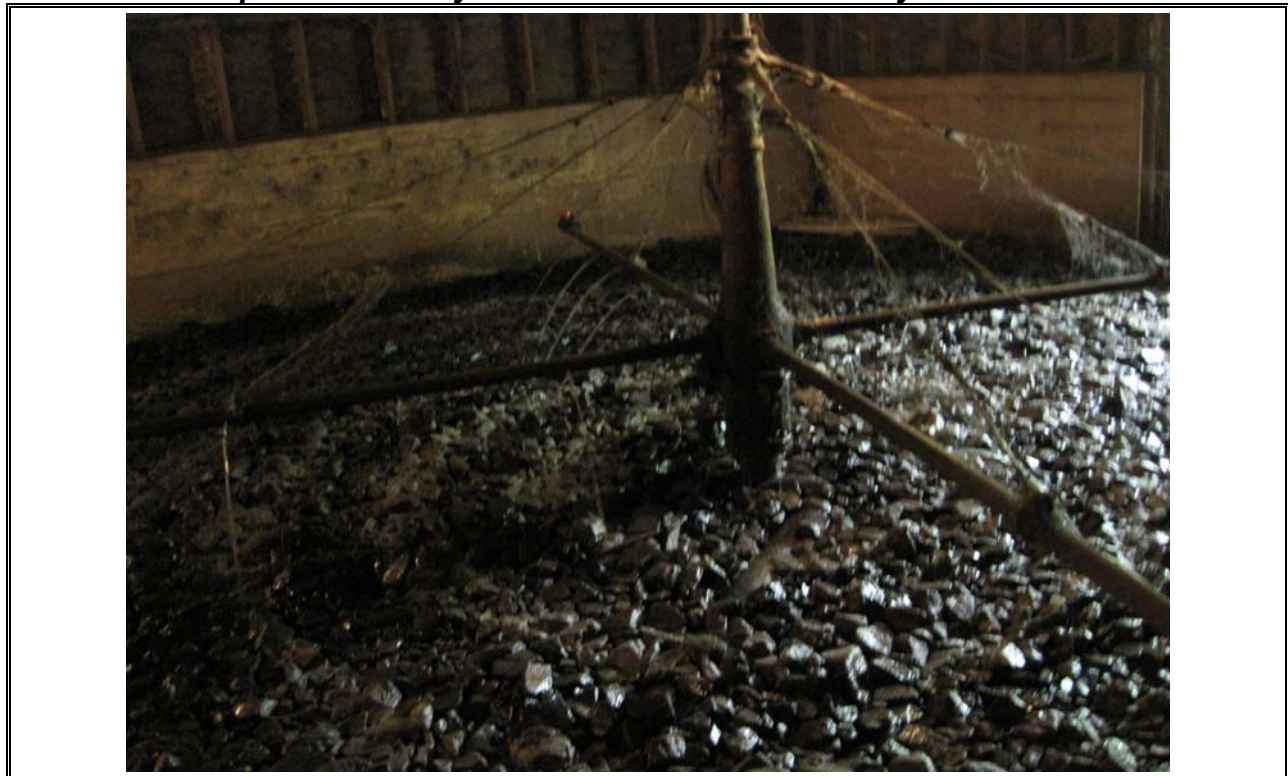
Photo 12 Uplands Park Distribution Arm Blockage
