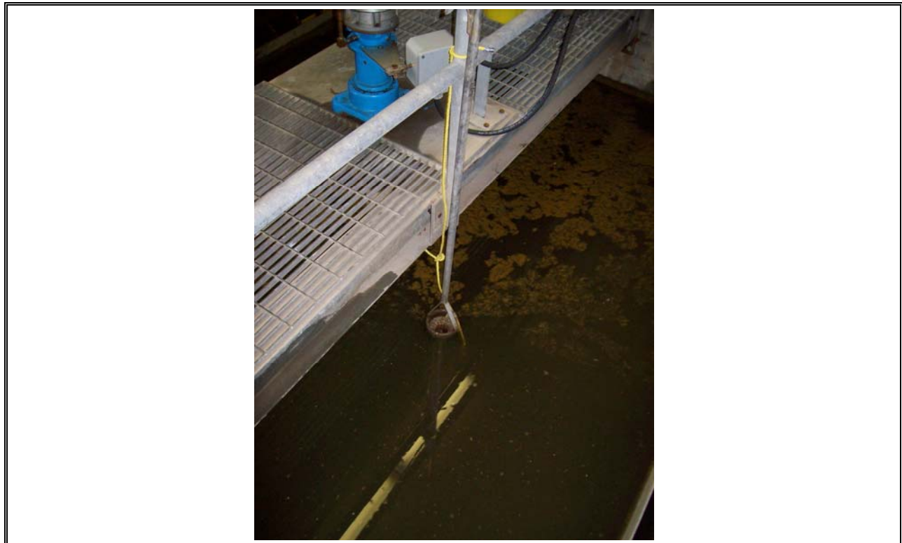
Photo 14 Lockview Manual Skimming of Secondary Clarifier
