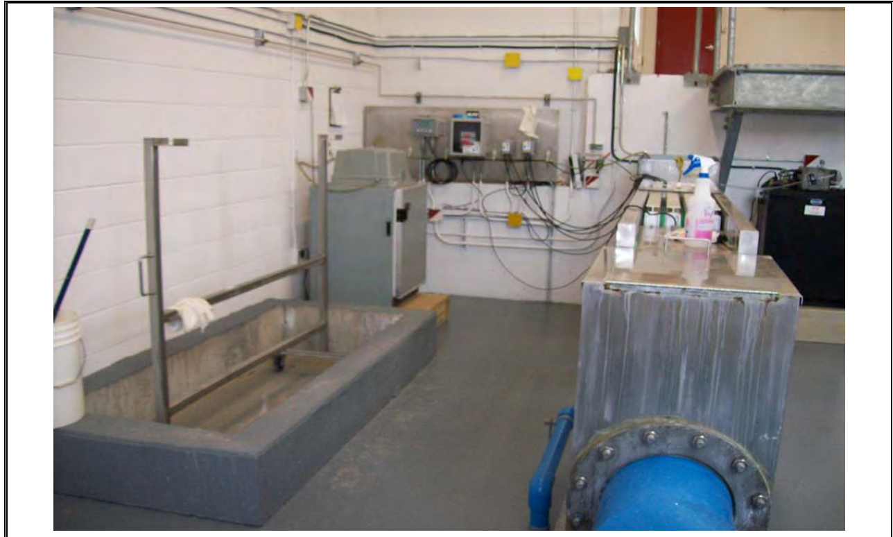
Photo 31 AeroTech UV System and Effluent
