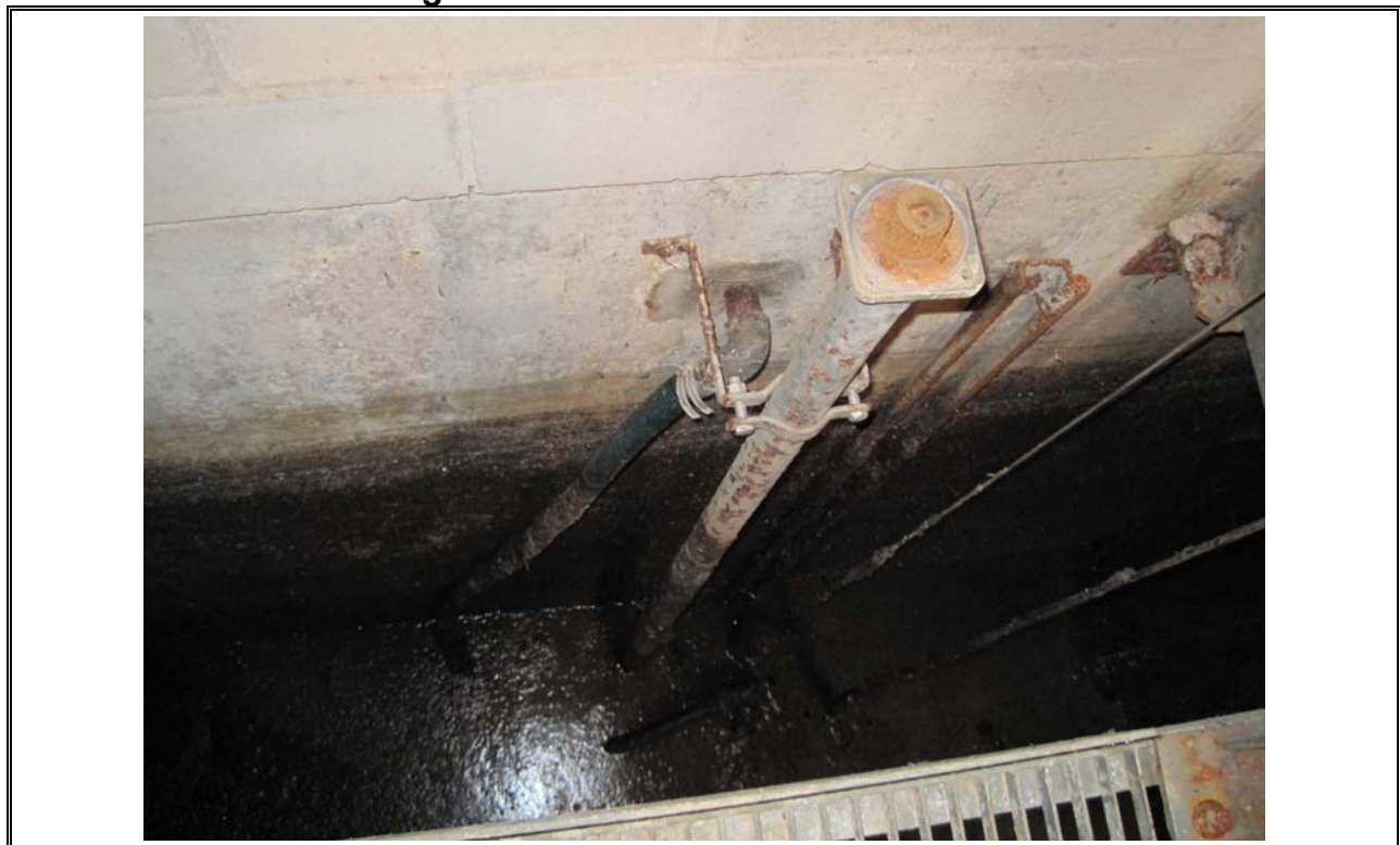
Photo 26 Waste Sludge Tank and Supernatant Line
