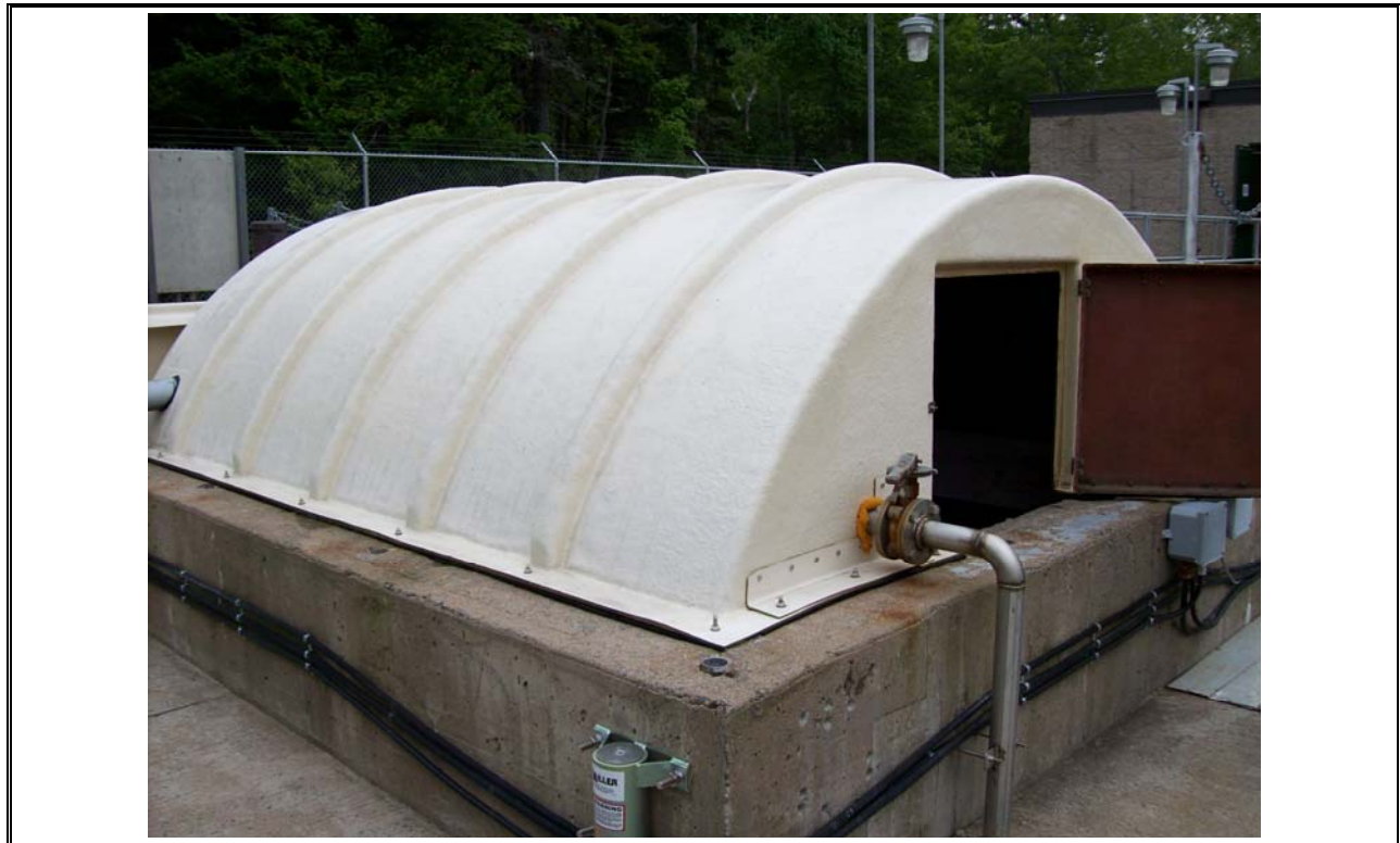
Photo 3 Lockview Covered Equalization Tank
