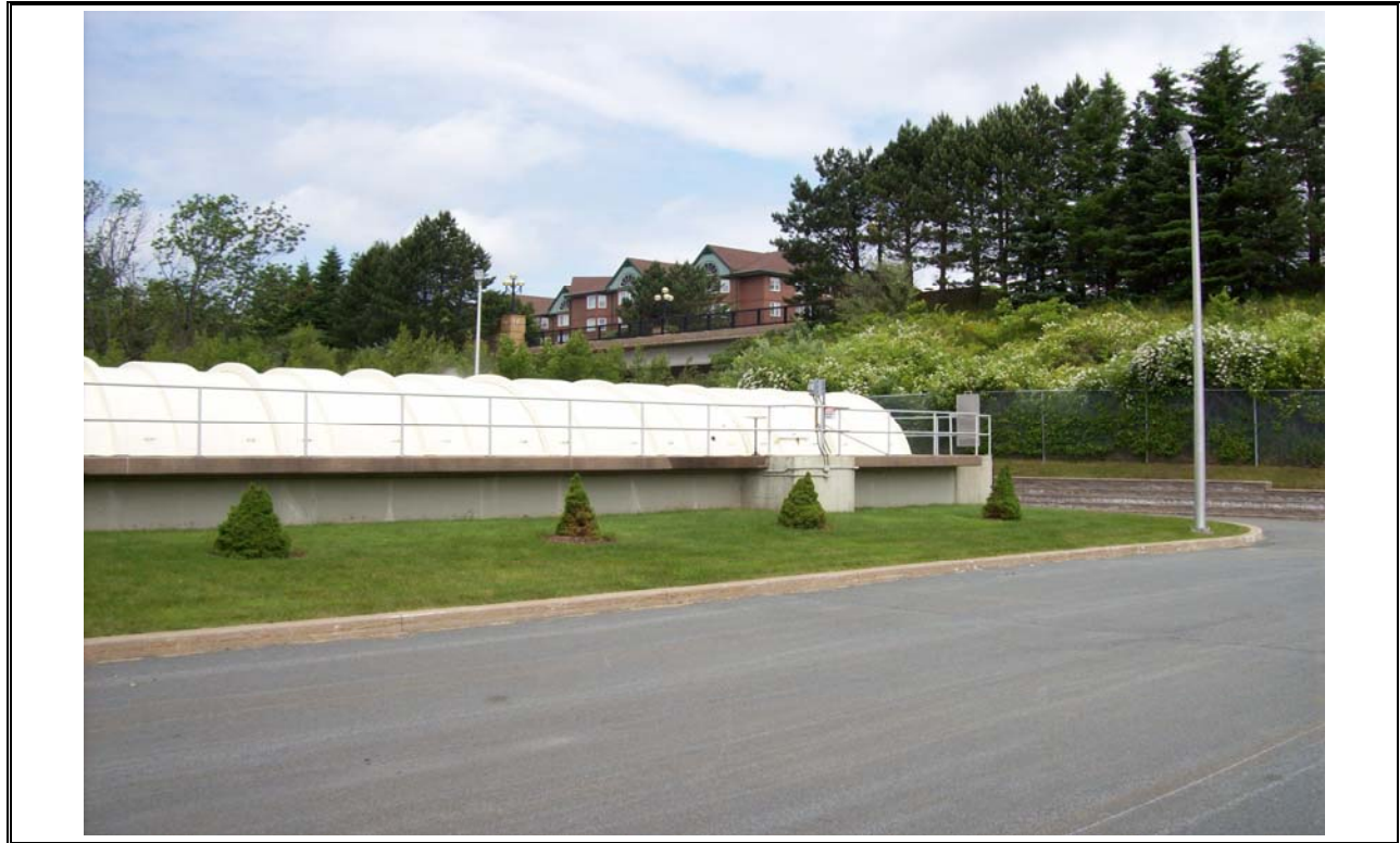
Photo 17 North Plant Covered Primary Clarifiers
