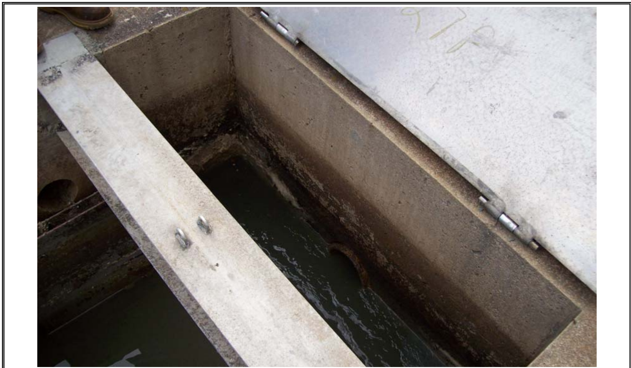
Photo 4 Grit Removal and Influent Line to Screen
