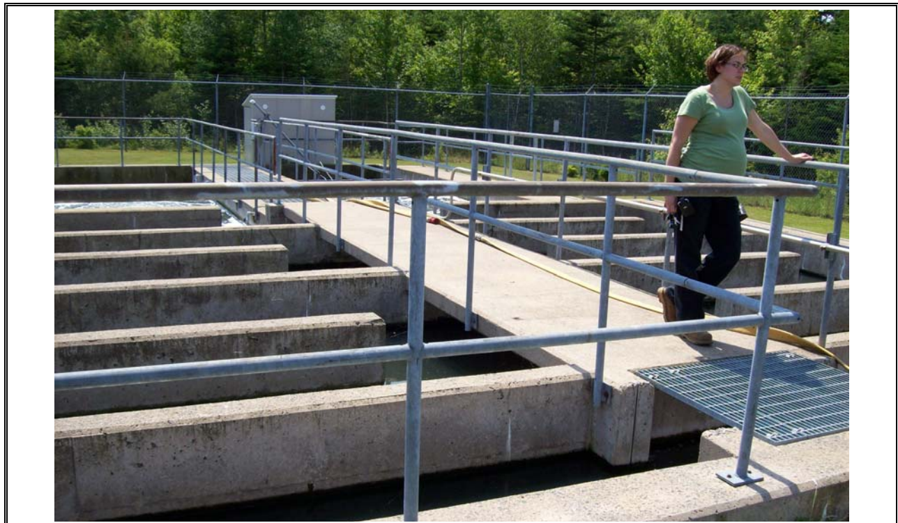
Photo 36 Chlorination/Post Aeration Tanks
