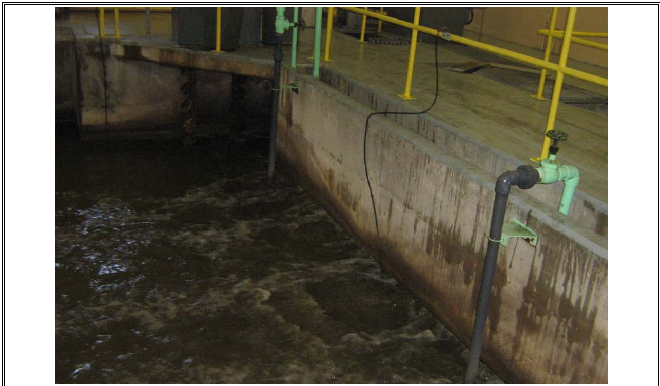
Photo 12 Aerated Grit Chamber
