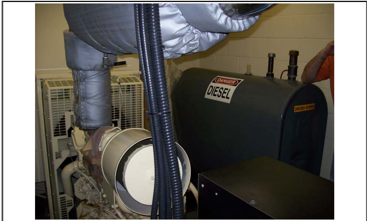
Photo 31 Lockview Diesel Tank for Genset
