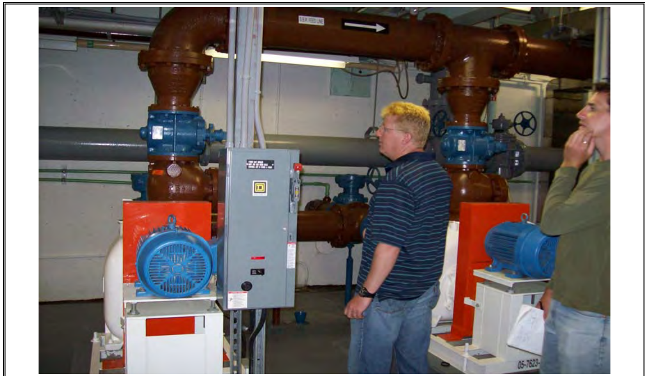
Photo 22 AeroTech SBR Feed Pumps
