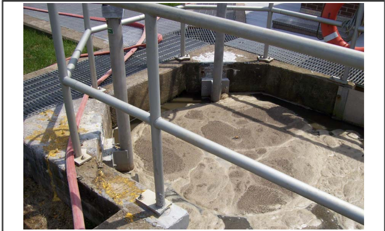
Photo 33 Secondary Clarifier Influent Flow Control 2
