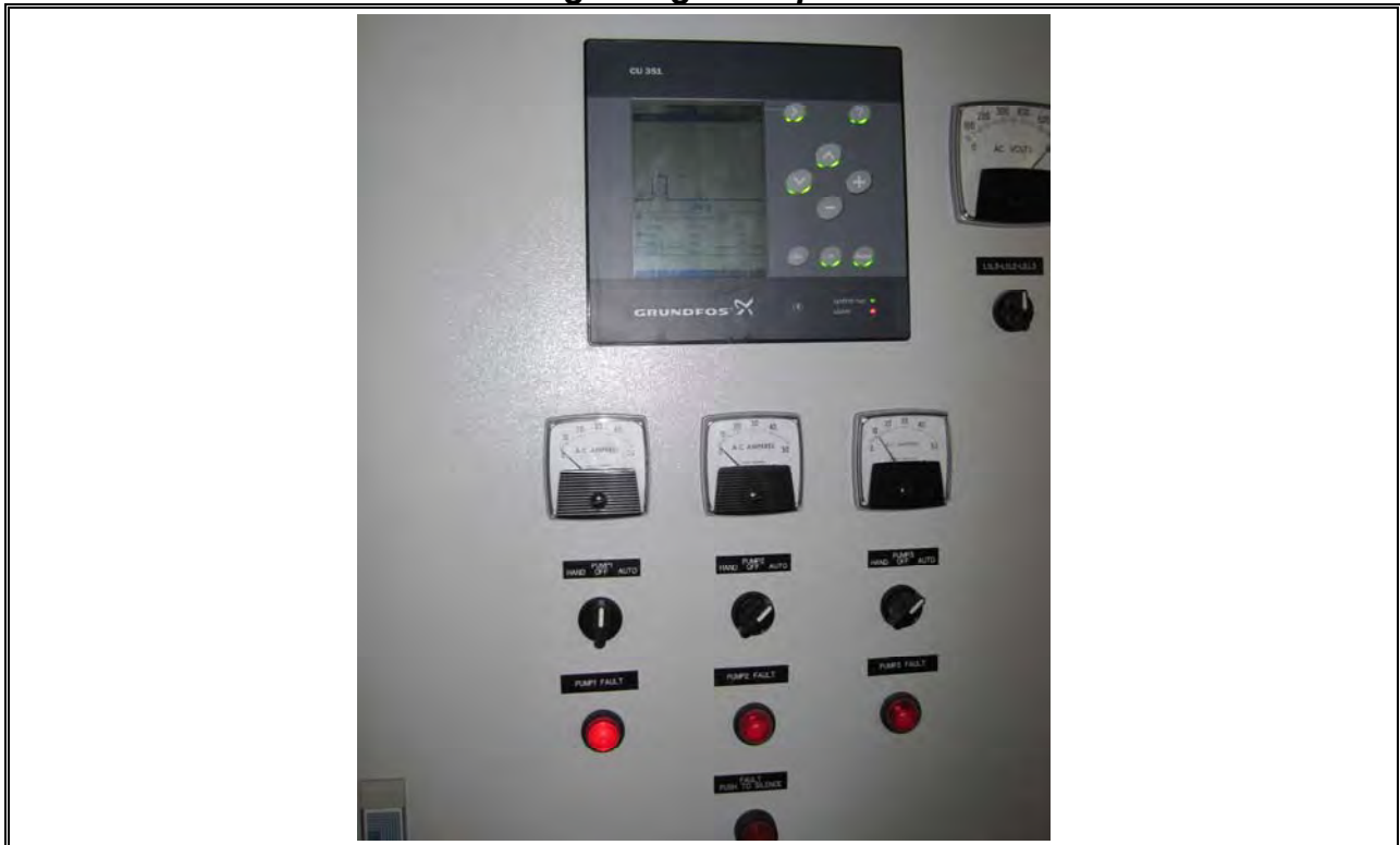
Photo 38 Dartmouth Sludge Pump Panel Controller
