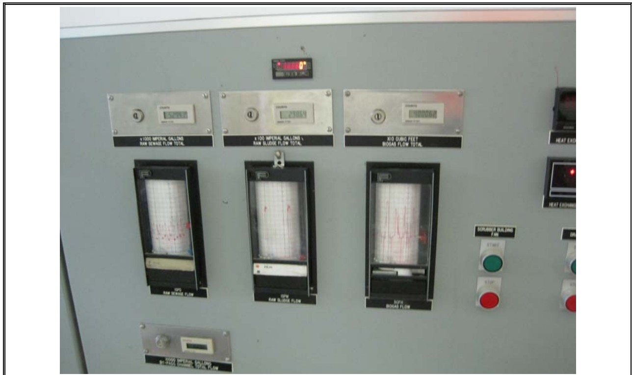
Photo 4 Eastern Passage Flow Tracking Panel
