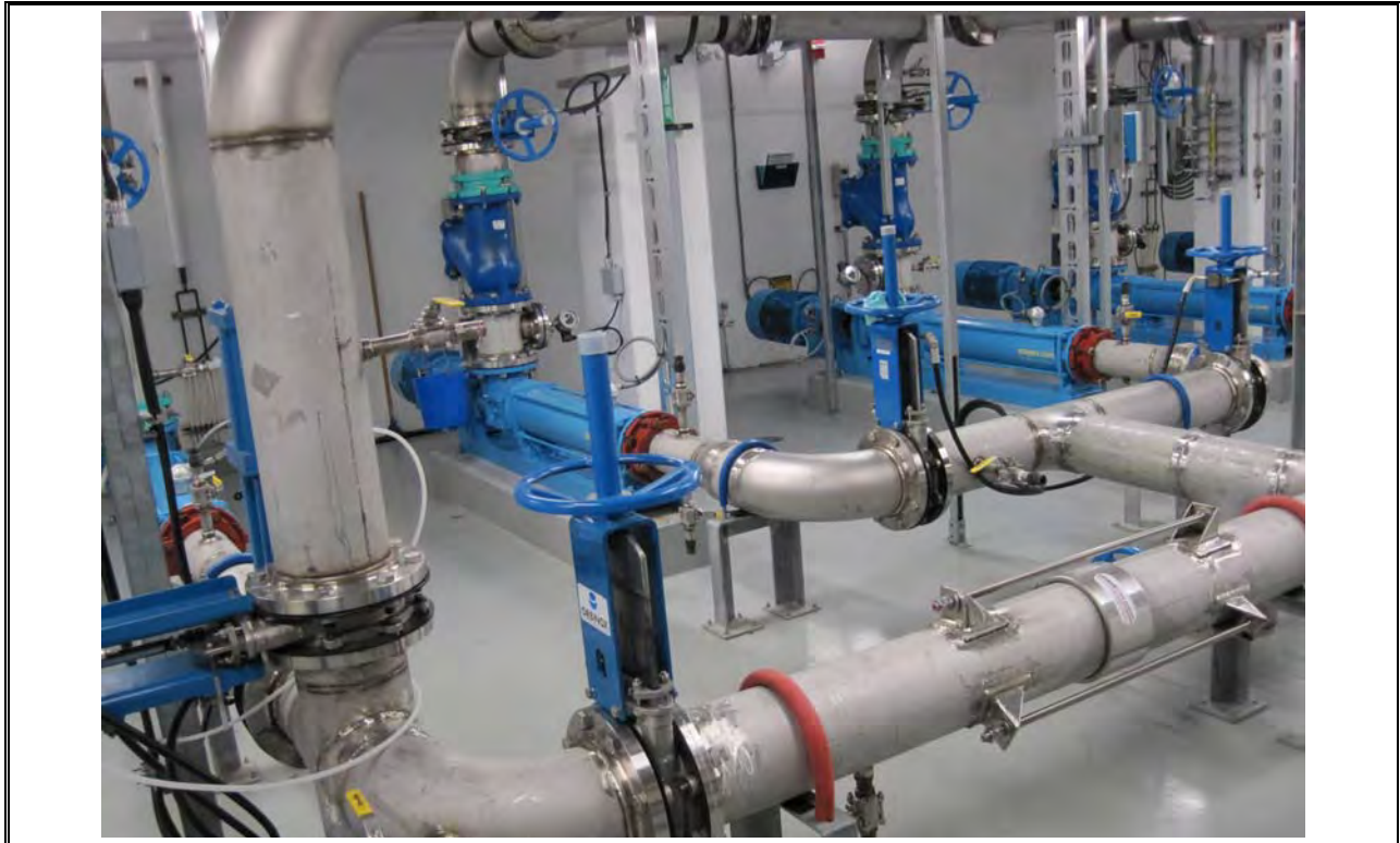
Photo 37 Dartmouth Densadeg Sludge Pumps
