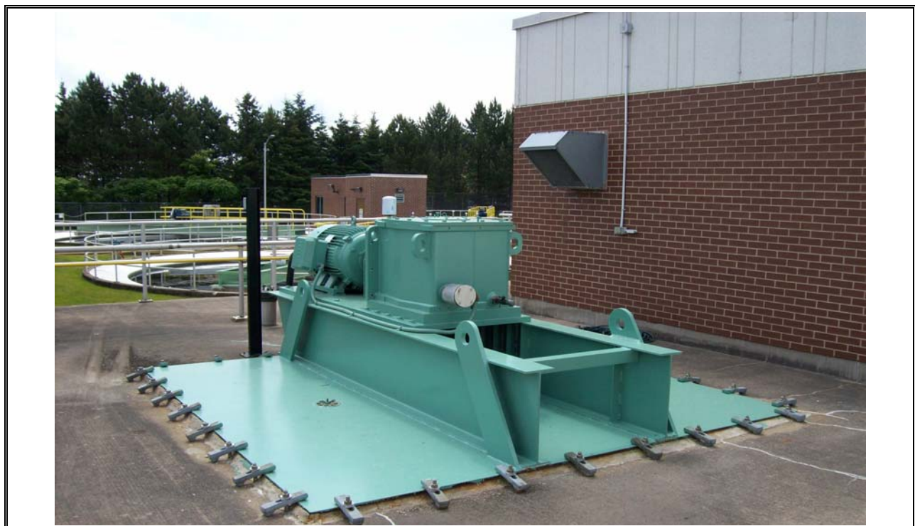
Photo 22 Bioreactor Paddle Mixer Motor
