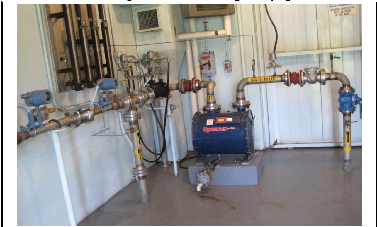
Photo 30 Eastern Passage Digester Gas Split to Boiler and/or Flare
