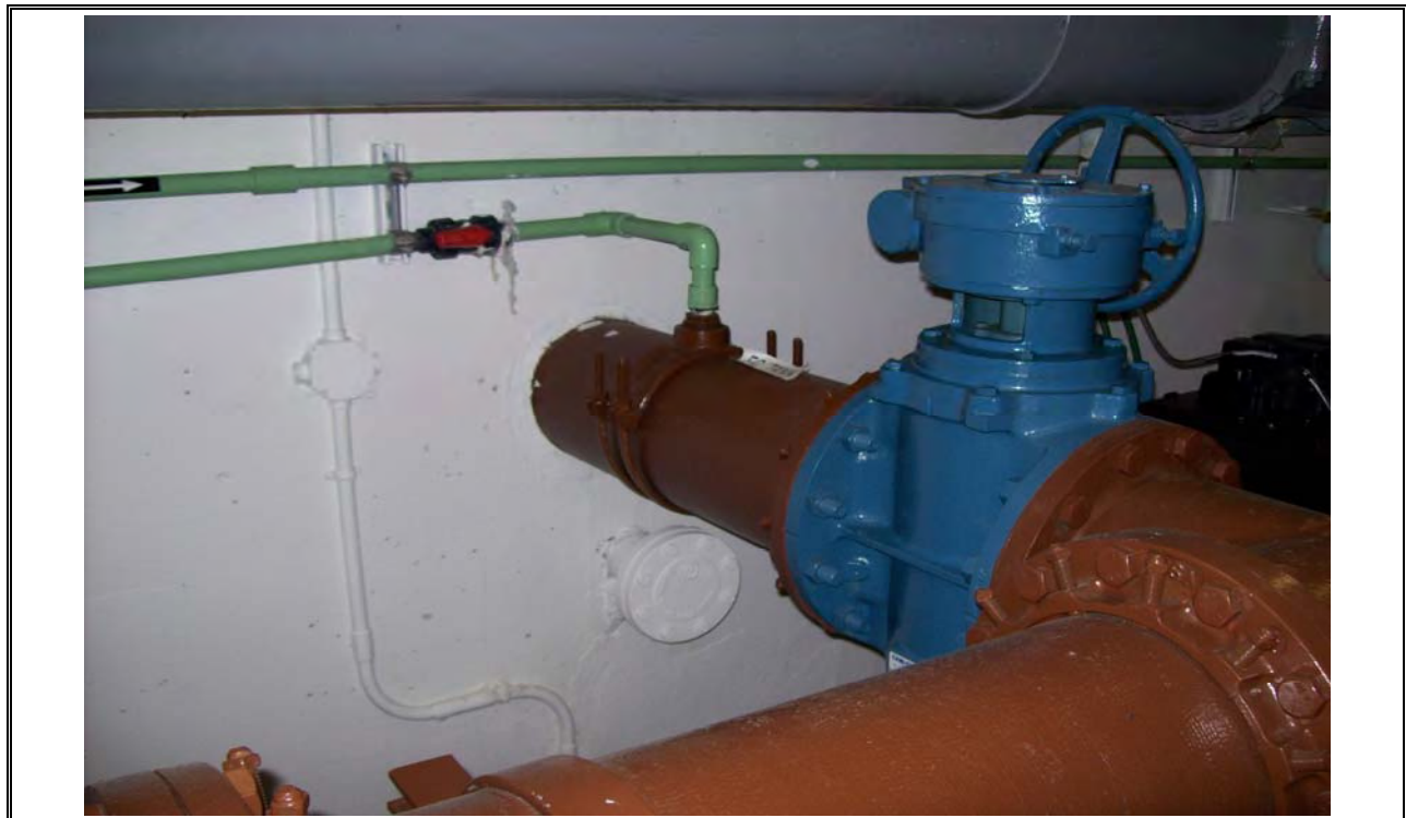
Photo 18 AeroTech Equalization Tank Effluent and Alum Injection Point
