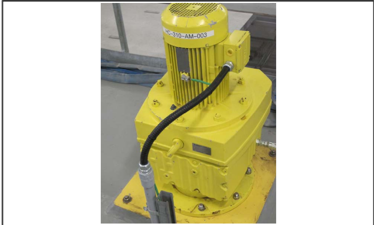
Photo 15 Herring Cove Rapid Mixer for Flocculation Tank
