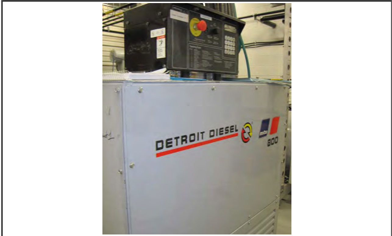
Photo 51 Dartmouth Diesel Generator Fuel
