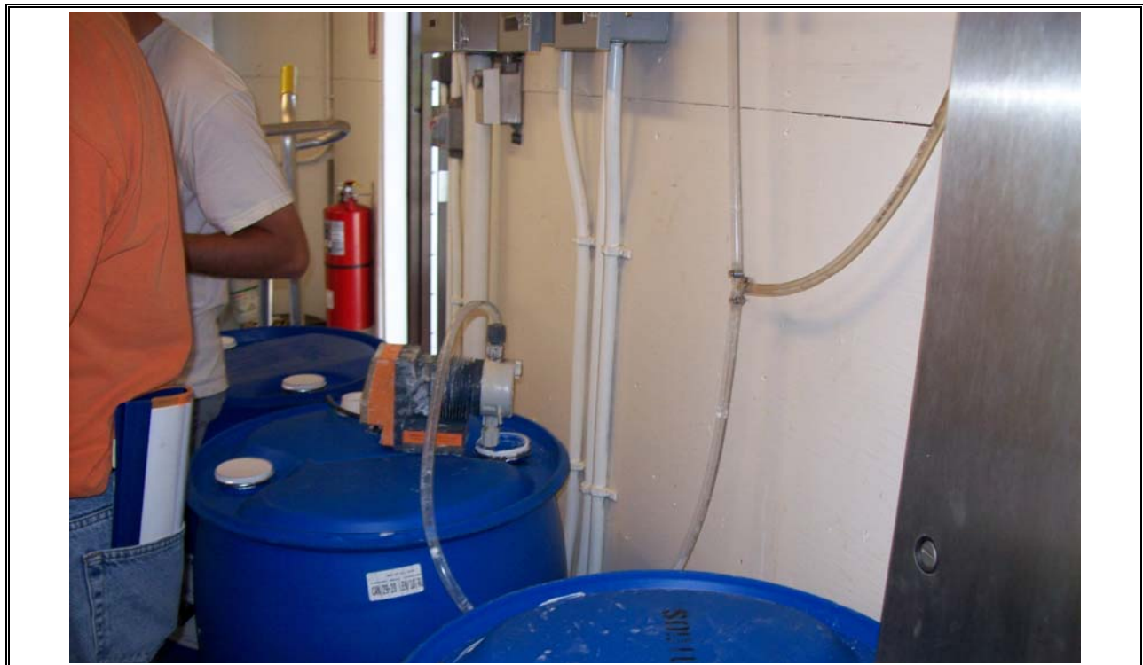
Photo 10 Lime Feed System
