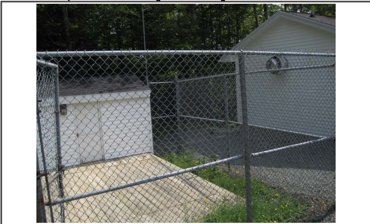
Photo 16 Uplands Park Secondary Clarifier and Chlorination Building
