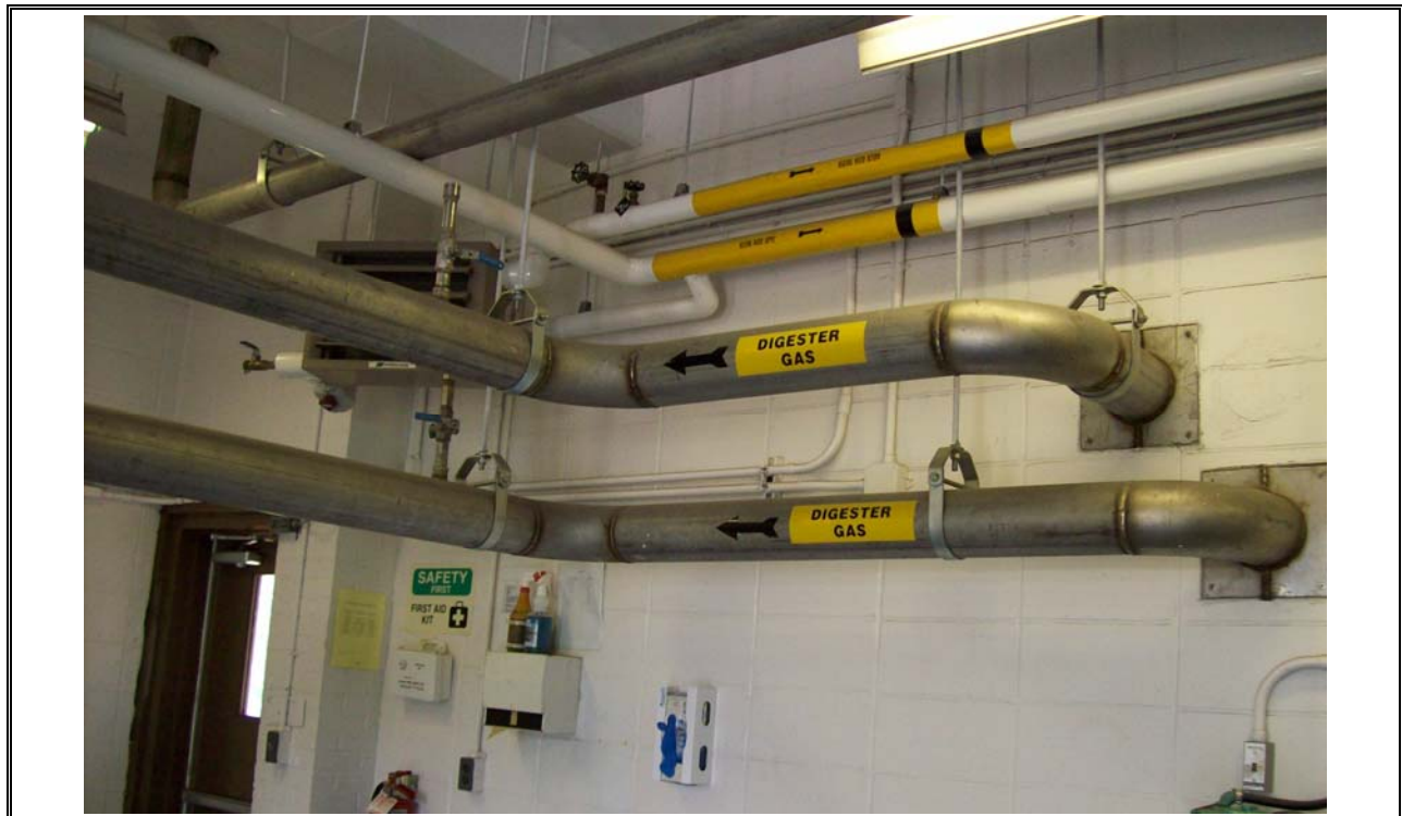
Photo 48 Digester Gas from Secondary Digester Cover
