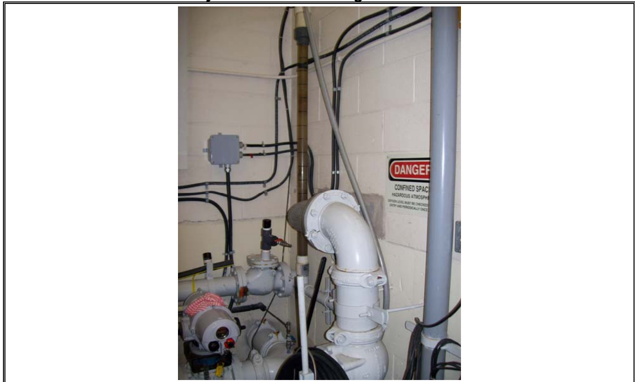
Photo 24 Lockview Filter Effluent Piping and Sightglass
