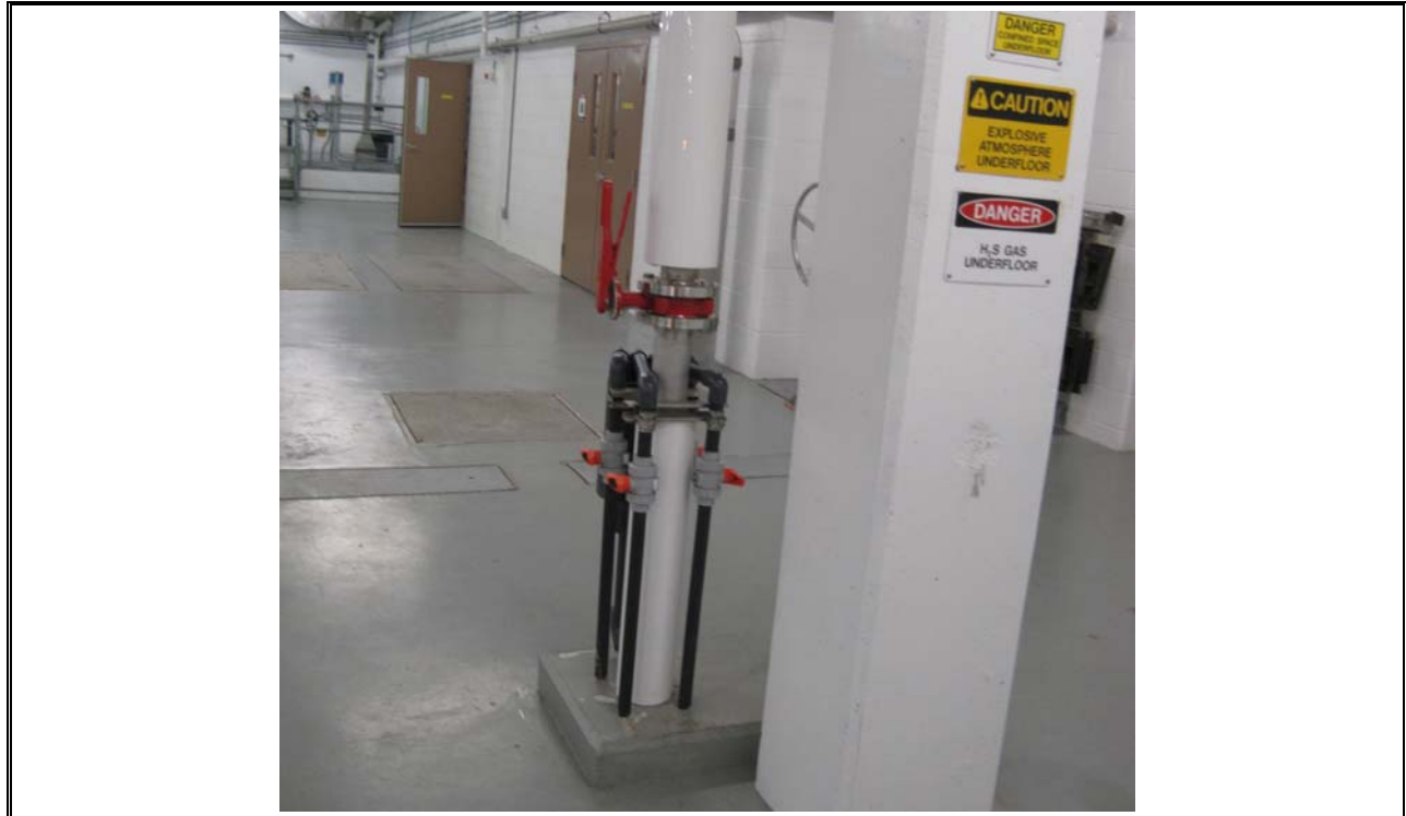
Photo 11 Herring Cove Two Trains of Grit Removal & Parshall Flumes Below Floor
