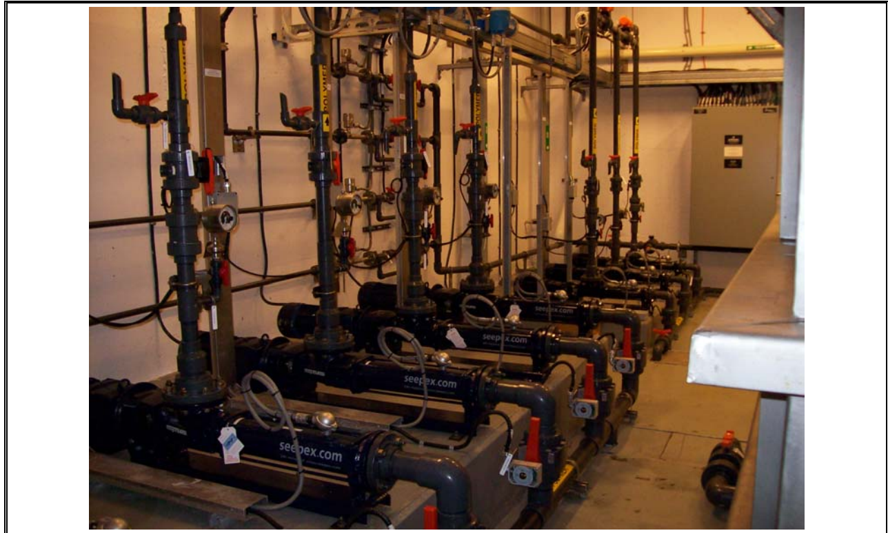
Photo 25 Halifax Densadeg Polymer Feed Pumps
