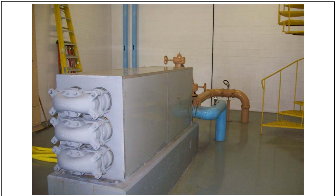
Photo 60 Heat Exchanger for Anaerobic Digester
