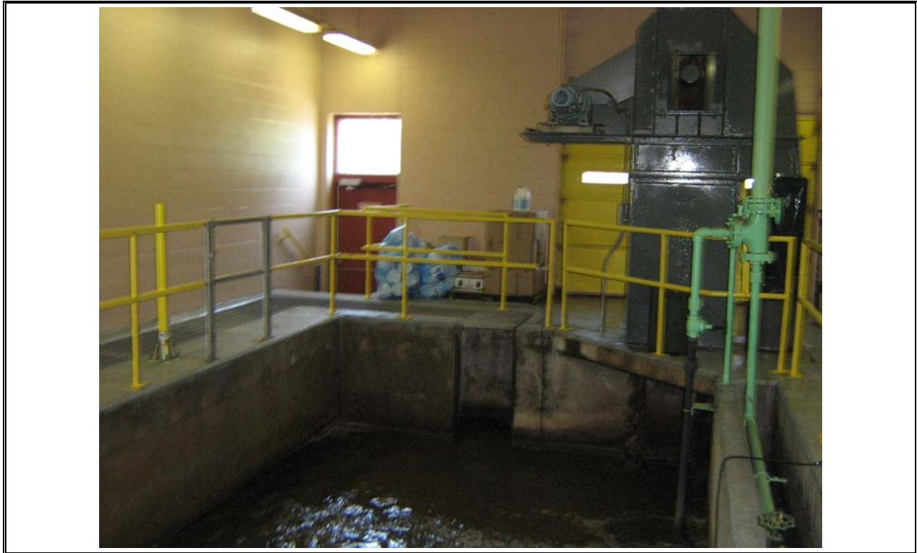
Photo 11 Aerated Grit chamber
