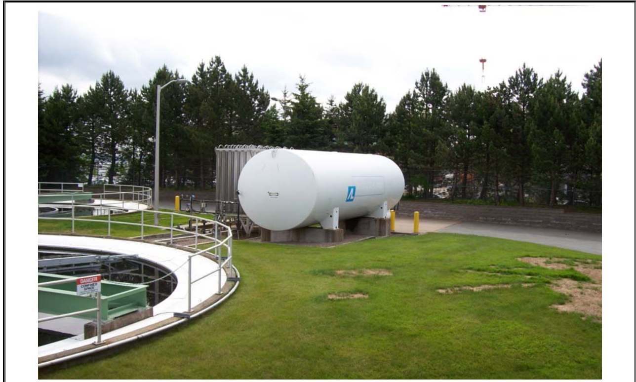
Photo 25 Oxygen Storage Tank
