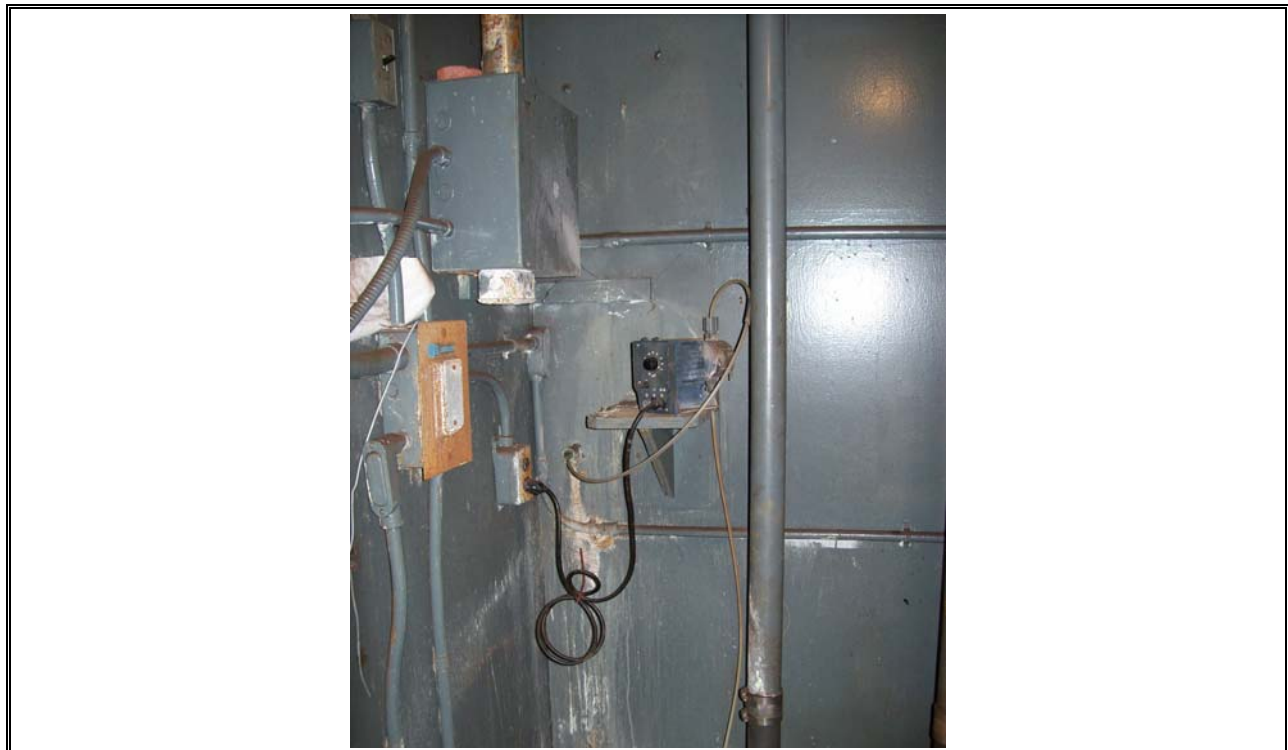
Photo 18 Wellington Chlorine Metering Pump
