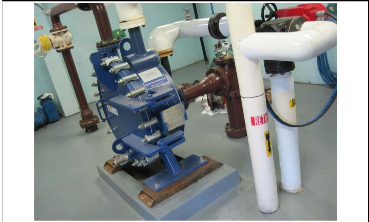
Photo 37 Eastern Passage Heat Exchanger for Sludge Recirculation
