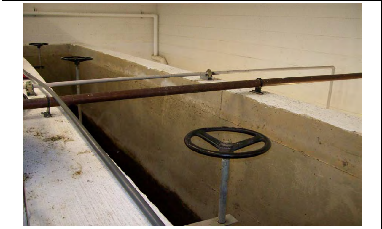
Photo 29 AeroTech Filter Backwash Channel
