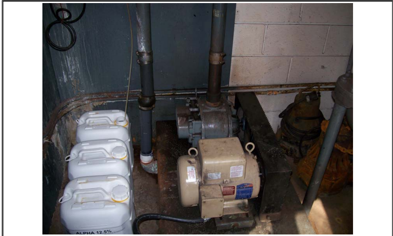
Photo 15 Wellington Blower and Chlorine Solution Storage
