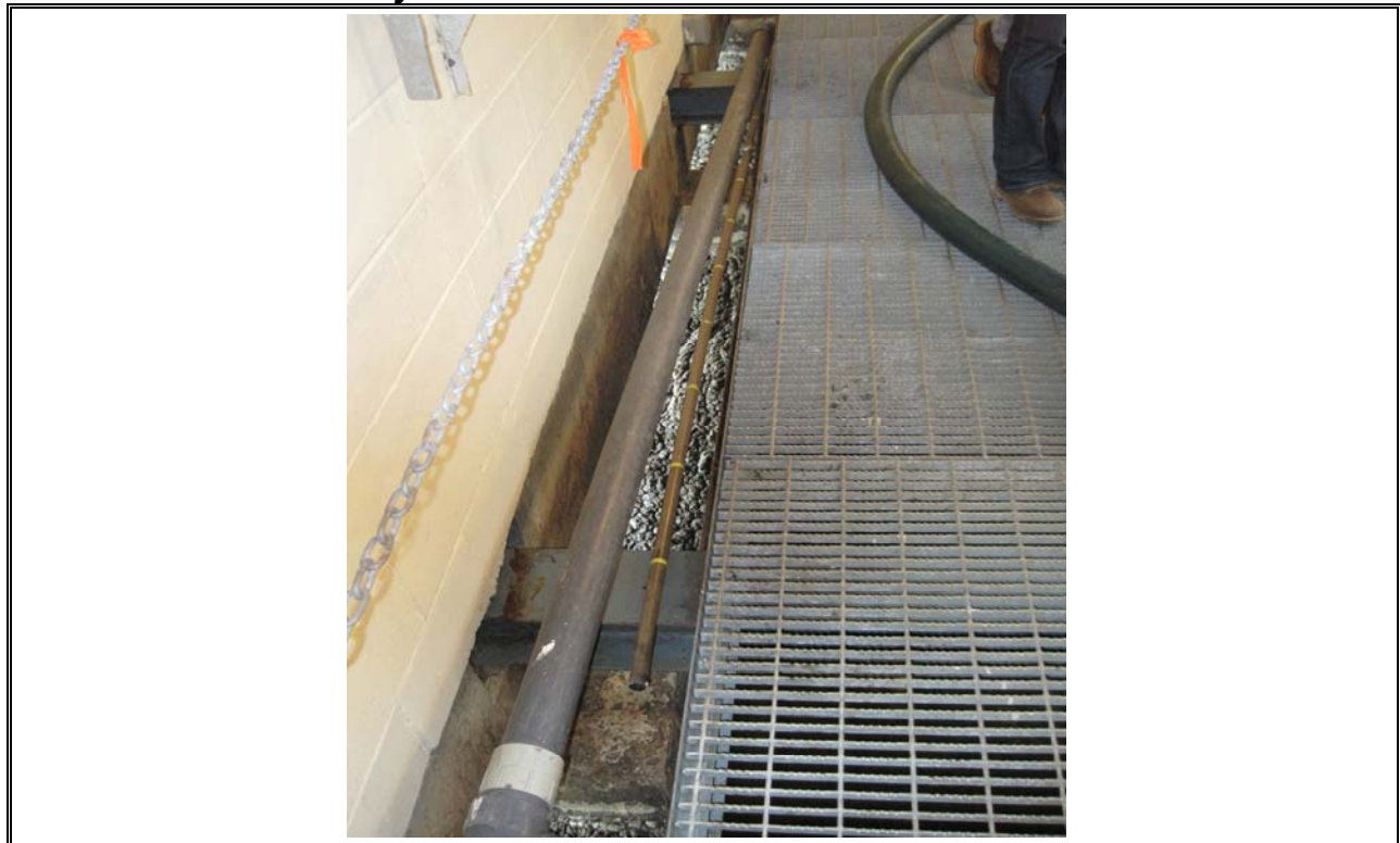
Photo 16 Scum Build-up in Secondary Clarifier Influent Channel
