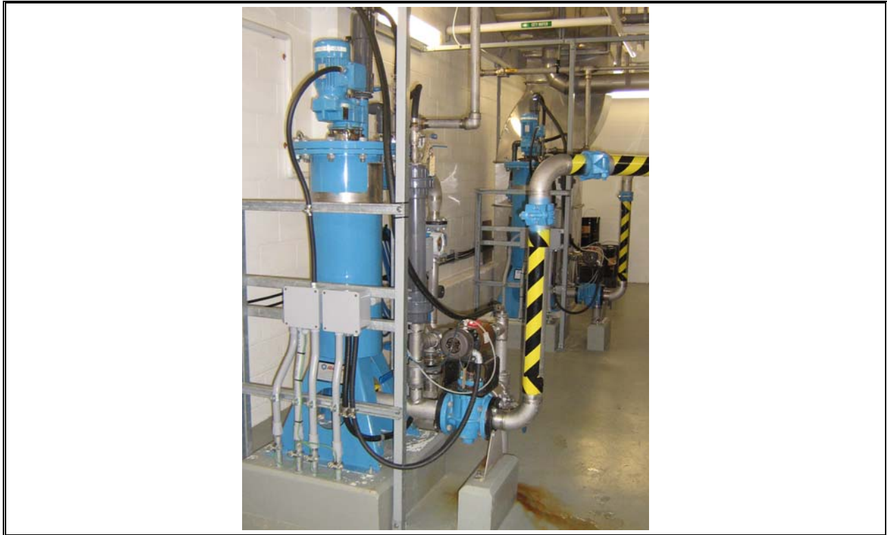
Photo 39 Herring Cove Sludge Flocculation Tank
