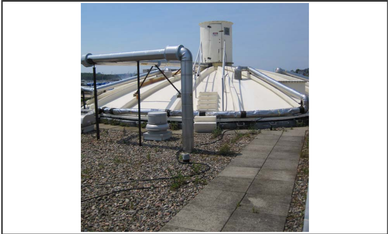
Photo 35 Eastern Passage Primary Digester Roof
