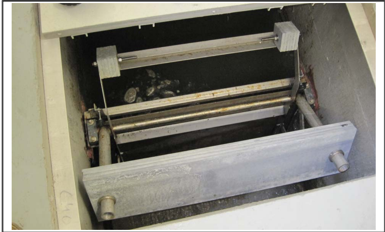
Photo 25 Herring Cove Final Effluent from UV Disinfection
