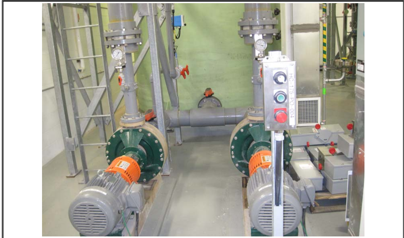
Photo 47 Herring Cove Wet Scrubber Solution Pumps
