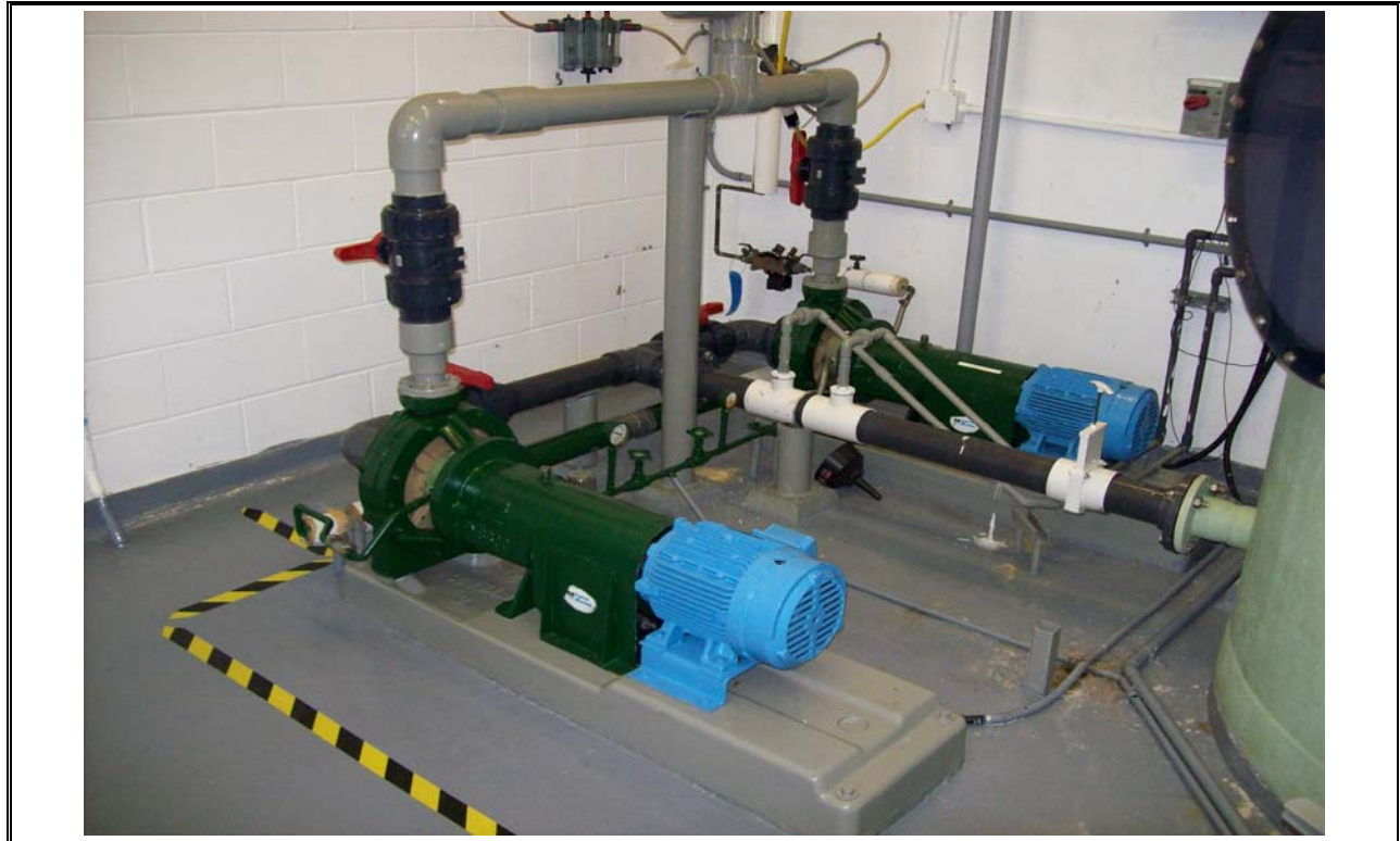
Photo 55 Wet Scrubber Recirculation Pumps
