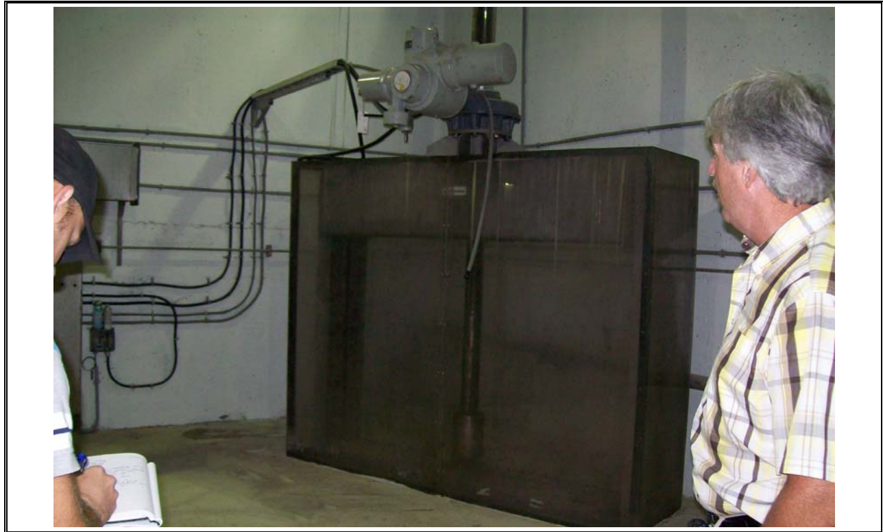
Photo 1 Halifax Main Influent Control Gate
