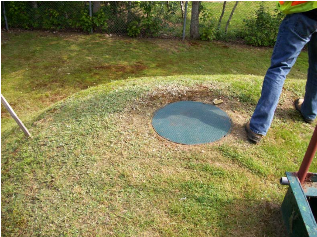
Photo 13 Wellington Effluent Manhole
