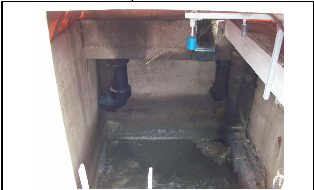
Photo 4 Lockview Equalization Tank and Ultrasonic
