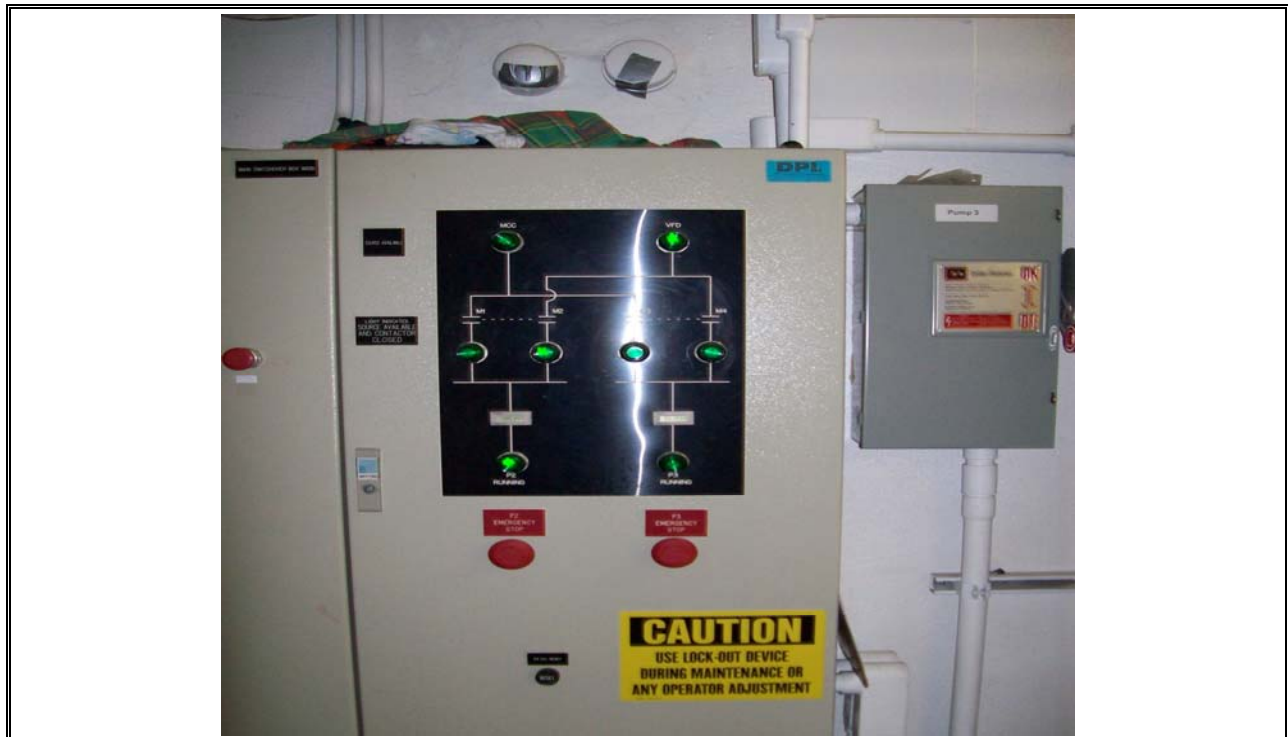
Photo 4 Influent Pumping Station Controls
