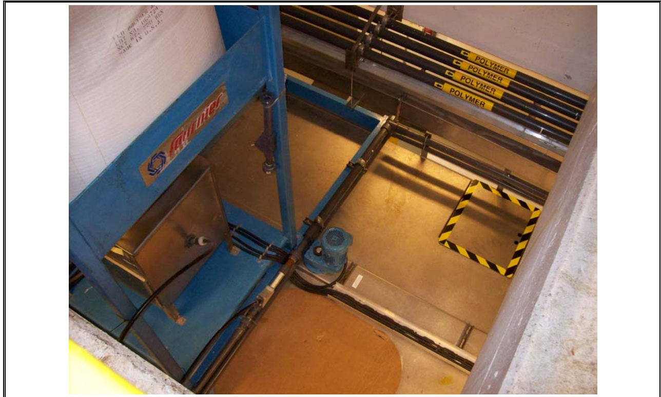
Photo 27 Halifax Densadeg Polymer Make-Up System
