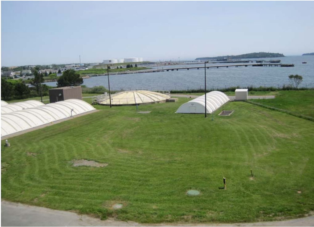
Photo 39 Eastern Passage Area Available for Expansion in Existing Fenced Area
