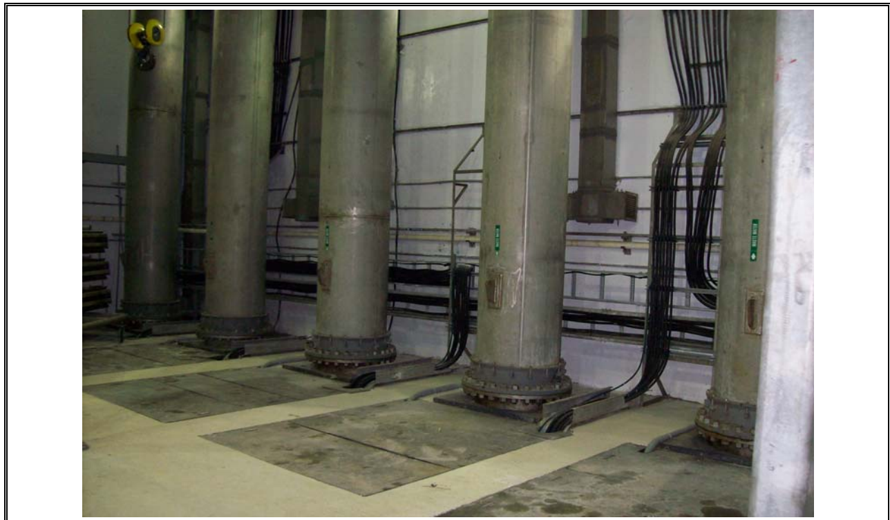
Photo 2 Halifax Influent Wet Well Below Slab and Pump Discharge Lines
