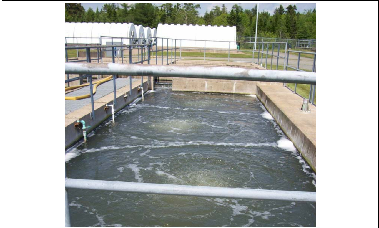
Photo 39 Post Aeration Tank
