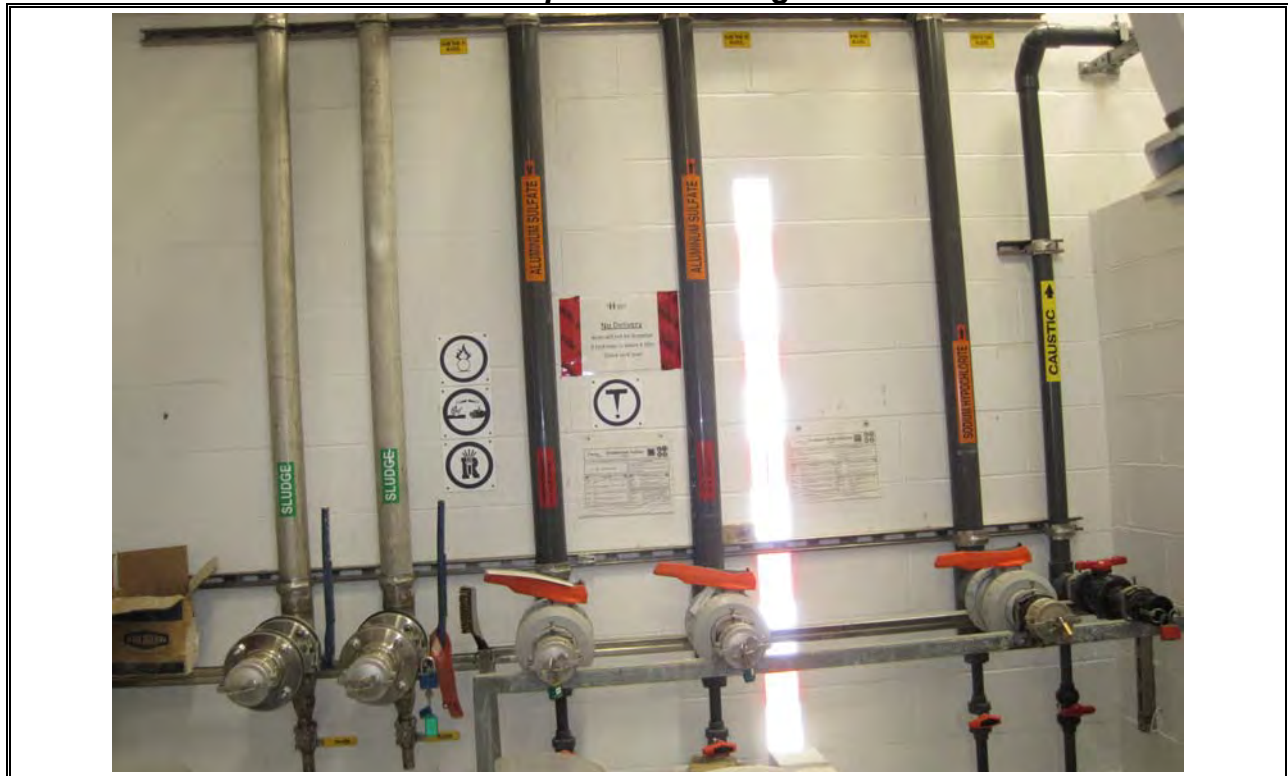
Photo 30 Dartmouth Chemical Piping – Alum, Caustic, Sodium Hypochlorite
