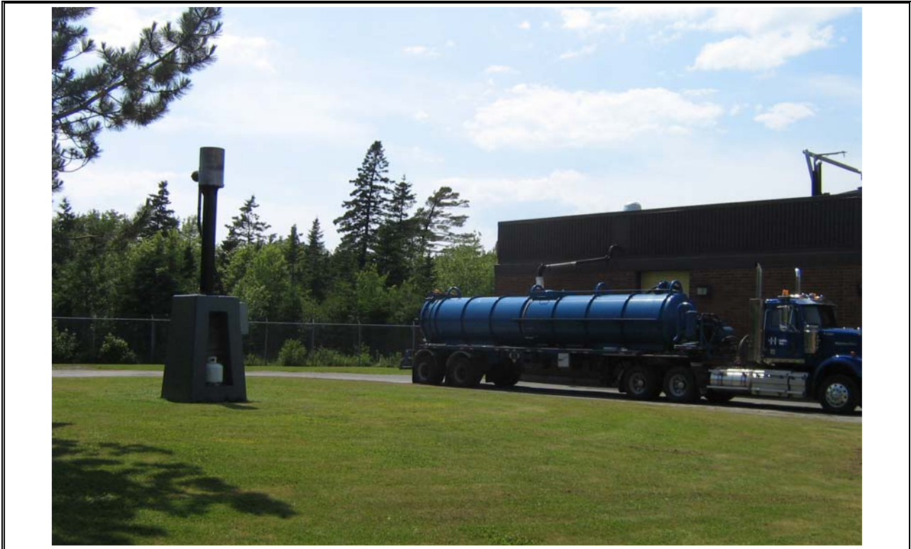
Photo 57 Sludge Loading Area and Flare Stack
