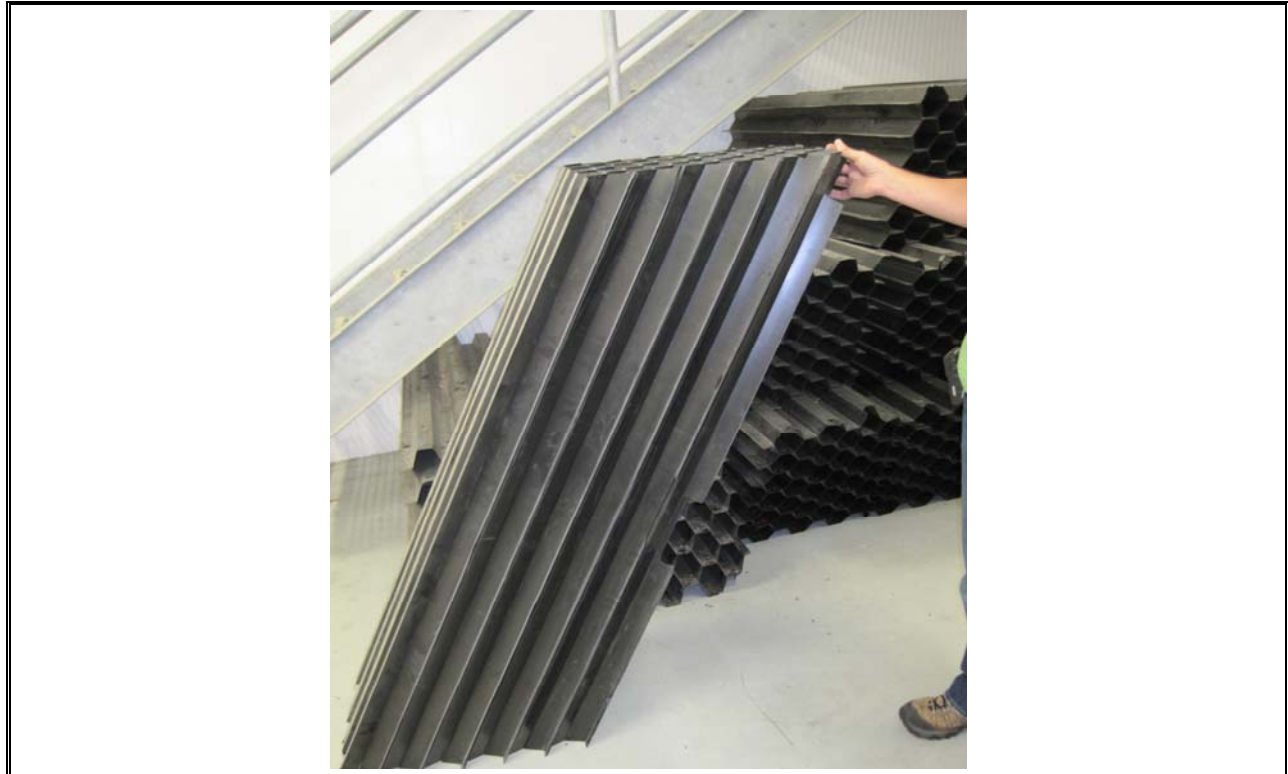
Photo 17 Herring Cove Inclined Tube Settlers Placed in Settling Zone of Densadeg
