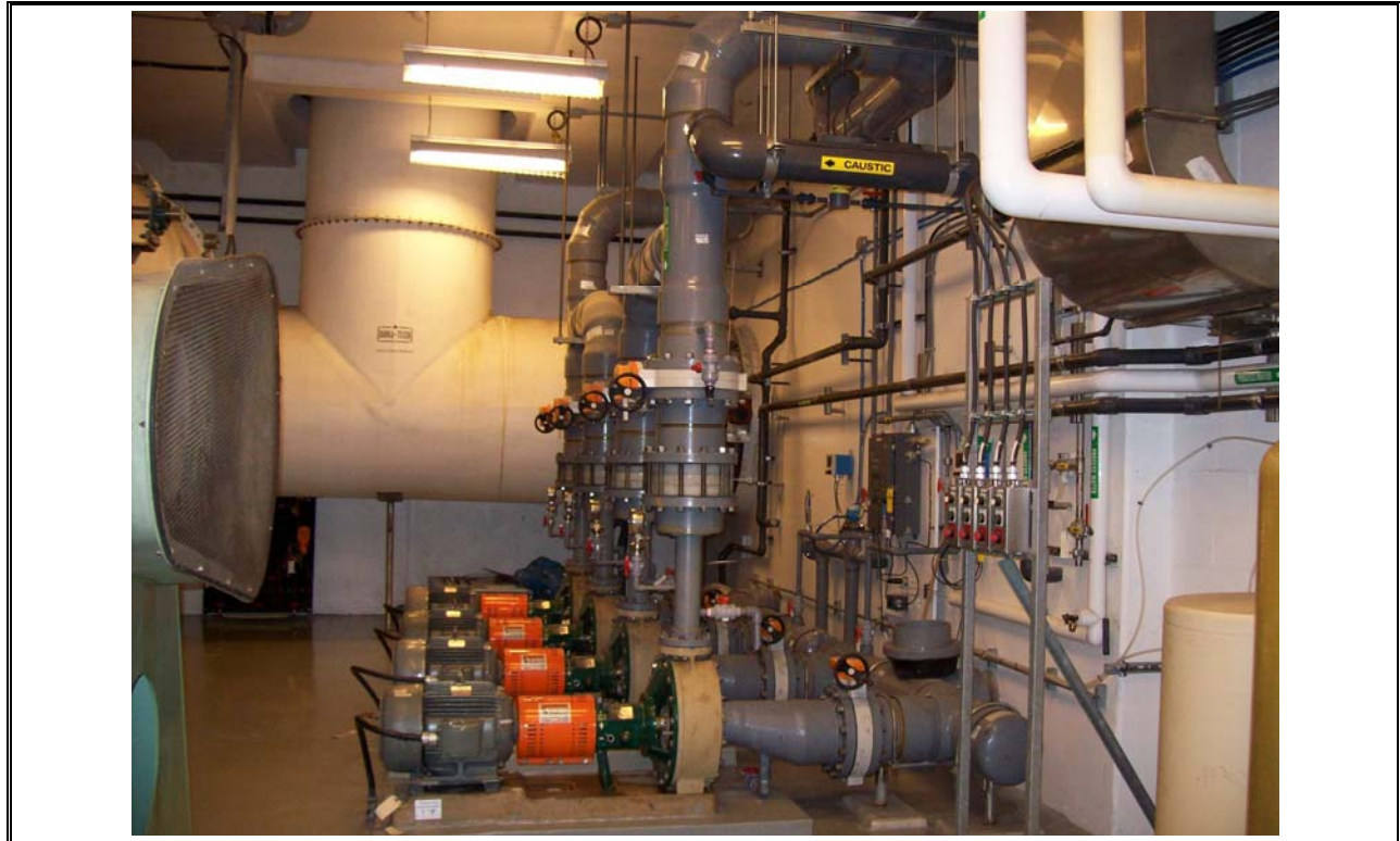
Photo 37 Halifax Odour Control Wet Scrubber Solution Pumps & Wet Scrubber
