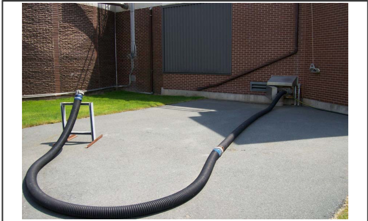
Photo 51 Sludge Truck Loading Area
