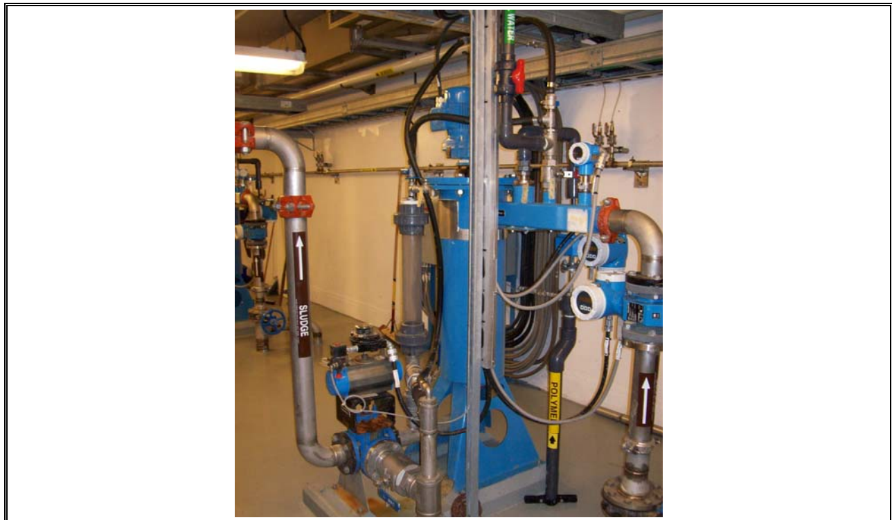
Photo 32 Halifax Sludge Flocculation Tank
