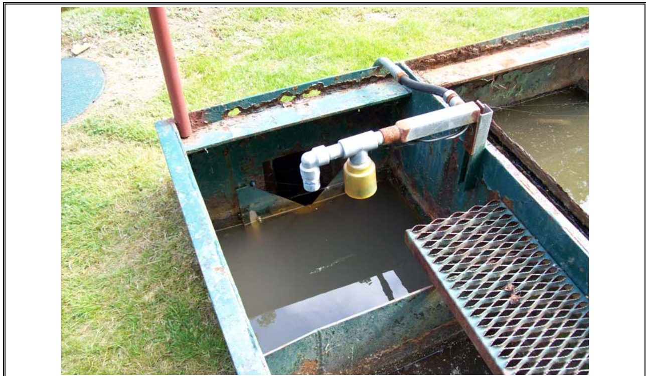
Photo 12 Wellington Effluent V-Notch Weir Flow Meter
