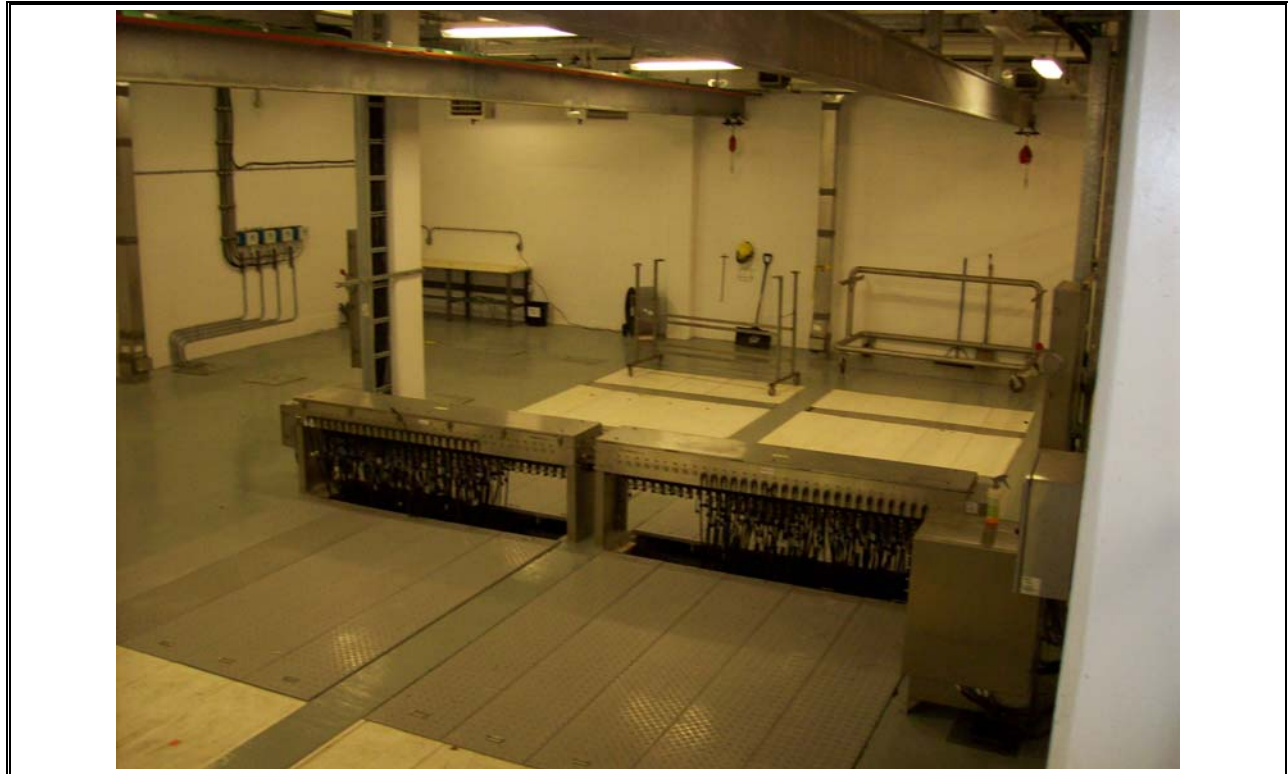
Photo 23 Halifax East UV Disinfection System
