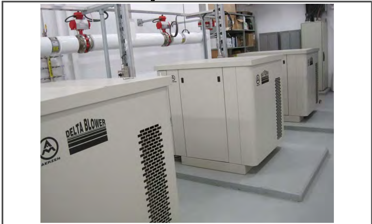
Photo 20 Dartmouth Blowers & Aeration Equipment
