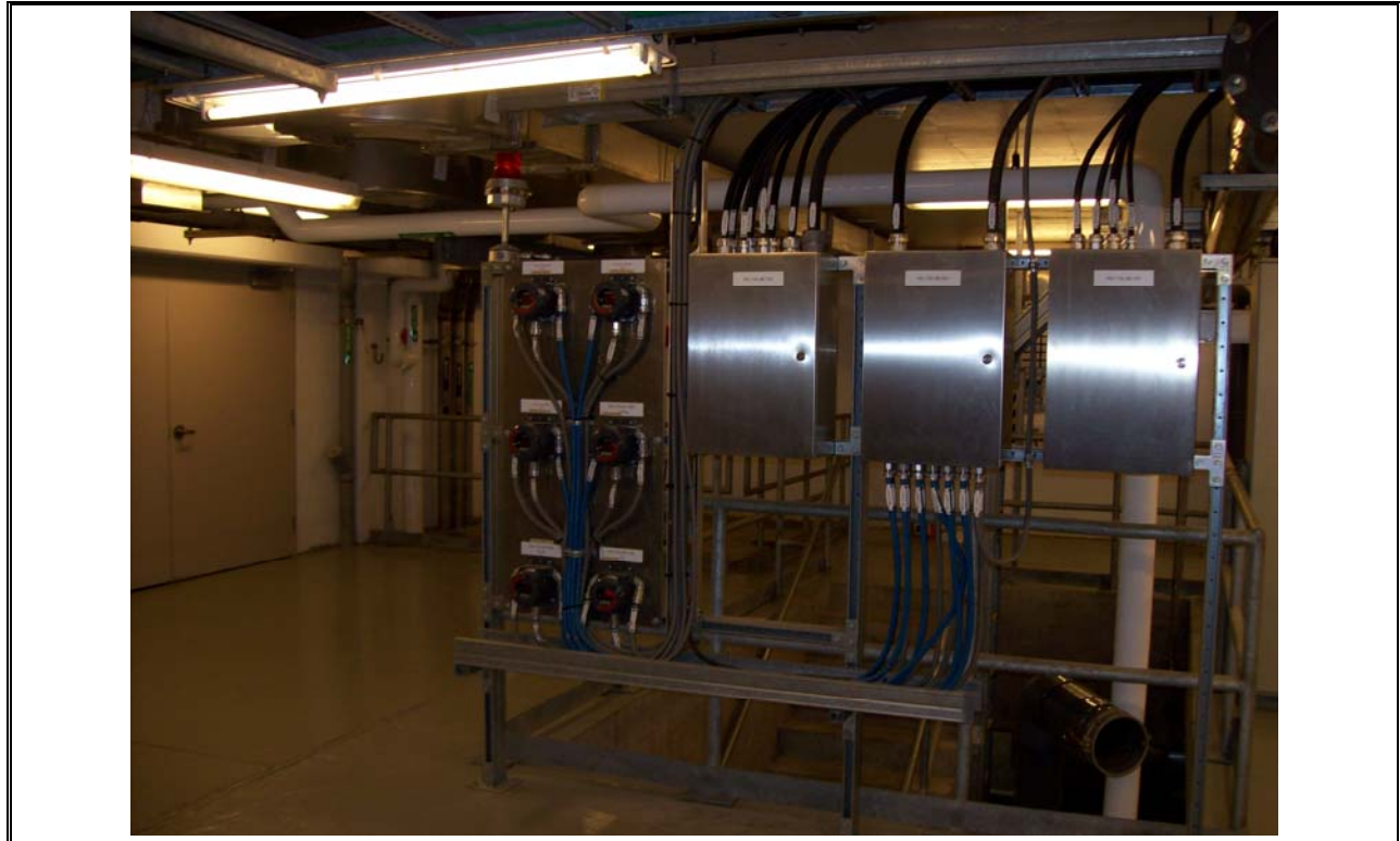
Photo 9 Halifax Influent PS Gas Detectors
