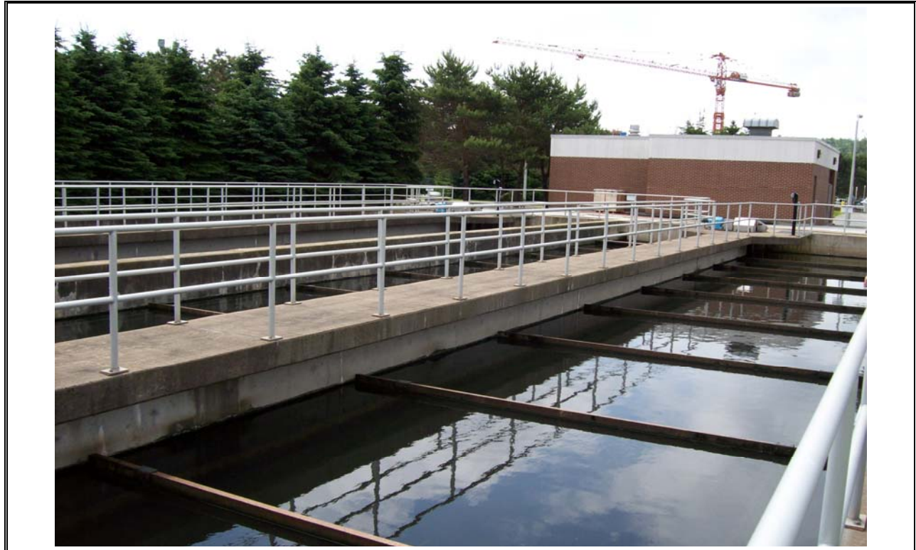
Photo 19 North Plant Rectangular Primary Clarifiers
