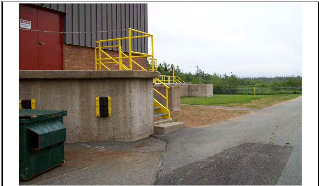
Photo 2 AeroTech Headworks Building and Equalization Tanks
