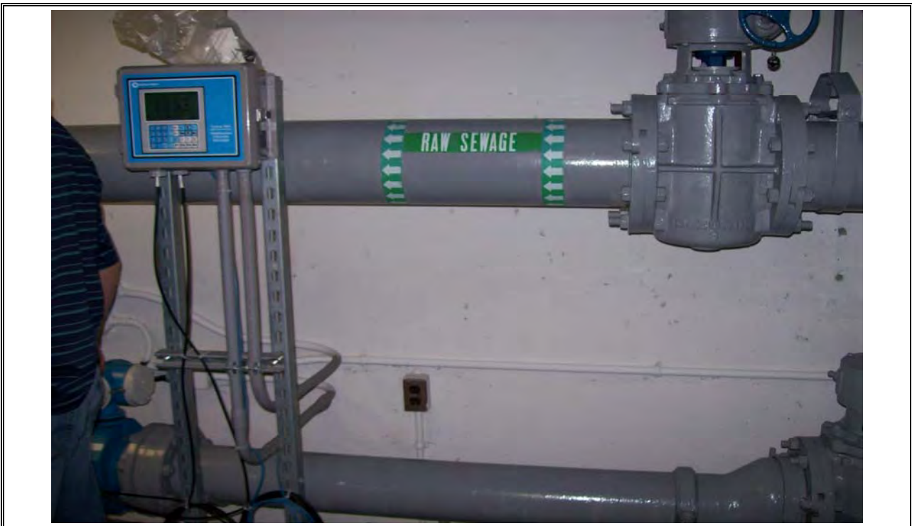
Photo 10 AeroTech Influent Wastewater Magmeter Control Panel
