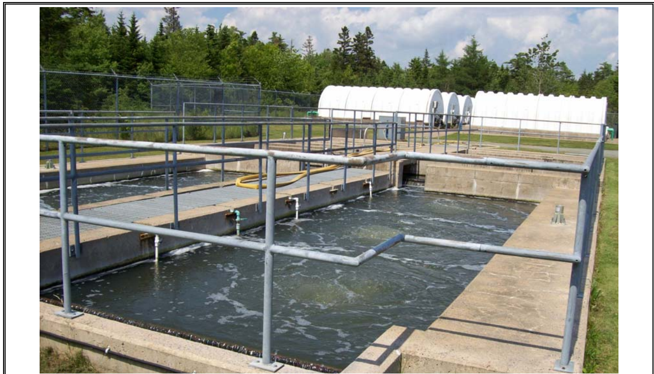
Photo 40 Post Aeration Tank
