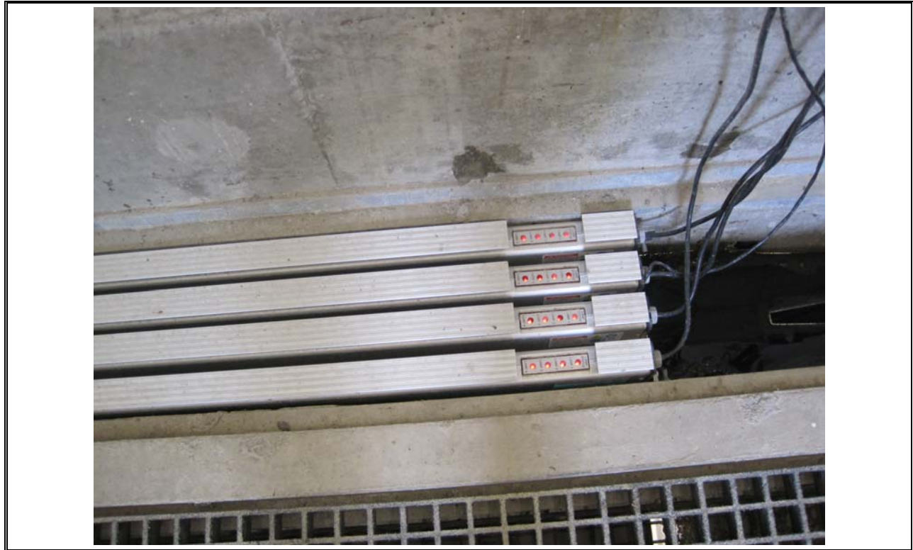
Photo 27 Uplands Park UV Disinfection – 4 Tubes x 4 Bulbs
