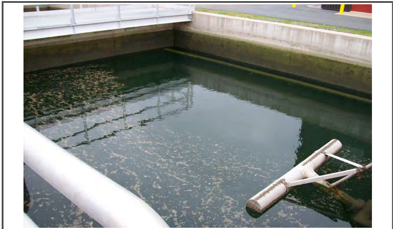
Photo 24 AeroTech SBR Decant Mechanism
