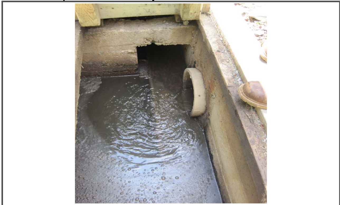
Photo 18 Uplands Park Secondary Clarification Uneven Flow Splitting
