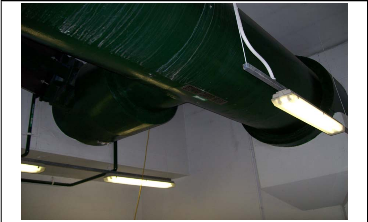
Photo 31 Secondary Clarifier Influent Piping
