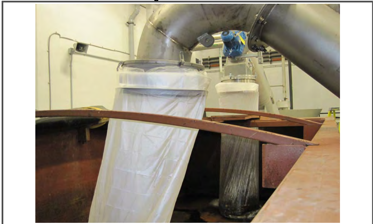
Photo 14 Dartmouth Screenings and Grit Collection
