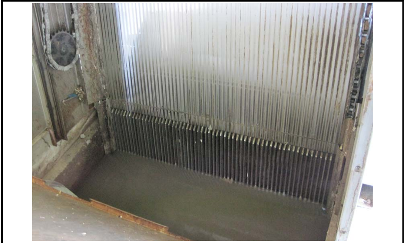
Photo 9 Eastern Passage Coarse Bar Screen
