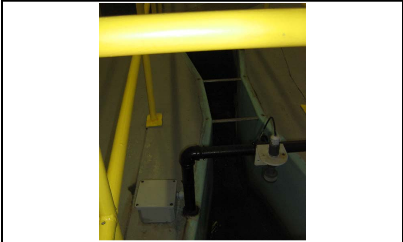
Photo 7 Parshall Flume Transducer
