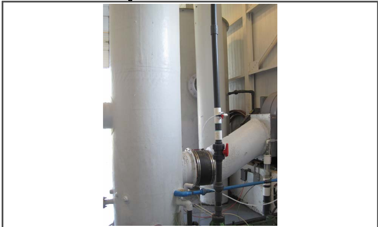
Photo 14 Eastern Passage Odour Control Wet Scrubber
