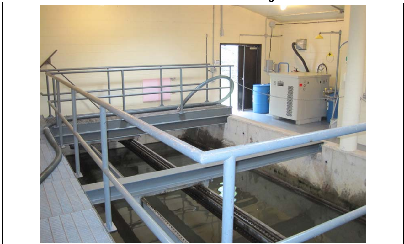
Photo 12 Secondary Clarifier and Blower
