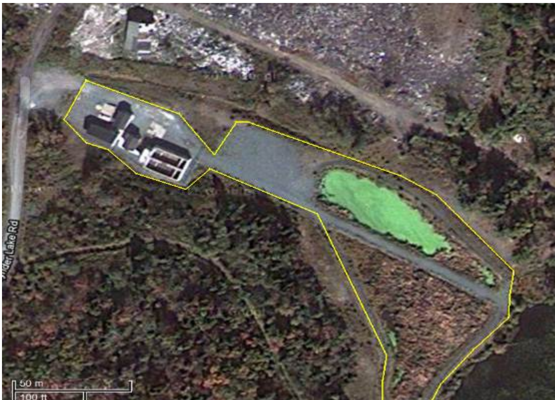
Figure 2.1 North Preston WWTF - Aerial View
