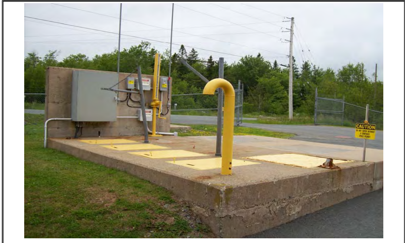
Photo 1 AeroTech Influent Pumping Station
