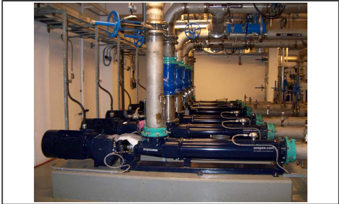
Photo 31 Halifax Sludge Pumps
