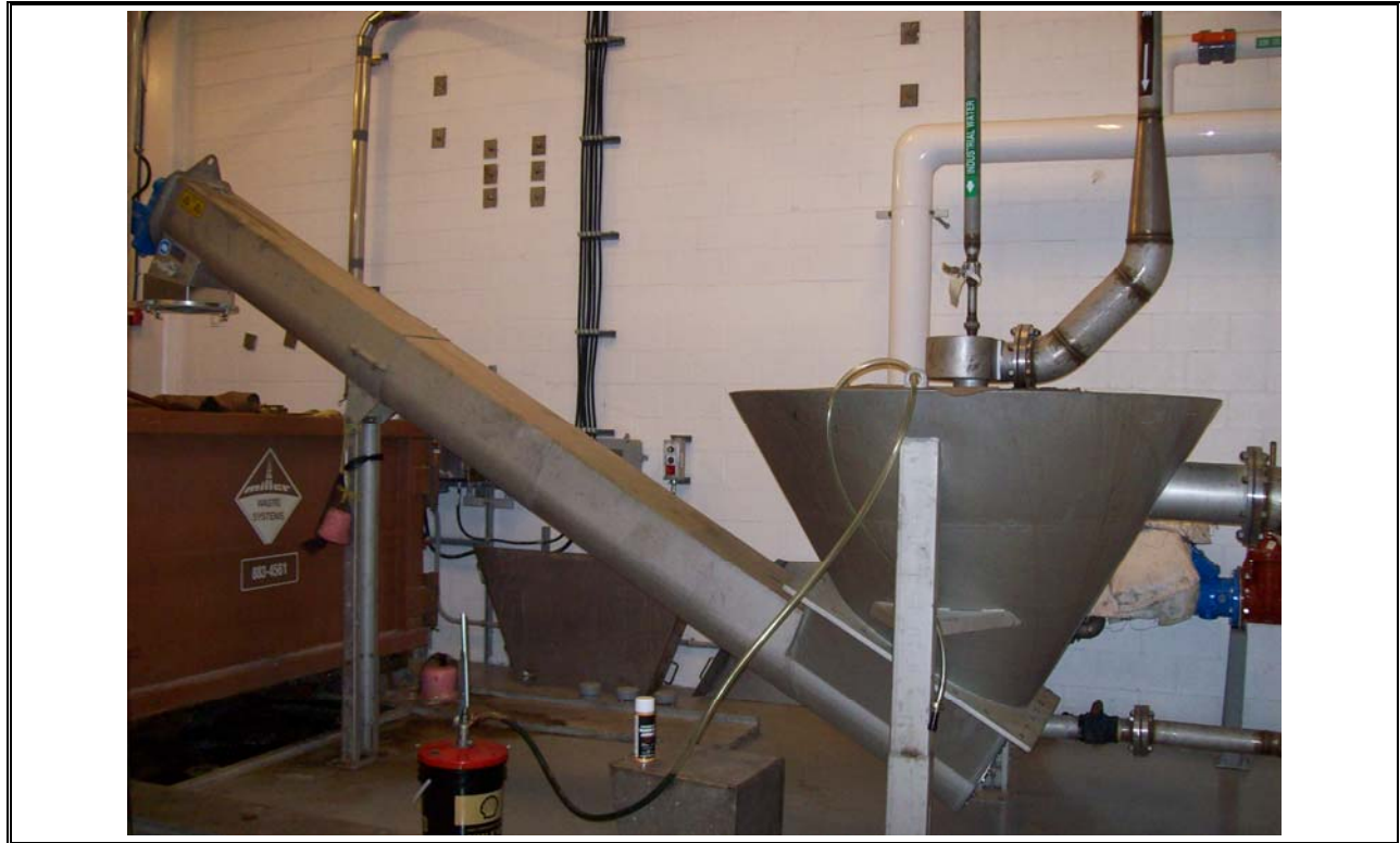
Photo 13 Halifax Grit Conveyor
