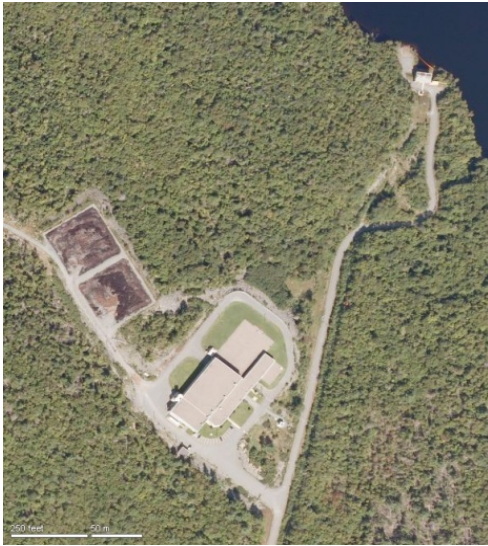
Figure 2.3 Lake Major Water Supply Plant - Aerial View
