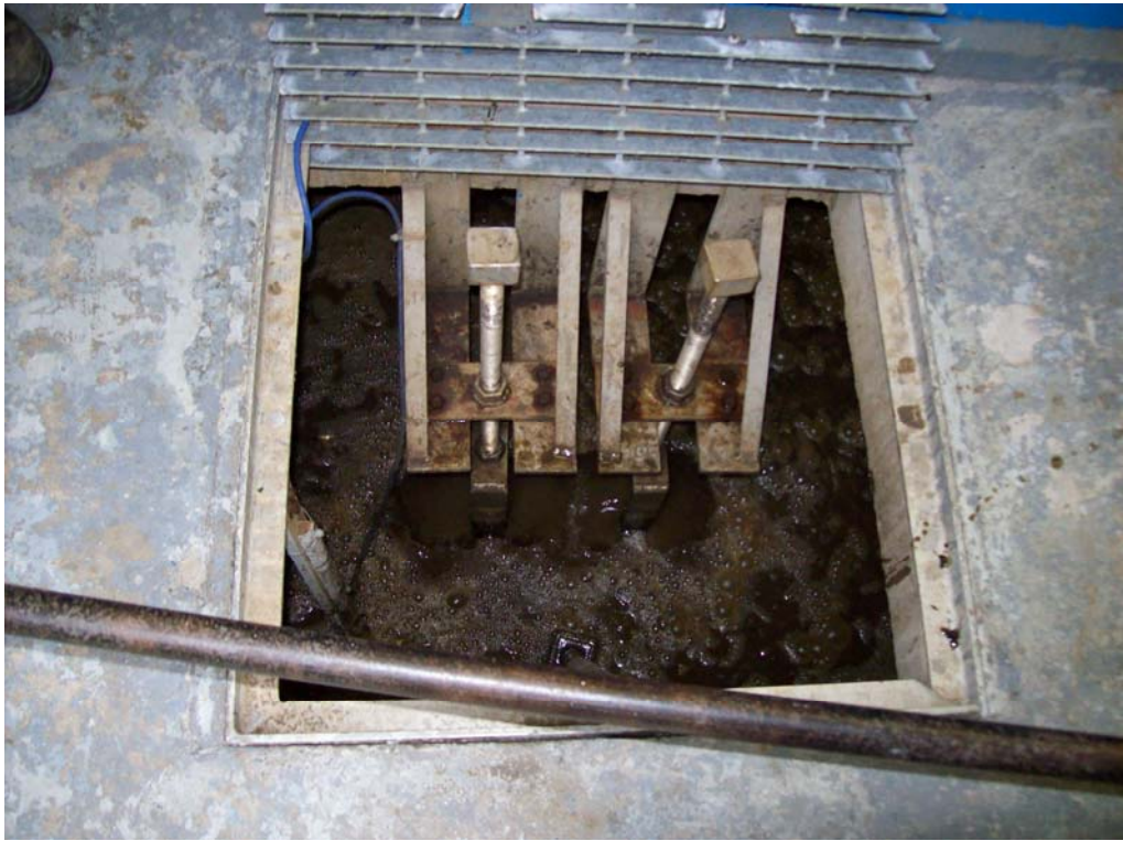
Photo 17 Lockview RAS Tank
