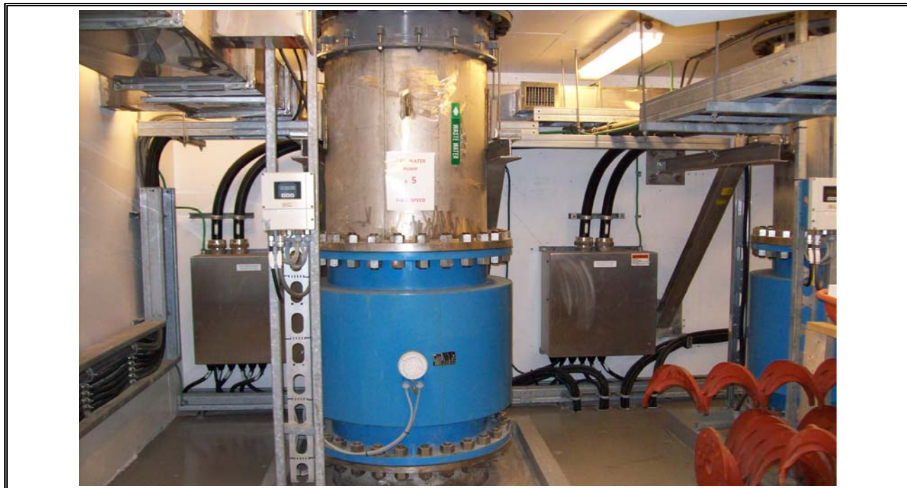
Photo 10 Halifax Raw Wastewater Magmeter on Raw Pump Discharge Line (typ)
