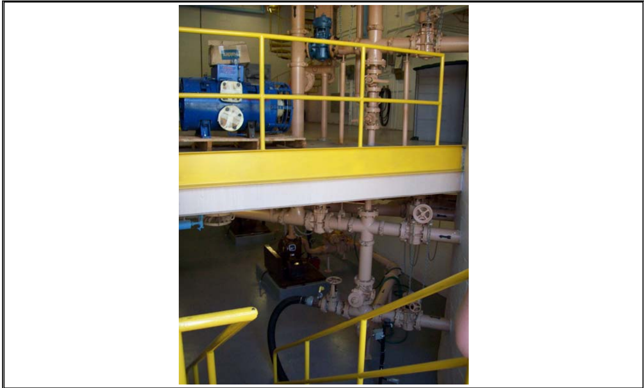
Photo 59 Digester Pipes for Mixing Sludge within Digester
