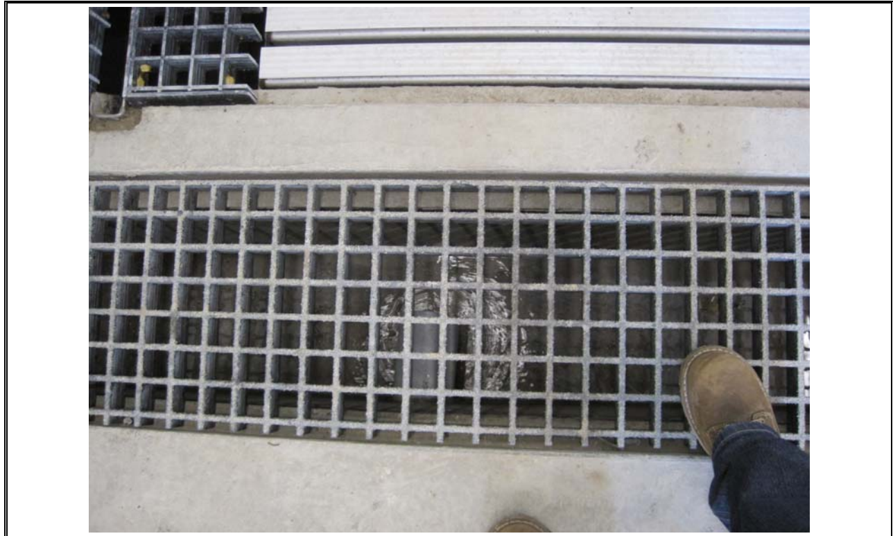
Photo 25 Uplands Park Bypass Line with Groundwater entering the Channel
