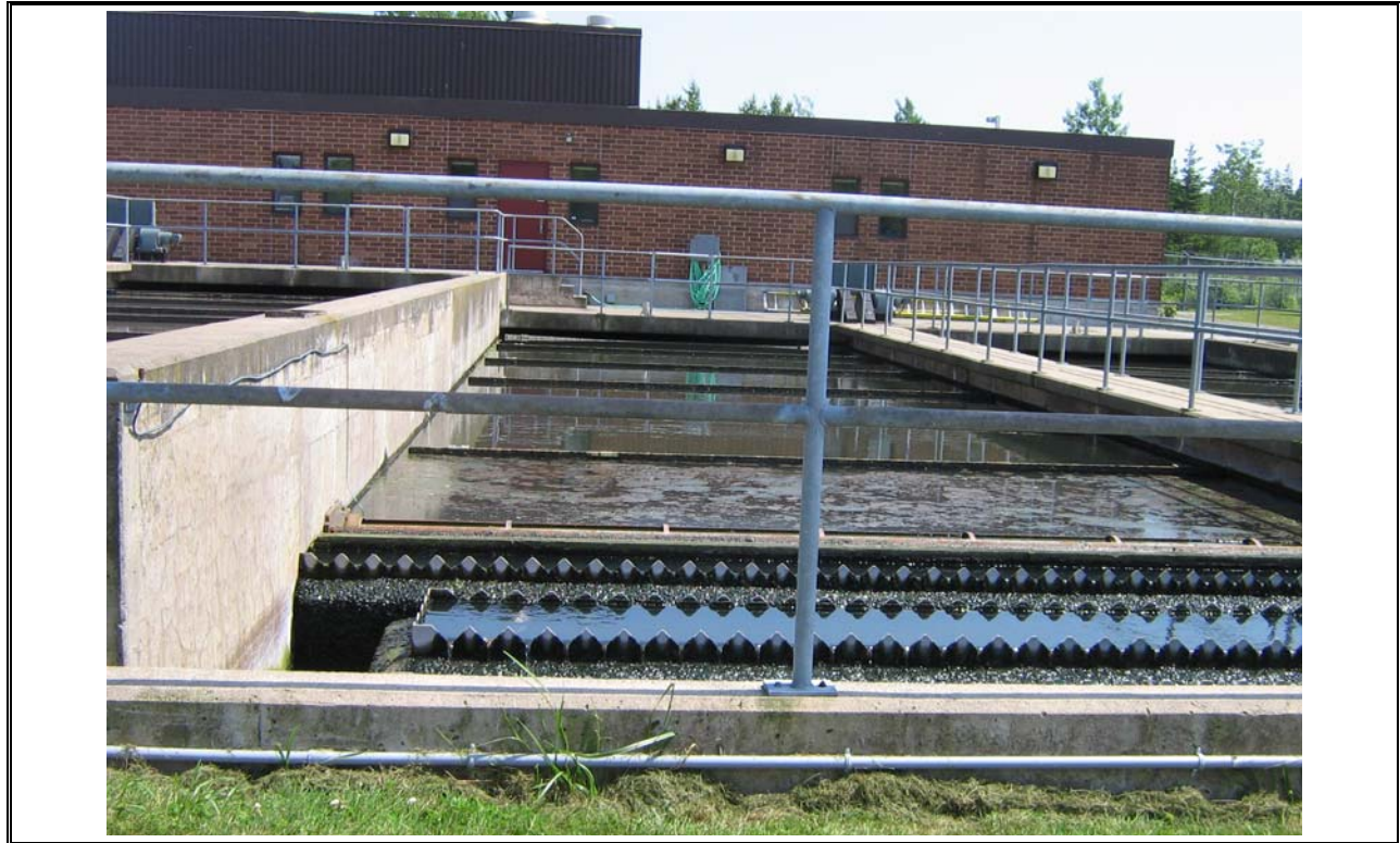
Photo 33 Secondary Clarifier Weirs and Effluent
