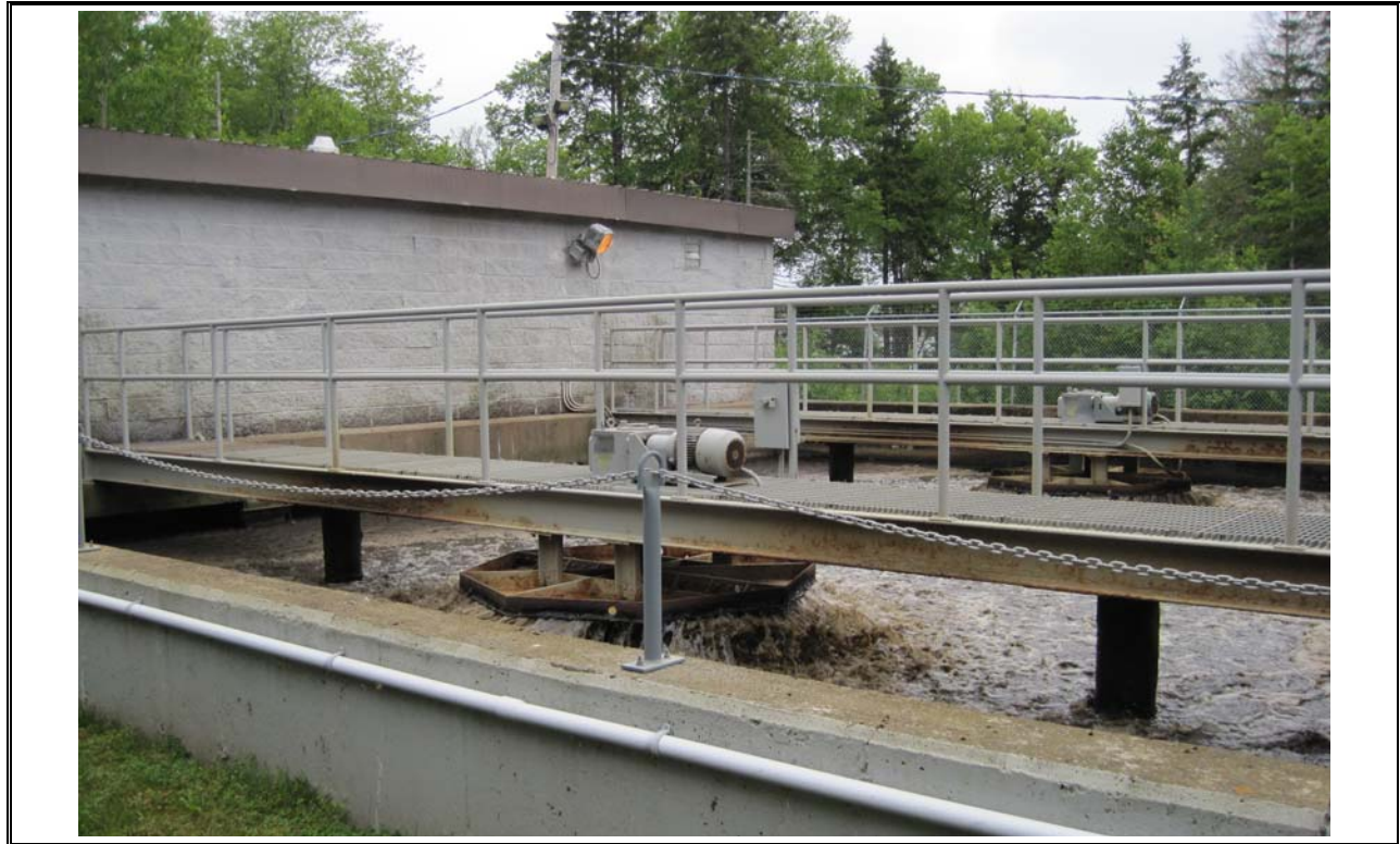
Photo 7 Mechanical Surface Aerators
