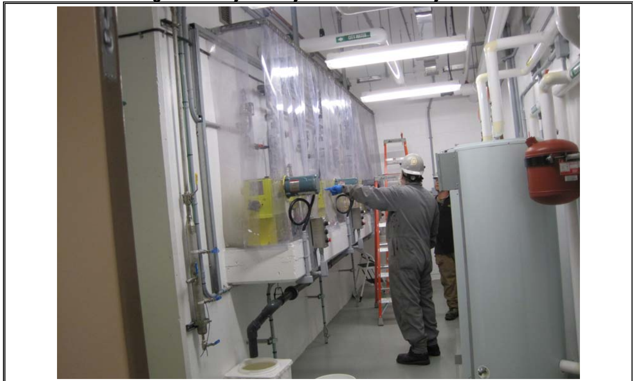
Photo 32 Herring Cove Chemical Metering
