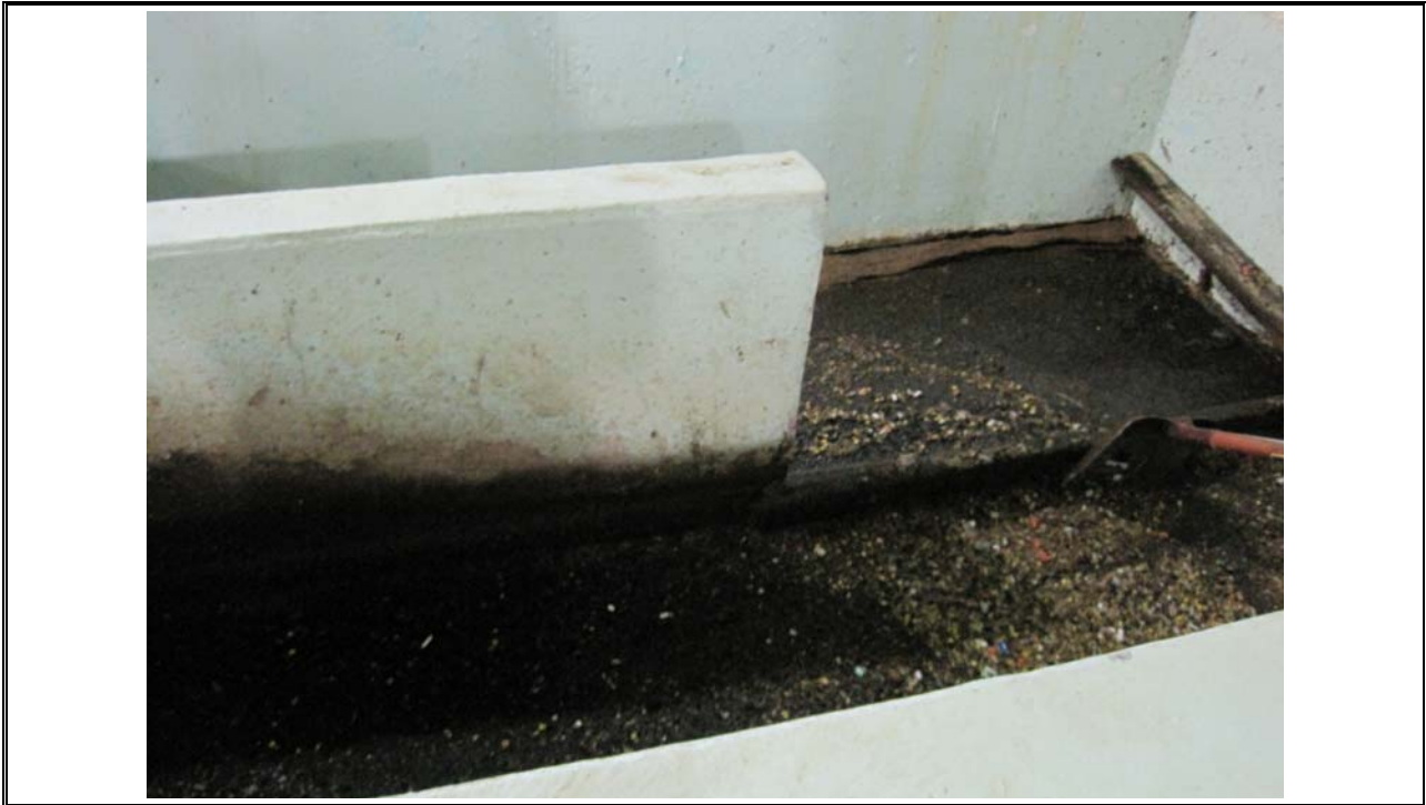
Photo 11 Eastern Passage Grit Removal Tank
