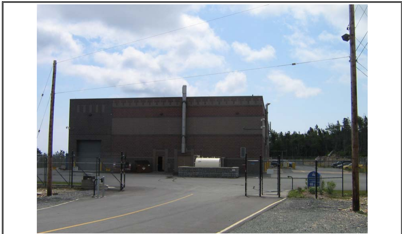
Photo 52 Herring Cove WWTP & Diesel Storage for Back-up Power
