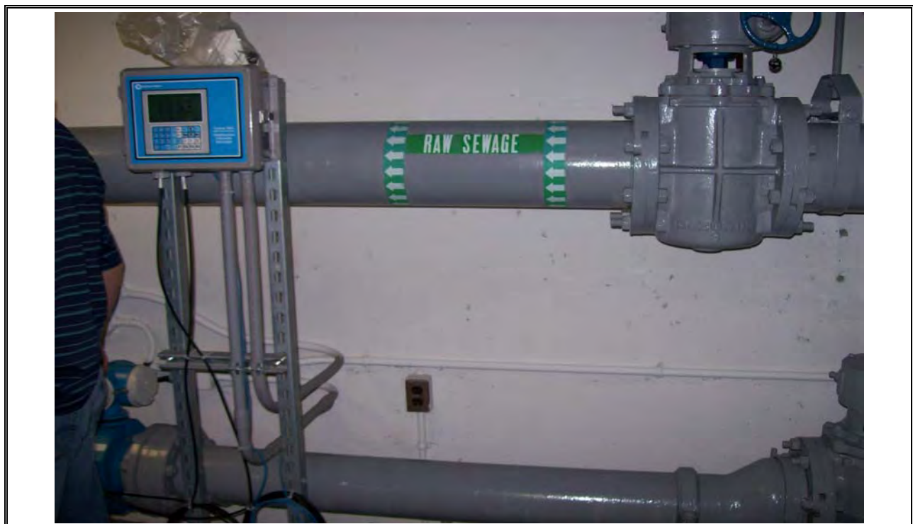
Photo 10 AeroTech Influent Wastewater Magmeter Control Panel
