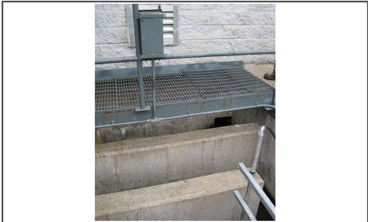
Photo 18 Chlorine Contact Tank
