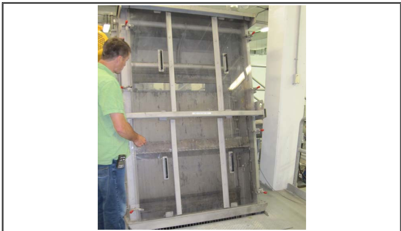
Photo 4 Herring Cove Automatic Coarse Bar Screen
