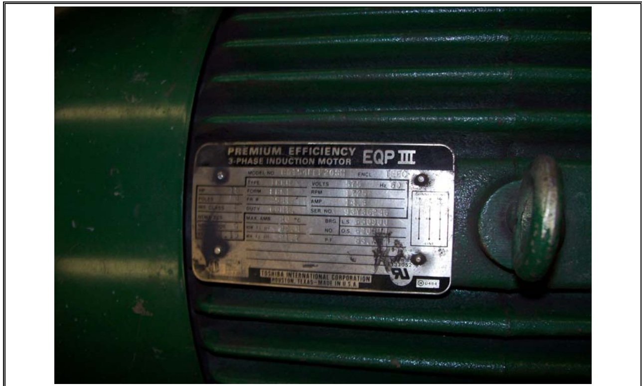
Photo 10 Lockview Blower Motor Nameplate
