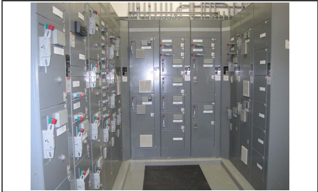
Photo 13 Herring Cove Headworks MCC Room
