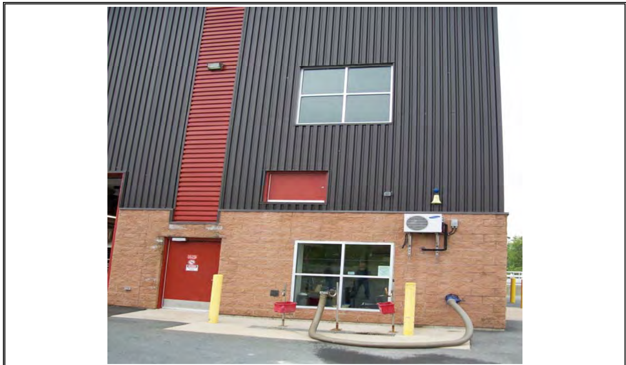
Photo 38 AeroTech Sludge Building
