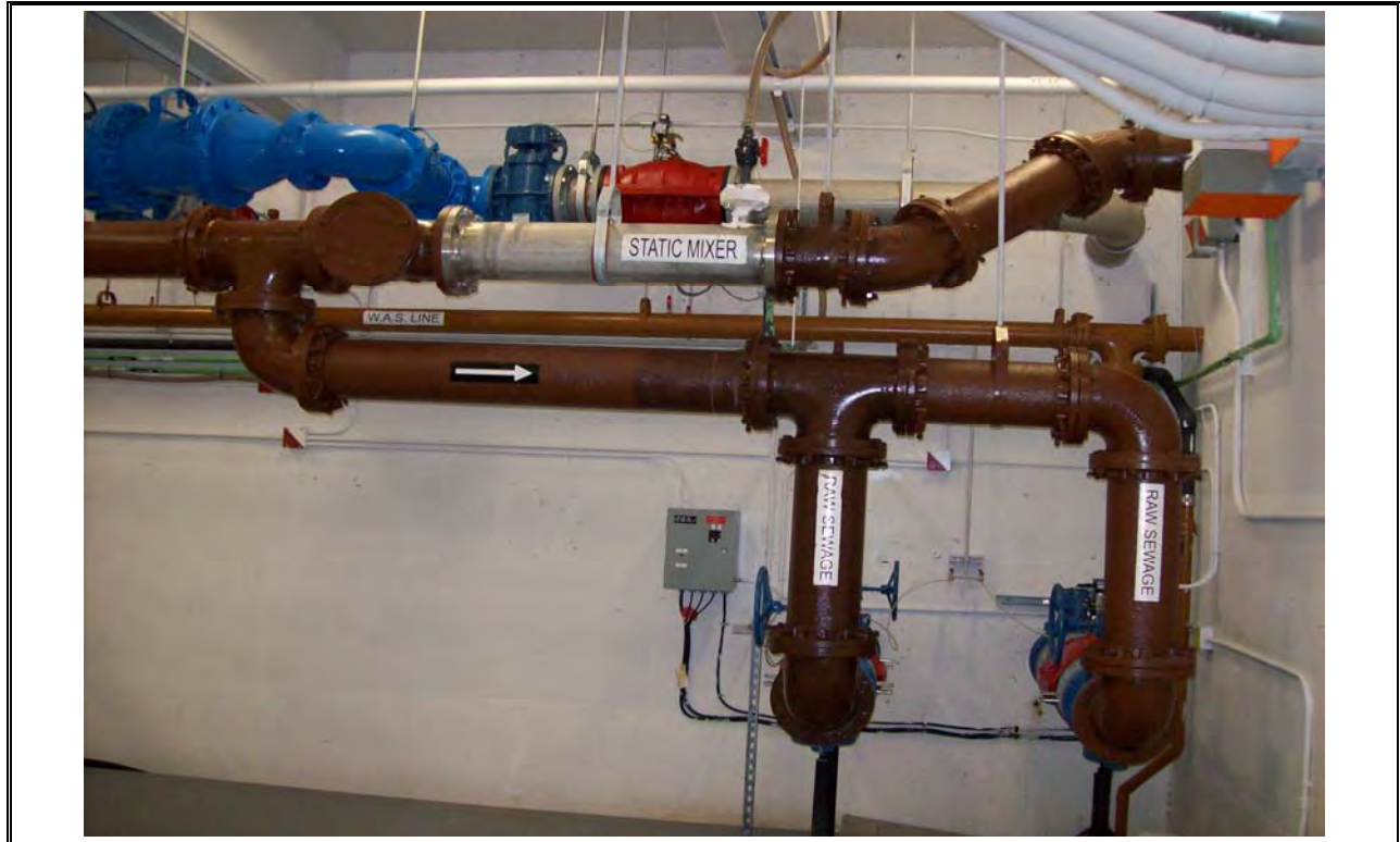
Photo 19 AeroTech Caustic Injection Point and Flash Mixer
