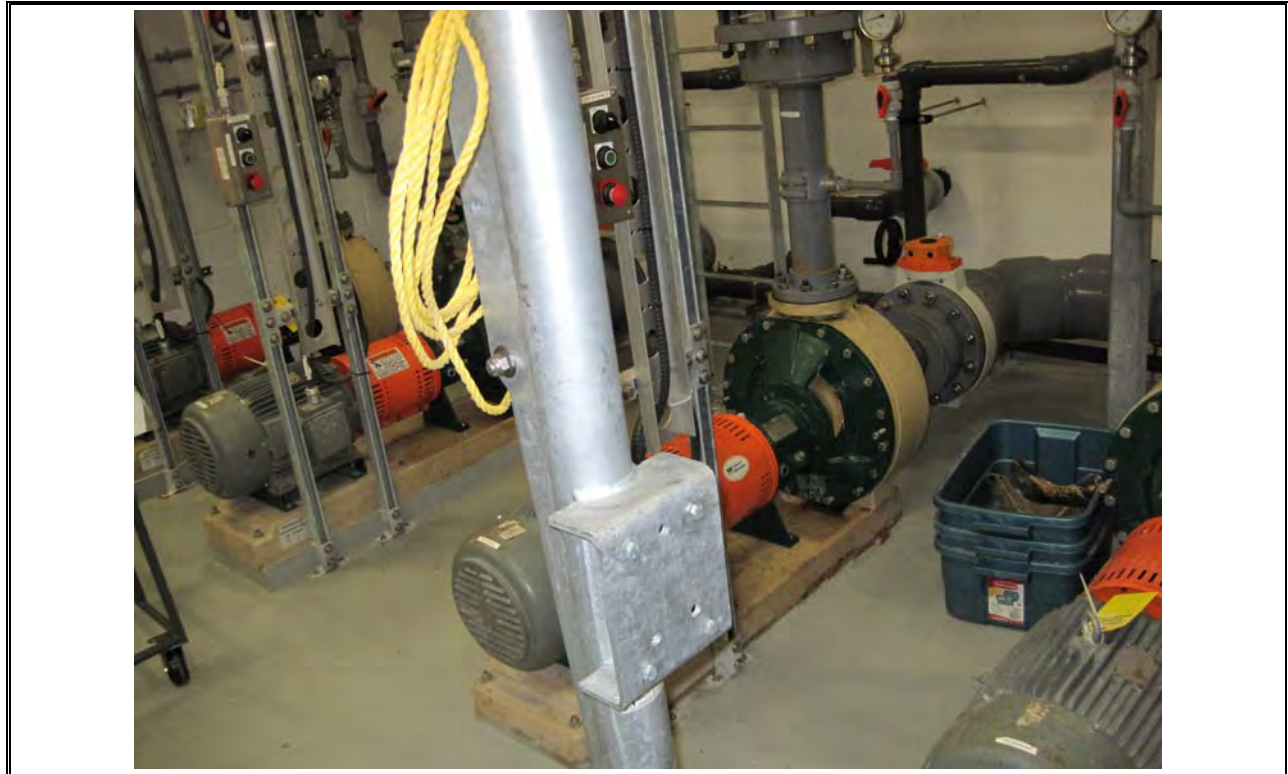
Photo 43 Dartmouth Odour Control Wet Scrubber Solution Pumps
