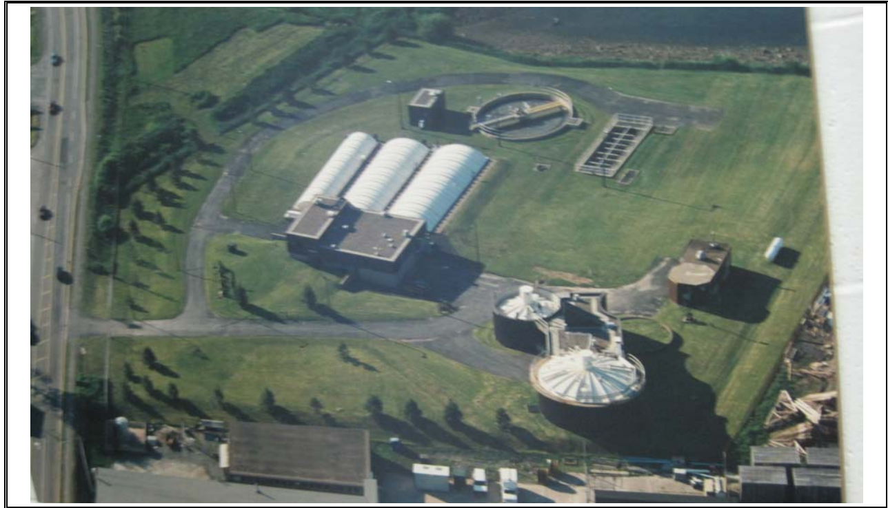
Photo 1 Eastern Passage Site Layout – Aerial View
