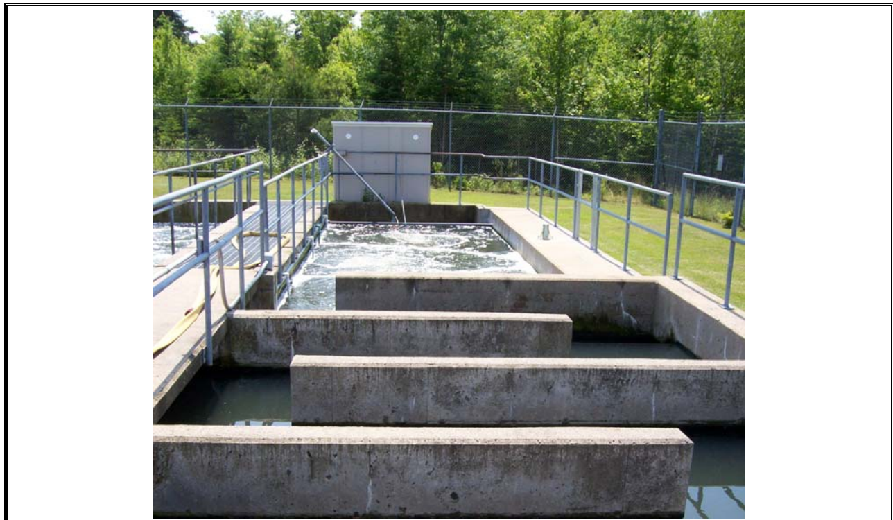
Photo 38 BLT Effluent Flows from Chlorination to Post Aeration
