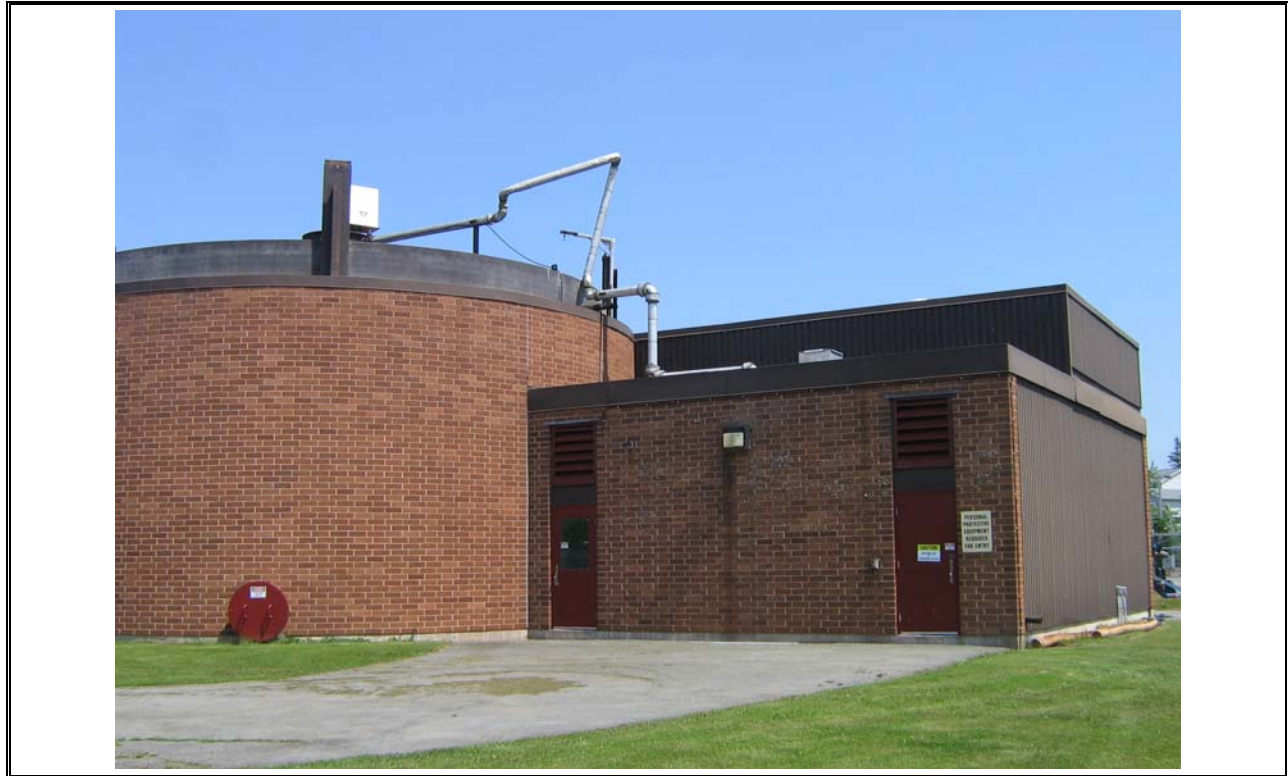
Photo 55 Anaerobic Digester and Building
