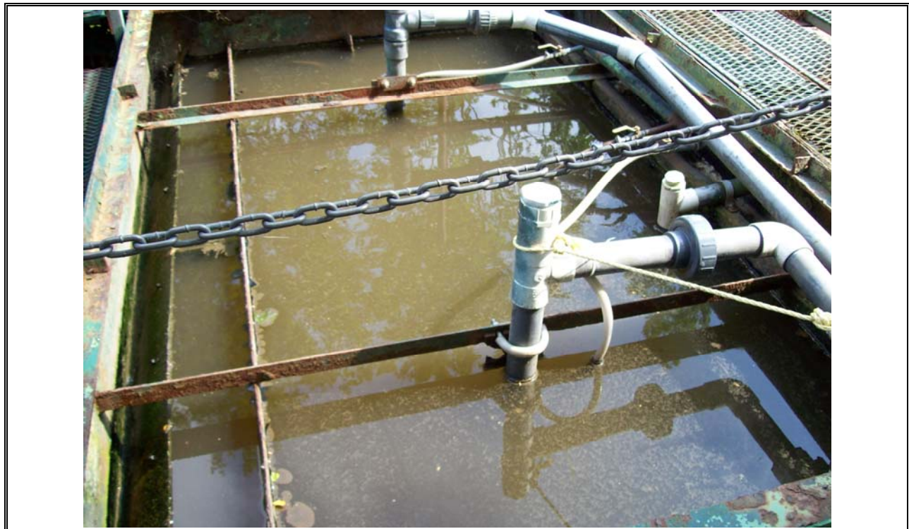
Photo 8 Wellington Secondary Clarifier and RAS Lines
