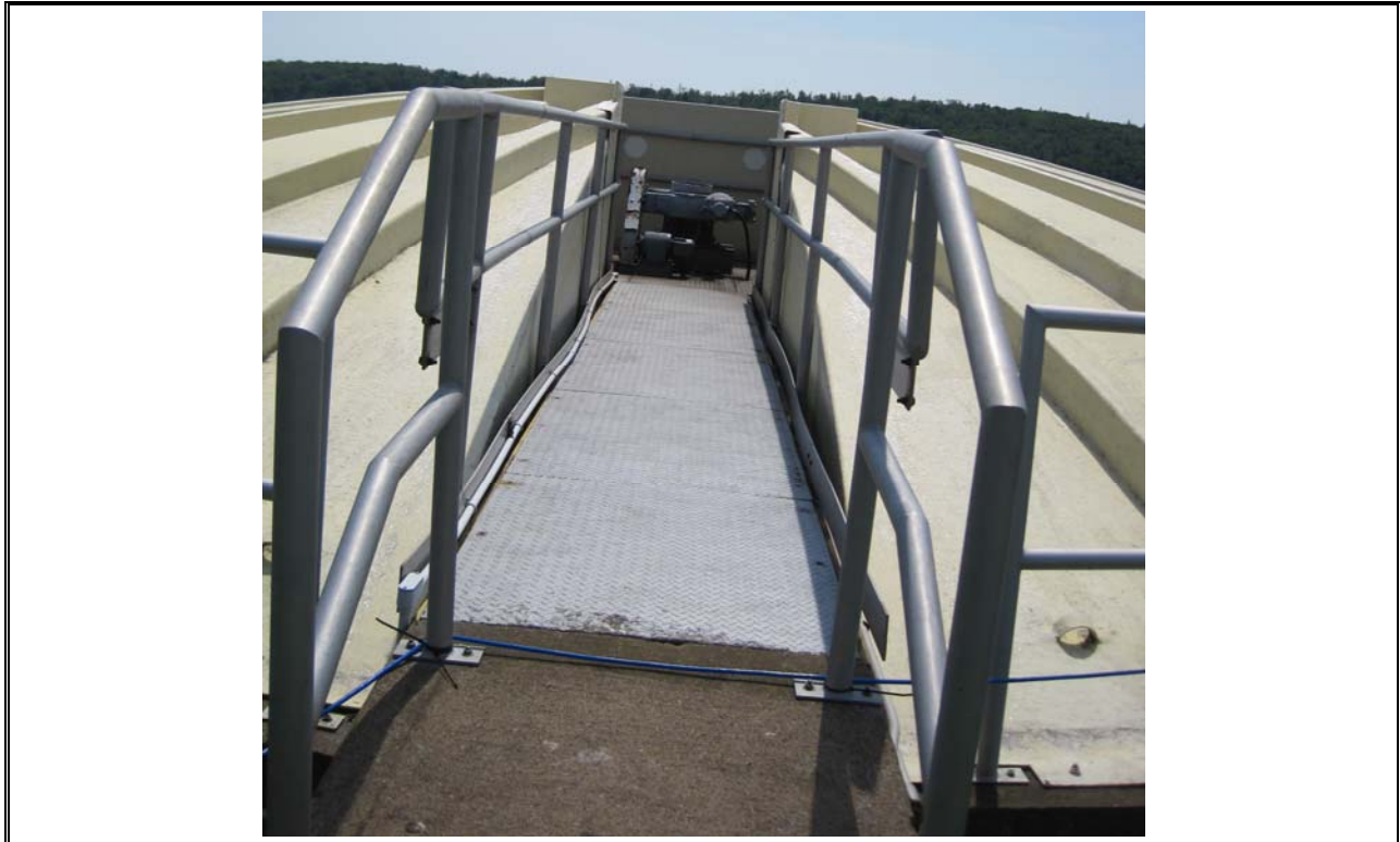
Photo 21 Eastern Passage Circular Chlorine Contact Chamber
