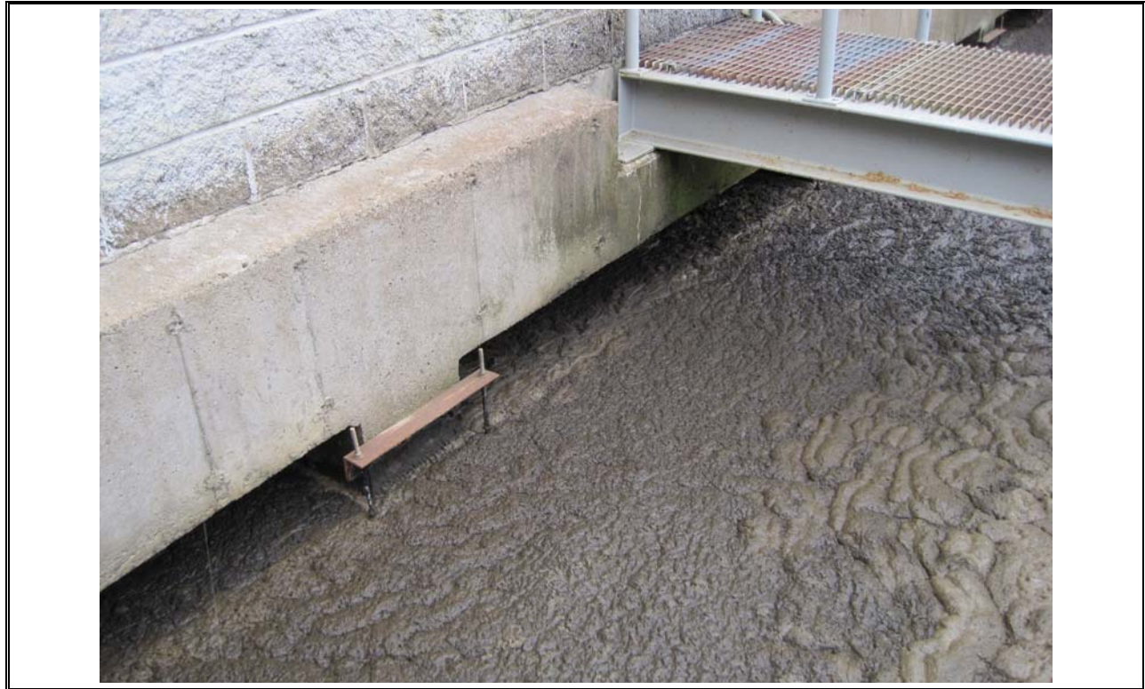
Photo 9 Aeration Tank Effluent to Secondary Clarifier
