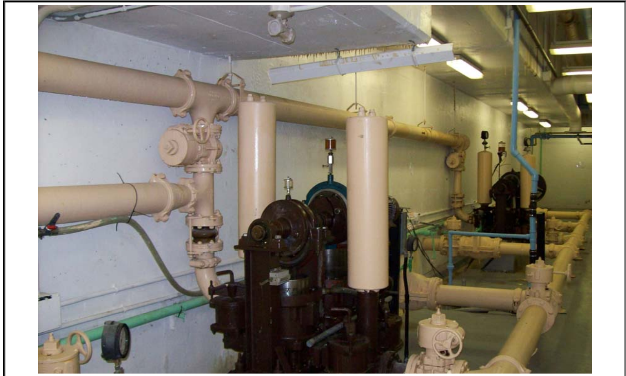
Photo 53 Primary Sludge Pumping System Located in Headworks Building
