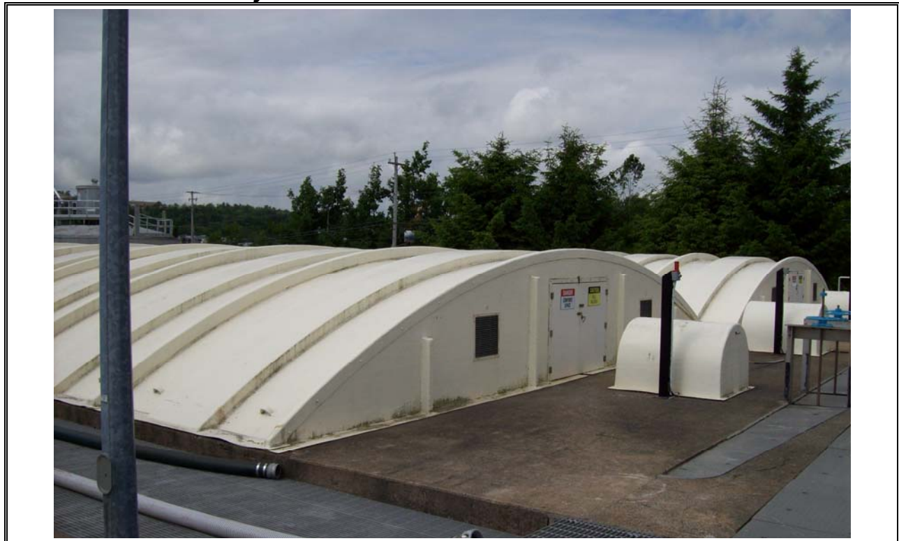
Photo 34 Secondary Covered Clarifiers
