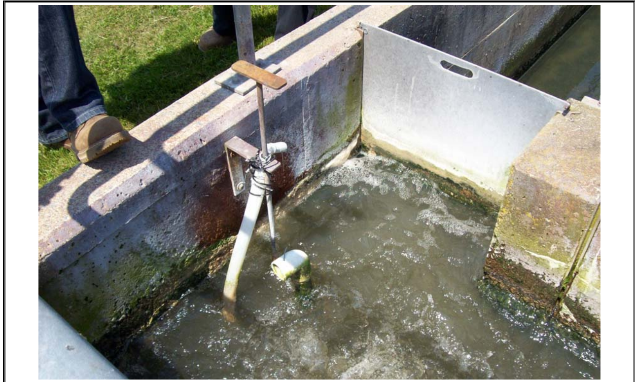
Photo 29 Alum Dosage Point and Flash Mixing
