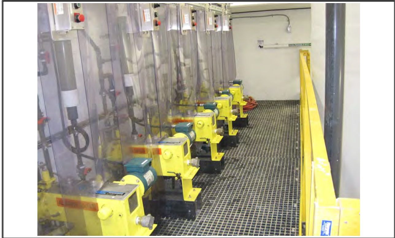
Photo 29 Dartmouth Alum Pumps and Metering
