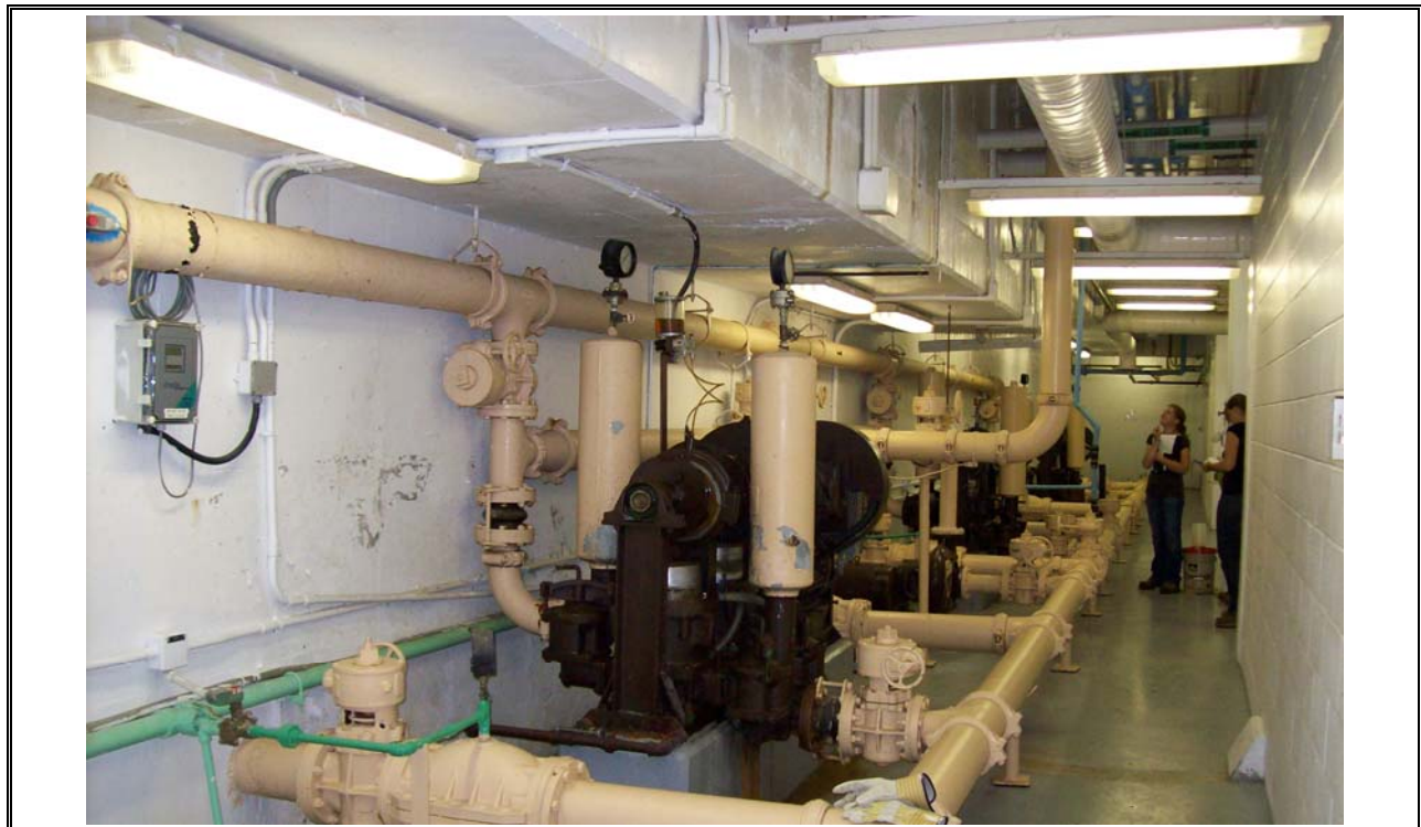
Photo 54 Primary and Secondary Sludge Pumping Systems
