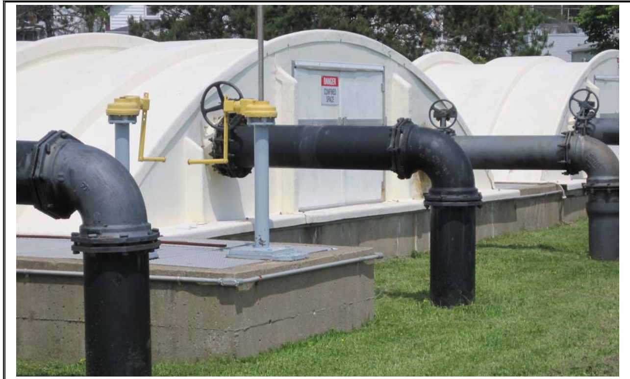
Photo 23 Eastern Passage Rectangular Chlorine Contact Tank
