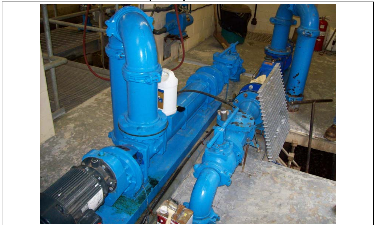
Photo 22 Lockview RAS Pumps
