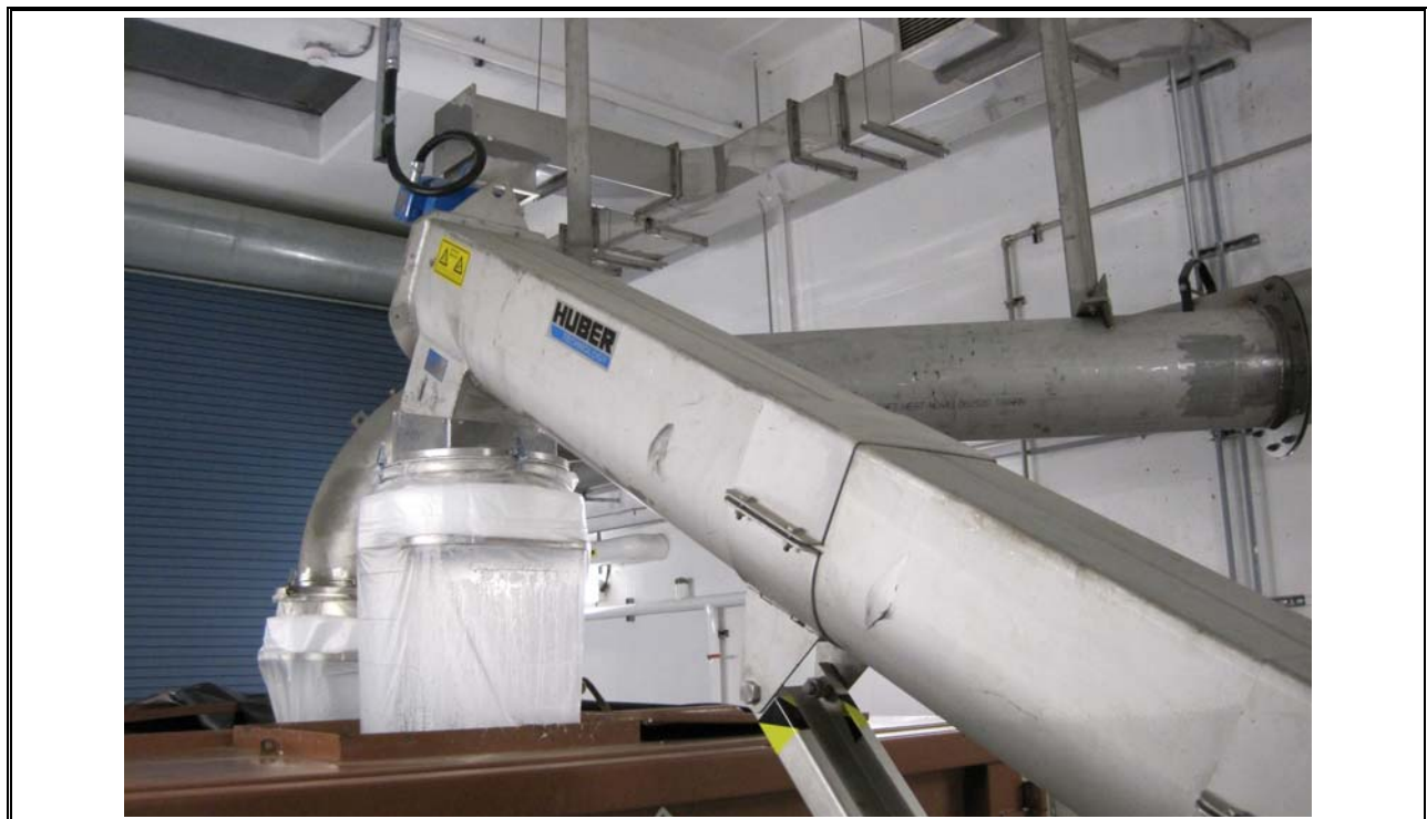
Photo 12 Herring Cove Screenings and Grit Disposal Bin
