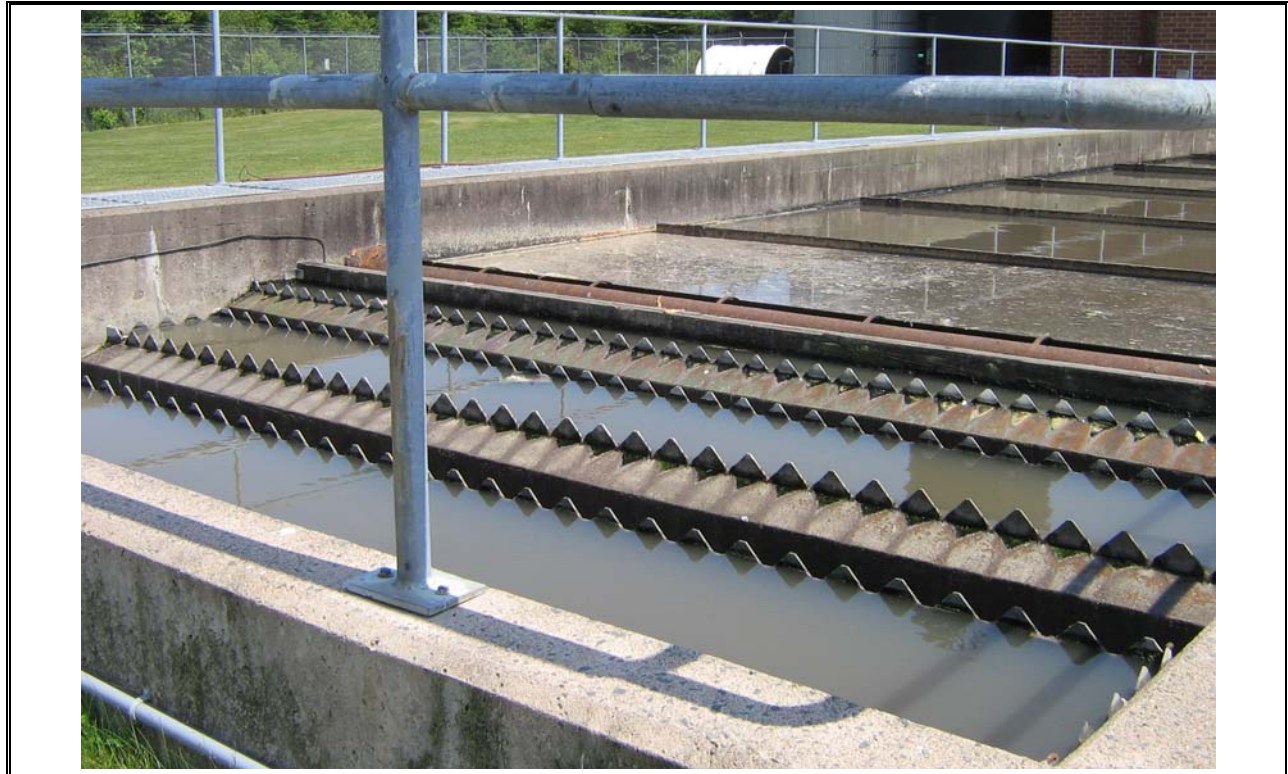
Photo 17 Primary Clarifier Effluent Wiers
