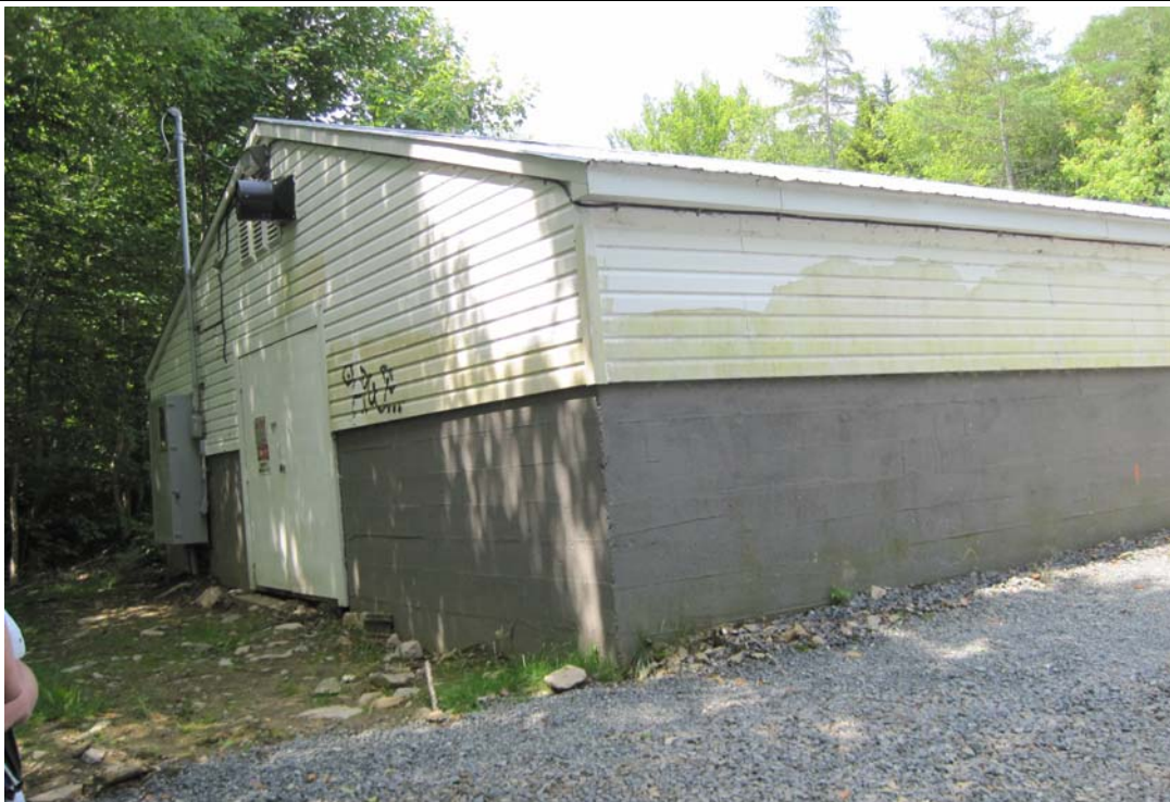
Photo 8 Uplands Park Trickling Filter Building
