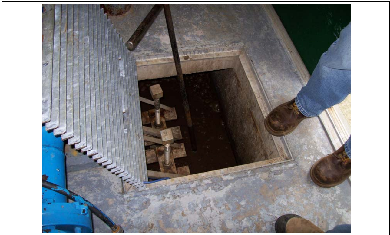
Photo 19 Lockview Hatch to RAS Tank
