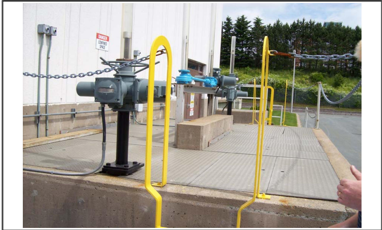
Photo 13 Primary Influent Splitter Box
