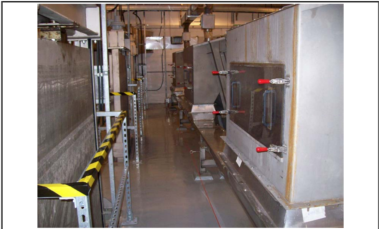
Photo 12 Halifax Fine Screens and Screenings Conveyor
