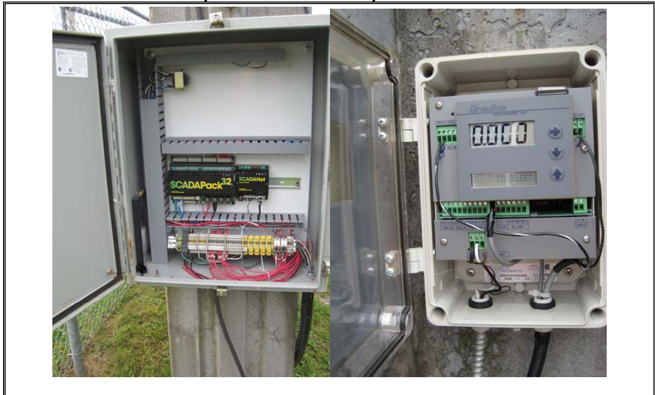
Photo 15 SCADA System panels
