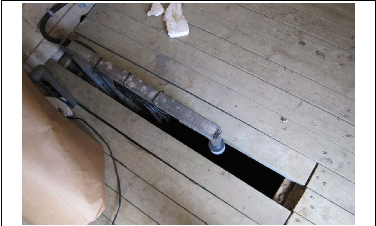
Photo 21 Uplands Park Transducer in Old Chlorination Building
