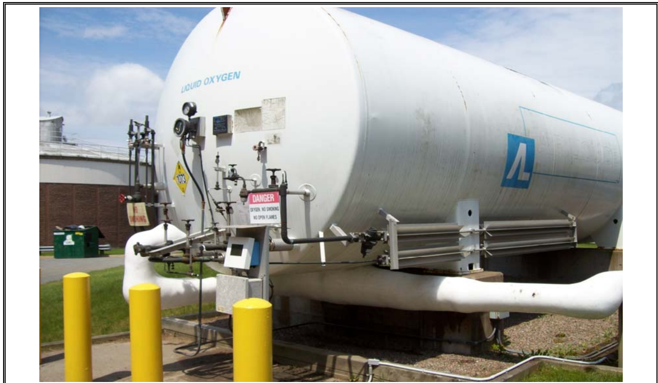
Photo 26 Oxygen Storage Tank
