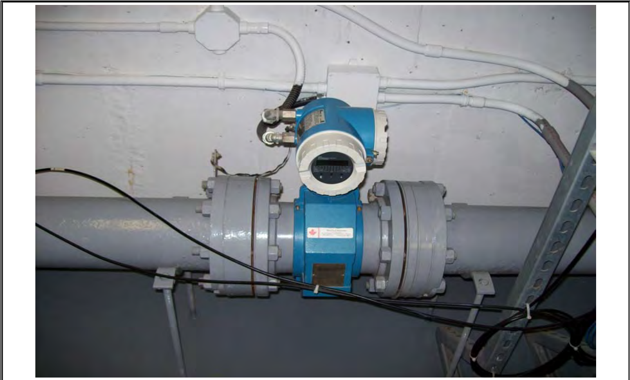
Photo 9 AeroTech Influent Wastewater Magmeter
