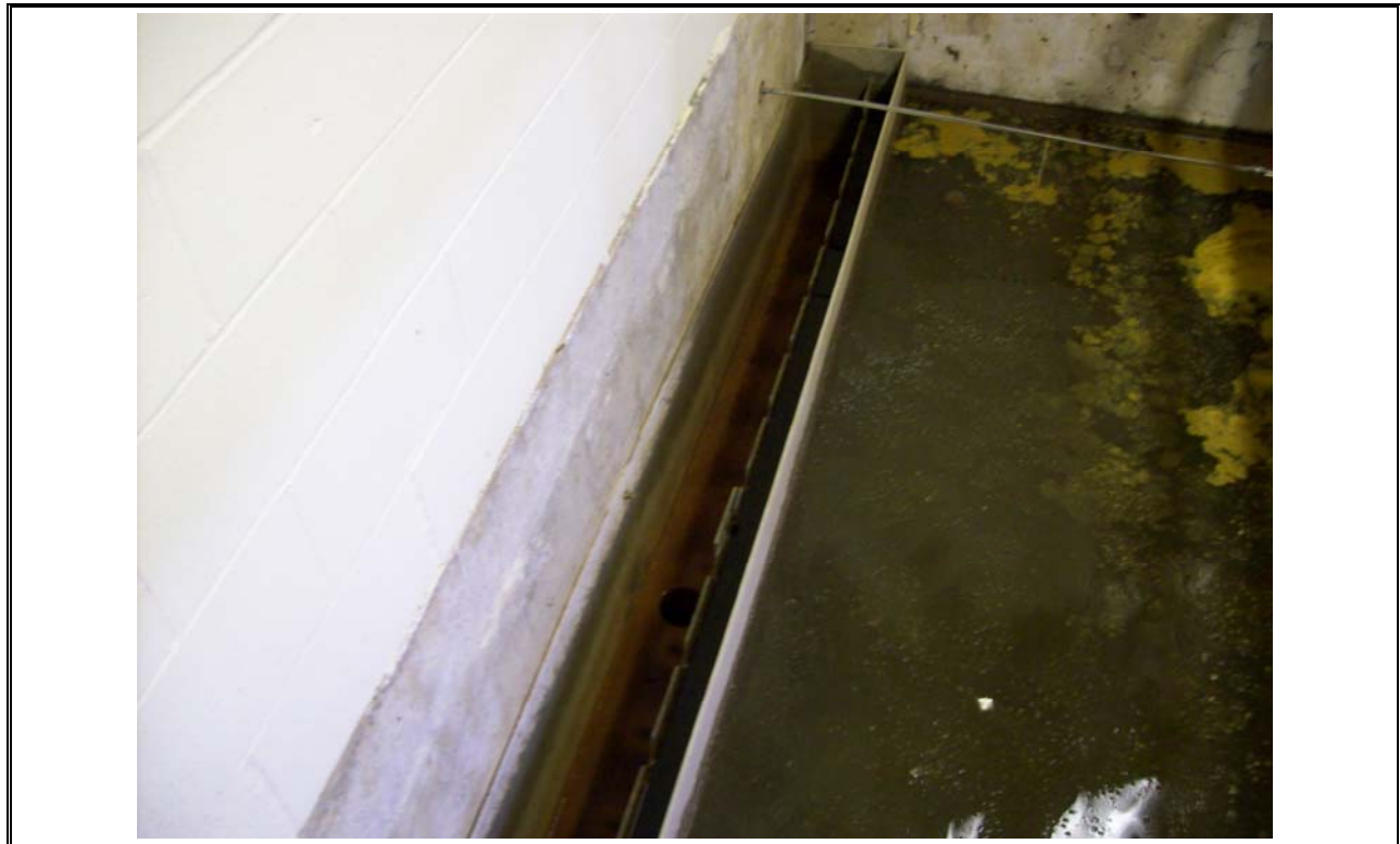
Photo 15 Lockview Clarifier Effluent Weir
