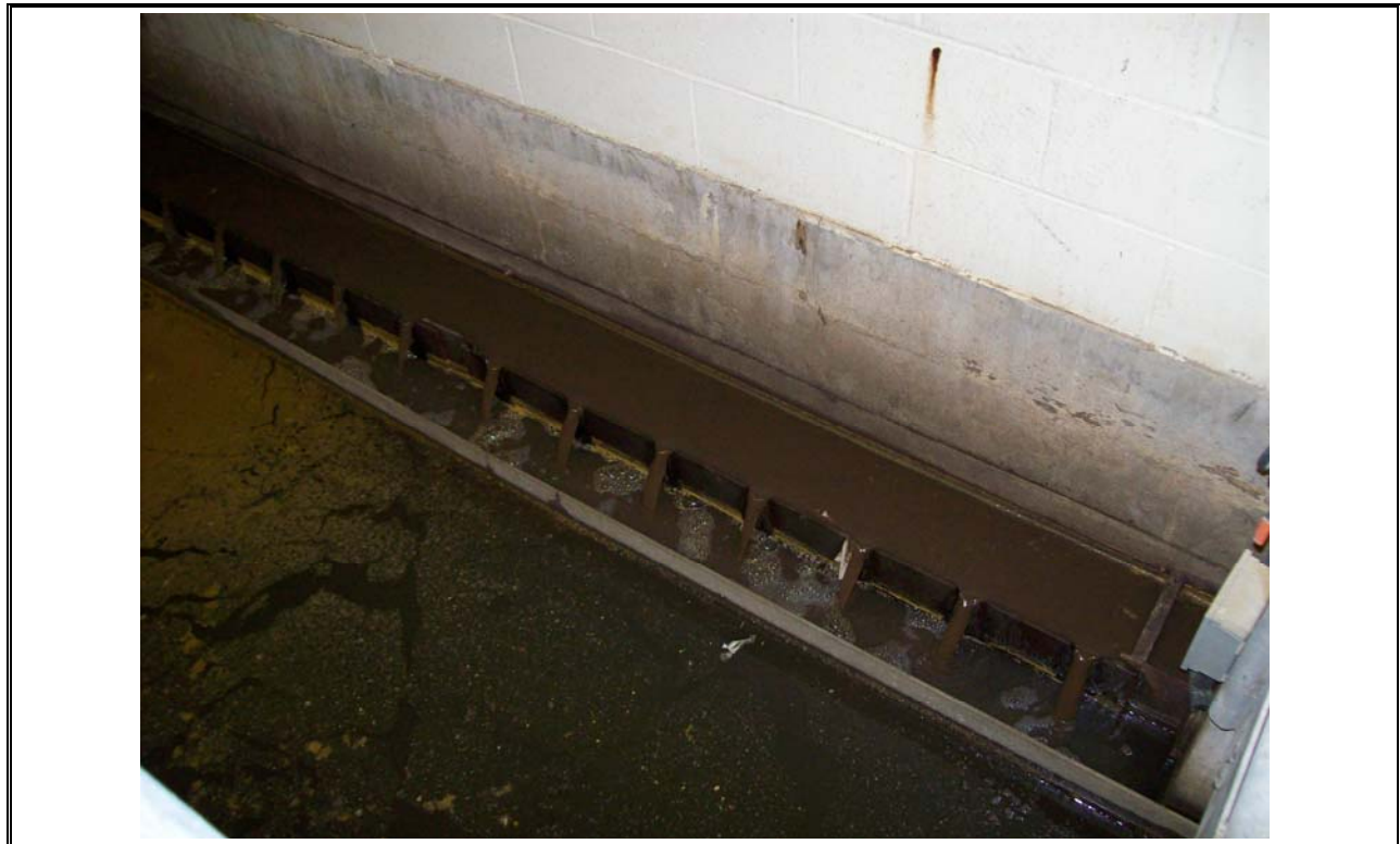
Photo 13 Lockview Clarifier Influent Weirs
