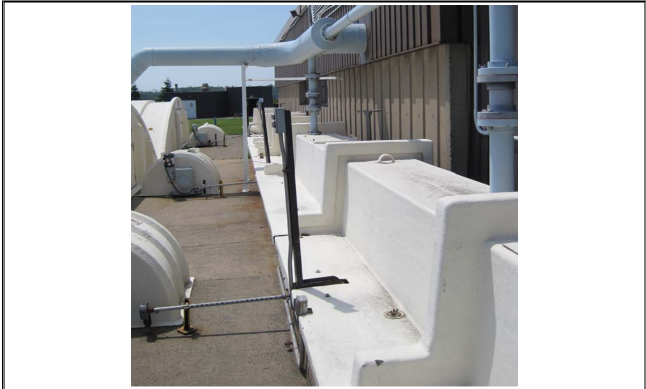
Photo 15 Eastern Passage Flow Covered Primary Clarifier Influent Channel
