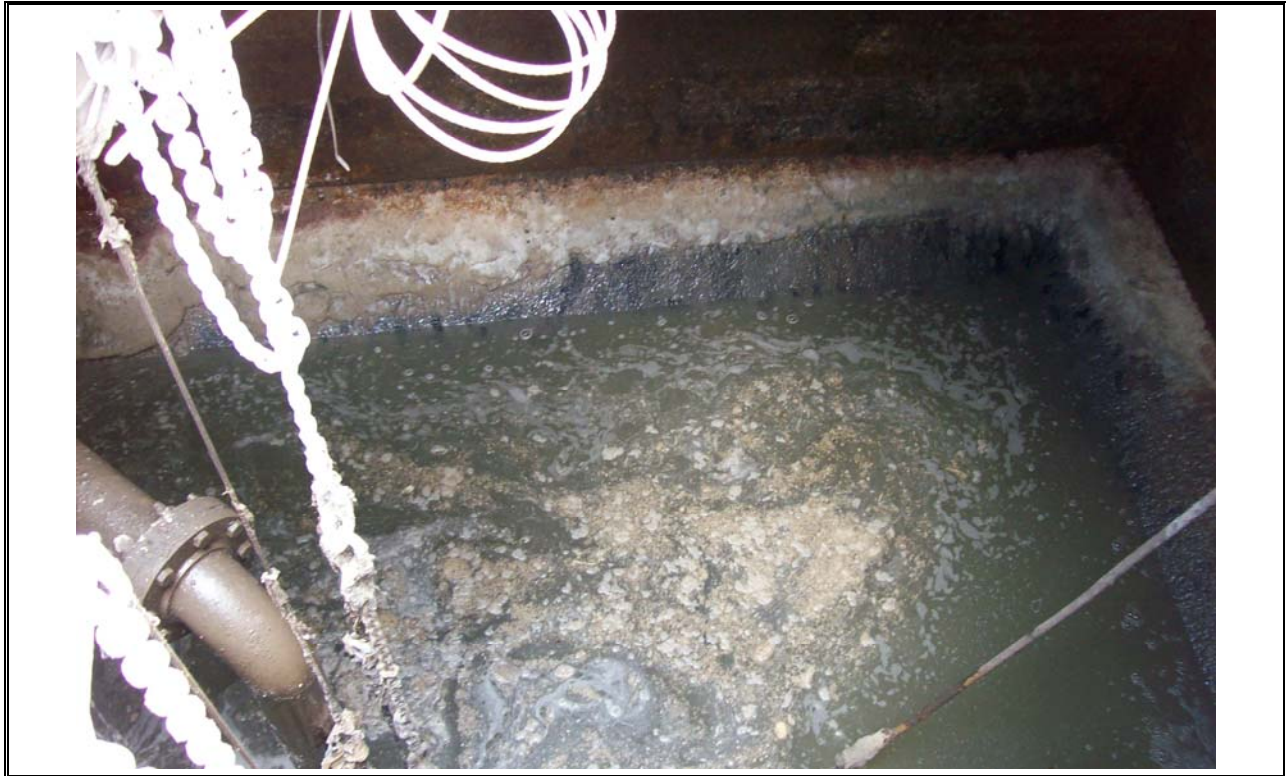
Photo 3 EQ Tank with Evidence of Grease Balls
