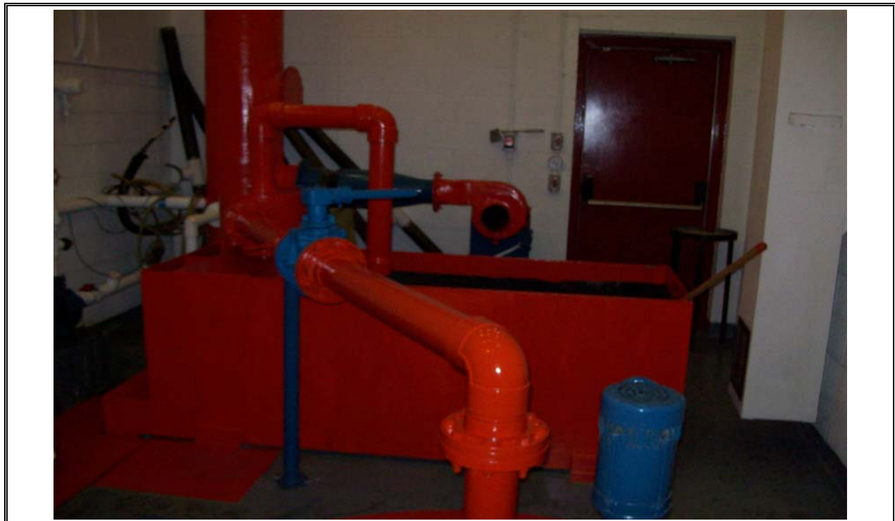
Photo 4 AeroTech Manual Grit Collection
