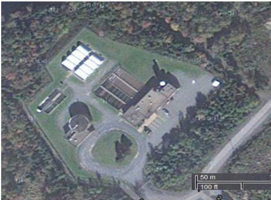
Figure 2.1 Lakeside Timberlea WWTF - Aerial View
