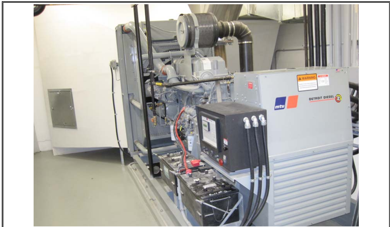
Photo 50 Herring Cove Back-up Generator
