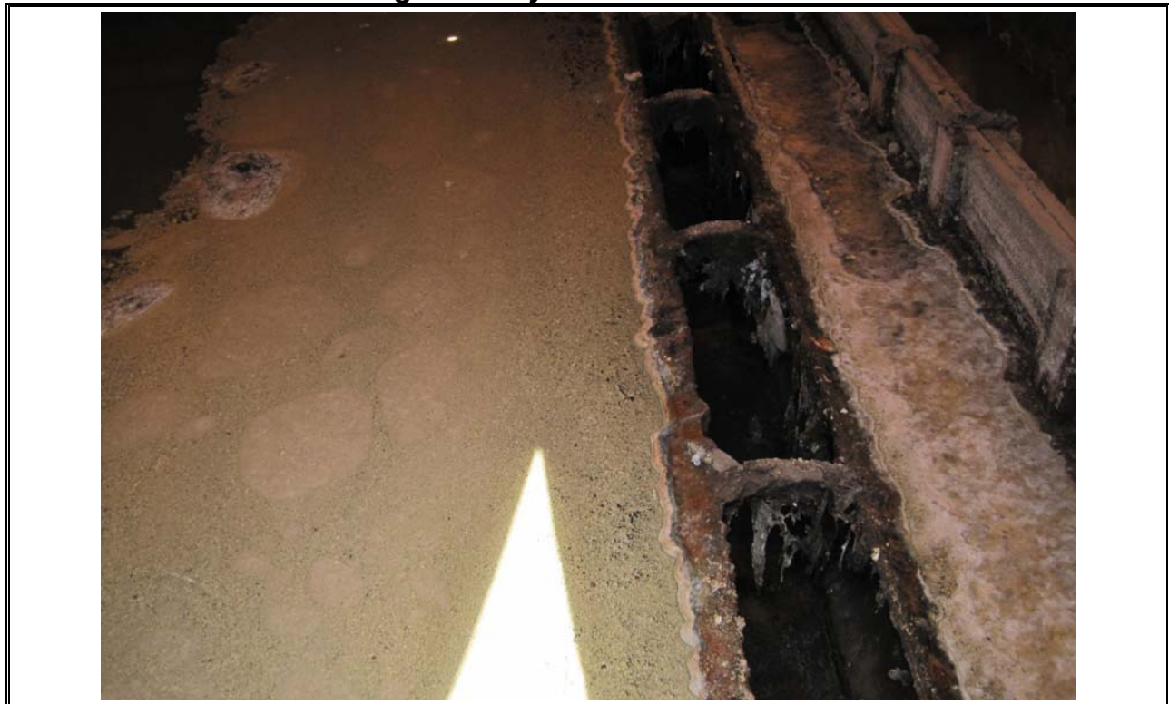
Photo 18 Eastern Passage Primary Clarifier Scum Trough
