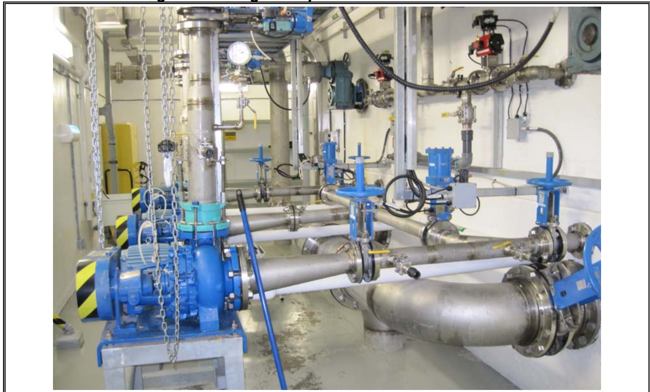
Photo 38 Herring Cove Solids Handling Pumps
