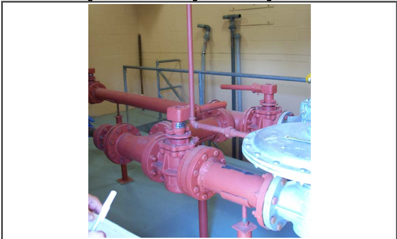
Photo 62 Gas Piping for Flare Stack from Digester
