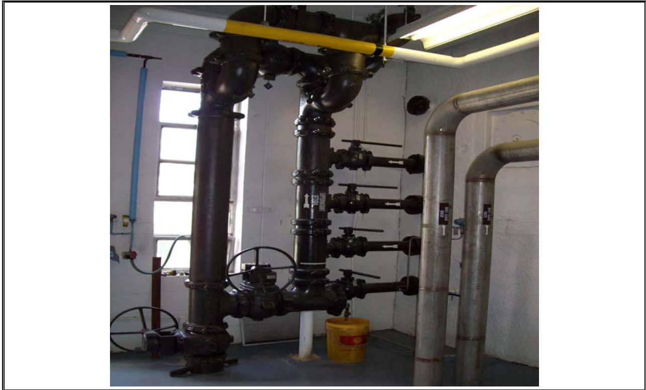
Photo 49 Supernatant Lines from Secondary Digester
