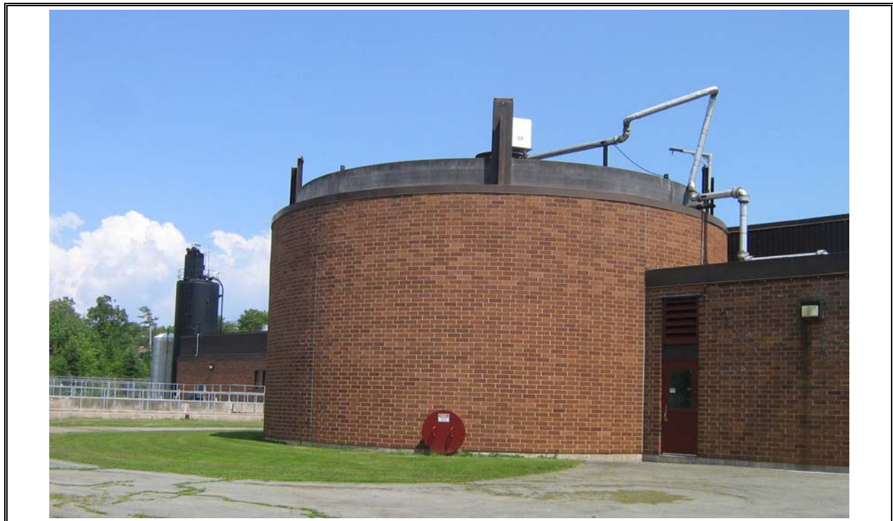
Photo 56 Anaerobic Digester
