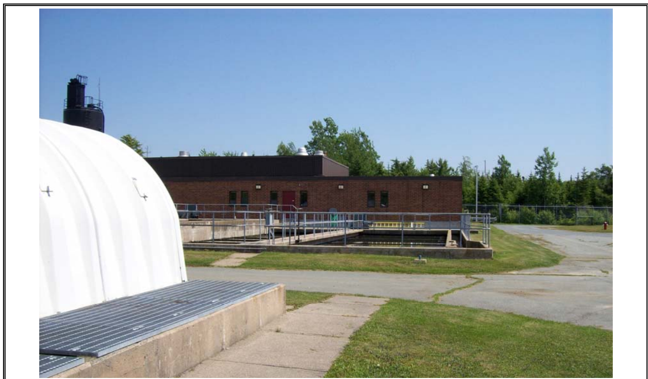
Photo 28 Channel from RBCs to Secondary Clarification
