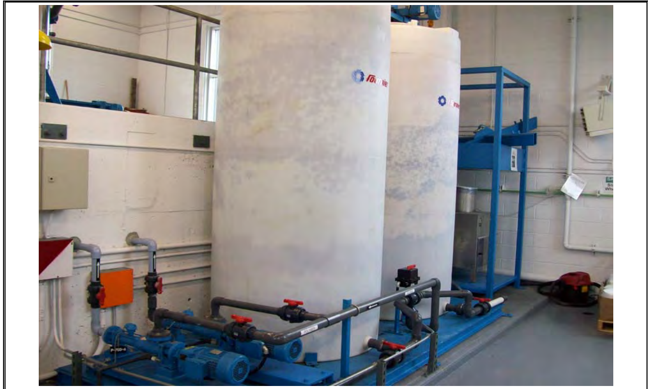
Photo 35 AeroTech Sludge Handling Polymer
