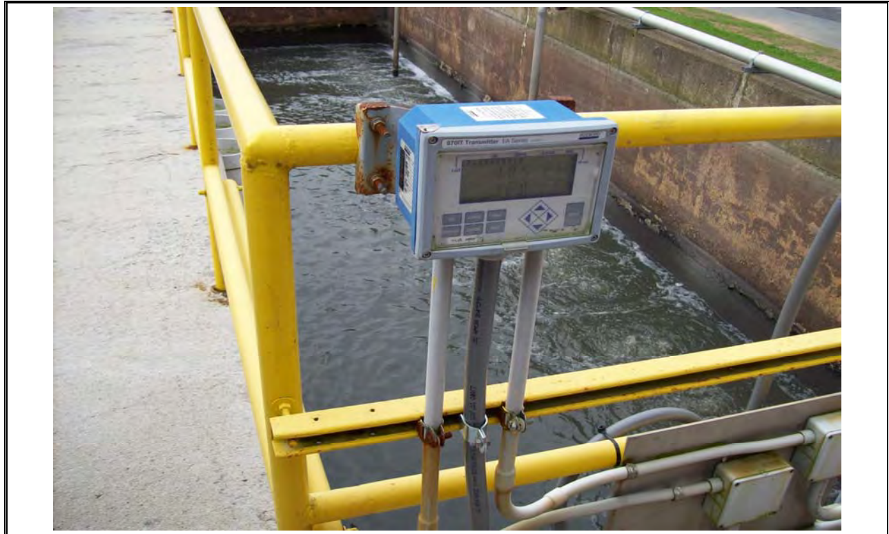
Photo 13 AeroTech Equalization Tank 1 Online Temperature and pH
