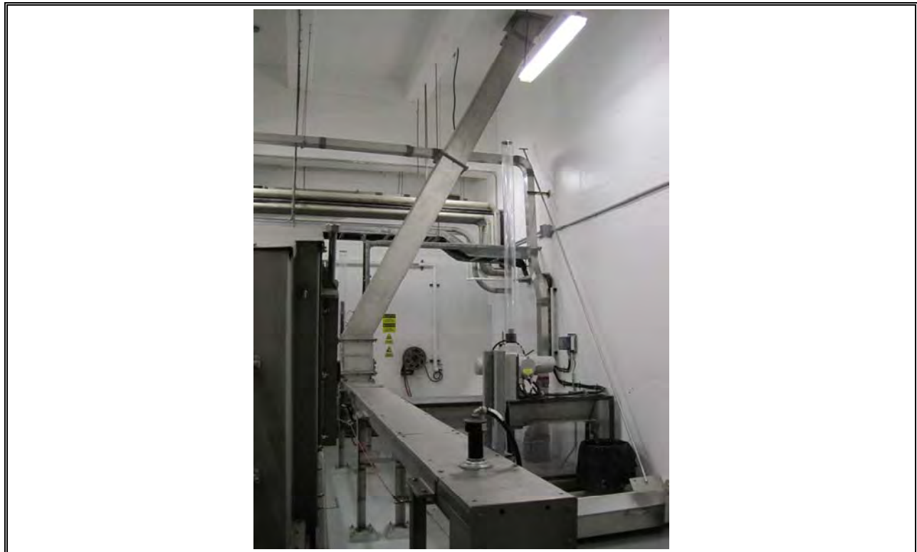
Photo 12 Dartmouth Screenings and Grit Conveyor
