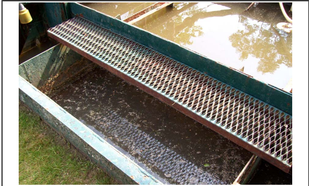
Photo 11 Wellington Effluent Channel Chlorine Contact Area
