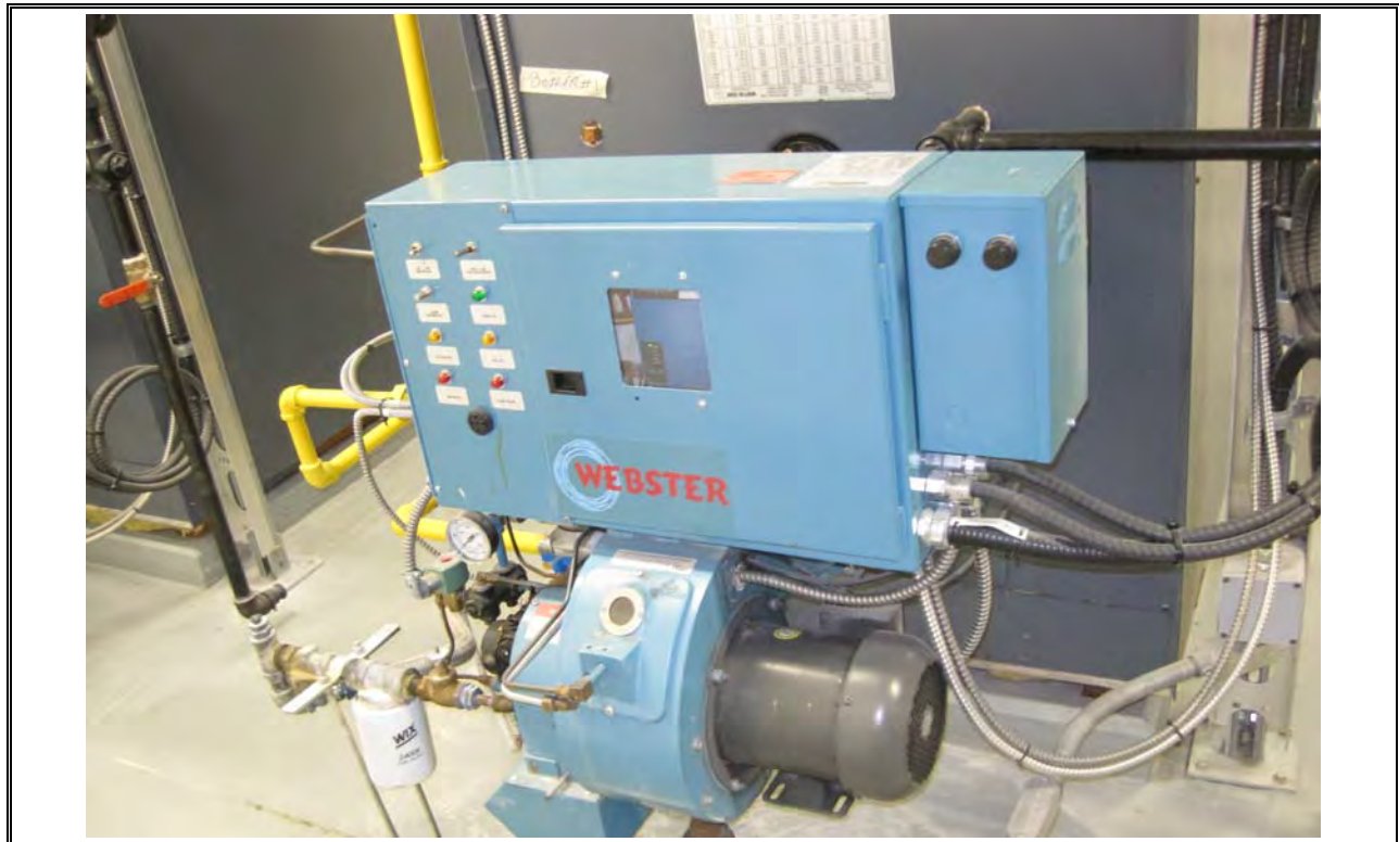
Photo 48 Dartmouth Boiler Equipment
