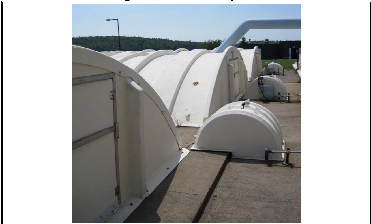
Photo 16 Eastern Passage Covered Primary Clarifiers
