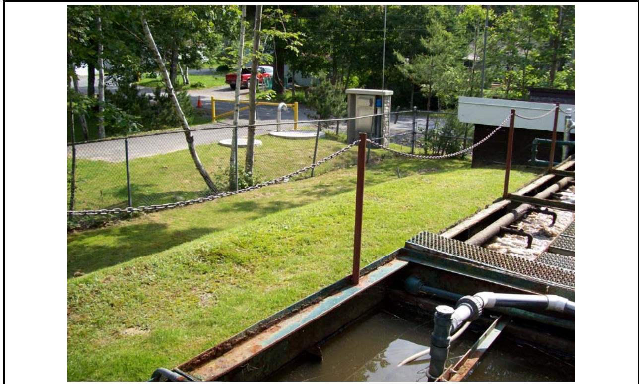
Photo 3 Wellington Influent Pumping Station & Site for New Facility
