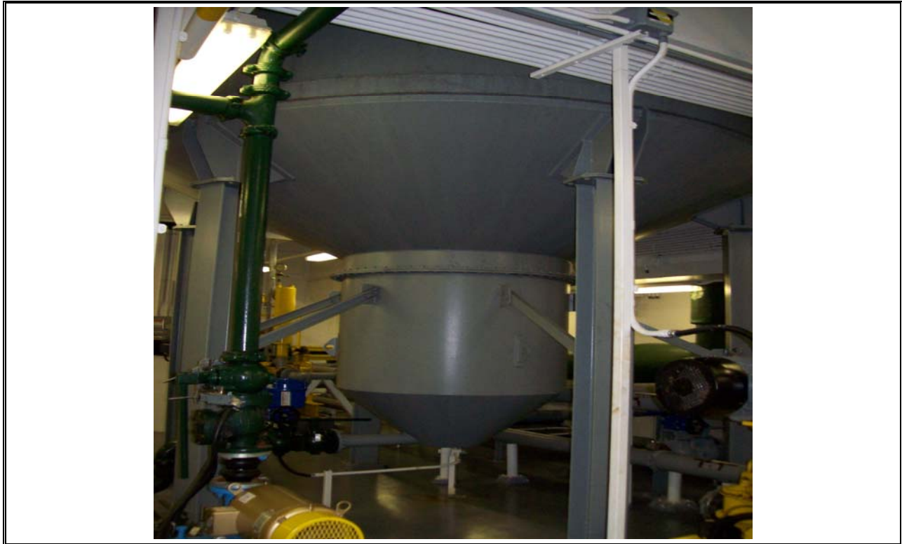
Photo 11 Grit Vortex Separator
