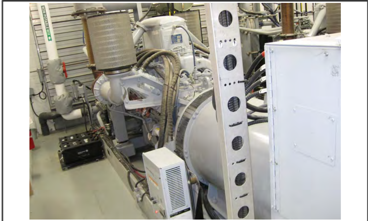
Photo 49 Dartmouth Back-up Generator
