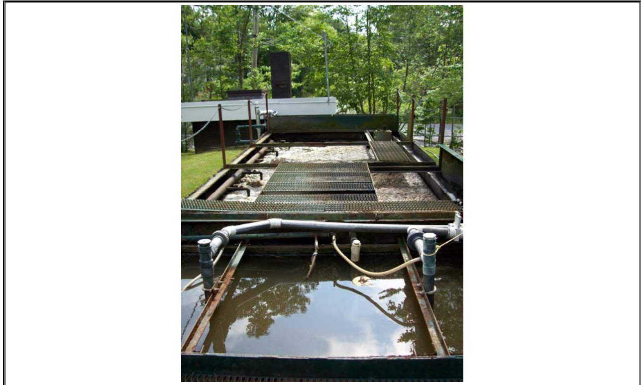
Photo 1 Wellington Package Plant Overview
