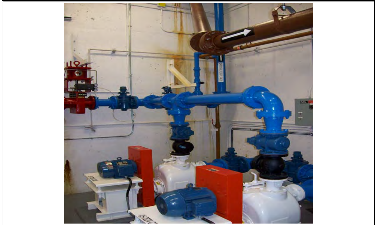
Photo 27 AeroTech Filter Feed Pumps
