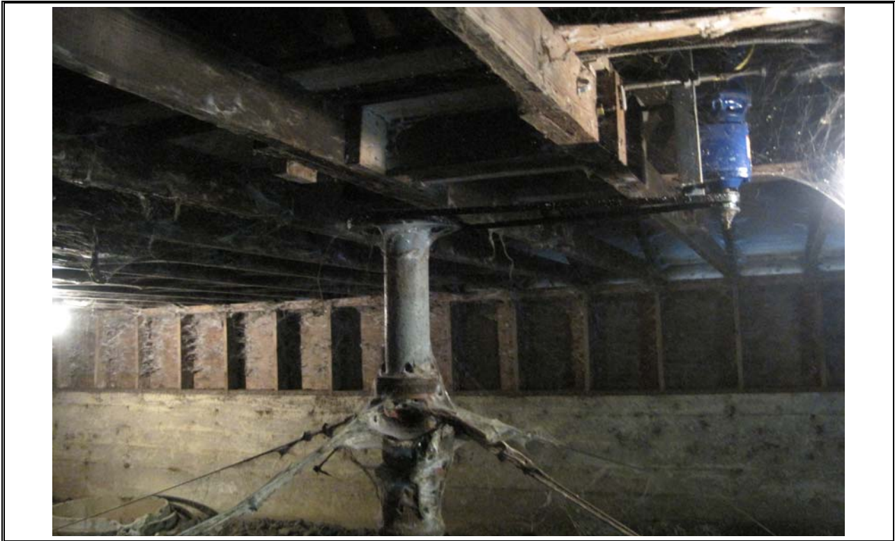
Photo 13 Uplands Park Distribution Arm Gear Box Broken
