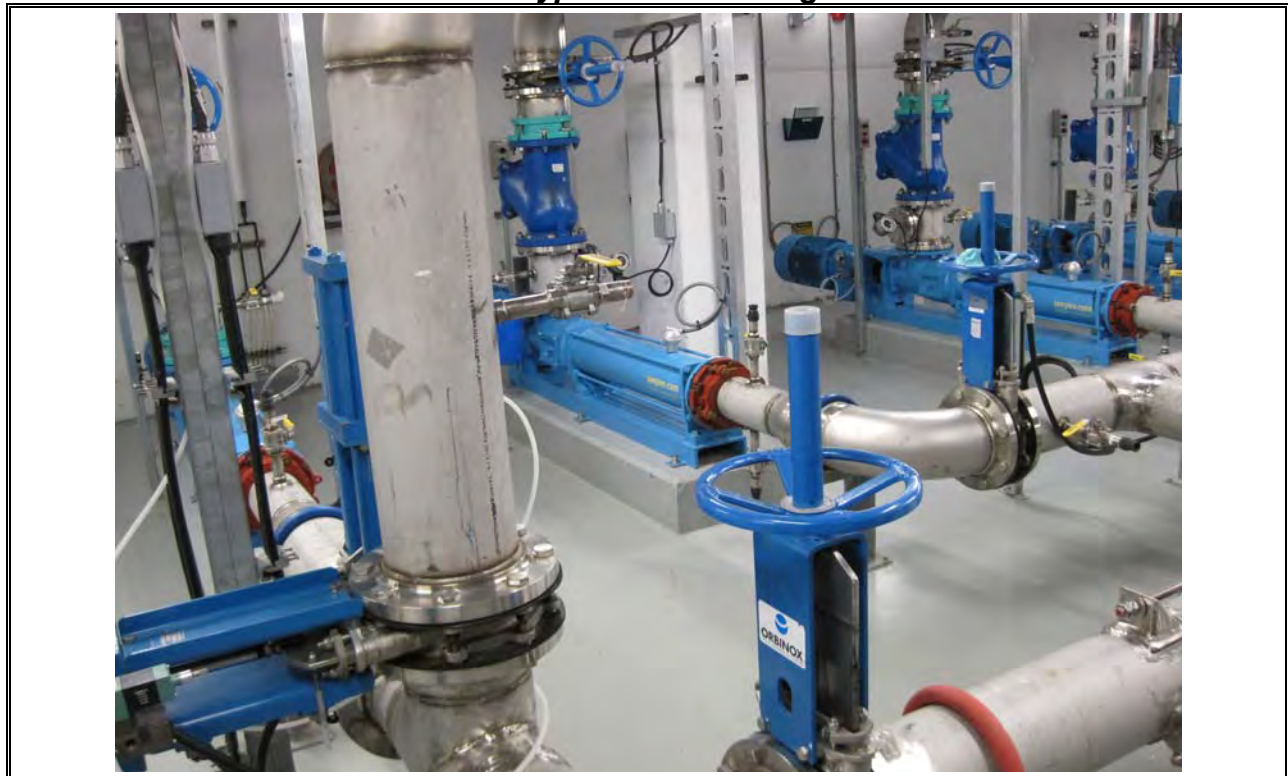
Photo 36 Dartmouth Densadeg Sludge Pumps
