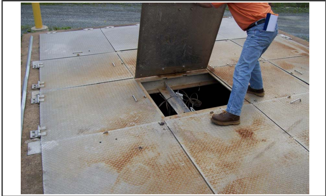
Photo 1 EQ Tank Below Checker Plate
