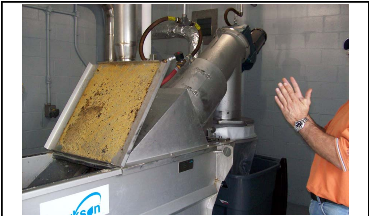
Photo 8 Screen and Screenings Bin
