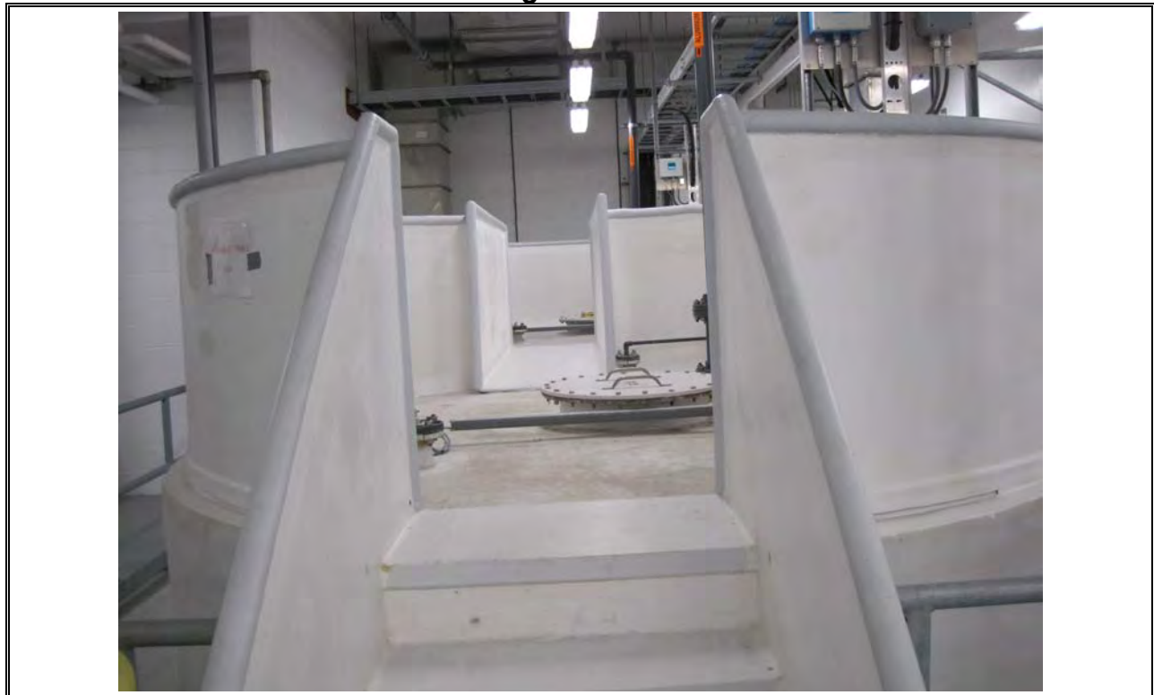
Photo 28 Dartmouth Alum Storage Tanks
