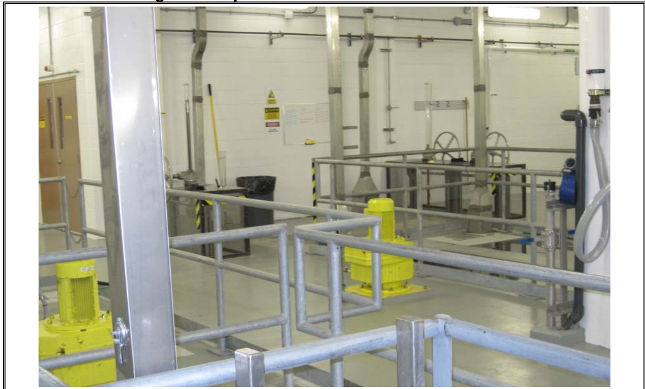
Photo 16 Herring Cove Densadeg Flocculation Tanks Below Slab
