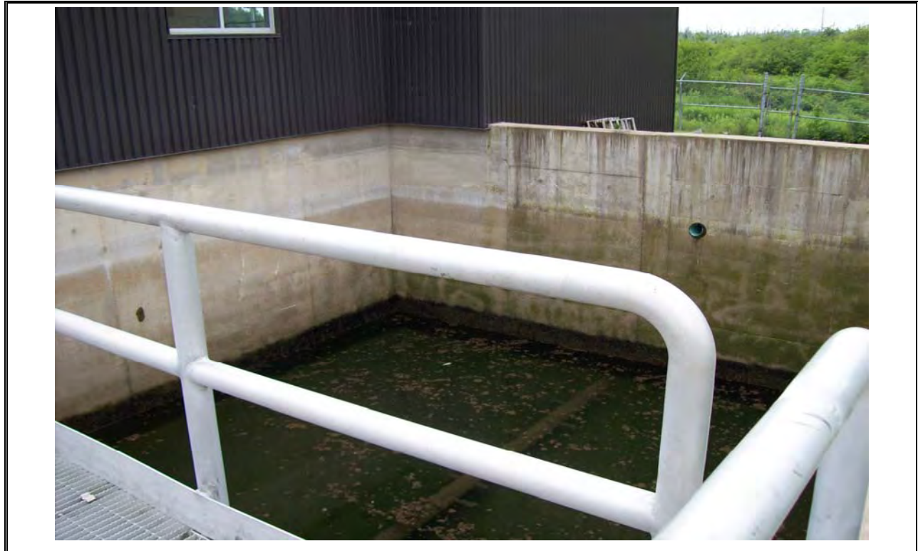
Photo 17 AeroTech Post Equalization Tank with Emergency Overflow
