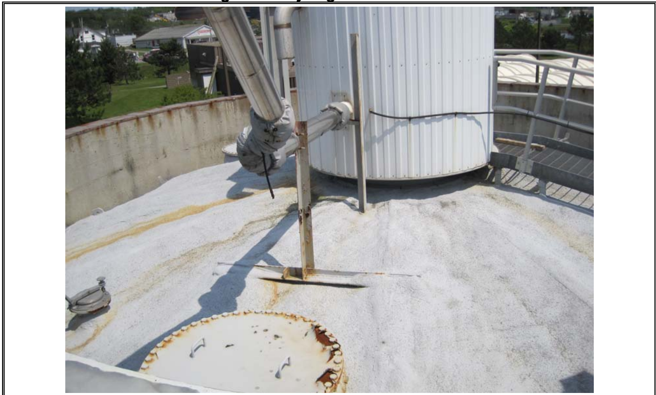
Photo 36 Eastern Passage Secondary Digester Roof
