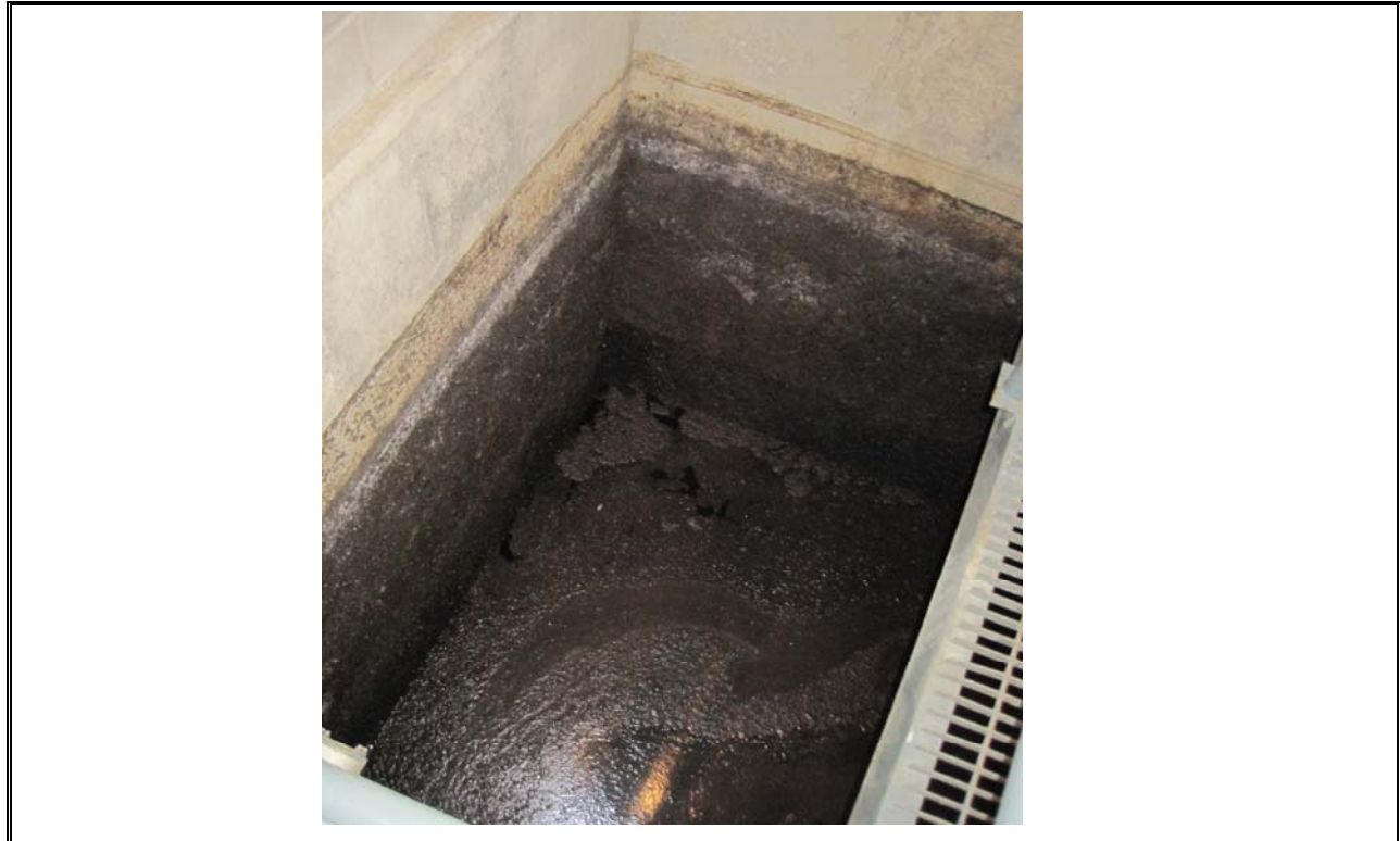
Photo 25 Waste Sludge Tank
