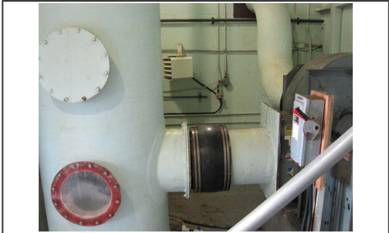
Photo 13 Eastern Passage Odour Control Wet Scrubber
