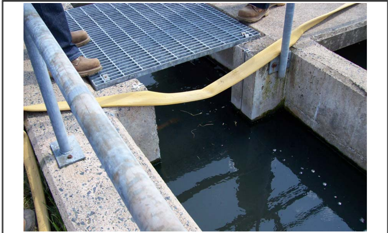
Photo 37 Hypochlorite Addition Point
