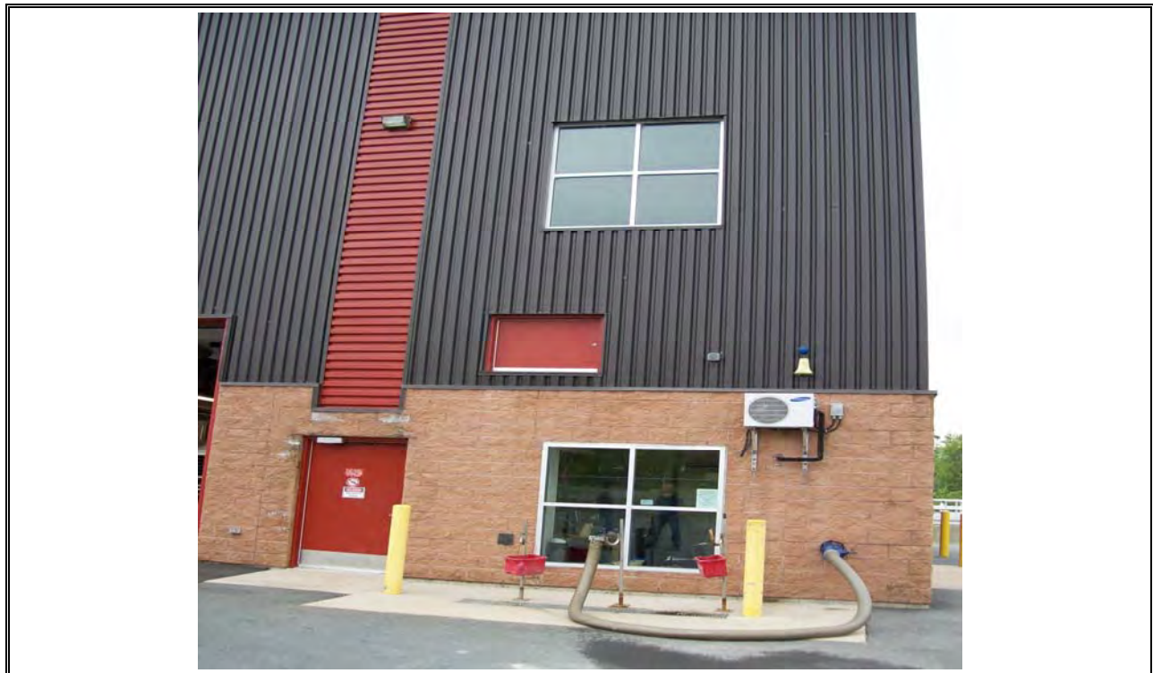
Photo 38 AeroTech Sludge Building
