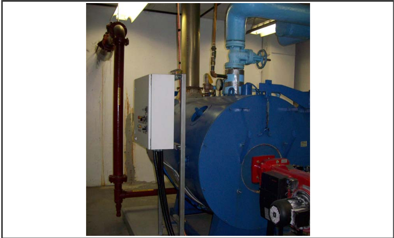
Photo 51 Boiler Located in Headworks Building
