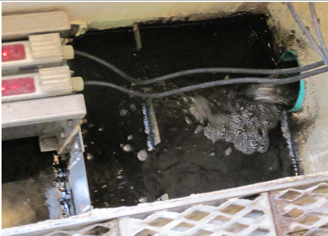
Photo 11 Polishing Pond Outlet to UV Disinfection (below surface)
