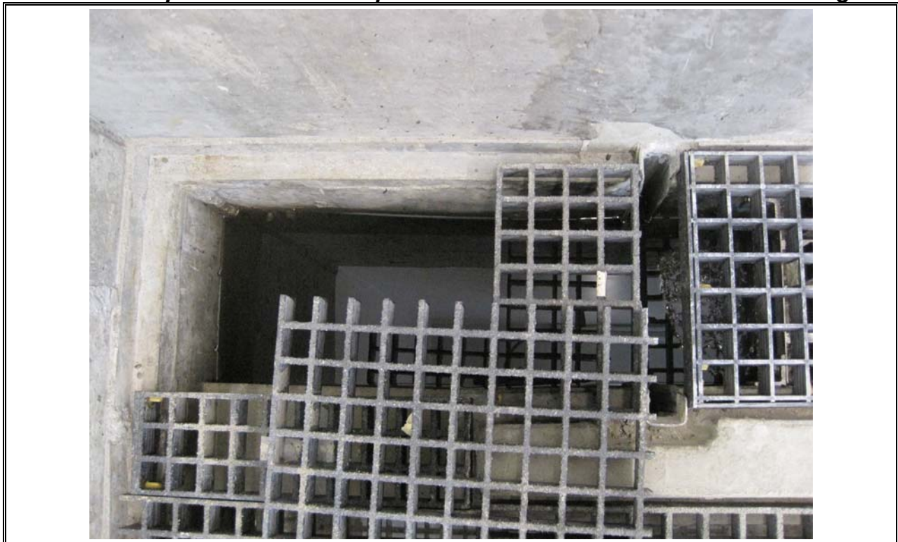
Photo 24 Uplands Park Influent to UV Disinfection Building & Bypass Weir
