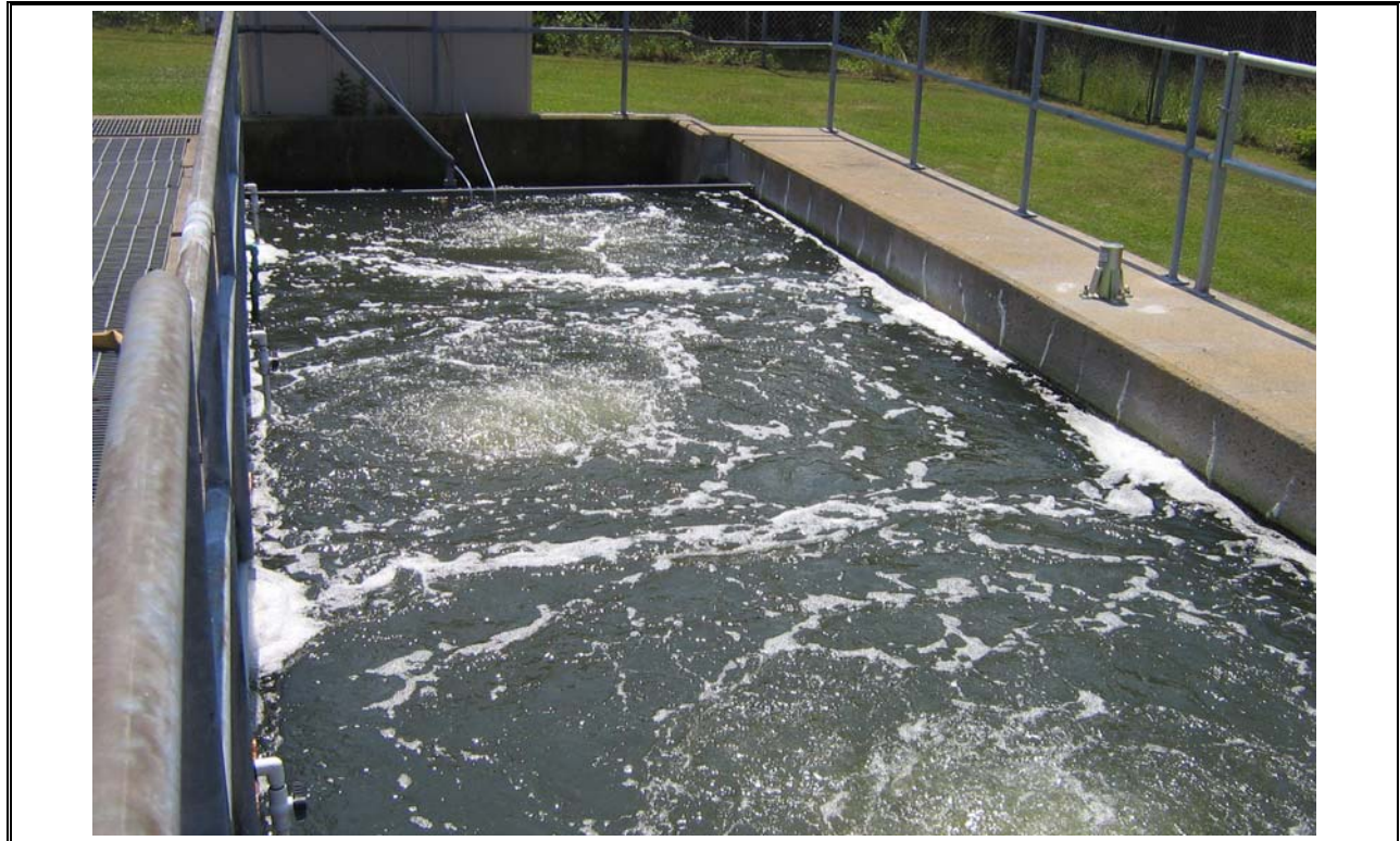
Photo 41 Post Aeration and Effluent DO Meter
