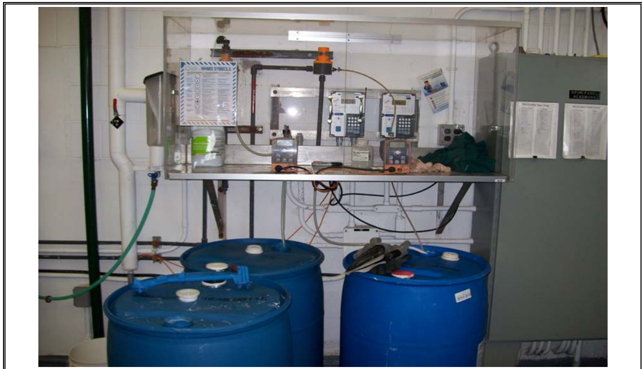
Photo 52 Odour Control Chemicals
