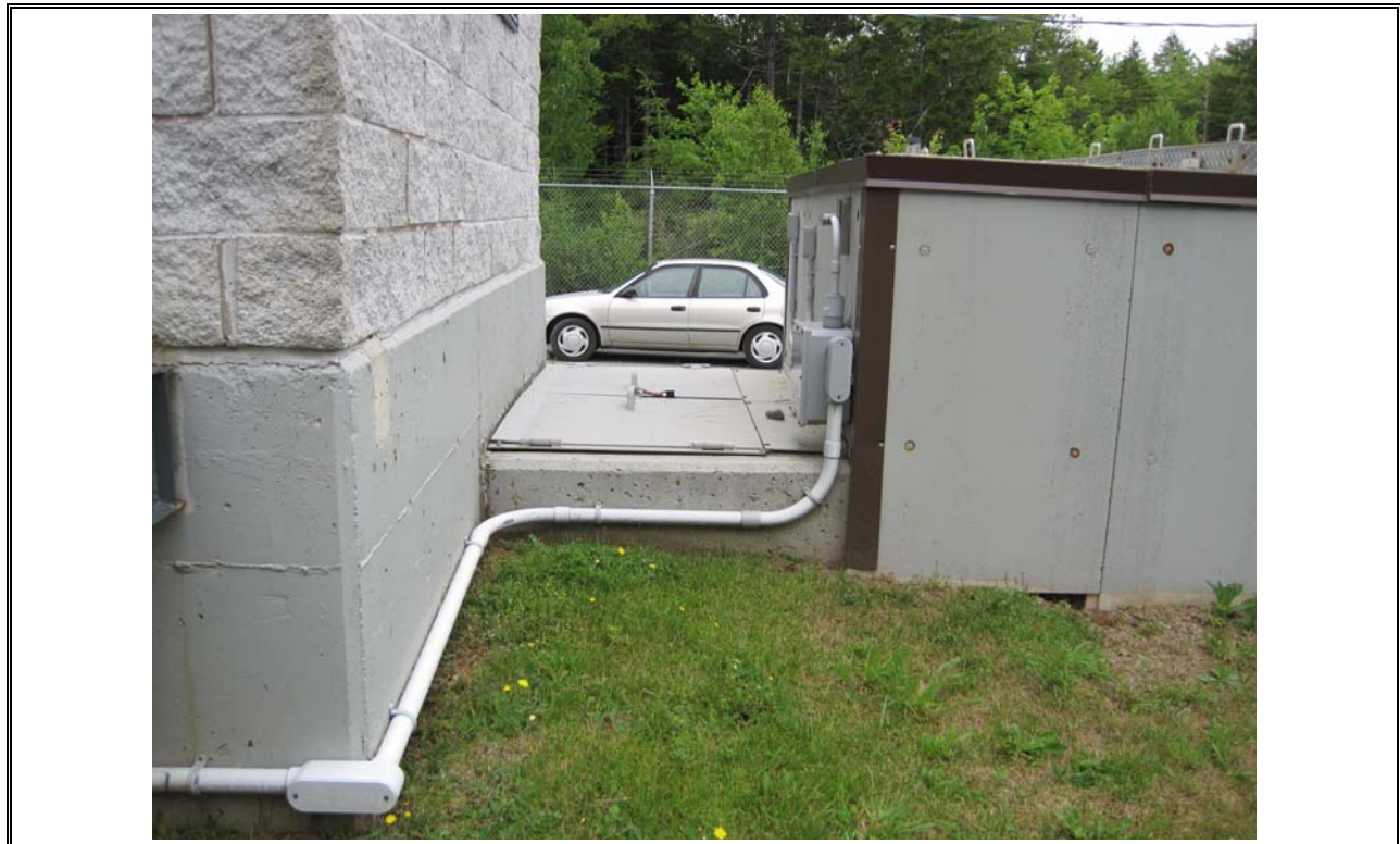
Photo 2 Line from Inlet Box to Headworks
