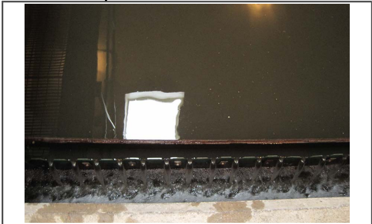
Photo 14 Secondary Clarifier Effluent Weir
