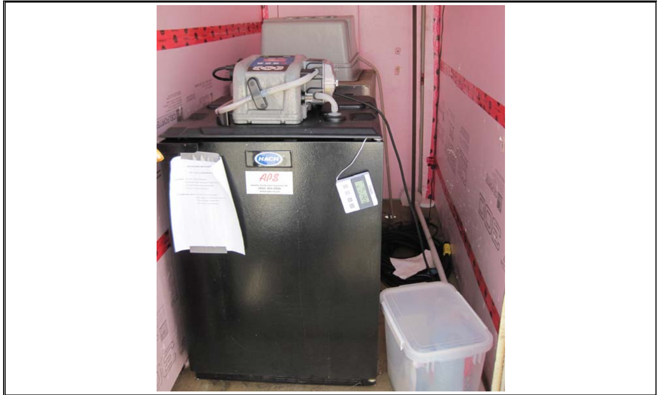
Photo 25 Eastern Passage Effluent Autosampler
