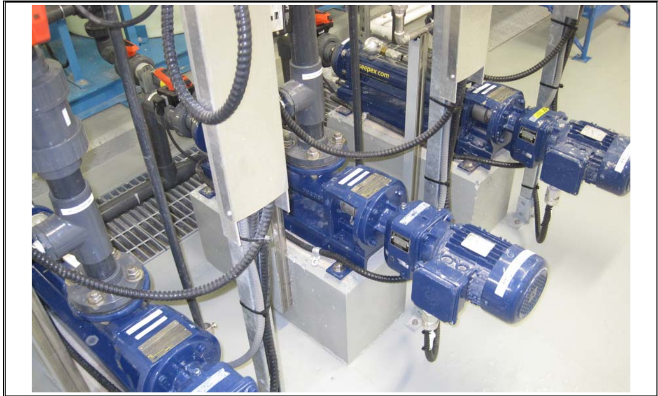
Photo 37 Herring Cove Sludge Pumps
