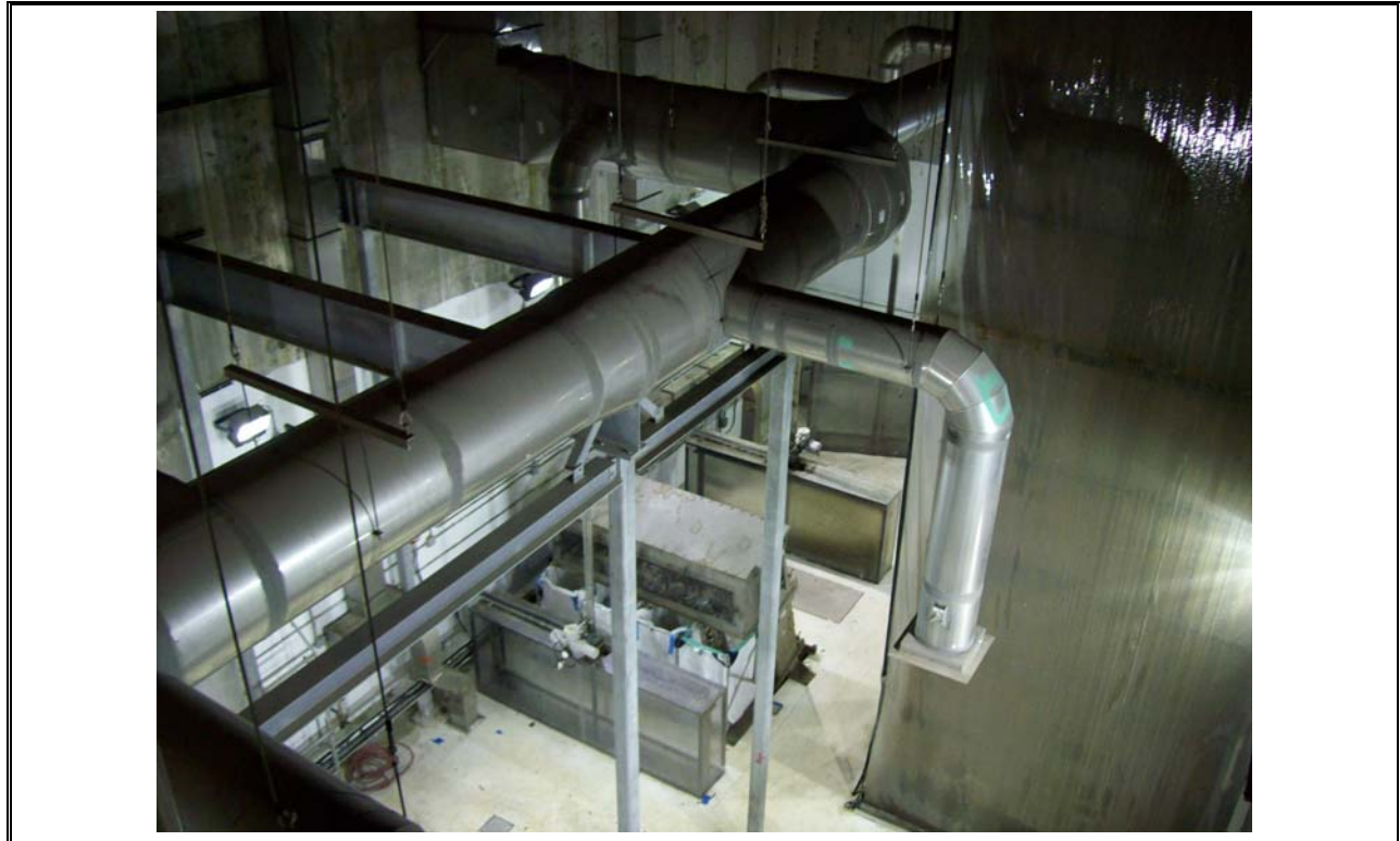
Photo 5 Halifax Mechanical Screen and Back-Up Mechanical Screen
