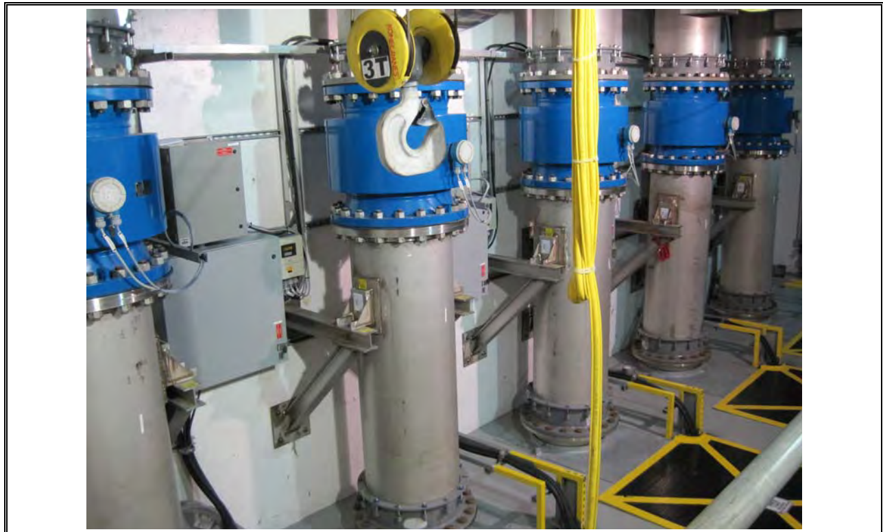
Photo 4 Dartmouth Raw Wastewater Pumps and Magmeters
