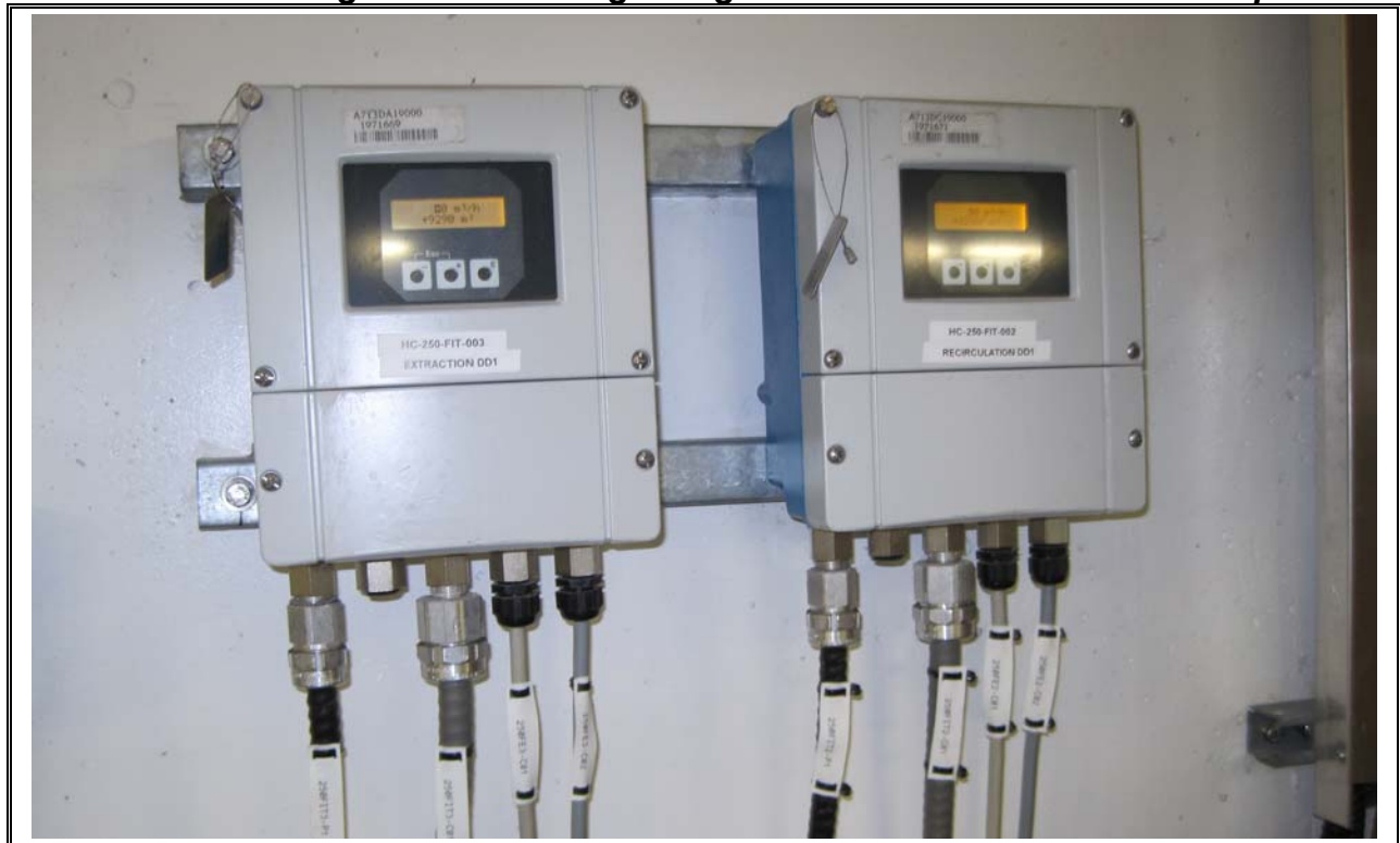
Photo 36 Herring Cove Extraction and Recirculation Pump Metering
