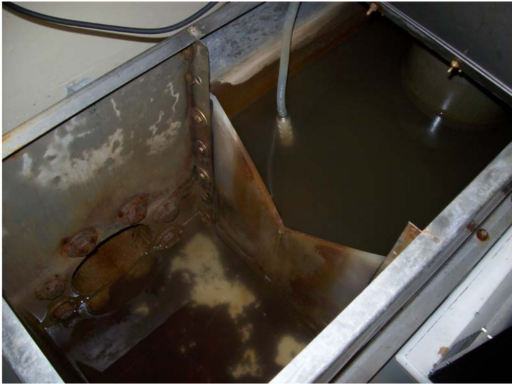
Photo 27 Lockview Effluent V-notch Weir Flow Meter & Effluent Sample Tubing
