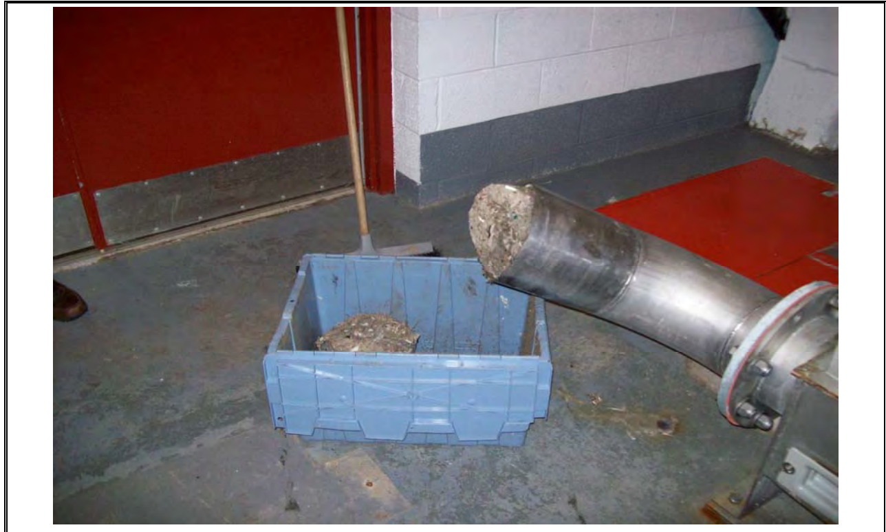
Photo 7 AeroTech Screenings Bin
