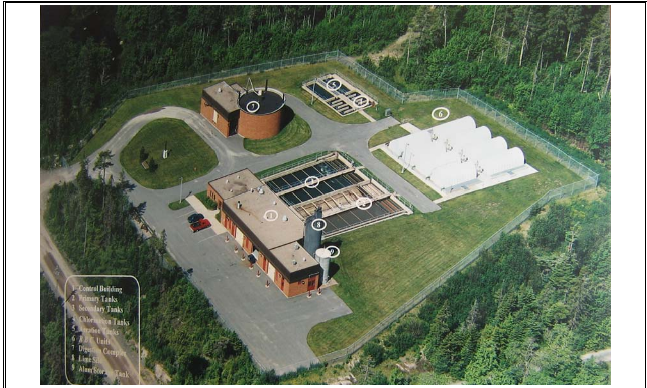
Photo 1 Aerial View of Site Layout
