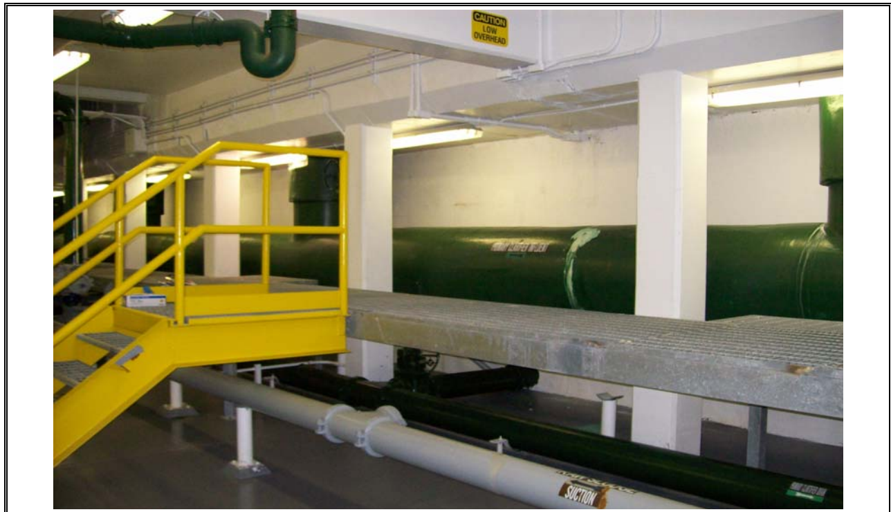
Photo 16 North Plant Primary Clarifier Influent Line
