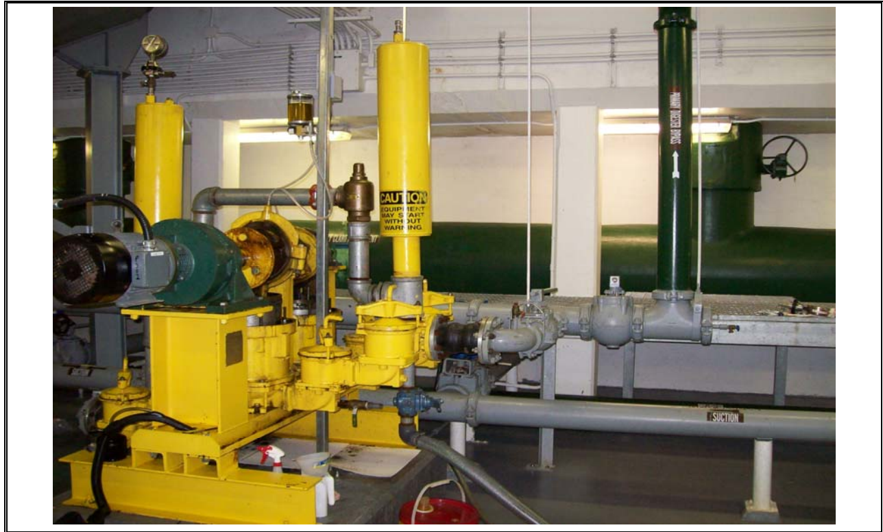
Photo 45 Co-thickened Sludge Pump
