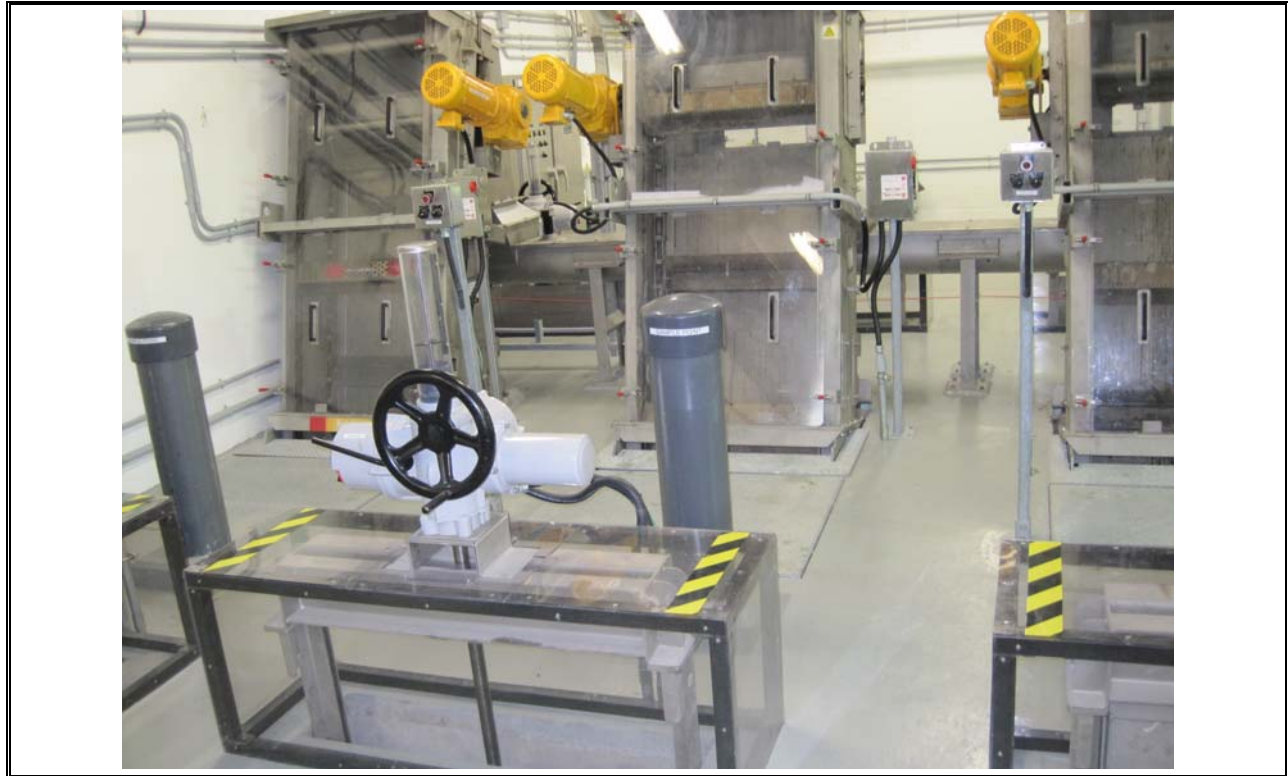
Photo 9 Herring Cove Fine Bar Screens
