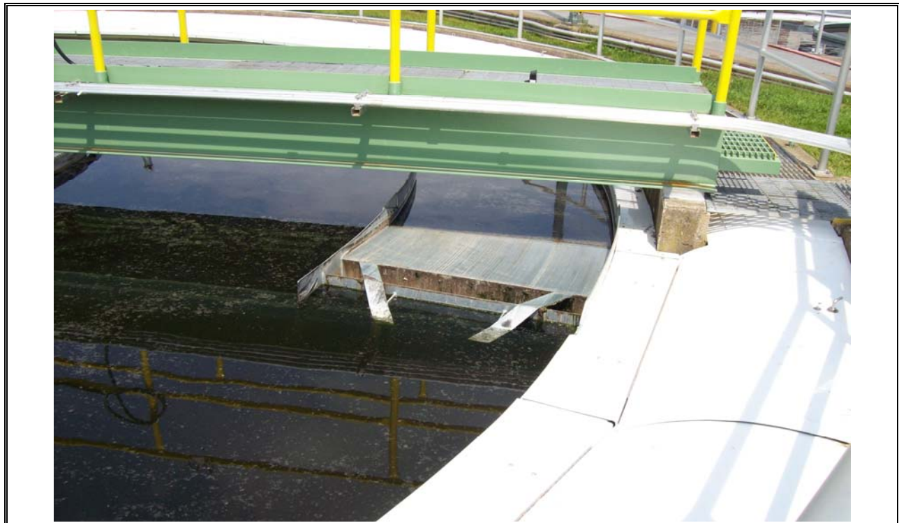
Photo 38 Secondary Clarifier Covered Troughs
