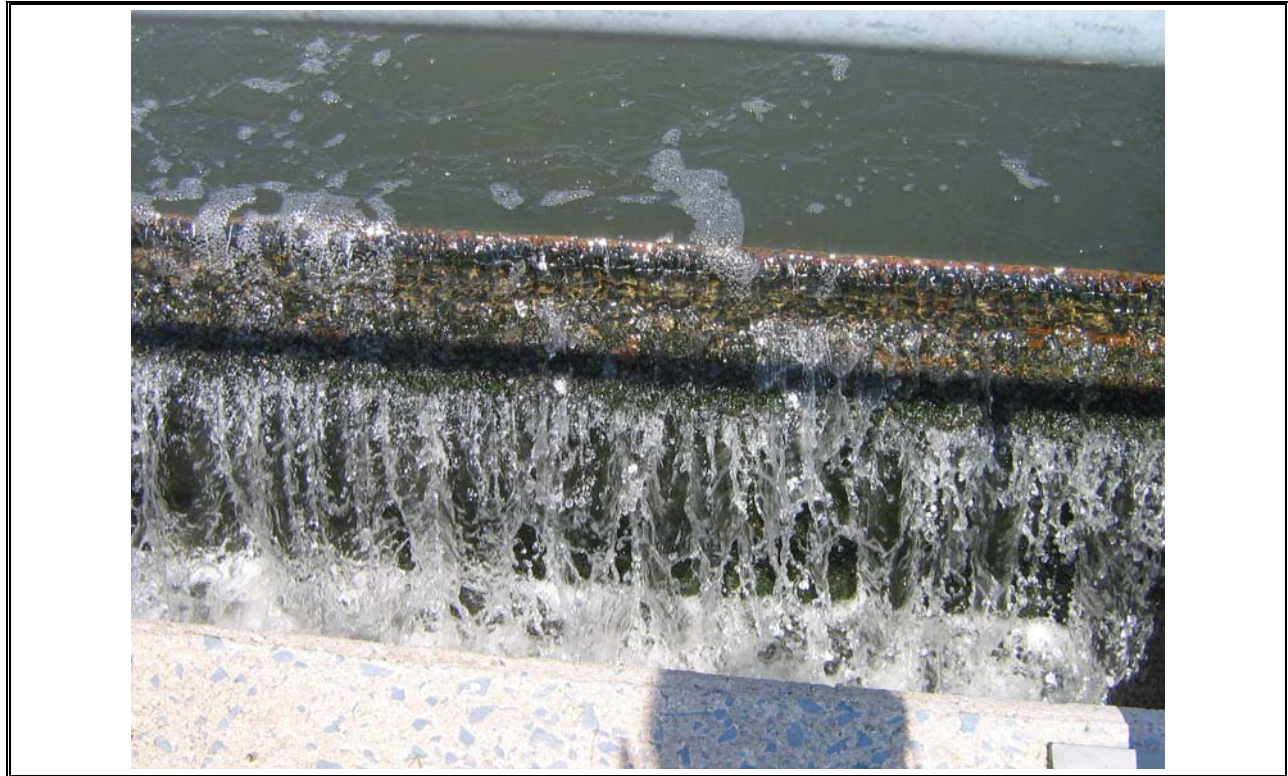
Photo 43 Effluent from Post Aeration Tank to Nine Mile River
