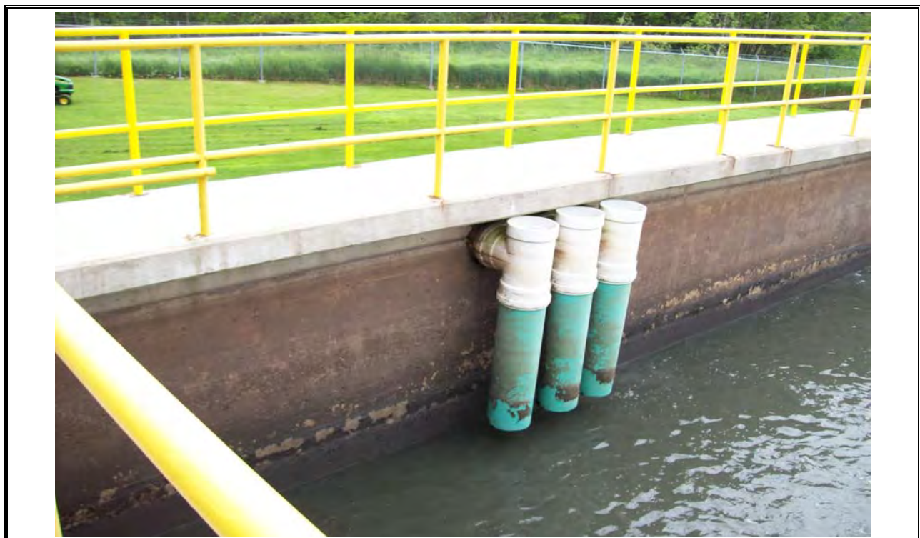
Photo 14 AeroTech Equalization Tank 1 Overflow to Equalization Tank 2
