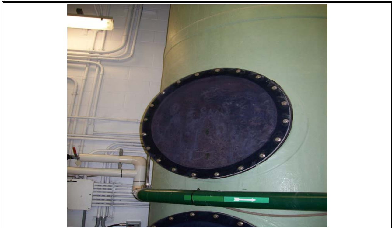
Photo 54 Wet Scrubber Media
