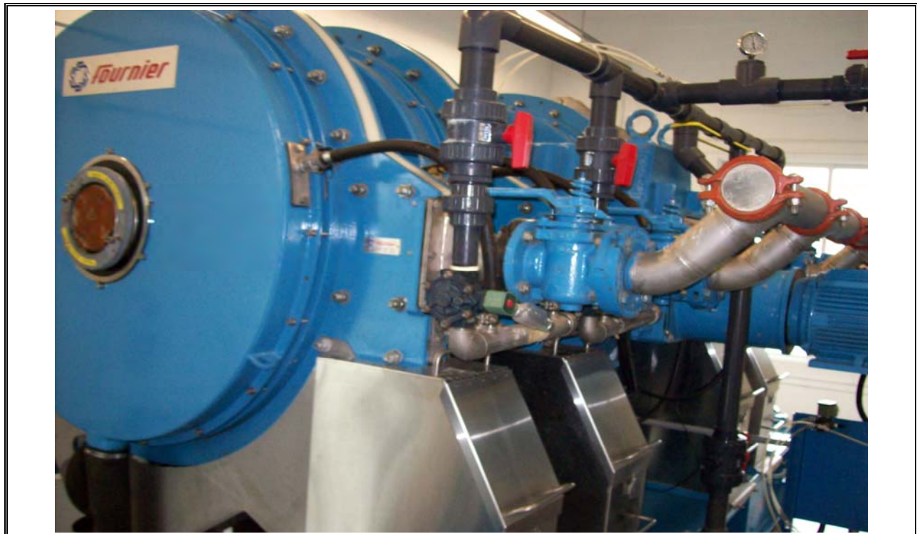
Photo 36 AeroTech Sludge Dewatering Presses
