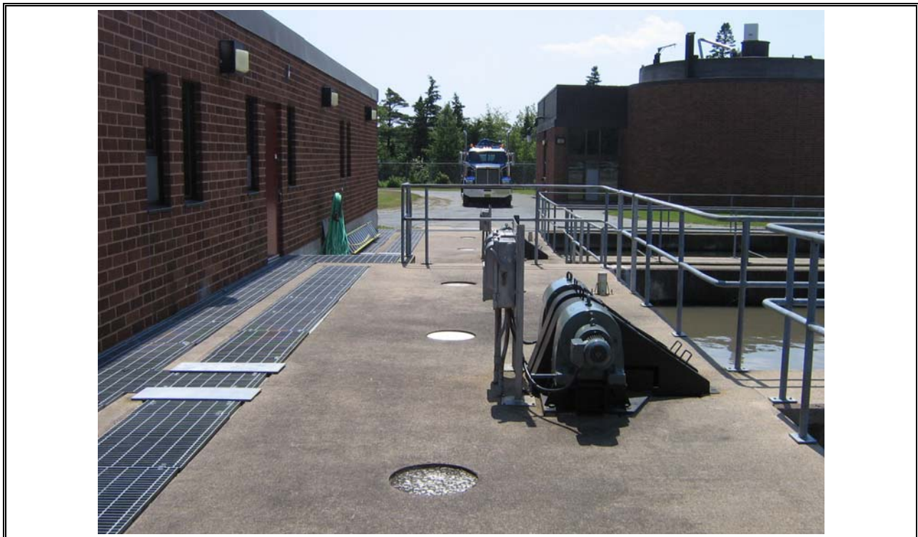
Photo 14 Wastewater Flowing from Headworks to Primary Clarification
