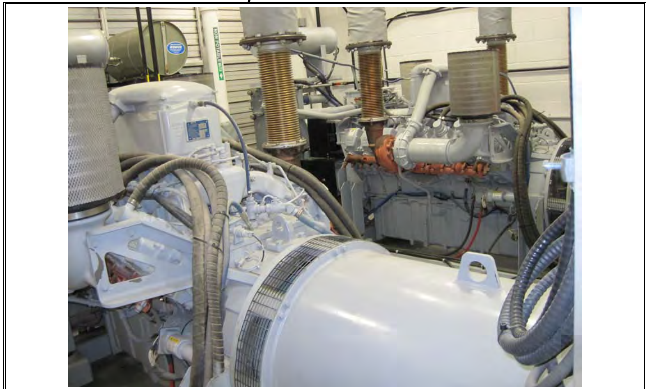
Photo 50 Dartmouth Back-up Generator
