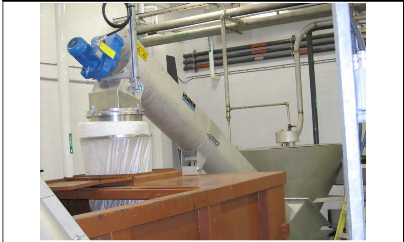
Photo 13 Dartmouth Screenings and Grit Waste Bin
