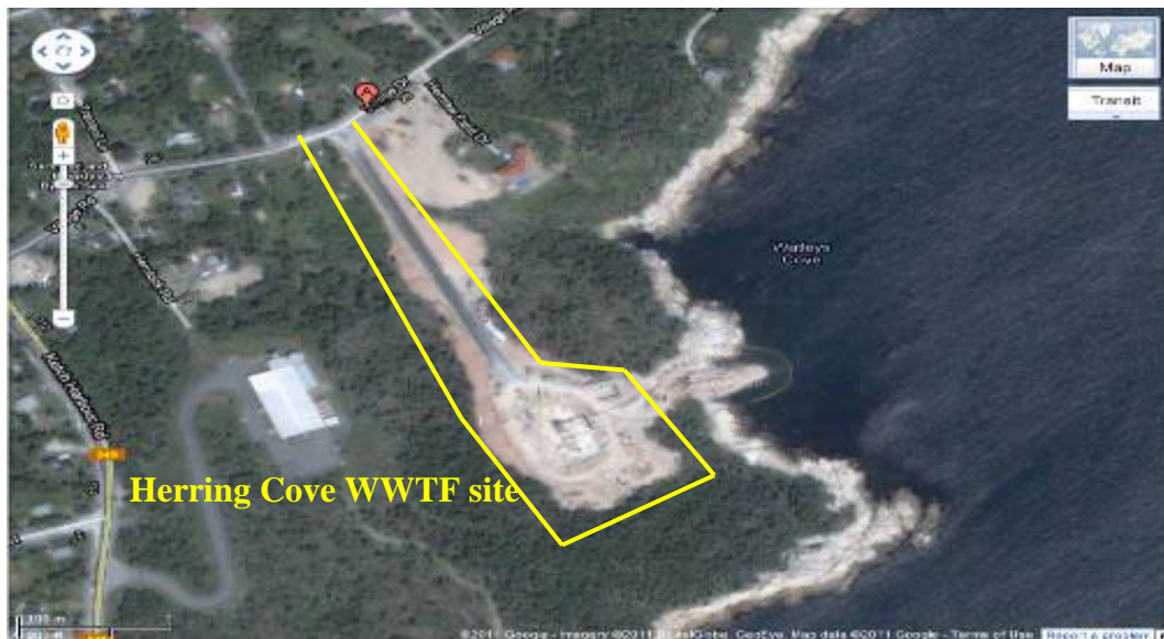
Figure 2.1 Herring Cove WWTF under Construction - Aerial View
