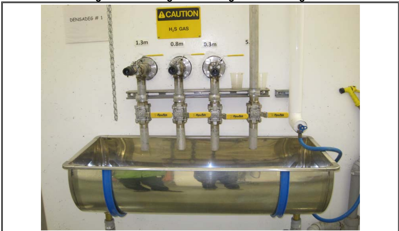
Photo 20 Herring Cove Densadeg Sedimentation Zone Sludge Blanket Sampling Sink
