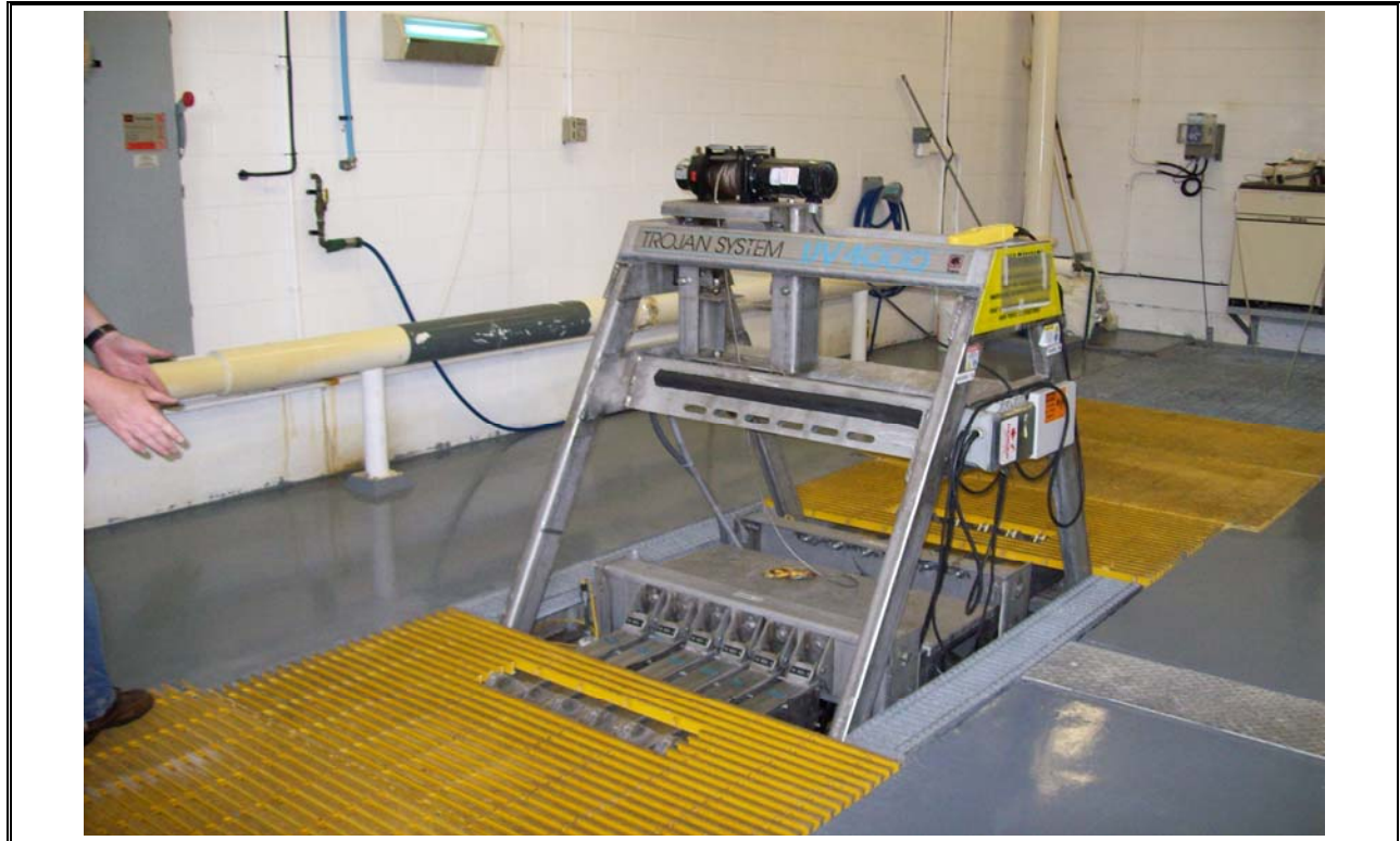
Photo 39 UV Disinfection System
