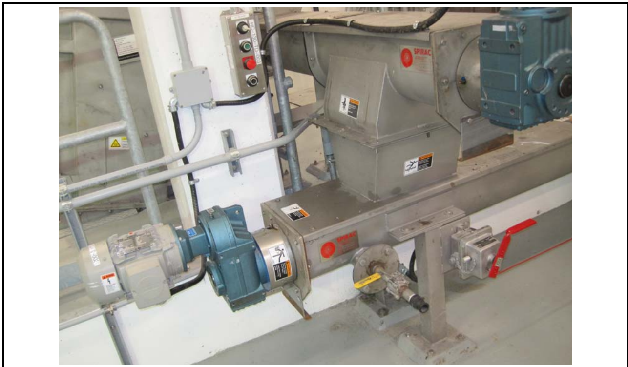
Photo 6 Herring Cove Screenings Conveyor
