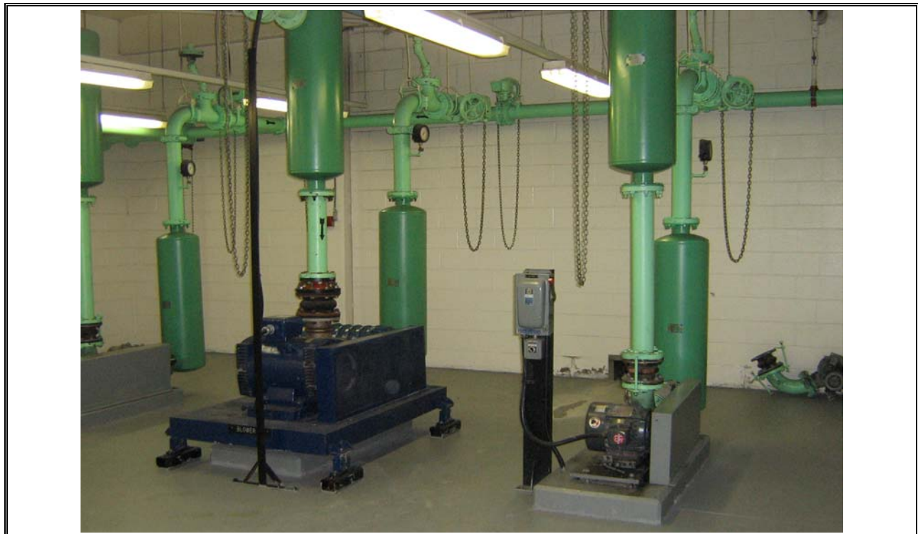
Photo 50 Compressors for Air Supply to the Plant
