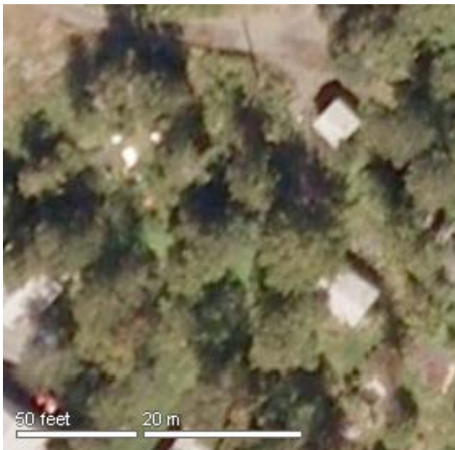
Figure 2.11 Silver Sand Water Supply Plant - Aerial View
