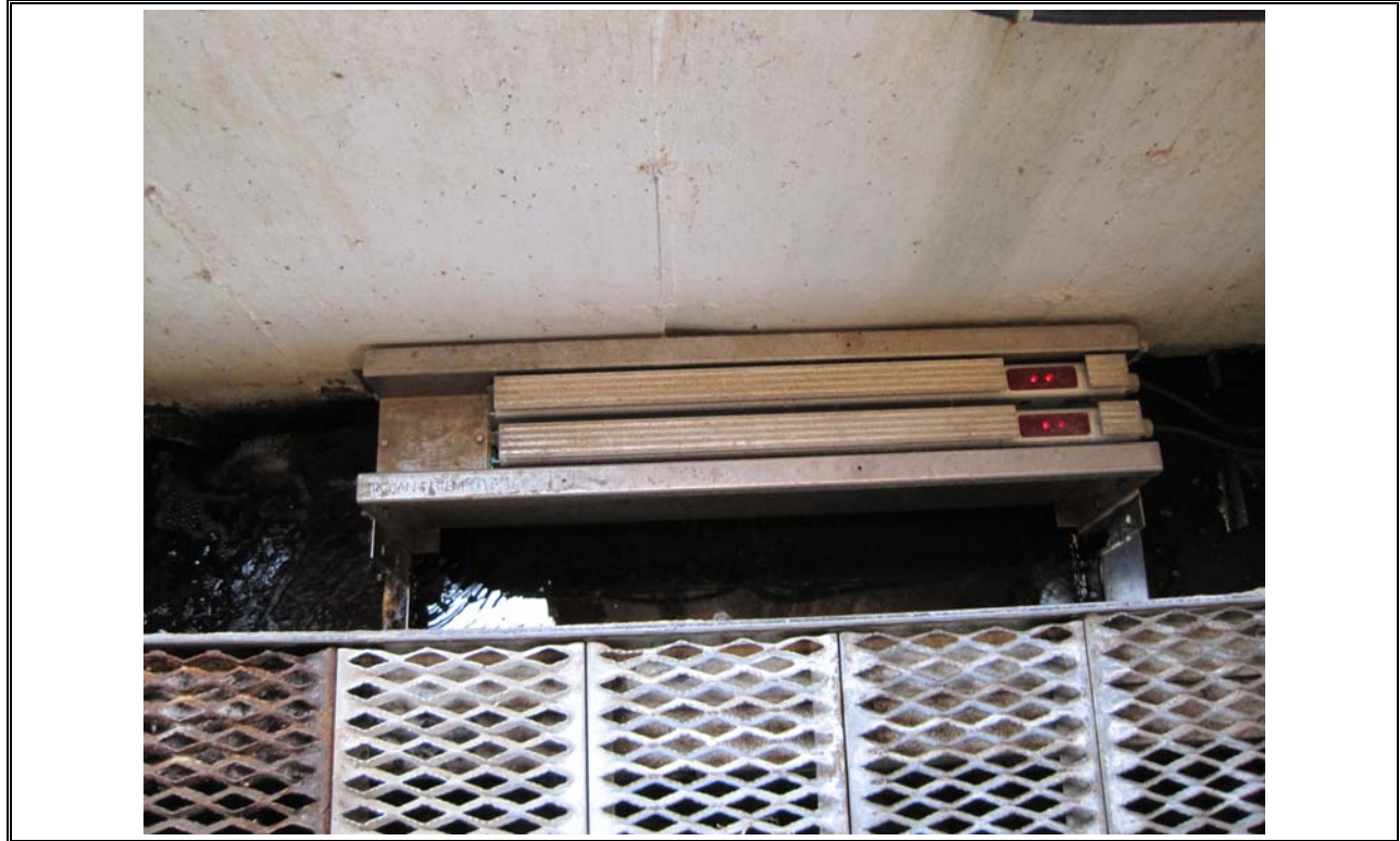
Photo 13 Trojan UV Disinfection System
