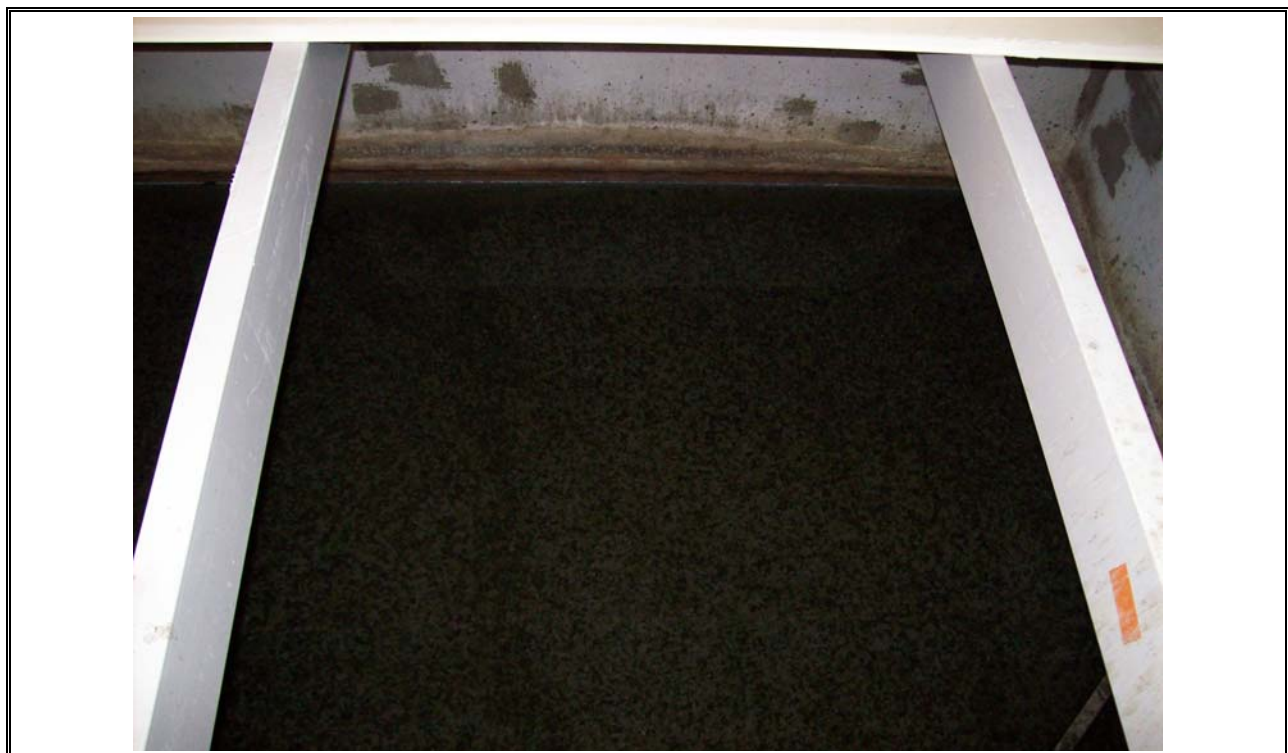
Photo 16 Halifax Densadeg Flocculation Tank
