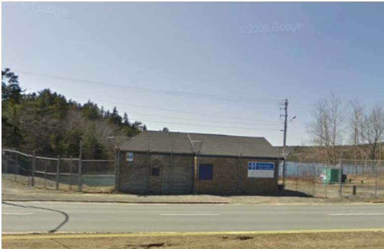
Figure 2.1 Chain Lake Water Supply Plant (Emergency Supply) - Street View
