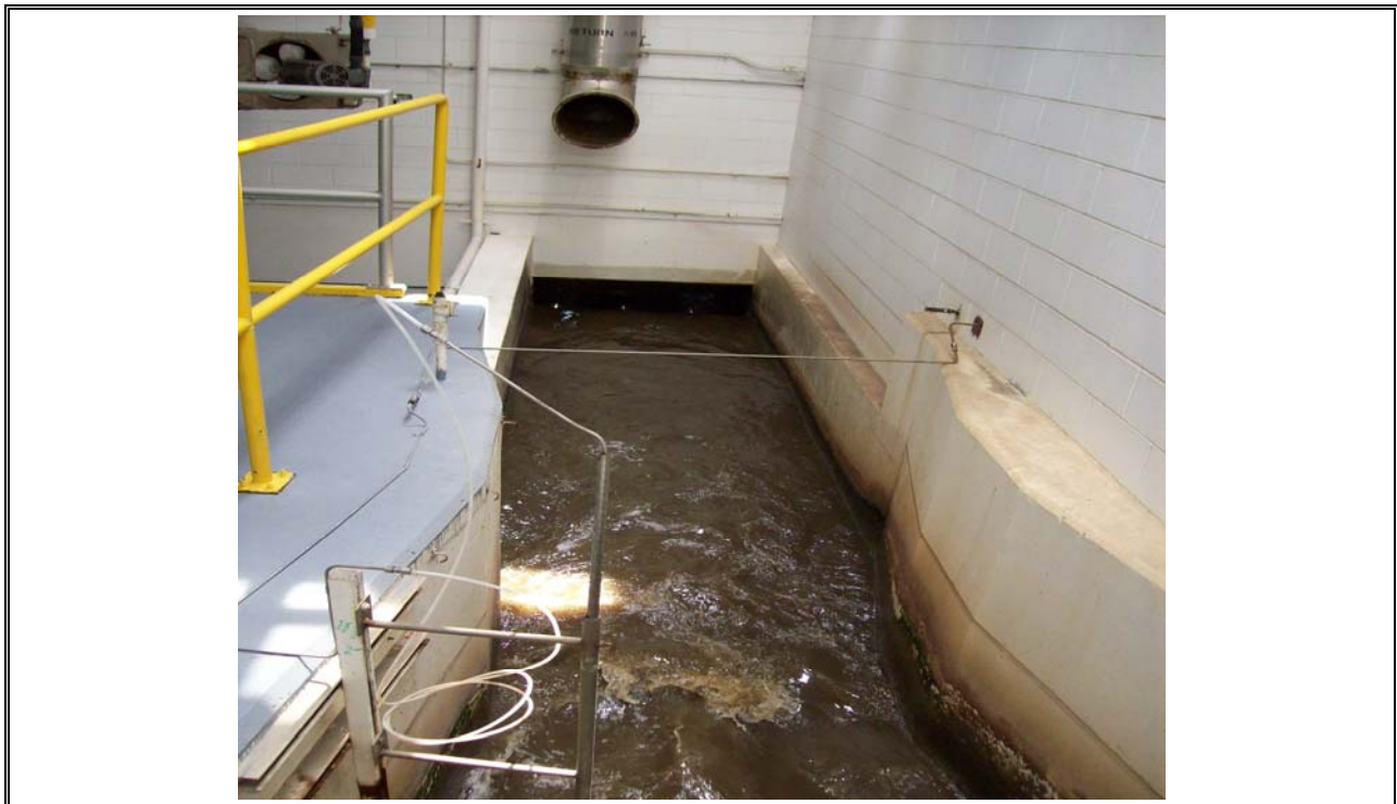
Photo 12 Influent Parshall Flume
