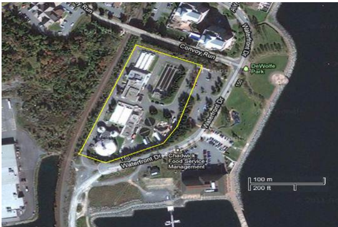
Figure 2.1 Mill Cove WWTF - Aerial View
