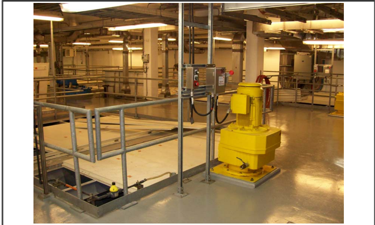
Photo 15 Halifax Densadeg Flocculation Tank Below Slab
