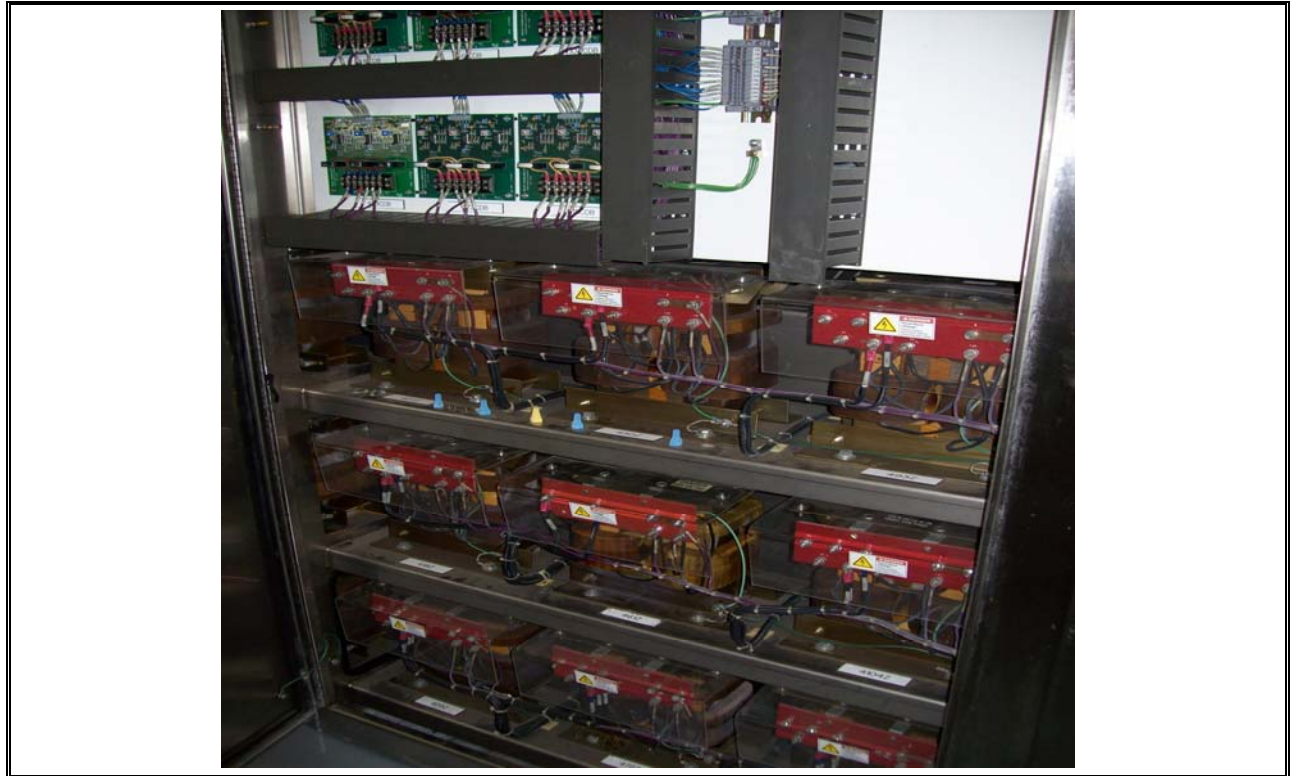
Photo 41 UV Disinfection System Ballast Electronics
