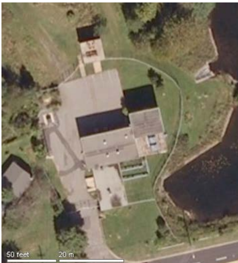
Figure 2.4 Lake Lamont Water Supply Plant (Emergency Supply) - Aerial View
