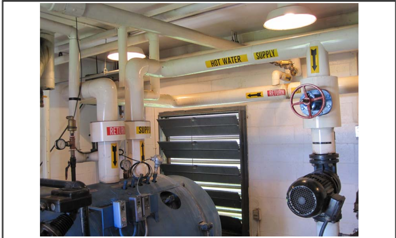
Photo 33 Eastern Passage Boiler Piping
