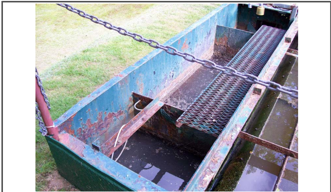
Photo 10 Wellington Effluent Channel and Sodium Hypochlorite Addition Point
