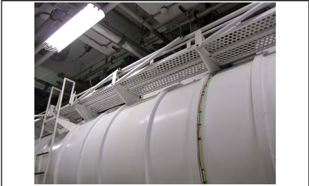
Photo 41 Dartmouth Sludge Loading Area onto Truck
