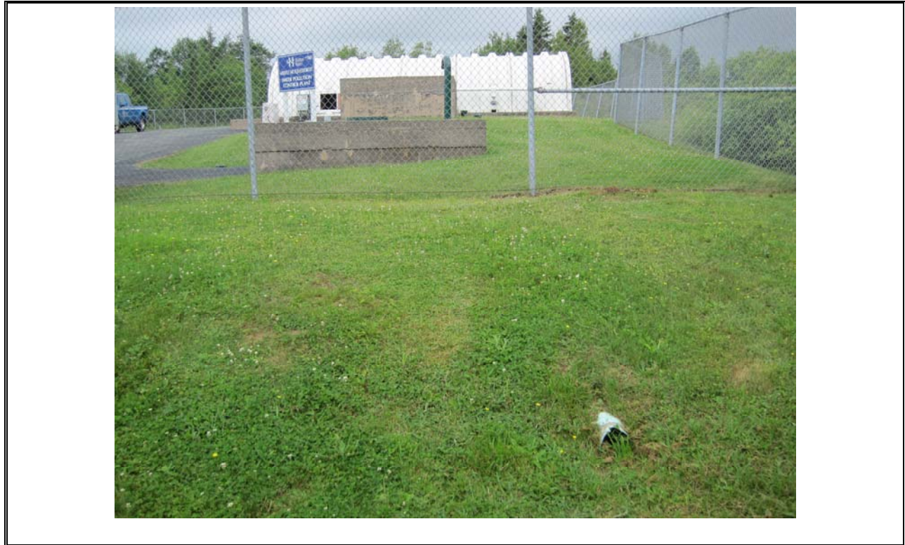
Photo 14 Middle Musquodoboit Overflow Pipe
