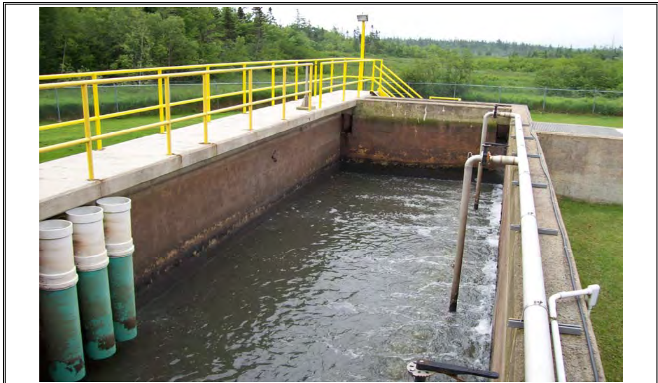
Photo 12 AeroTech Equalization Tank 1
