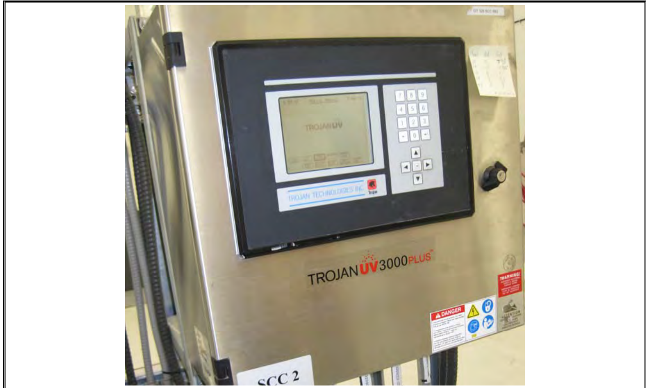
Photo 21 Dartmouth UV Disinfection Control Panel
