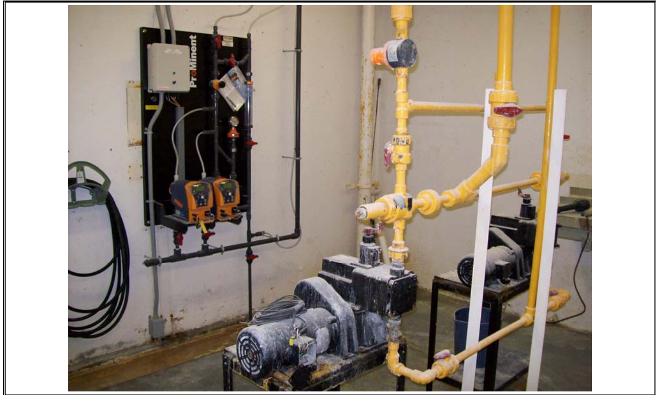
Photo 49 Metering for Lime Addition
