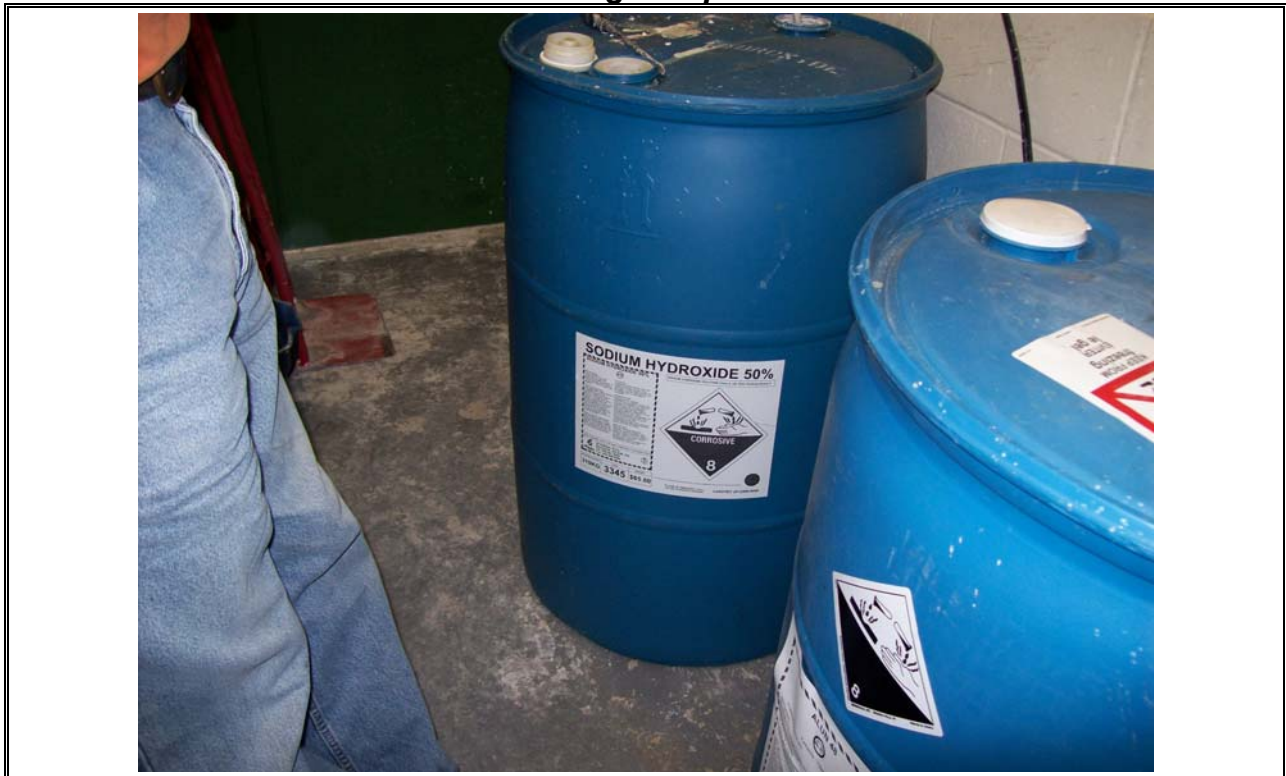
Photo 6 Lockview Caustic Storage Tanks
