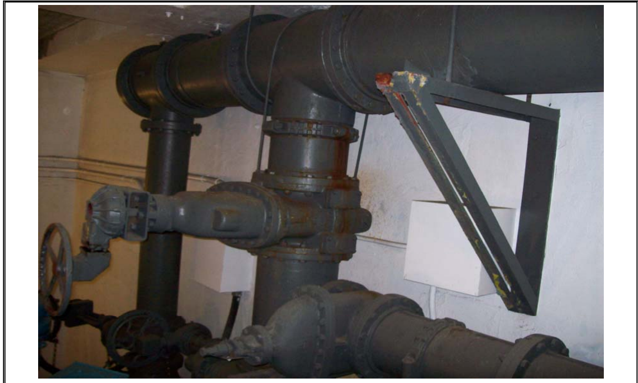
Photo 3 Influent Wastewater Piping
