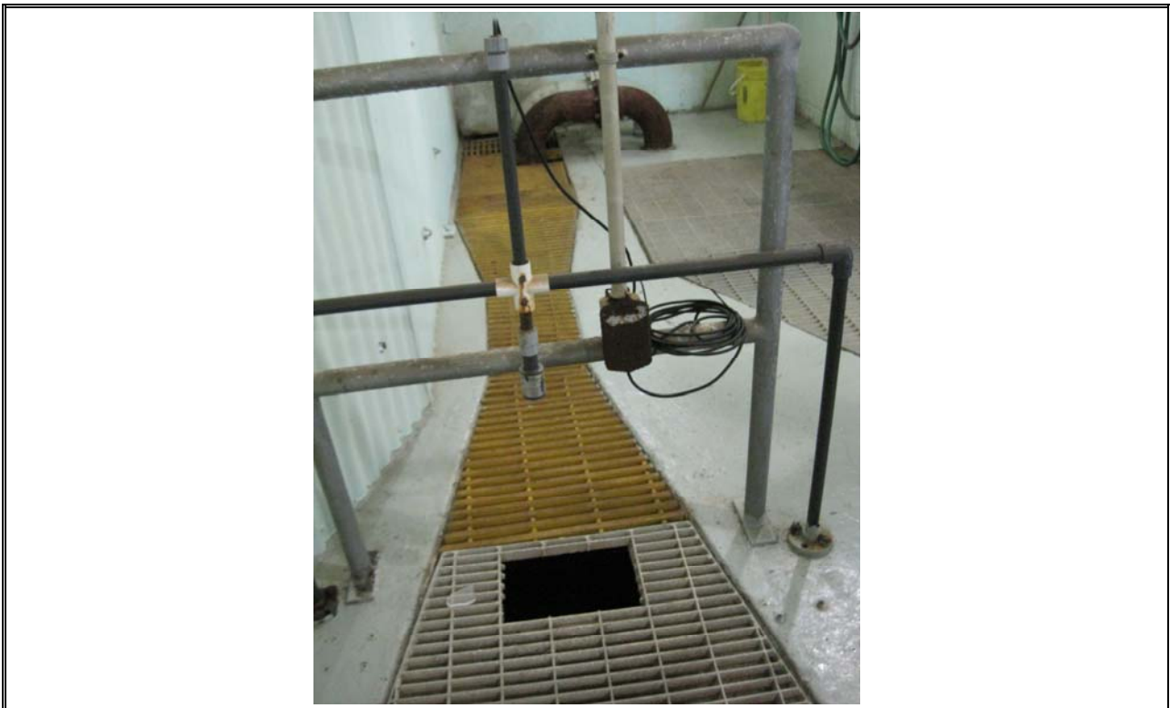
Photo 12 Eastern Passage Parshall Flume
