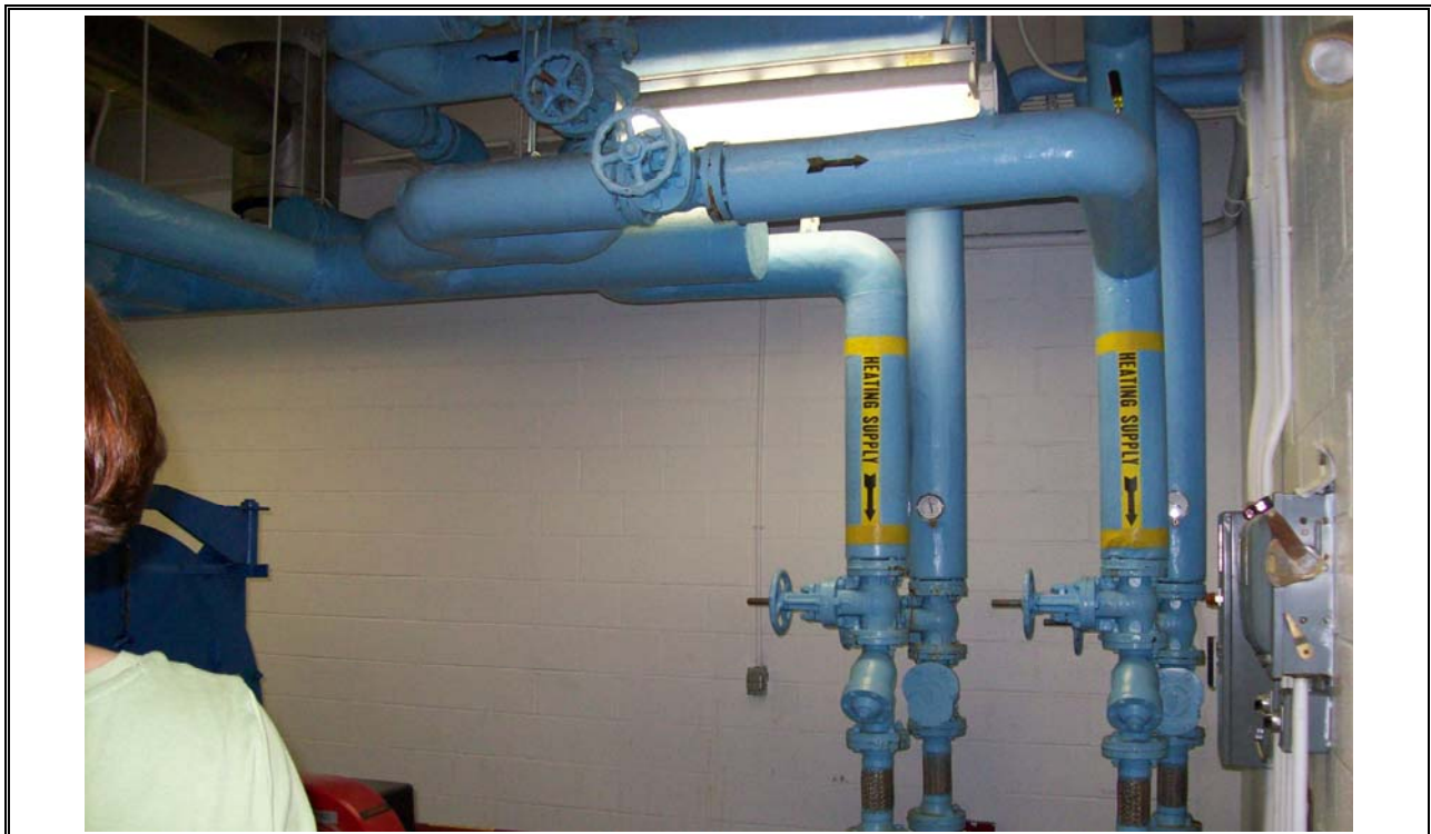
Photo 52 Heating Supply Pipes from Boiler
