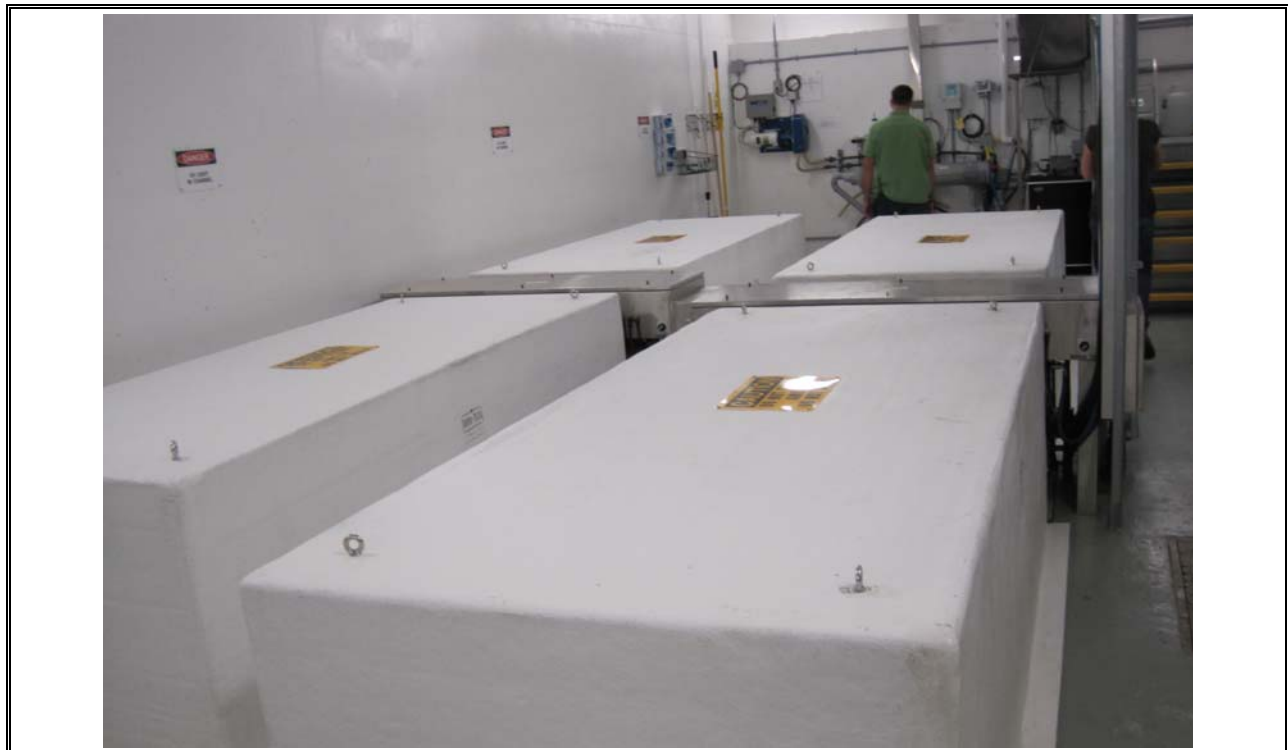
Photo 22 Herring Cove UV Disinfection Channels
