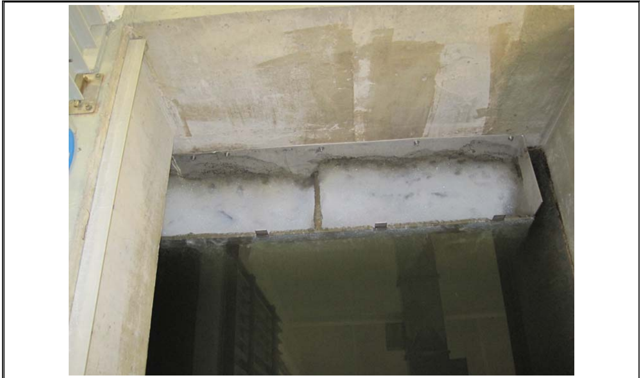
Photo 19 Herring Cove Foaming in Densadeg Effluent Trough
