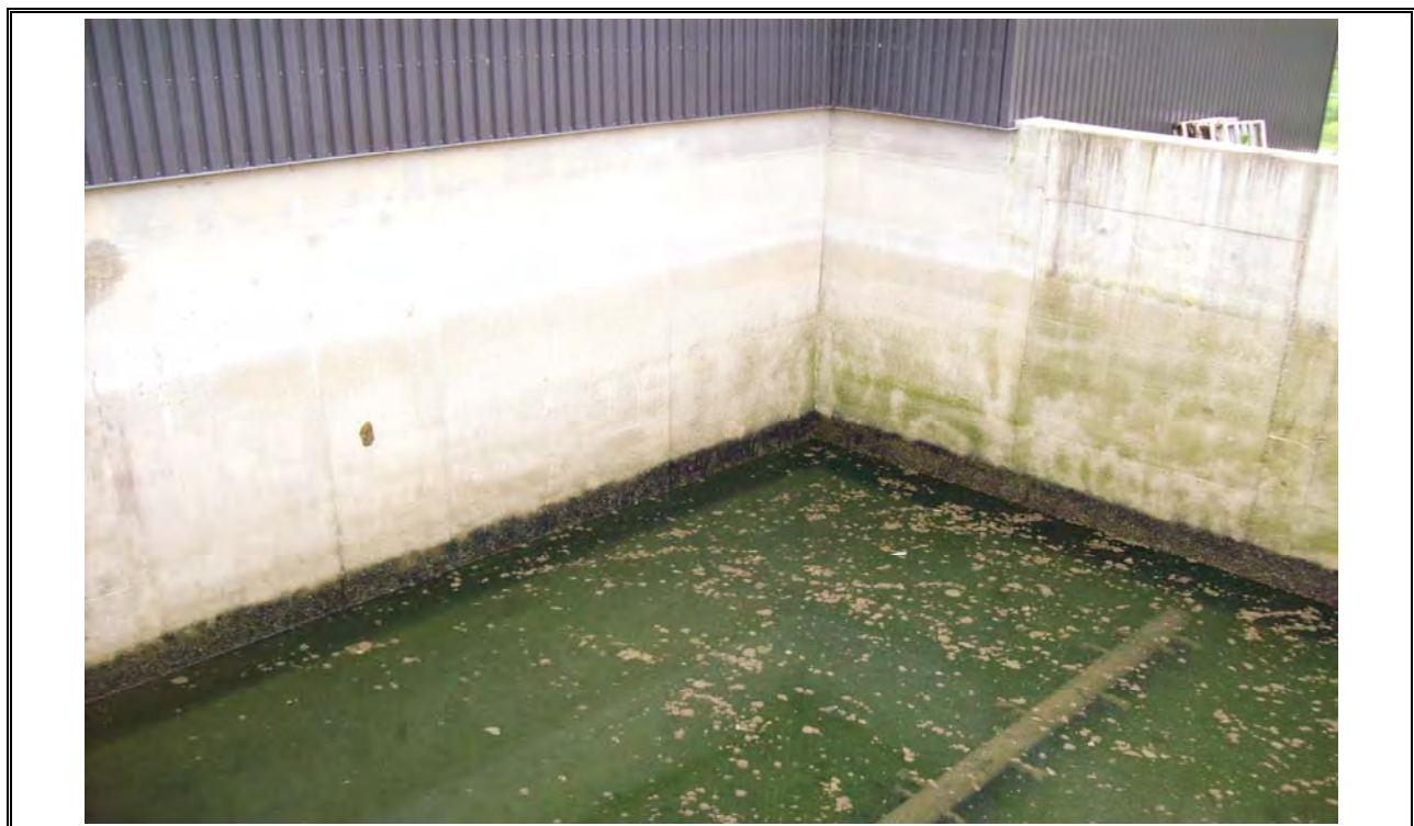
Photo 16 AeroTech post Equalization Tank
