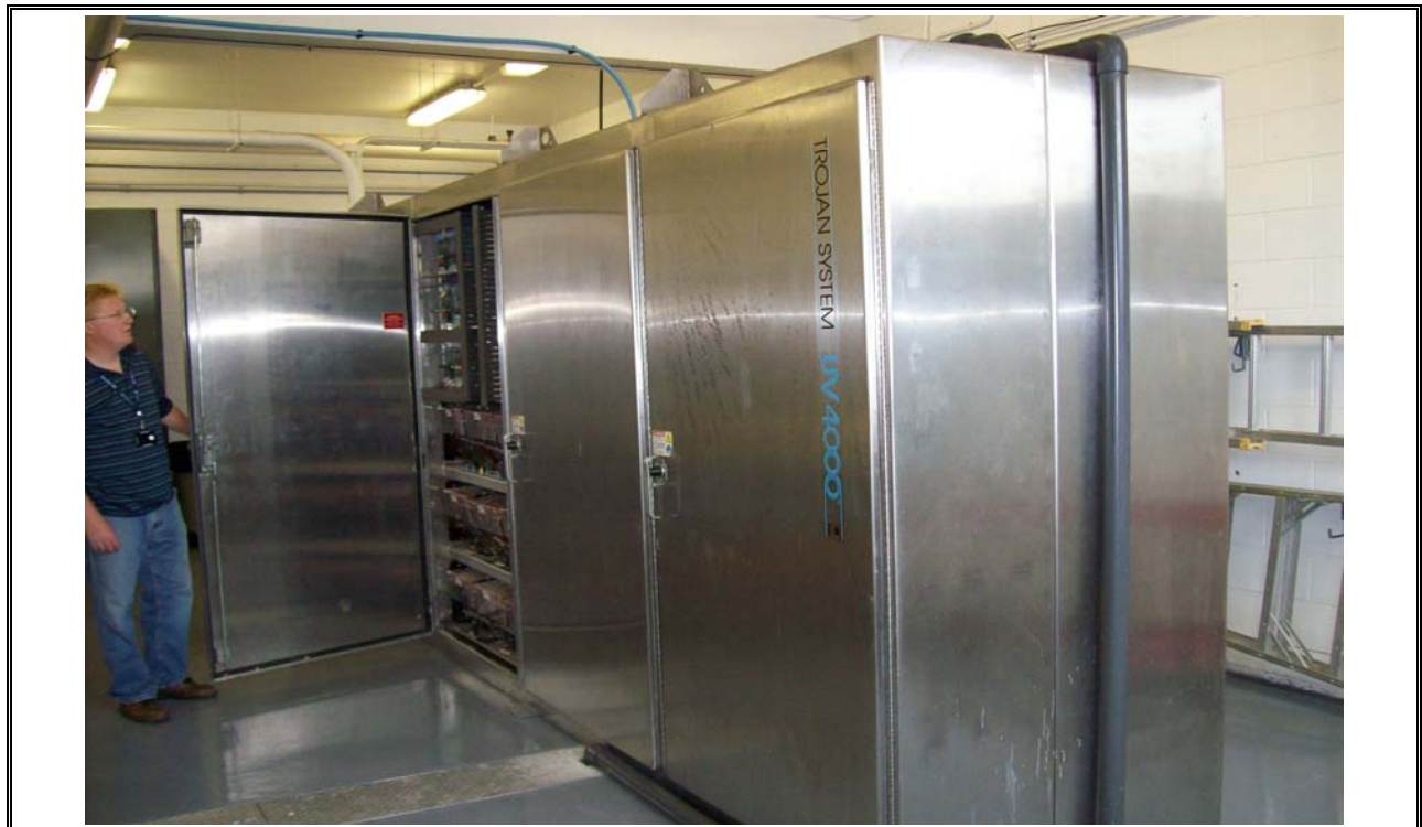
Photo 42 UV Disinfection System Ballasts
