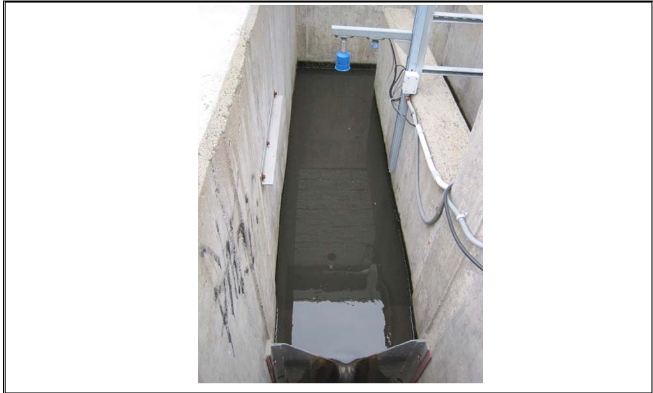
Photo 19 Effluent V-Notch Weir and Ultrasonic
