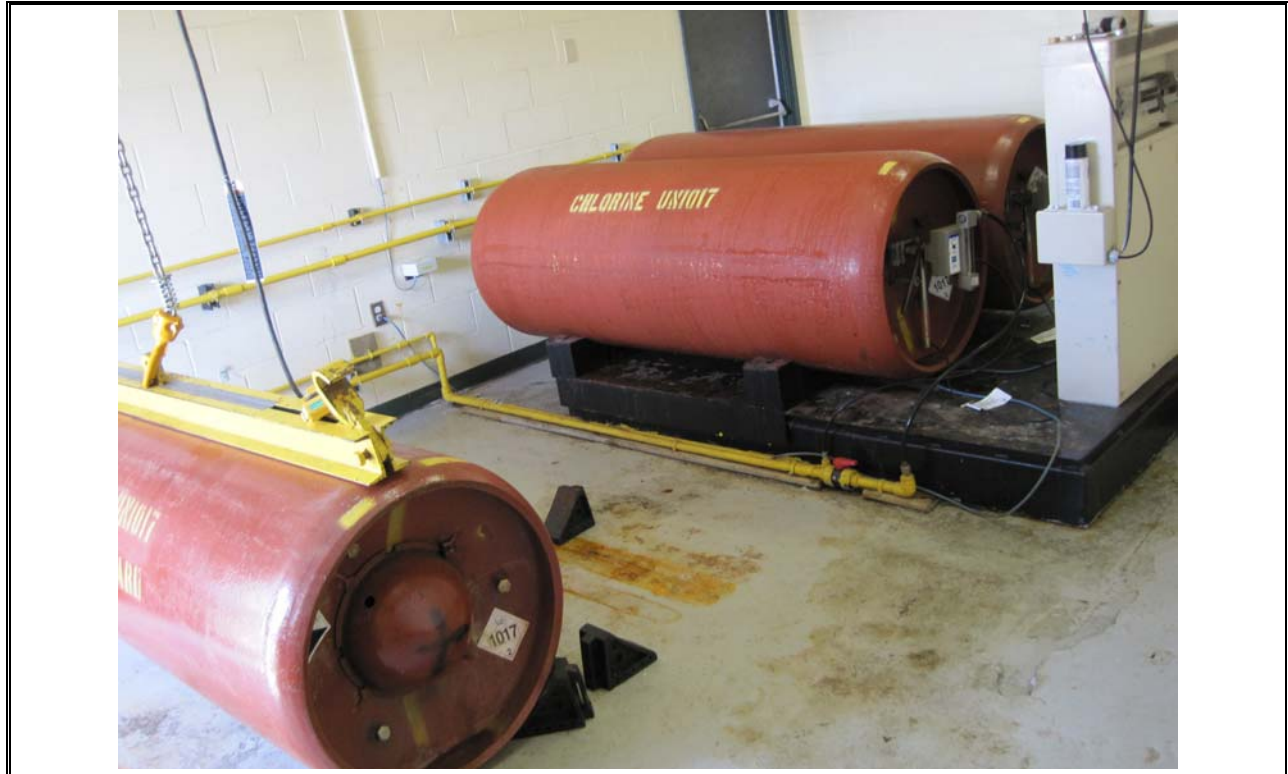
Photo 27 Eastern Passage Chlorine Gas Storage
