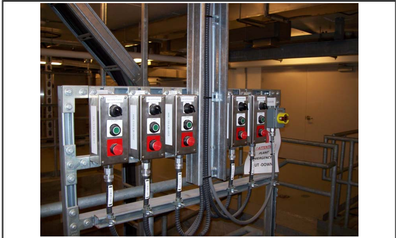
Photo 3 Halifax Control Panels for Raw Wastewater Pumps
