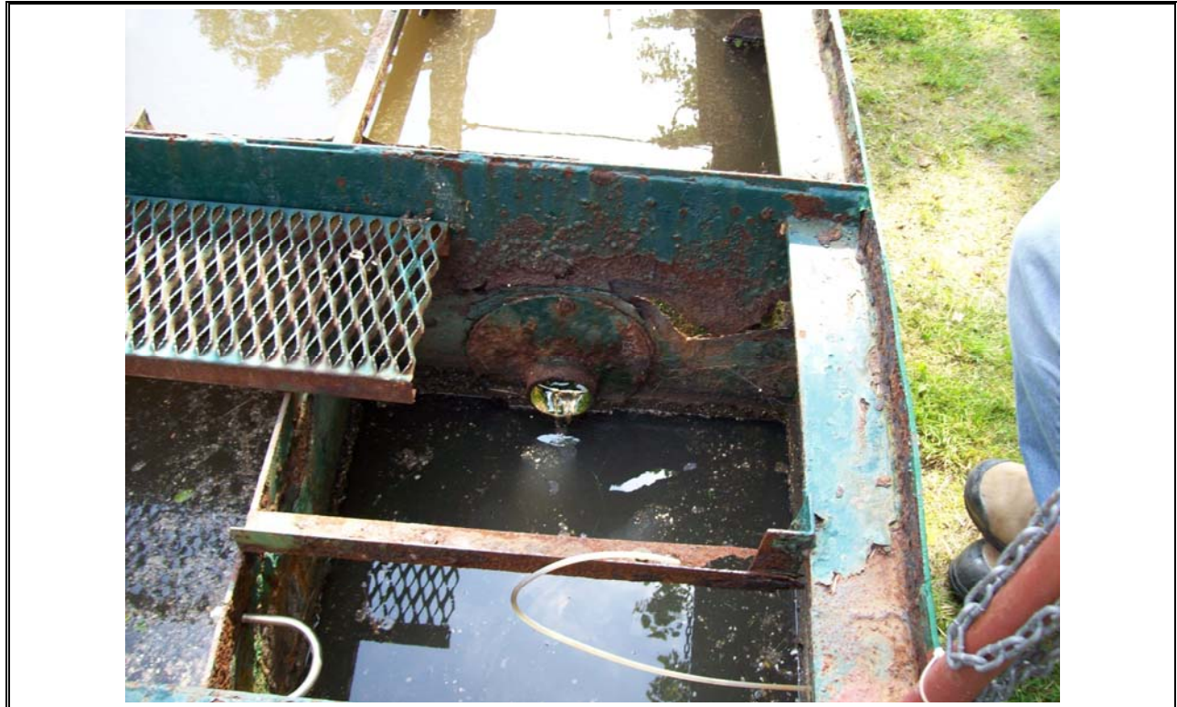
Photo 9 Wellington Effluent Channel and Sodium Hypochlorite Addition Point
