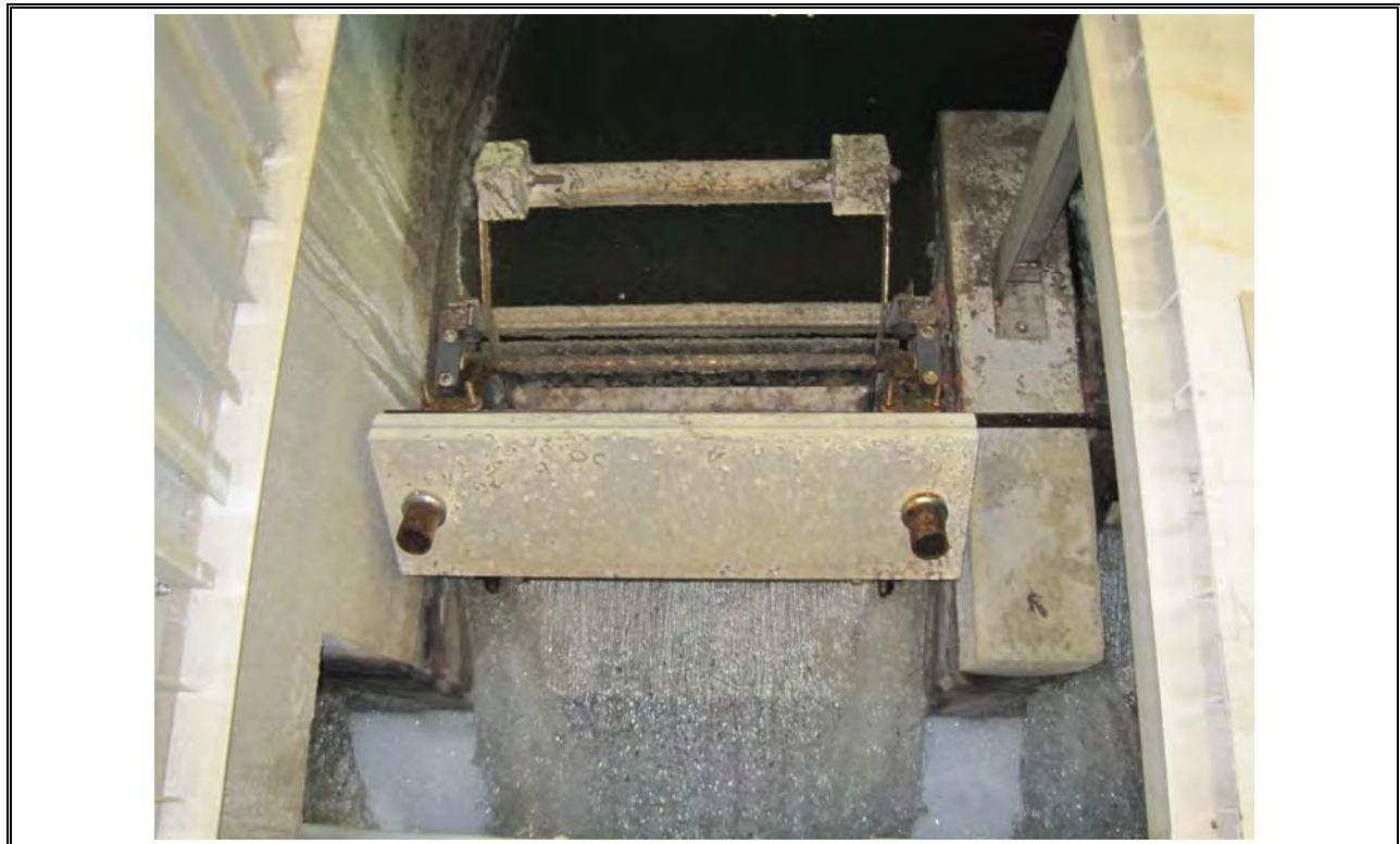
Photo 24 Dartmouth Final Effluent Downstream of UV Disinfection
