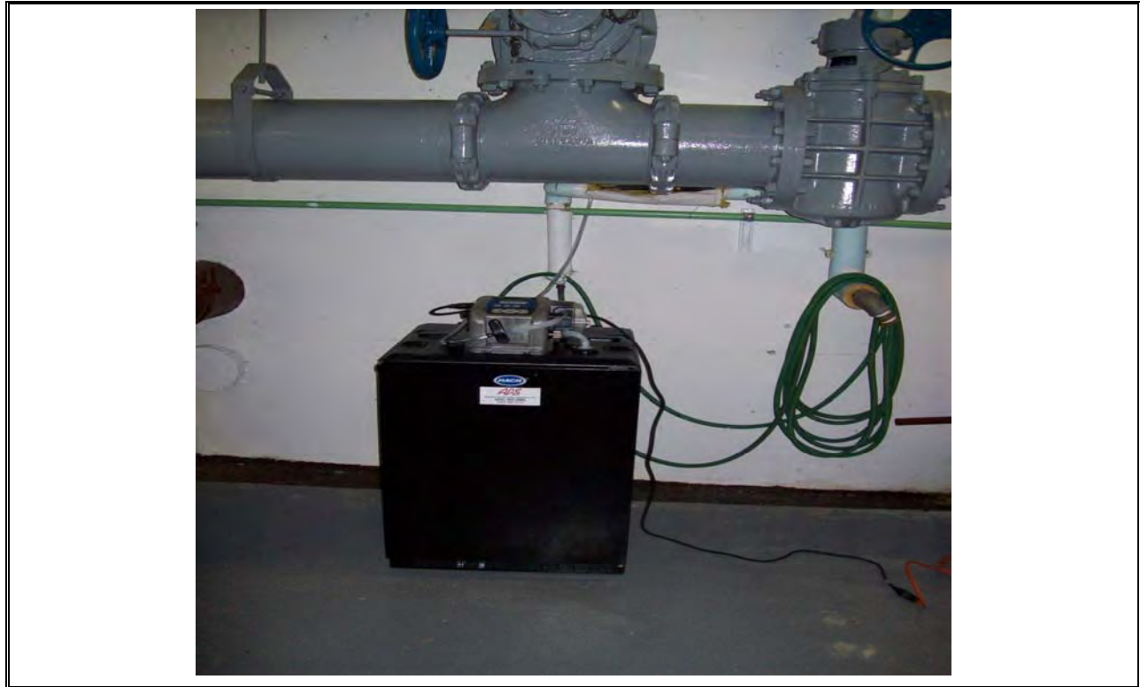
Photo 11 AeroTech Raw Wastewater Autosampler
