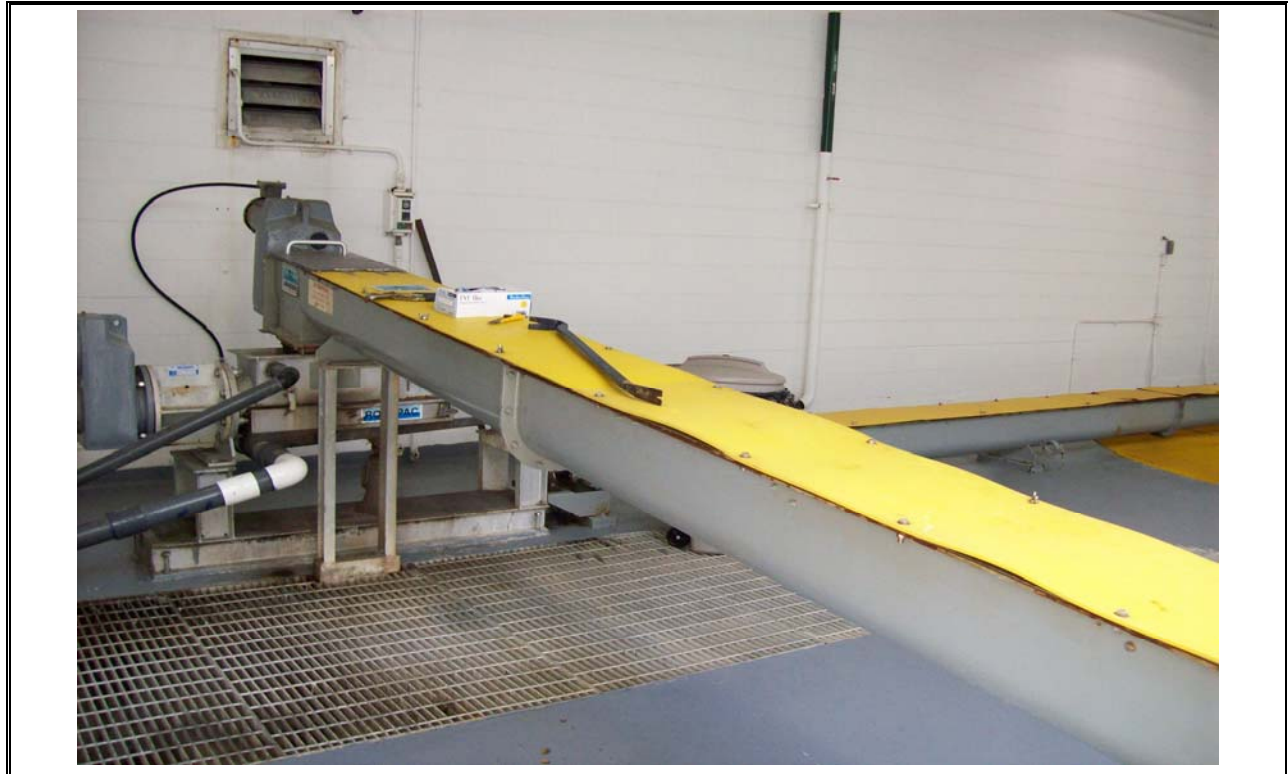
Photo 7 Screenings Classifier and Dewatering
