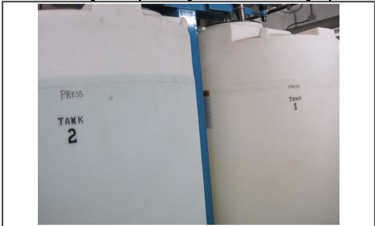
Photo 30 Herring Cove Polymer Storage Containers for Rotary Press Polymer
