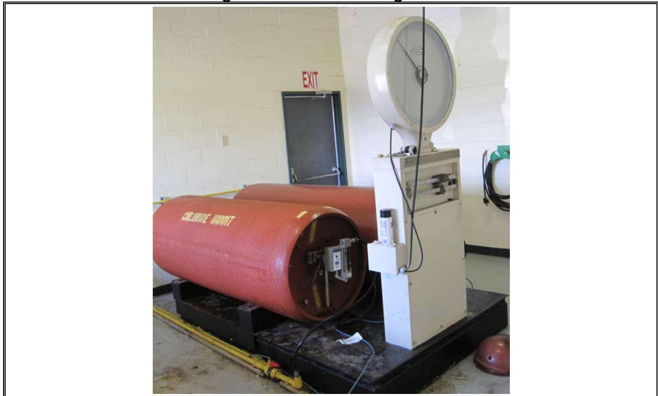
Photo 28 Eastern Passage Chlorine Gas Storage
