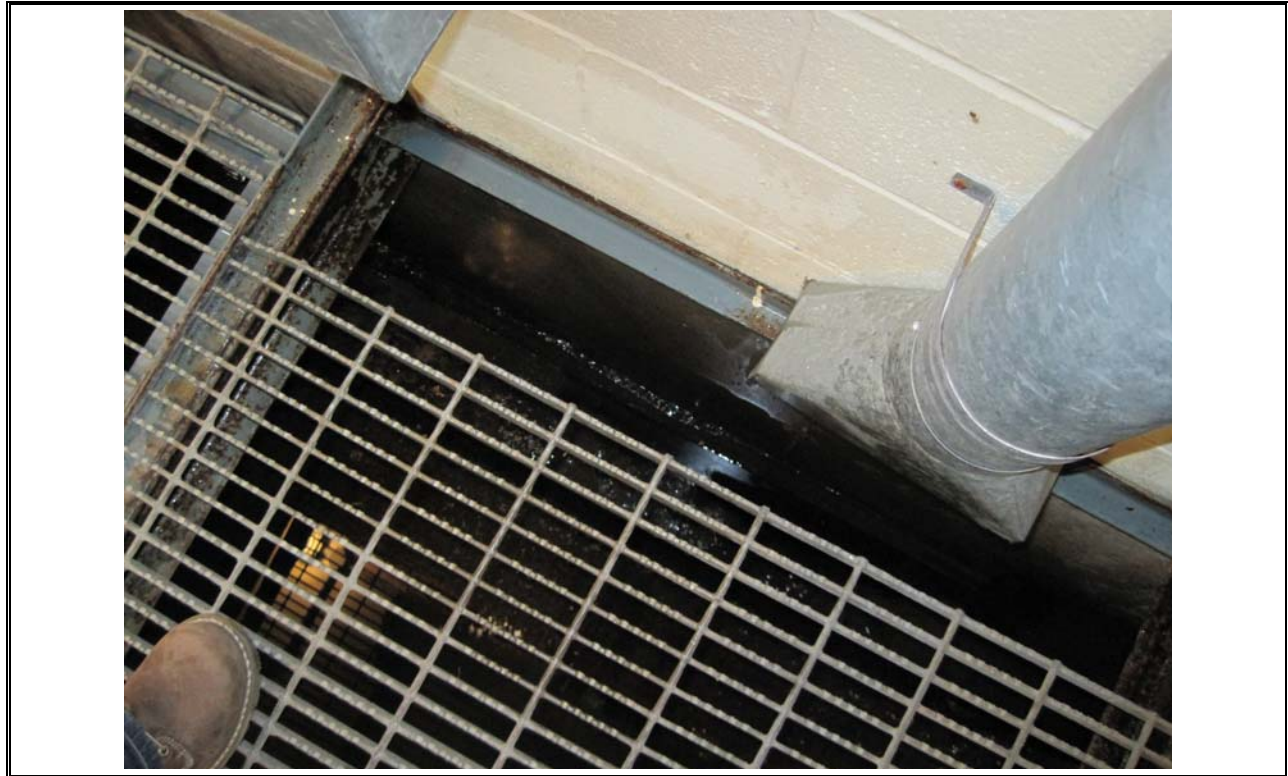
Photo 15 Secondary Clarifier Influent from Aeration Tank
