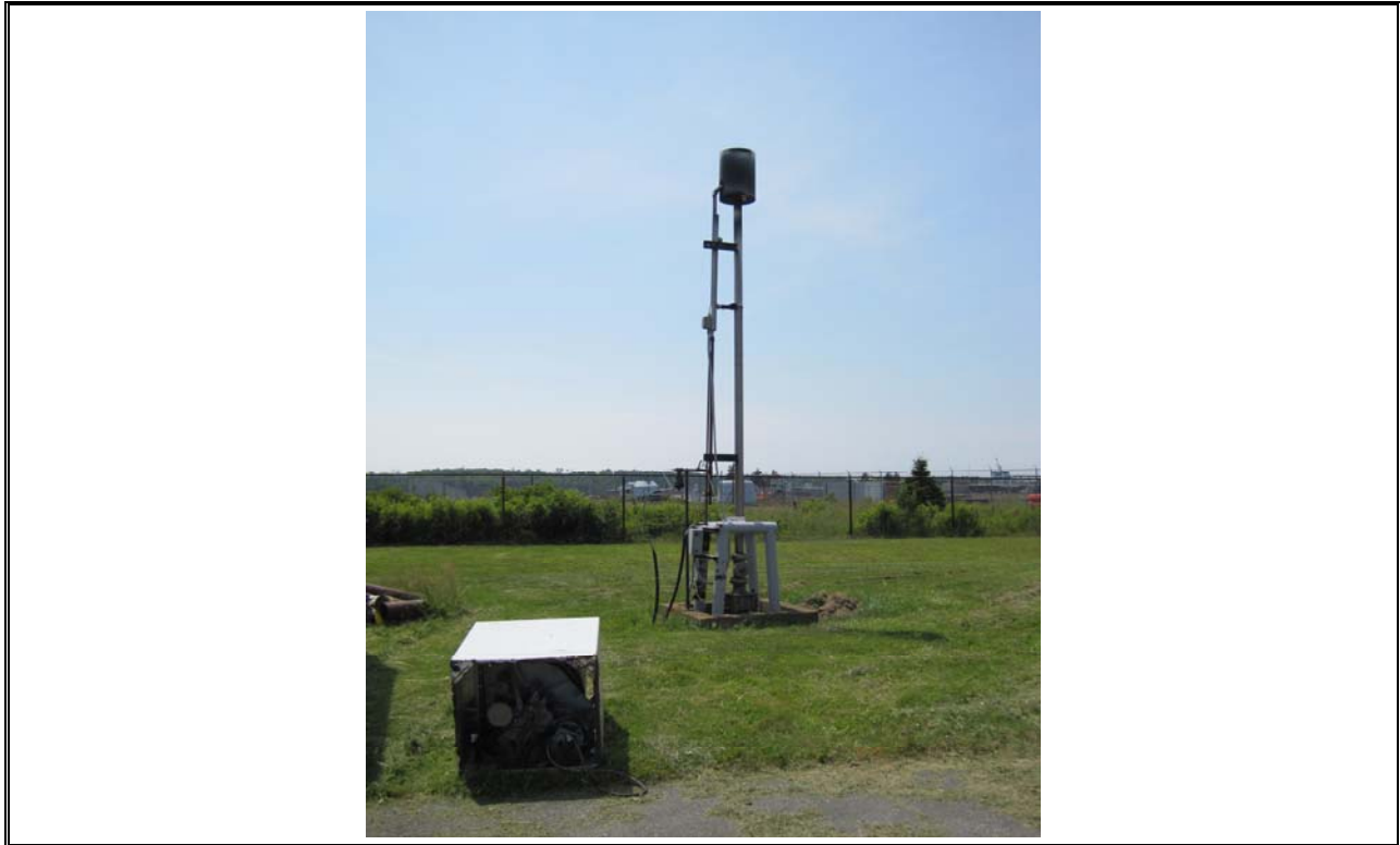
Photo 31 Eastern Passage Digester Flare
