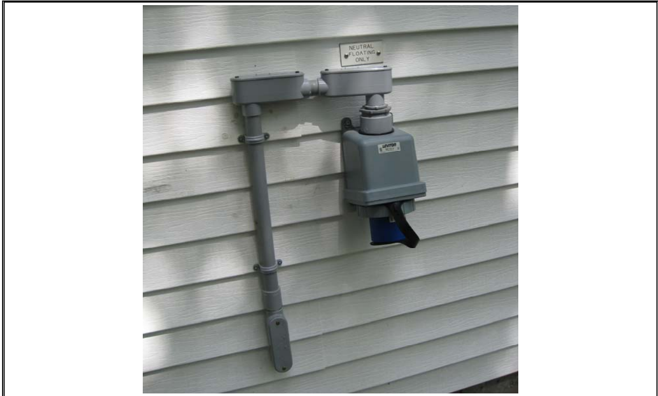
Photo 23 Uplands Park Hook-up for Portable Generator outside UV building
