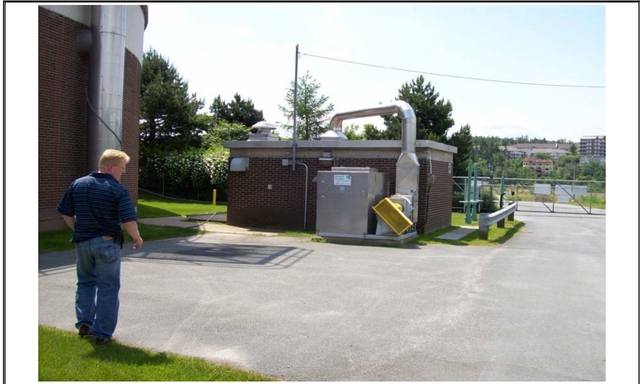
Photo 1 Mill Cove Influent Pumping Station
