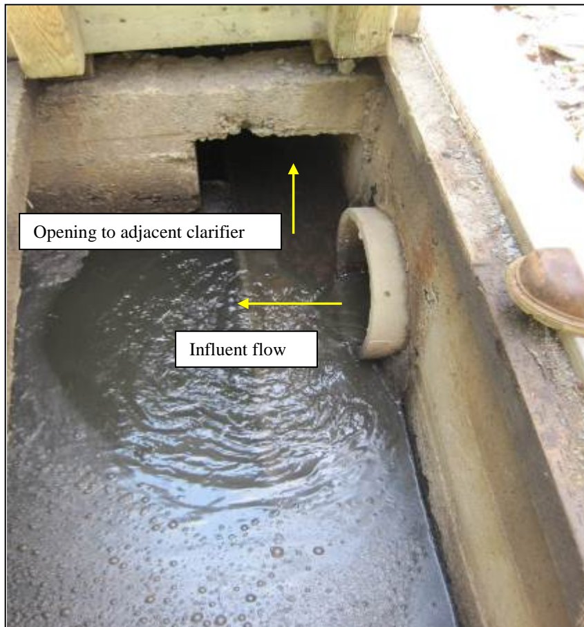
Figure 3.1 Flow splitting issues in clarifiers
