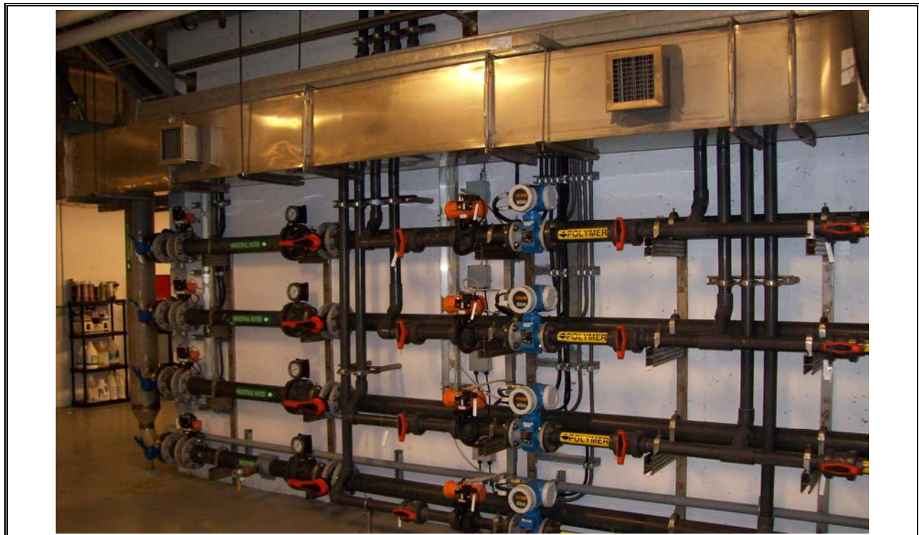
Photo 28 Halifax Densadeg Polymer Feed Lines
