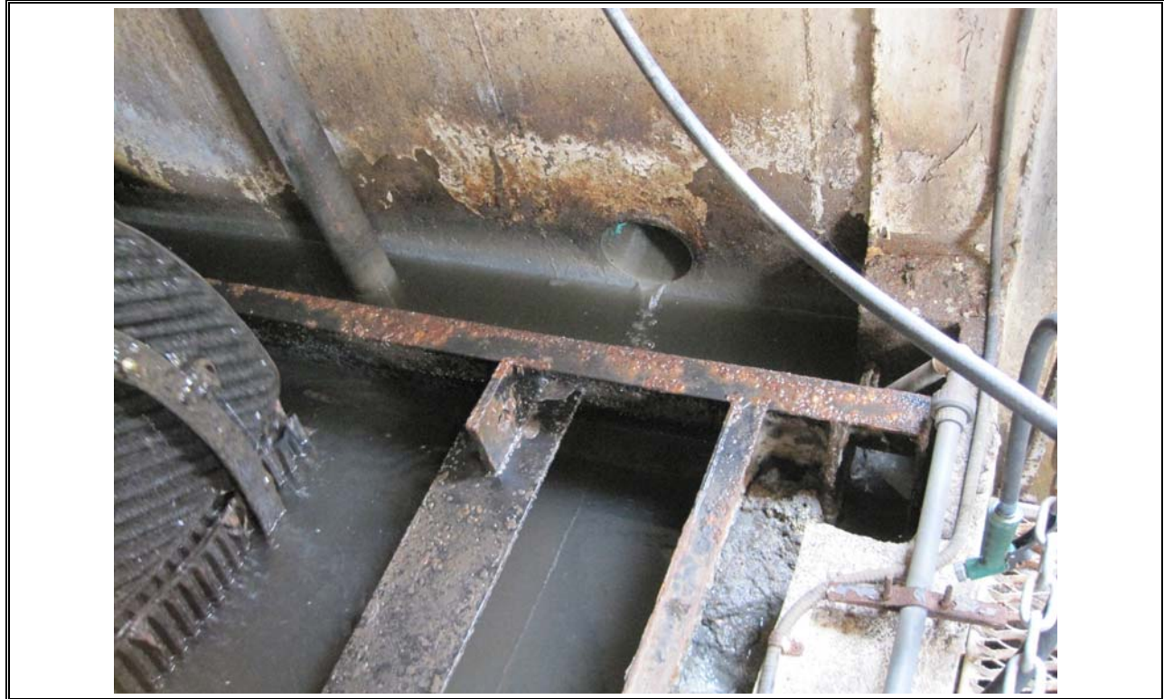
Photo 3 Middle Musquodoboit Flow into Primary Tank from Grit Removal
