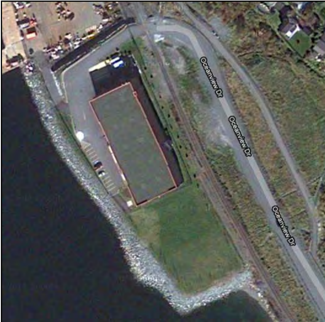
Figure 2.1 Dartmouth WWTF - Aerial View
