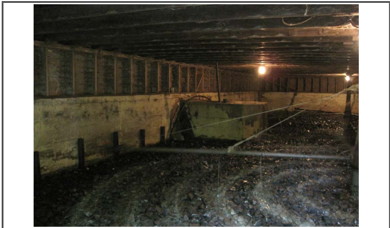
Photo 10 Uplands Park Trickling Filter & Inlet splitter box
