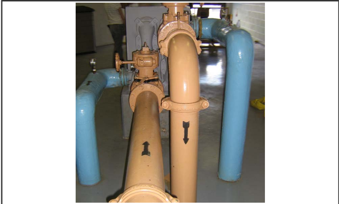
Photo 61 Sludge Recirculation through Heat Exchanger
