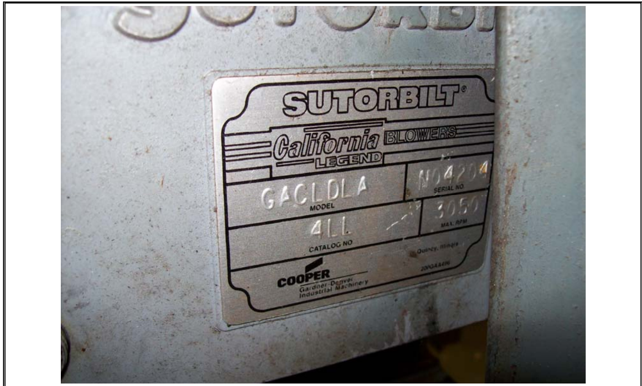
Photo 11 Lockview Blower Nameplate
