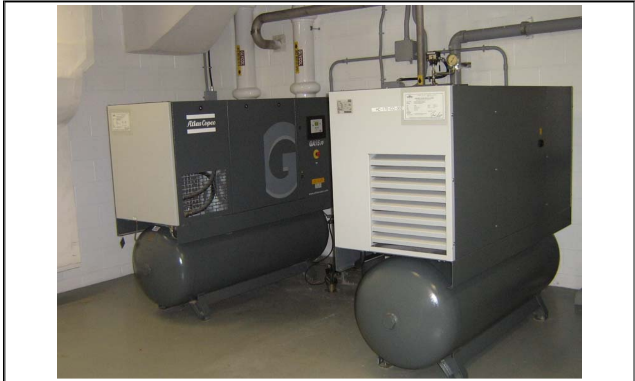
Photo 49 Herring Cove Rotary Screw Pump Compressors
