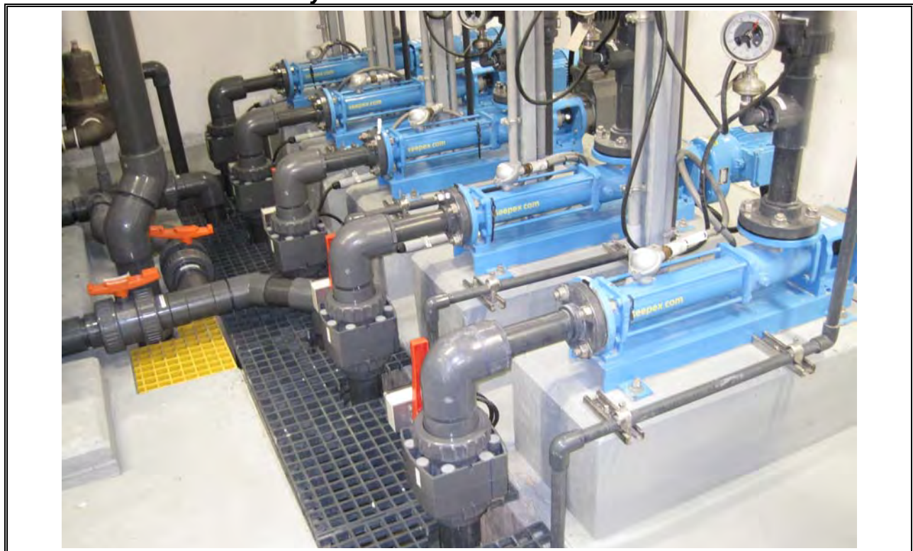
Photo 34 Dartmouth Polymer Pumps
