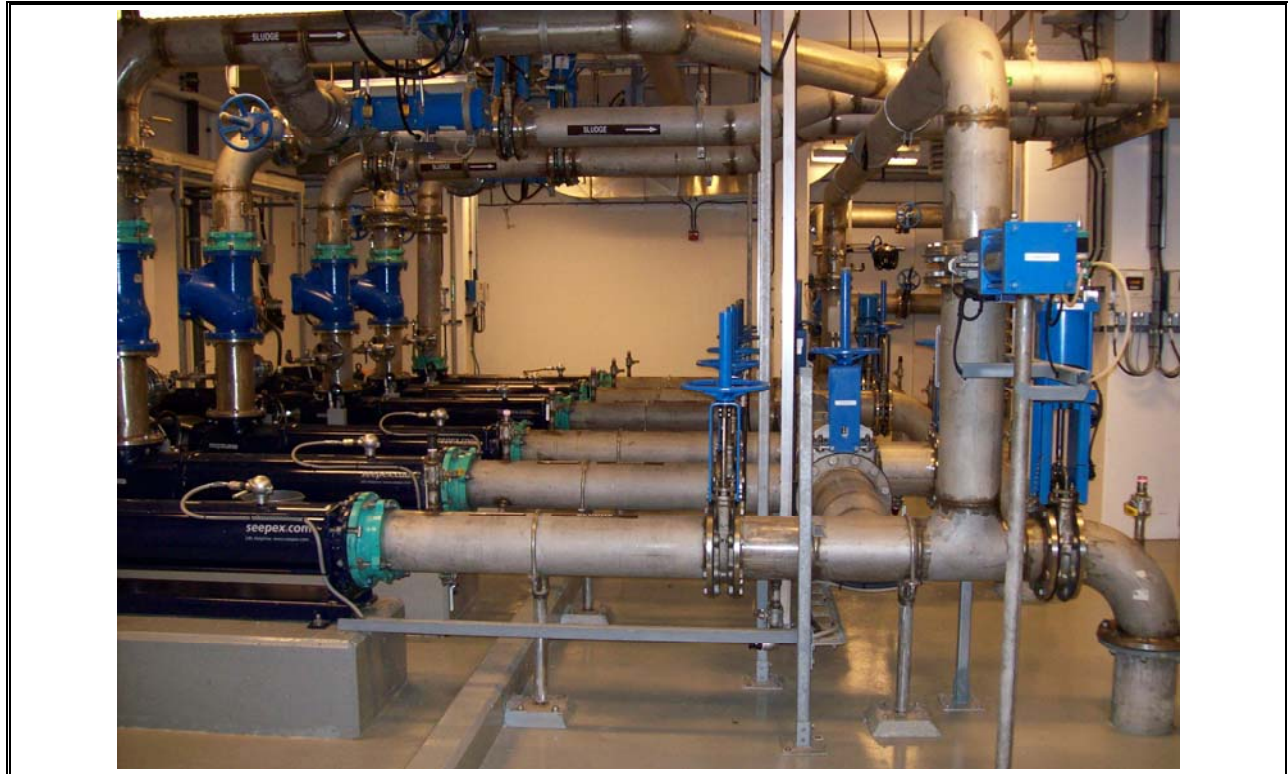
Photo 21 Halifax Densadeg Sludge Pumps
