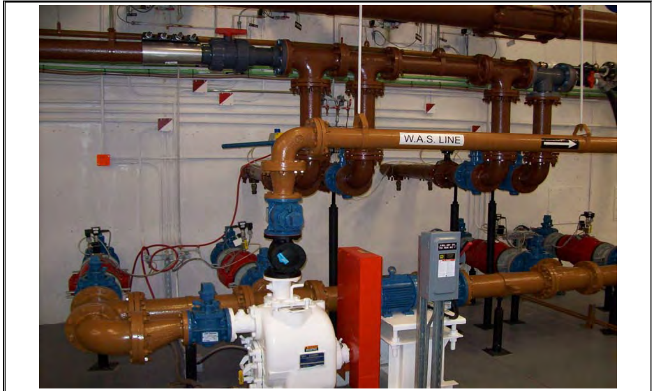
Photo 25 AeroTech SBR WAS Lines and Pump
