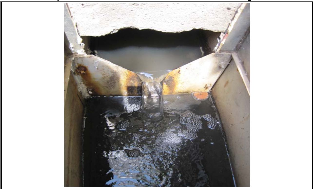
Photo 22 Uplands Park V-Notch Weir Following Old Chlorination Building
