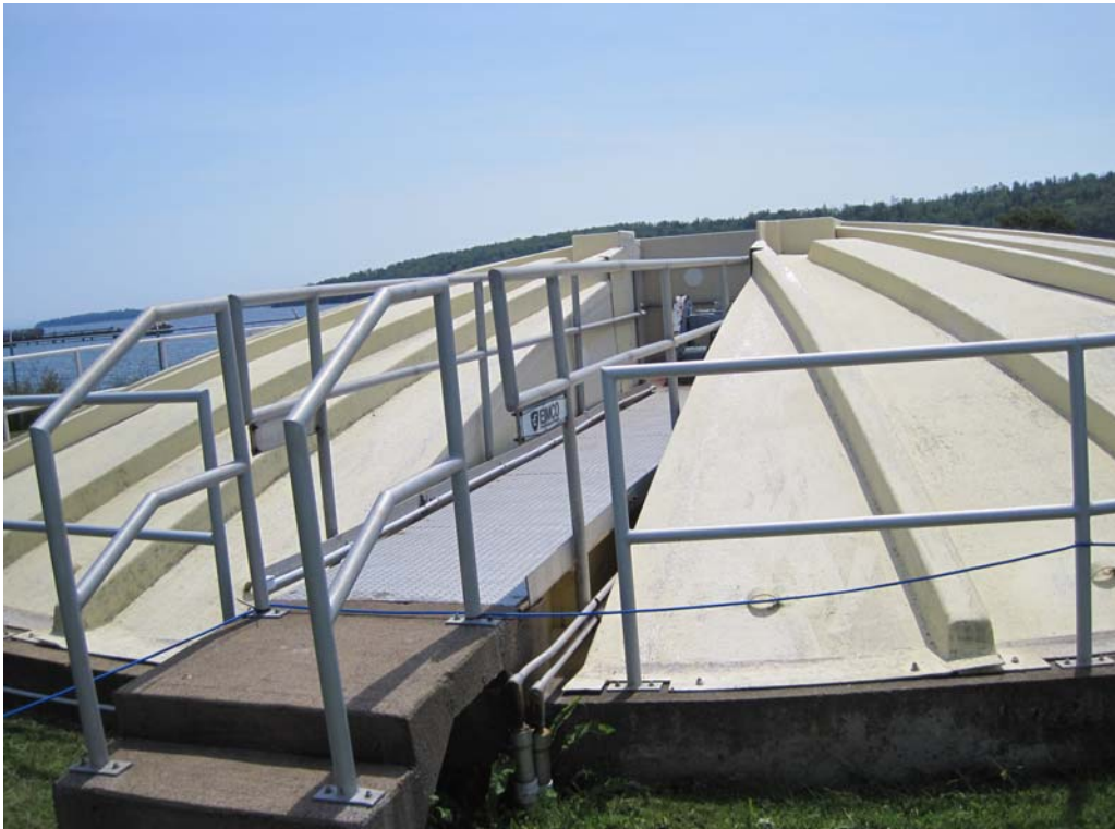
Photo 20 Eastern Passage Circular Chlorine Contact Chamber
