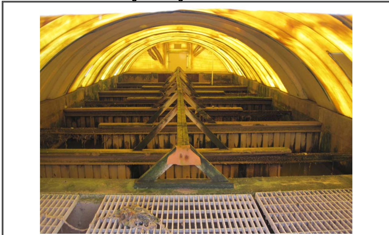
Photo 24 Eastern Passage Rectangular Chlorine Contact Tank
