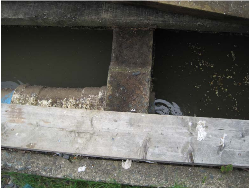
Photo 7 Uplands Park Uneven Primary Flow Split
