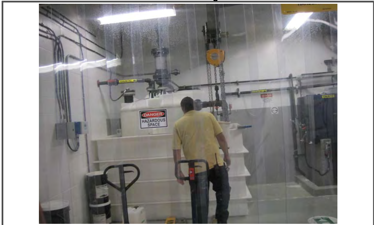
Photo 32 Dartmouth Caustic Storage
