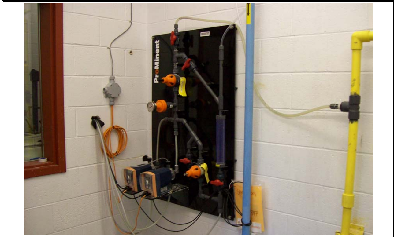
Photo 47 Hypochlorite Chemical Metering
