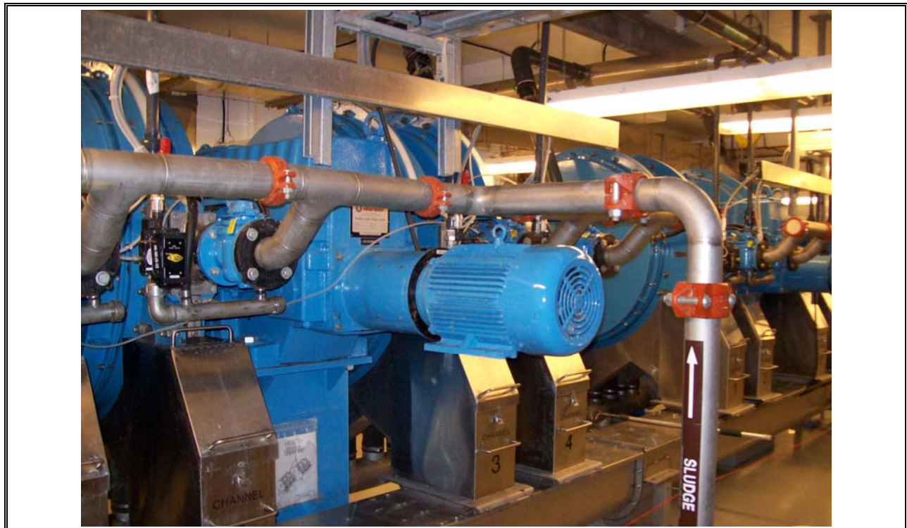
Photo 34 Halifax Fournier Rotary Presses
