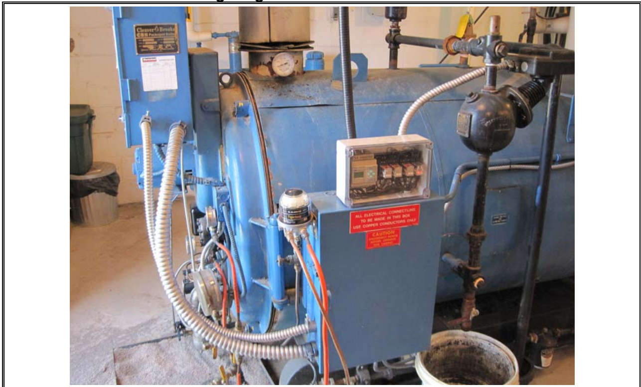
Photo 32 Eastern Passage Boiler
