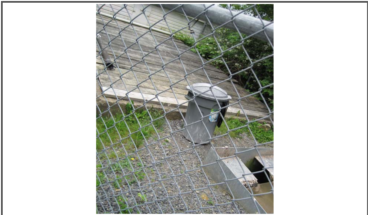
Photo 2 Uplands Park Bar Screening and Primary Clarification
