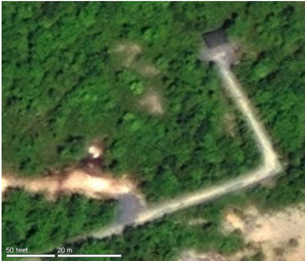
Figure 2.8 Five Island Lake Water Supply Plant - Aerial View
