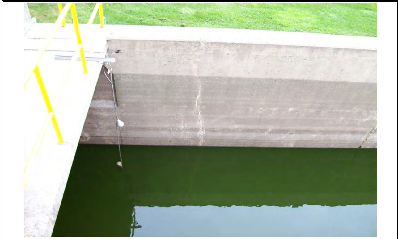
Photo 15 AeroTech Equalization Tank 2
