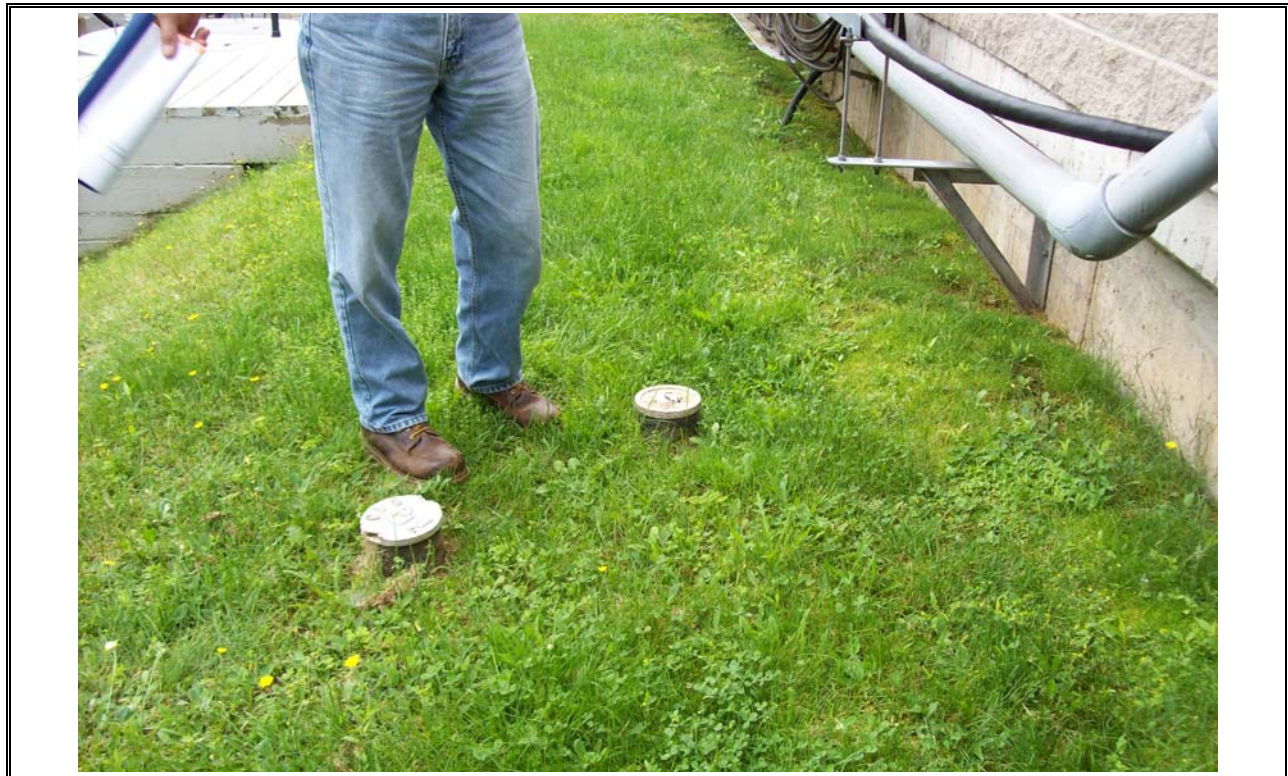
Photo 32 Lockview Valve Stems for Bypass Lines
