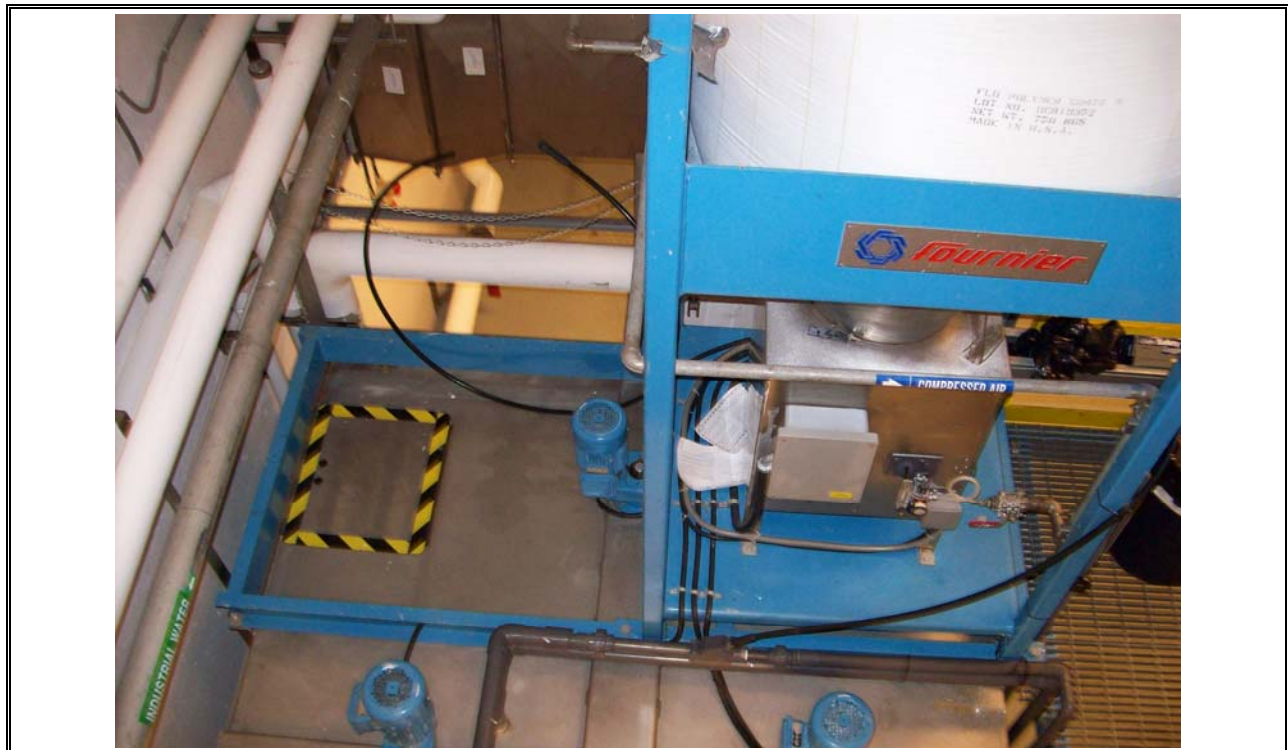
Photo 30 Halifax Rotary Press Polymer Make-Up System
