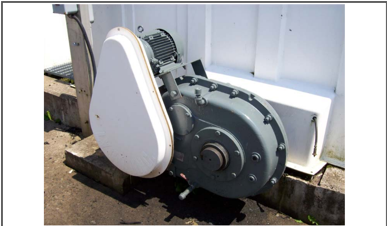
Photo 24 RBC Drive and Bearing Box Connected to RBC Shaft
