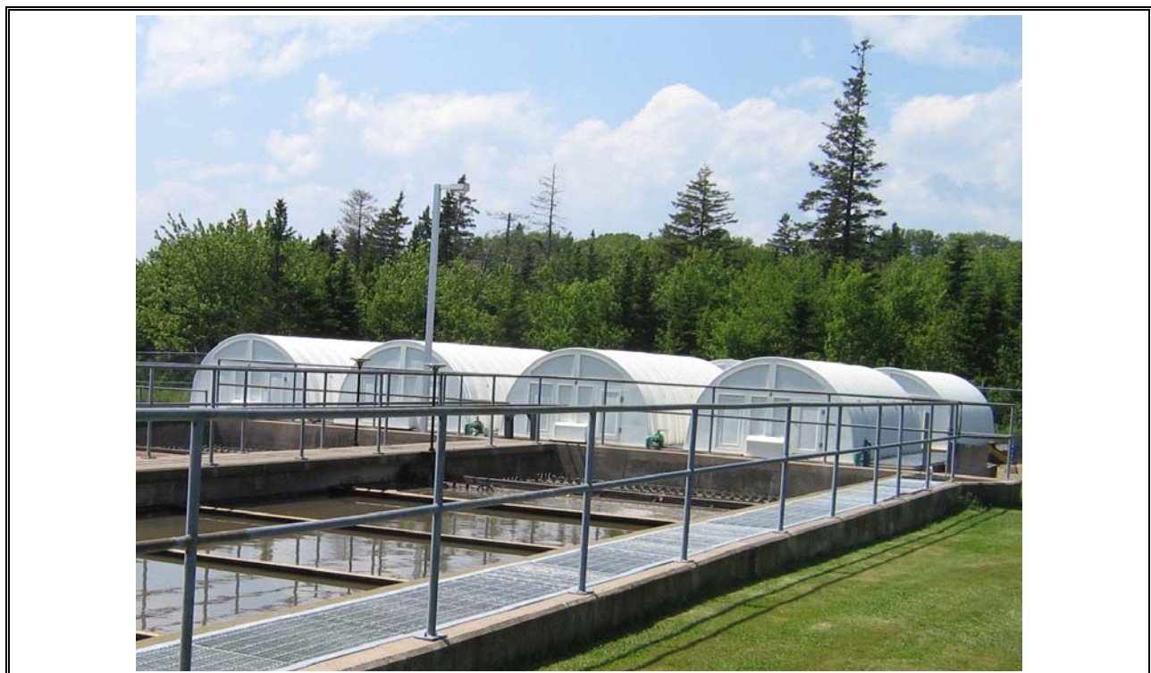
Photo 18 Rotating Biological Contactors (RBCs) – 2 Trains of 4 RBCs
