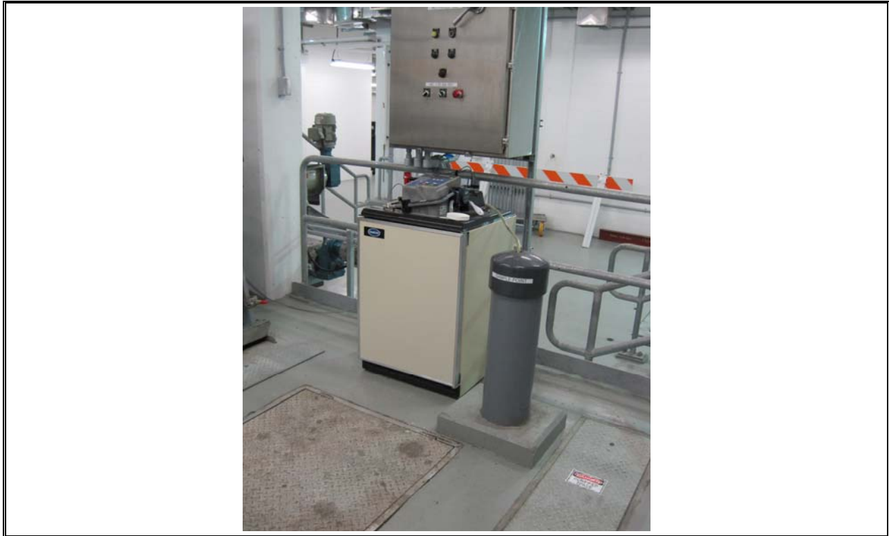
Photo 5 Herring Cove Influent Sampling Point
