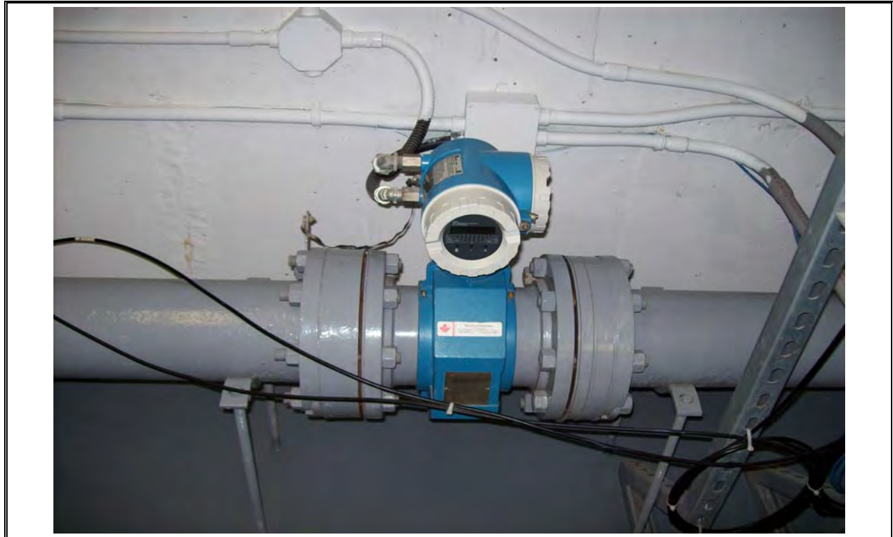
Photo 9 AeroTech Influent Wastewater Magmeter
