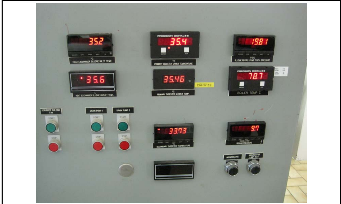
Photo 5 Eastern Passage Operator Control Panel
