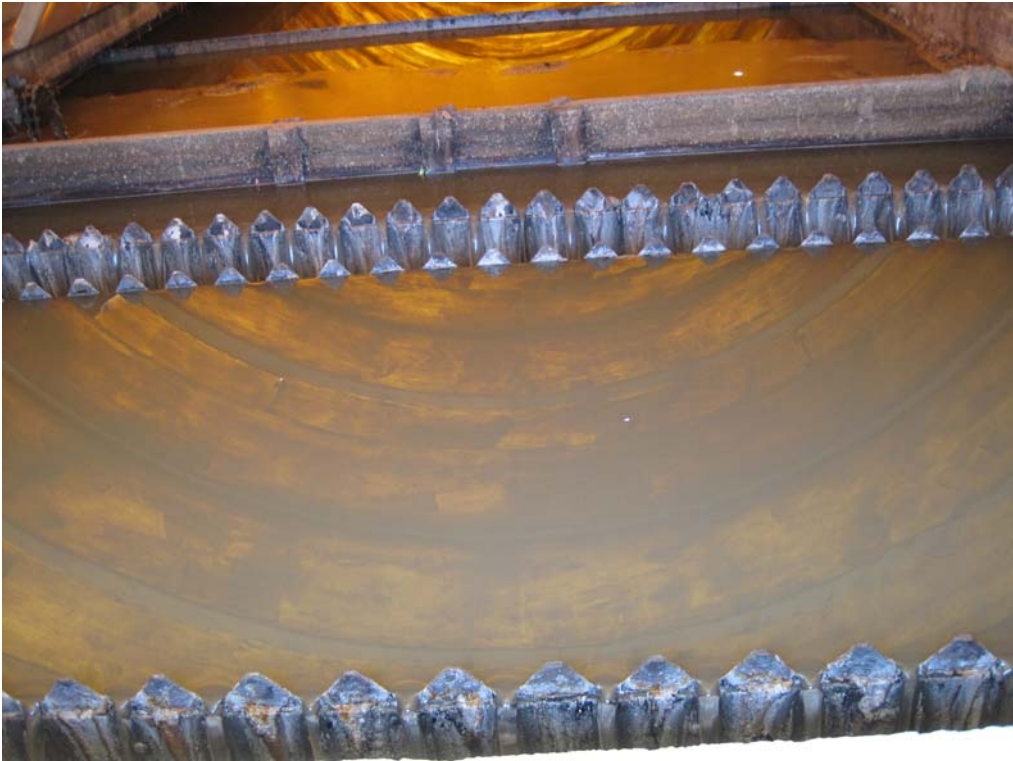
Photo 19 Eastern Passage Primary Clarifier Effluent Weirs
