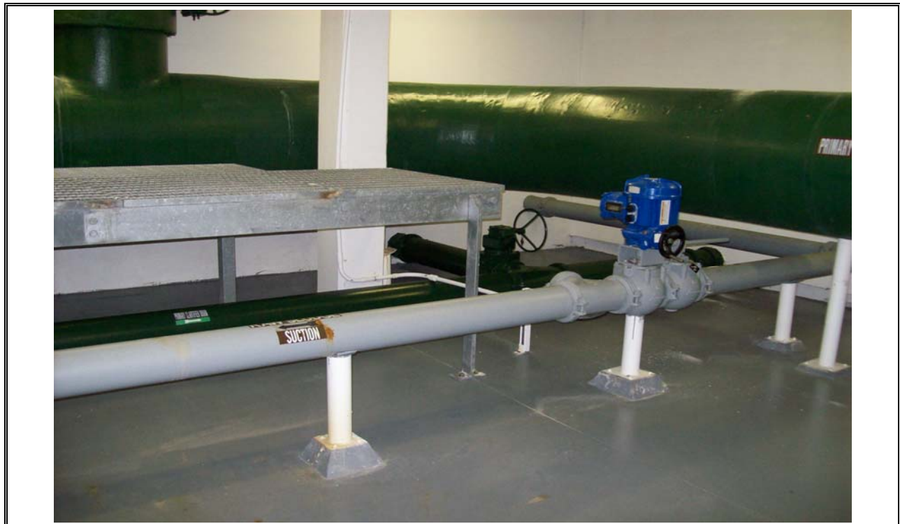
Photo 44 Co-thickened Sludge Line from North Plant Primary
