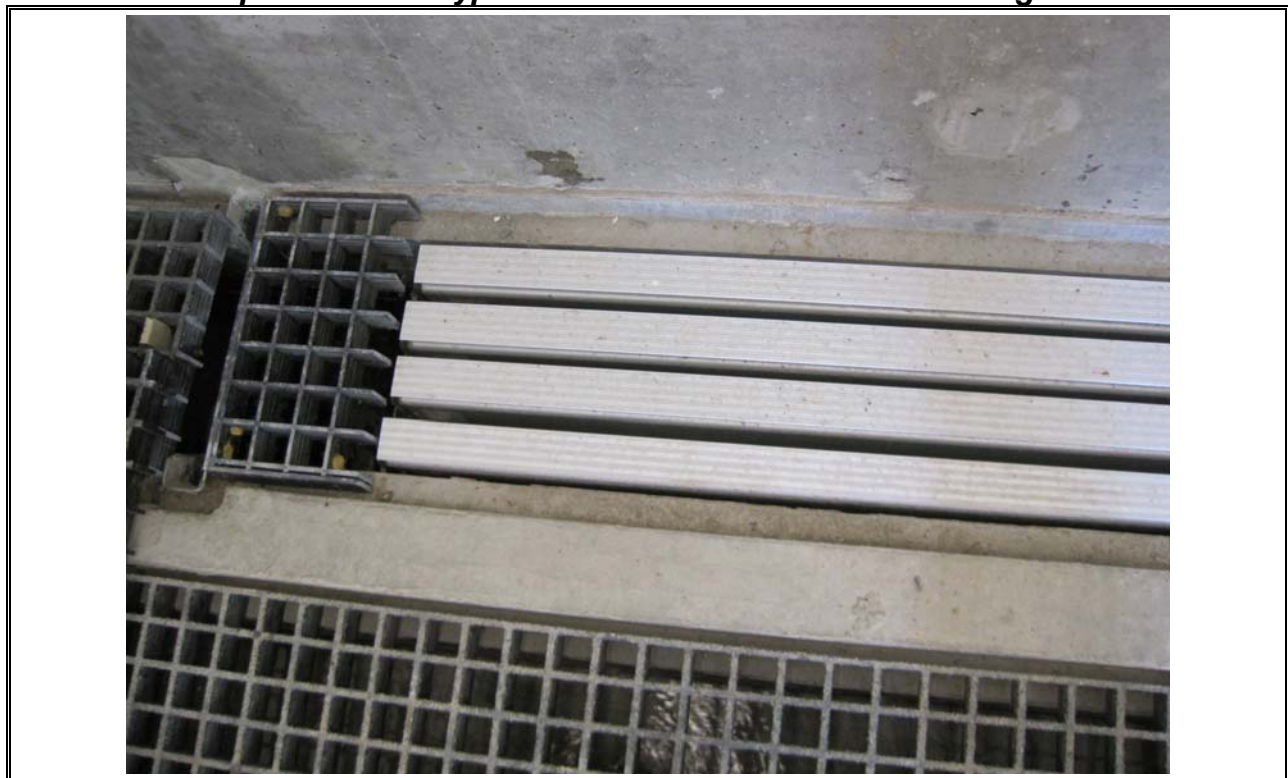
Photo 26 Uplands Park UV Disinfection & Bypass Line
