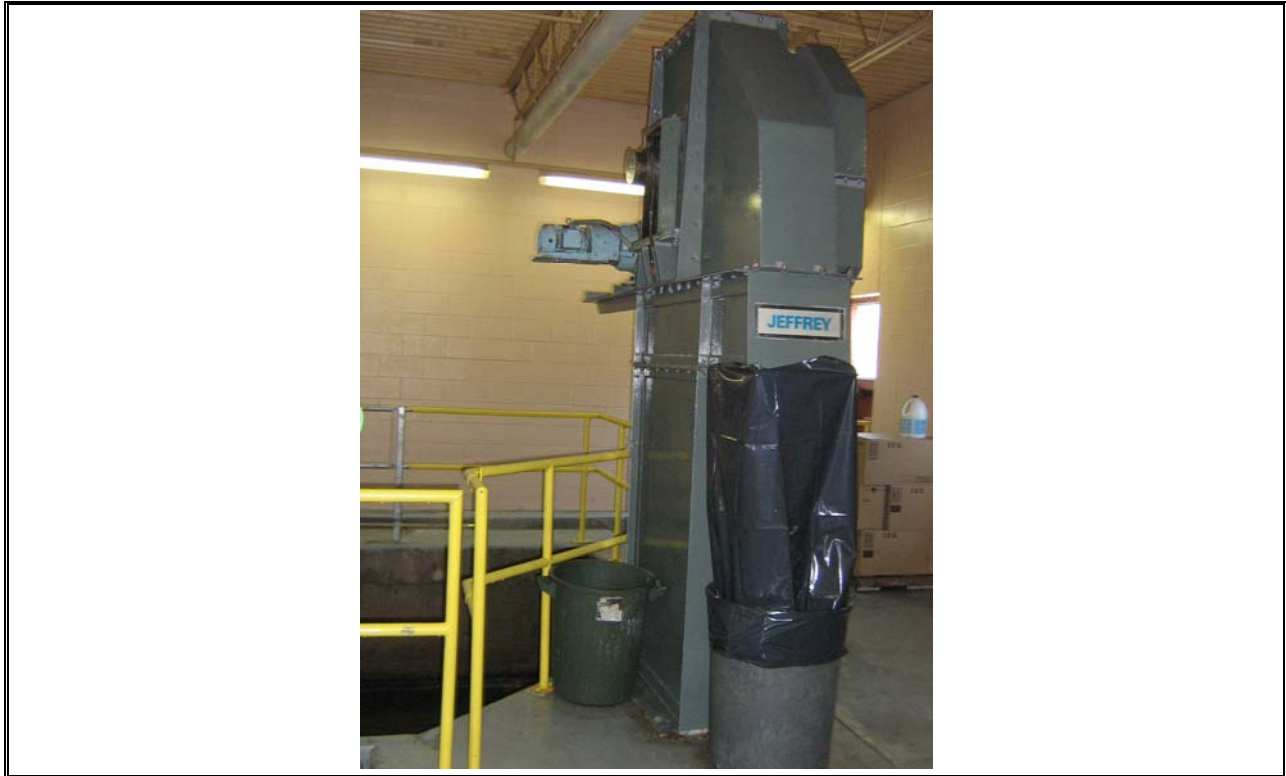
Photo 13 Grit Collected and Removed from Grit Chamber
