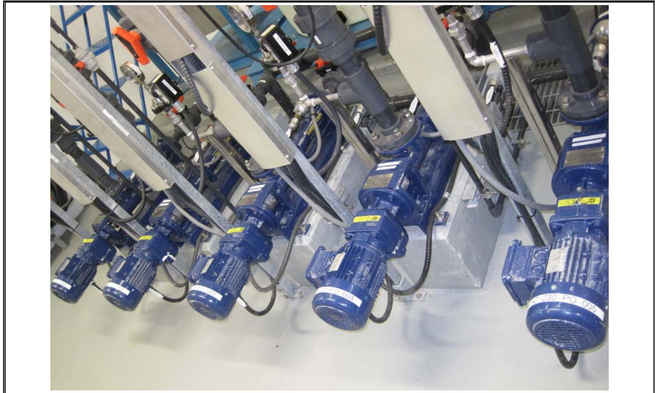
Photo 27 Herring Cove Polymer Pumps for Densadeg
