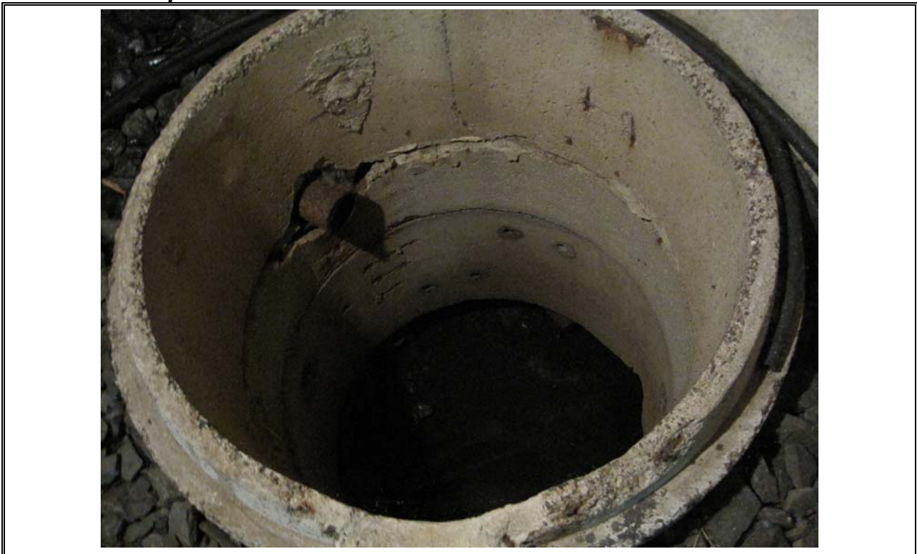
Photo 14 Uplands Park Trickling Filter Subdrain Collection Manhole
