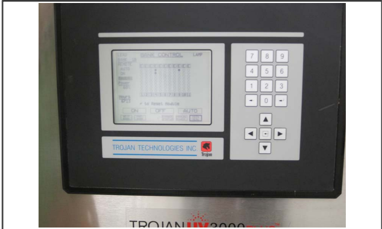
Photo 21 Herring Cove UV Disinfection Control Panel
