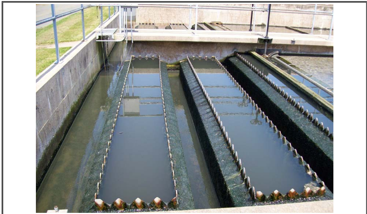
Photo 34 Secondary Clarifier Weirs and Effluent
