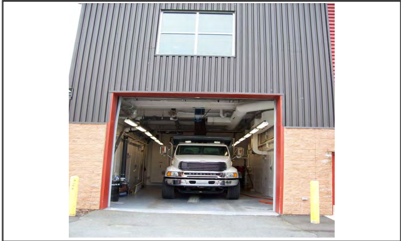
Photo 37 AeroTech Sludge Loading
