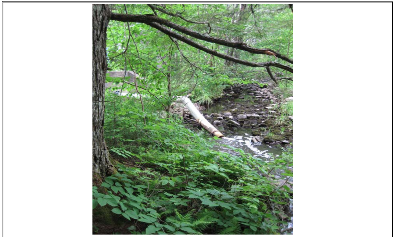
Photo 22 Outfall to Brook to Lisle Lake
