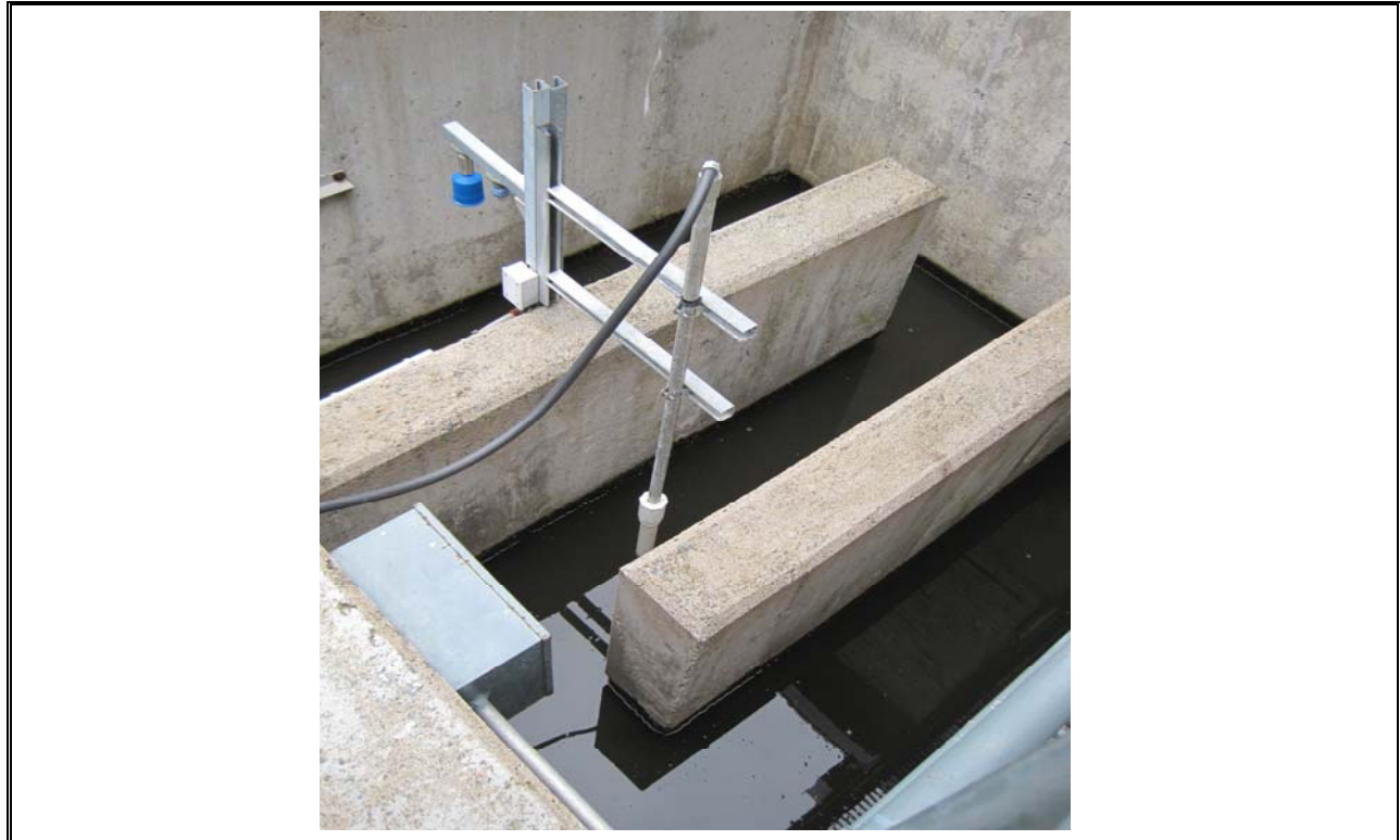
Photo 17 Chlorine Contact Tank
