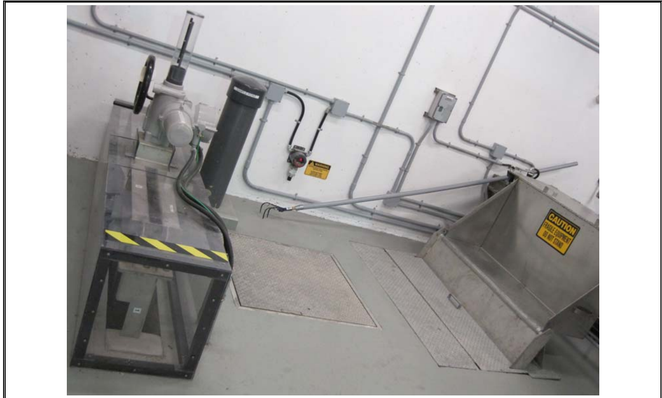
Photo 3 Herring Cove Weir Gate and Manual Coarse Bar Screen
