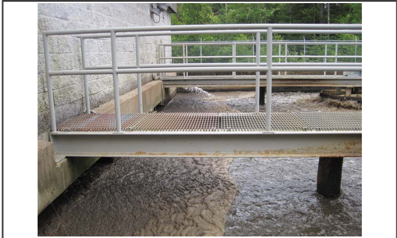
Photo 11 Aeration Tank and Wall of Clarifier Building
