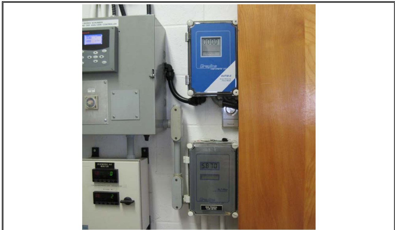
Photo 6 Eastern Passage Flow Meter Display
