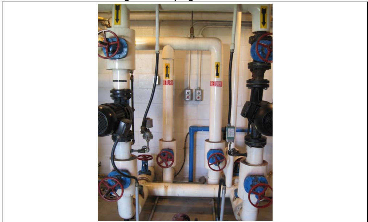
Photo 34 Eastern Passage Piping Returns for Boiler
