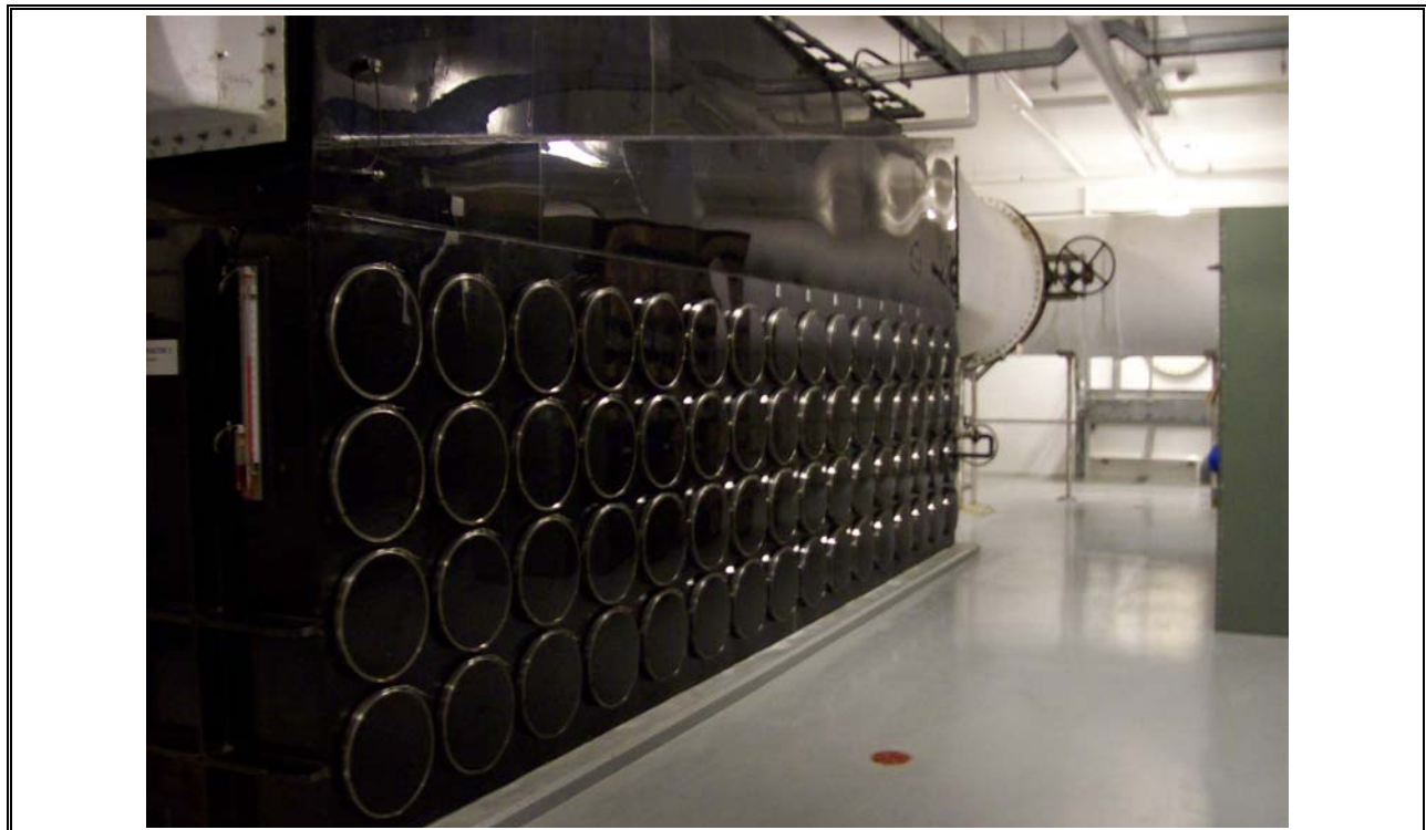
Photo 38 Halifax Odour Control Carbon Scrubber
