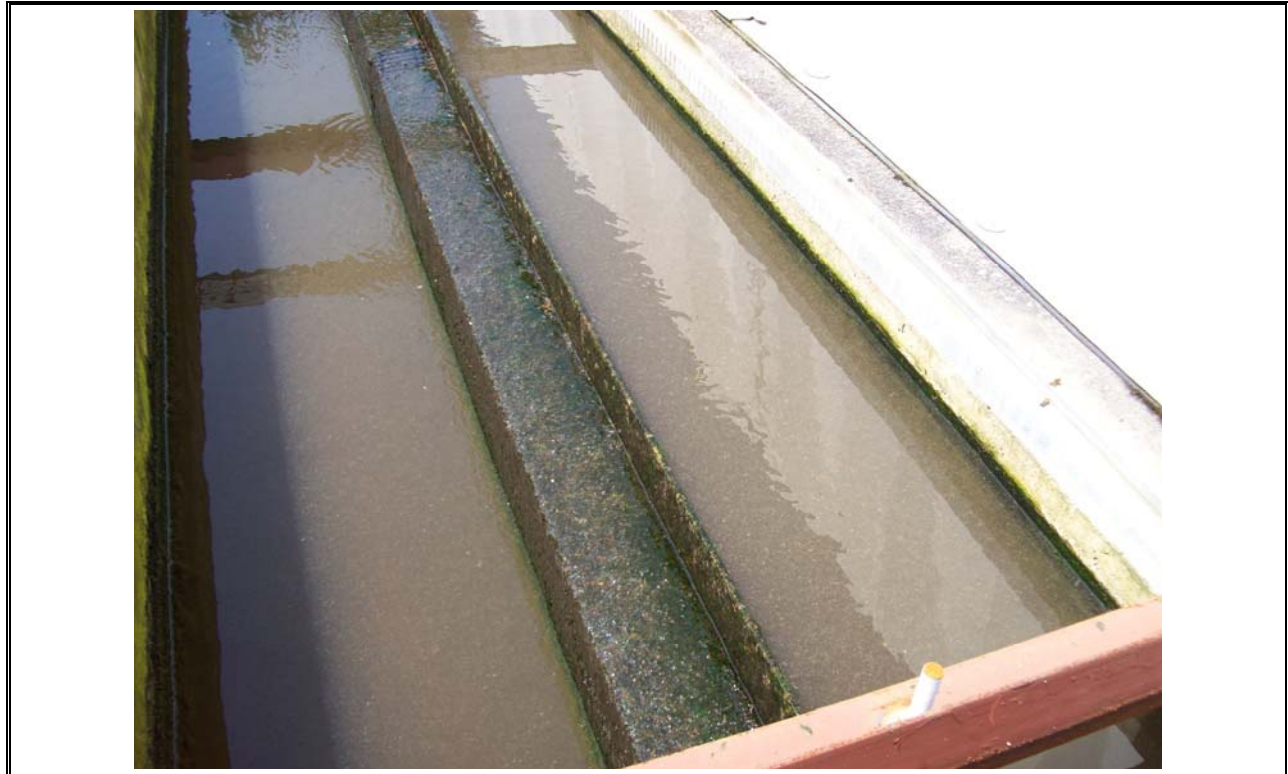
Photo 27 RBC Effluent to Secondary Clarification
