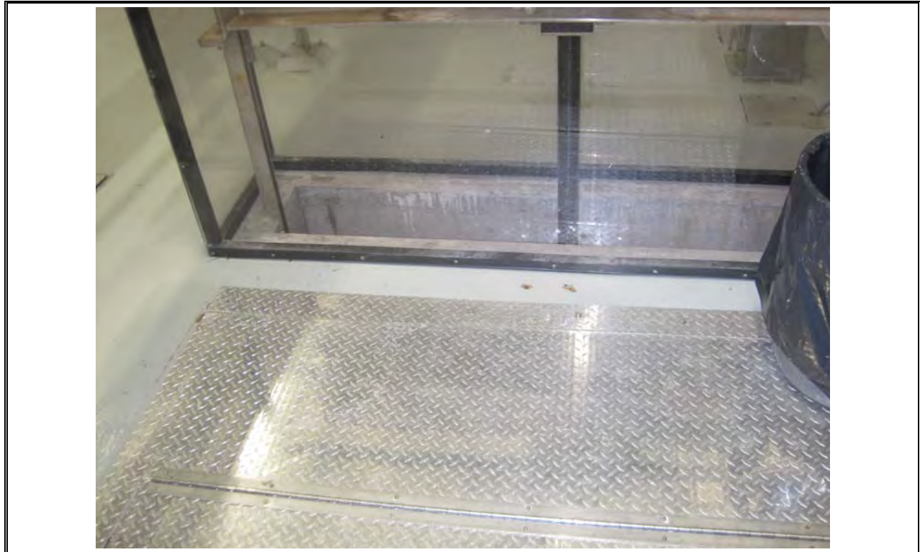
Photo 1 Dartmouth Influent Weir Gate
