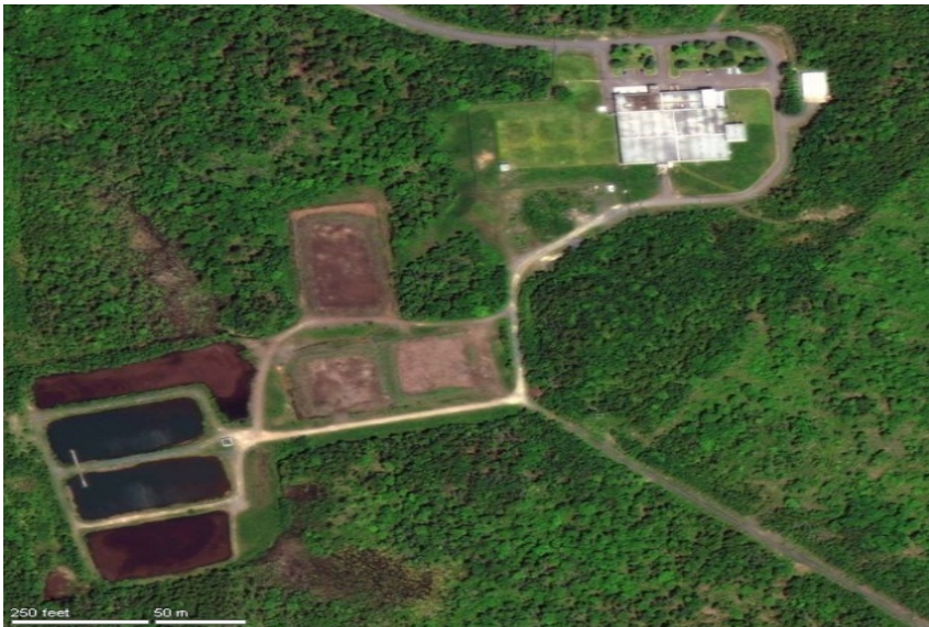
Figure 2. J.D. Kline Water Supply Plant - Aerial View
