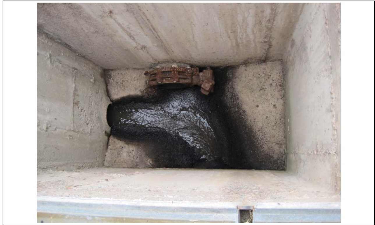
Photo 8 Middle Musquodoboit Bypass from Secondary Tank to UV Disinfection
