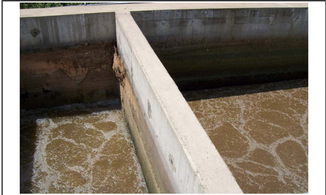
Photo 15 SBR Tanks in React Mode
