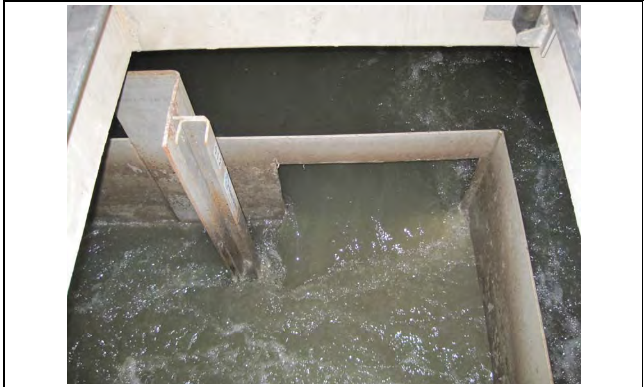
Photo 11 Dartmouth Grit Removal Channel With Hole Cut Into Channel
