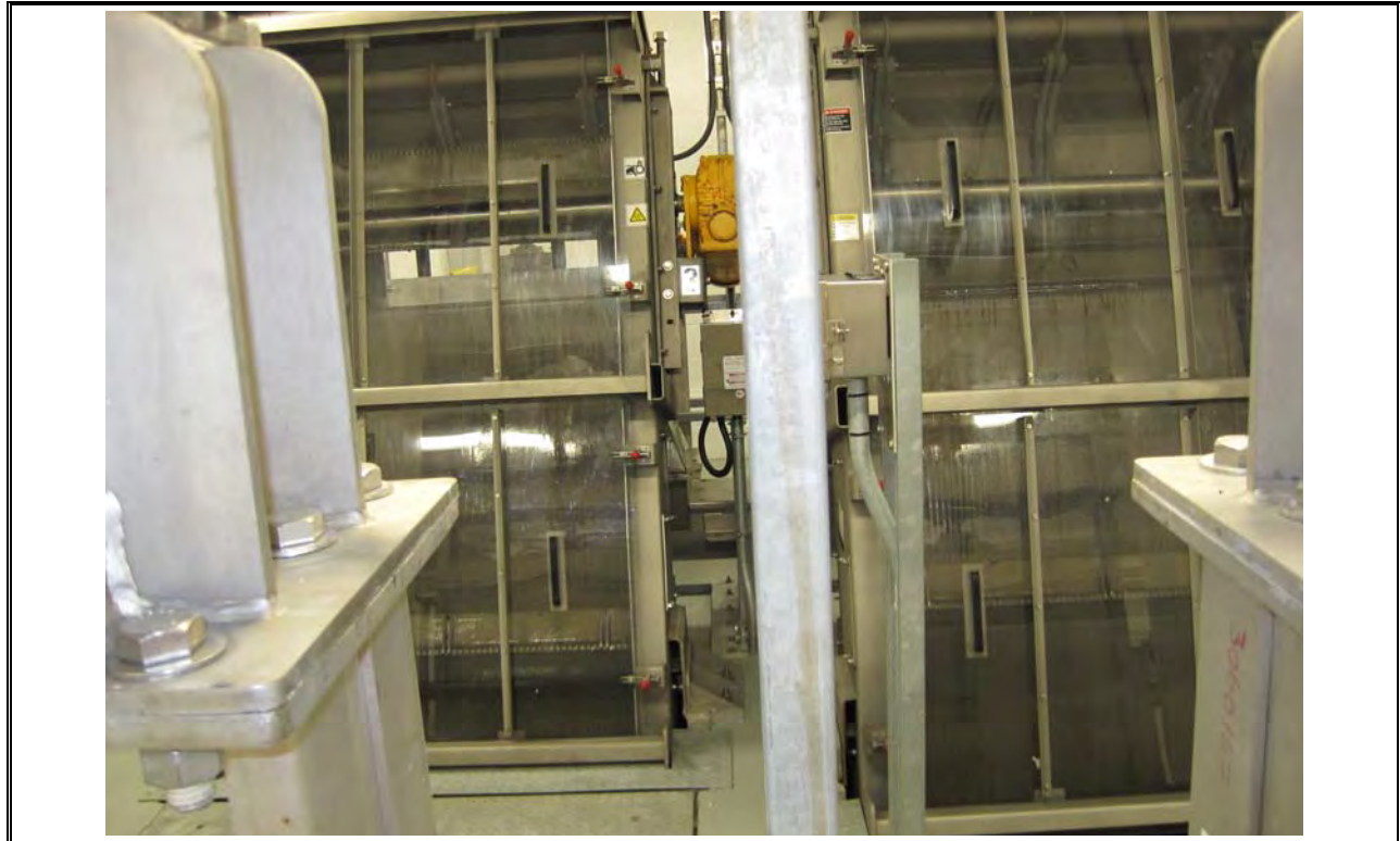
Photo 5 Dartmouth Fine Screens
