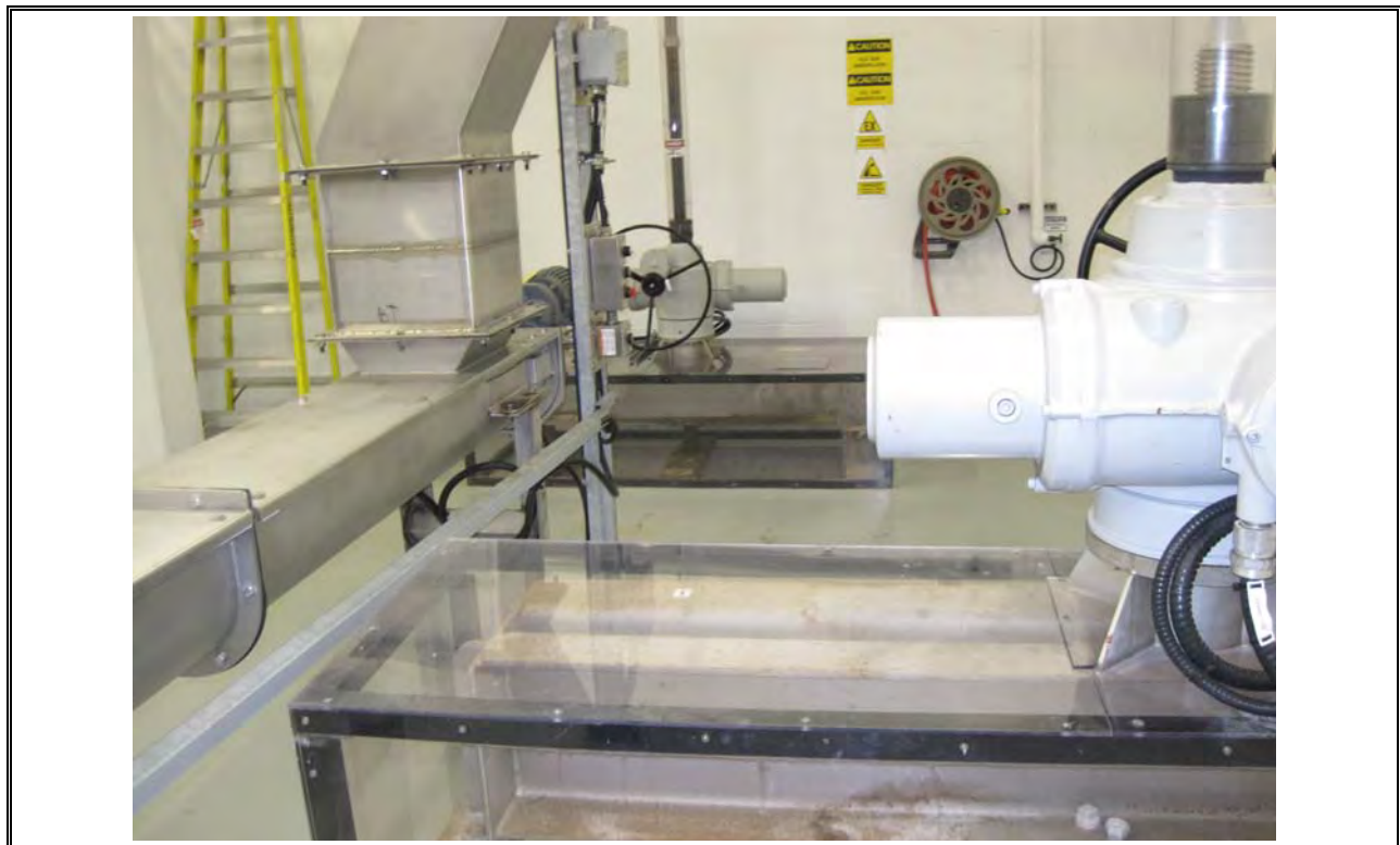
Photo 2 Dartmouth Screenings Conveyor
