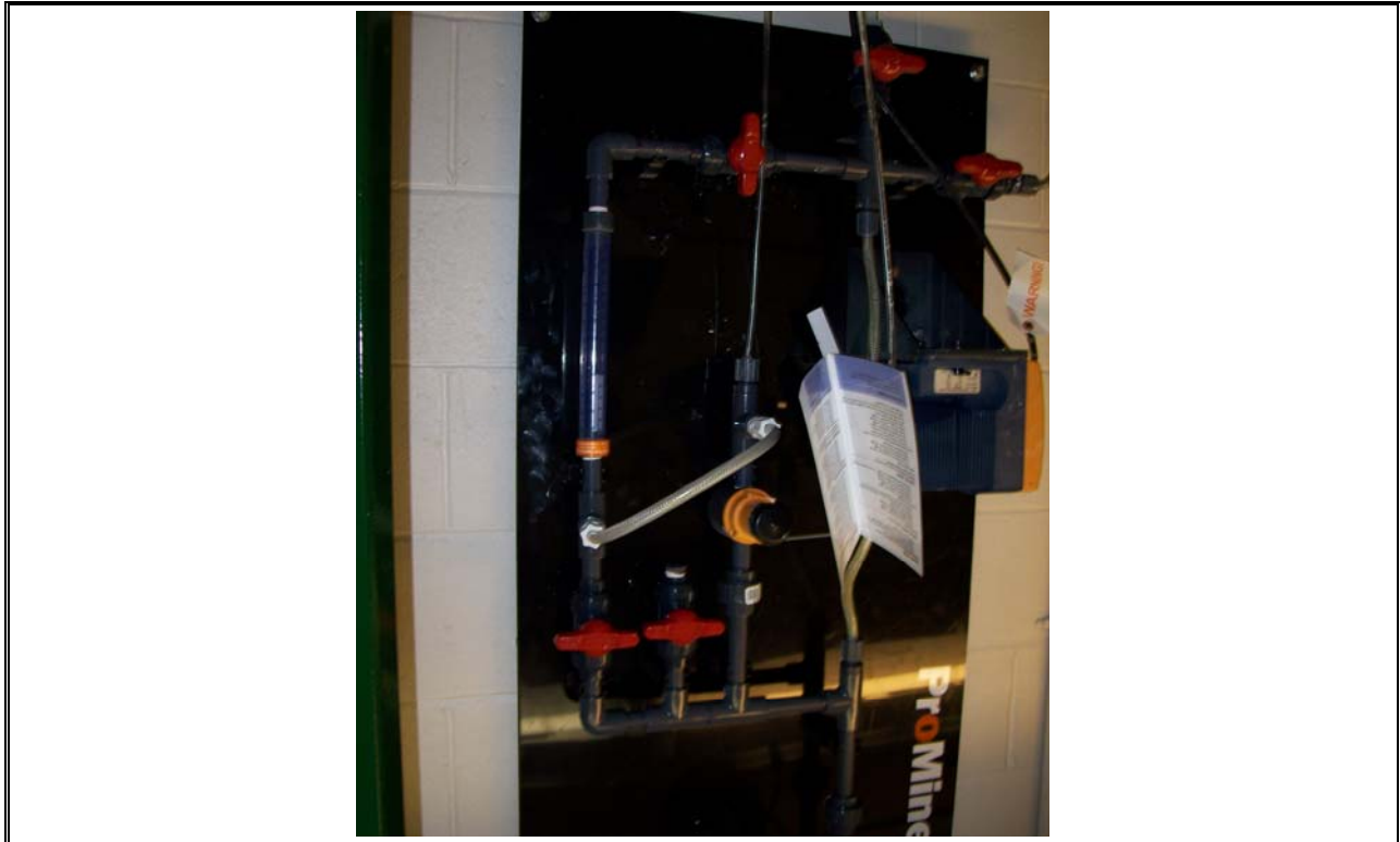
Photo 5 Lockview Caustic Metering Pumps
