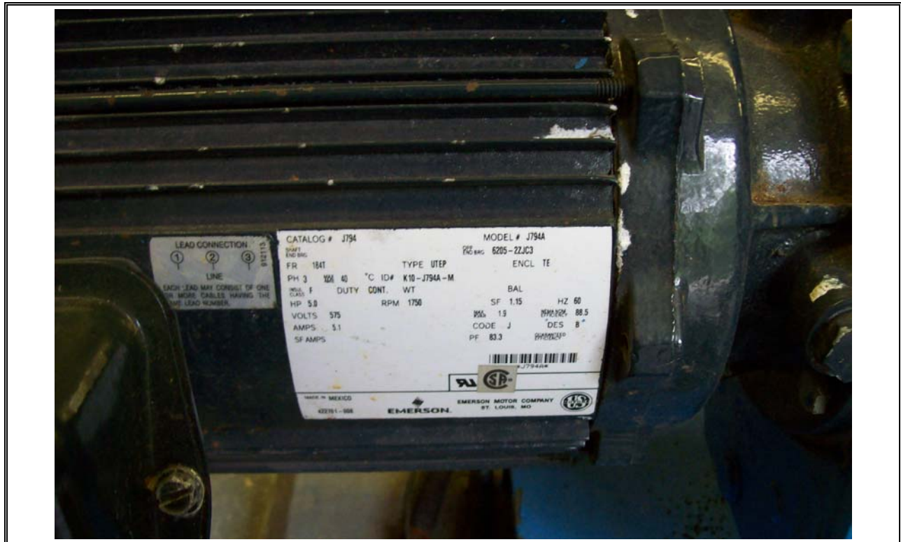
Photo 20 Lockview RAS Pump Motor Nameplate
