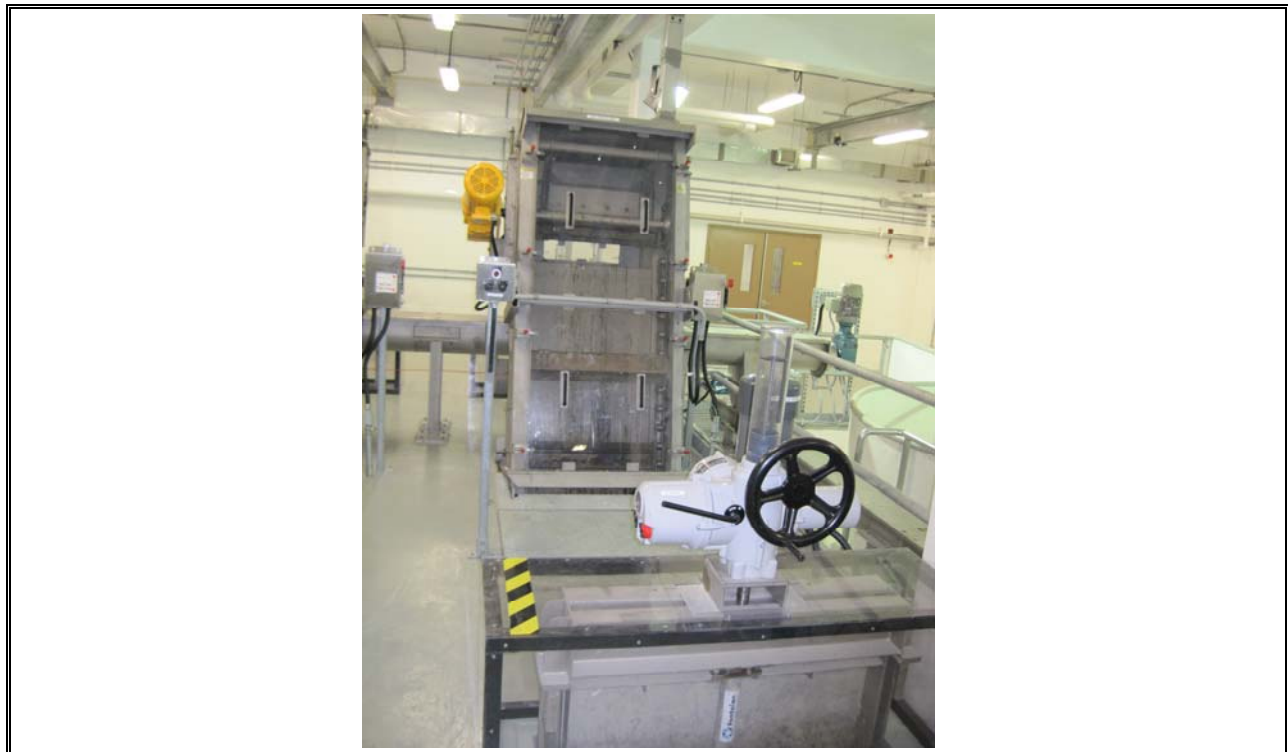
Photo 10 Herring Cove Automatic Fine Bar Screen
