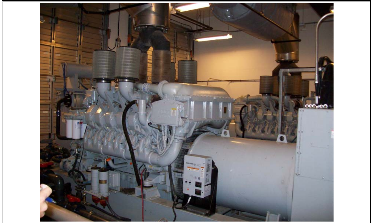
Photo 39 Halifax Generator for Back-Up Power
