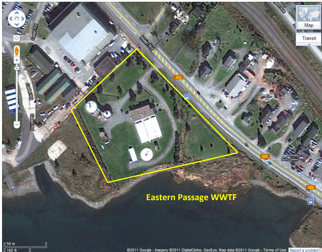
Figure 2.1 Eastern Passage WWTF - Aerial View
