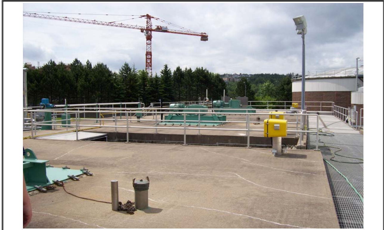
Photo 21 PureOx™ Bioreactors with Mixers
