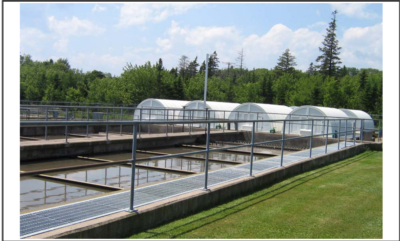
Photo 15 P Primary Clarification with Chain and Flight Mechanism
