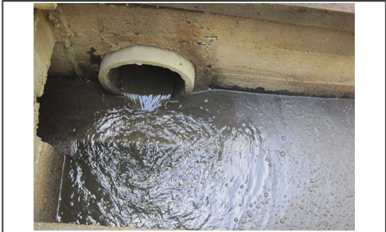
Photo 17 Uplands Park Secondary Clarifier Influent
