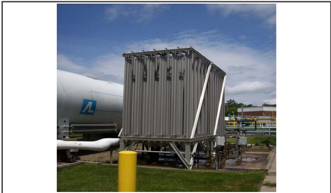
Photo 24 Oxygen Storage System
