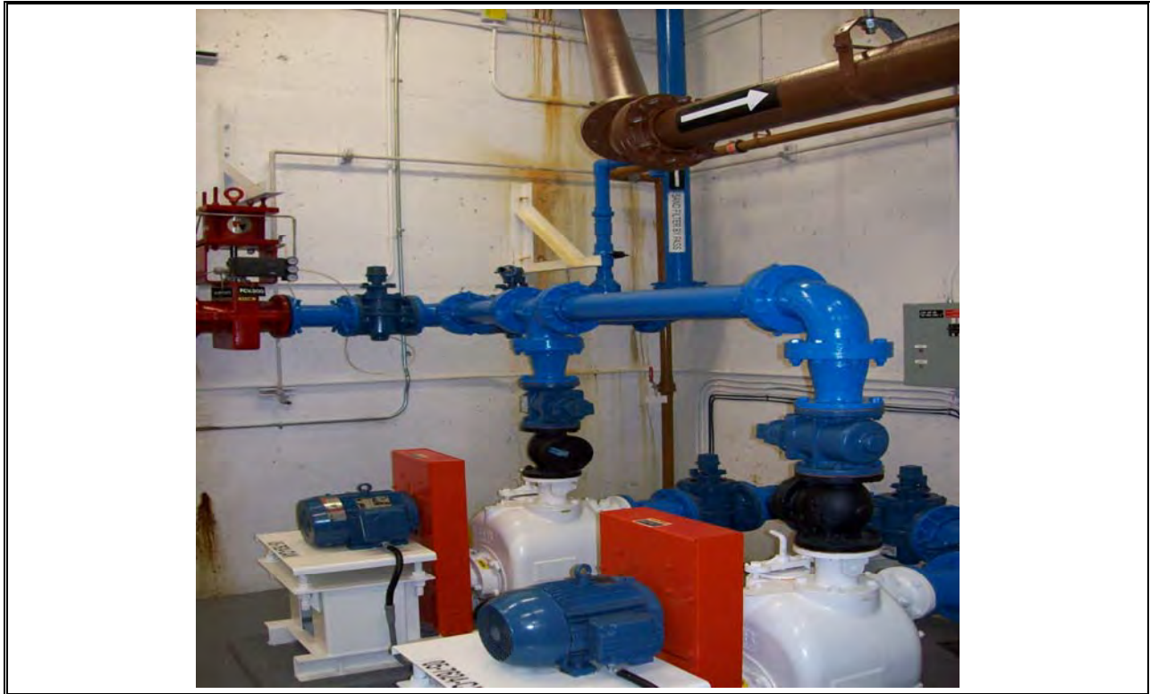
Photo 27 AeroTech Filter Feed Pumps
