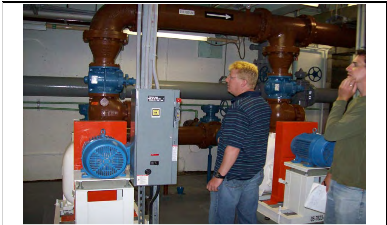
Photo 22 AeroTech SBR Feed Pumps
