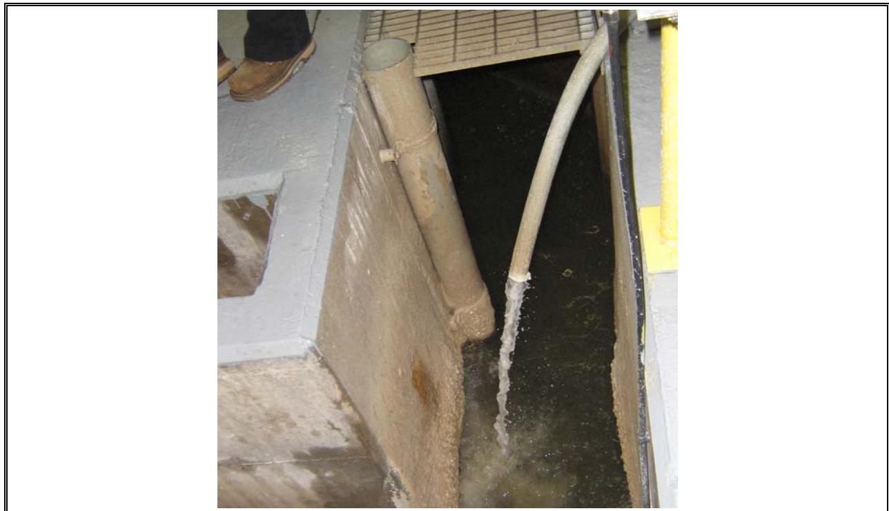
Photo 10 Lime addition and Supernatant Return Following Parshall Flume
