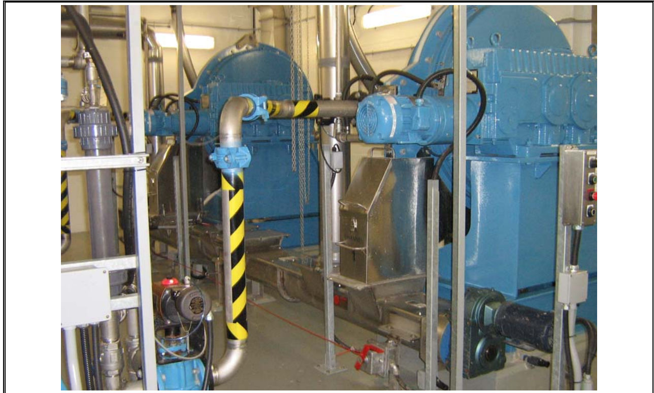
Photo 41 Herring Cove Fournier Rotary Presses
