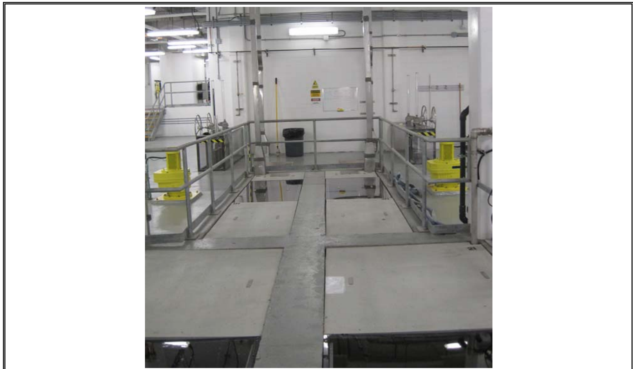
Photo 14 Herring Cove Densadeg Enhanced Primary Treatment
