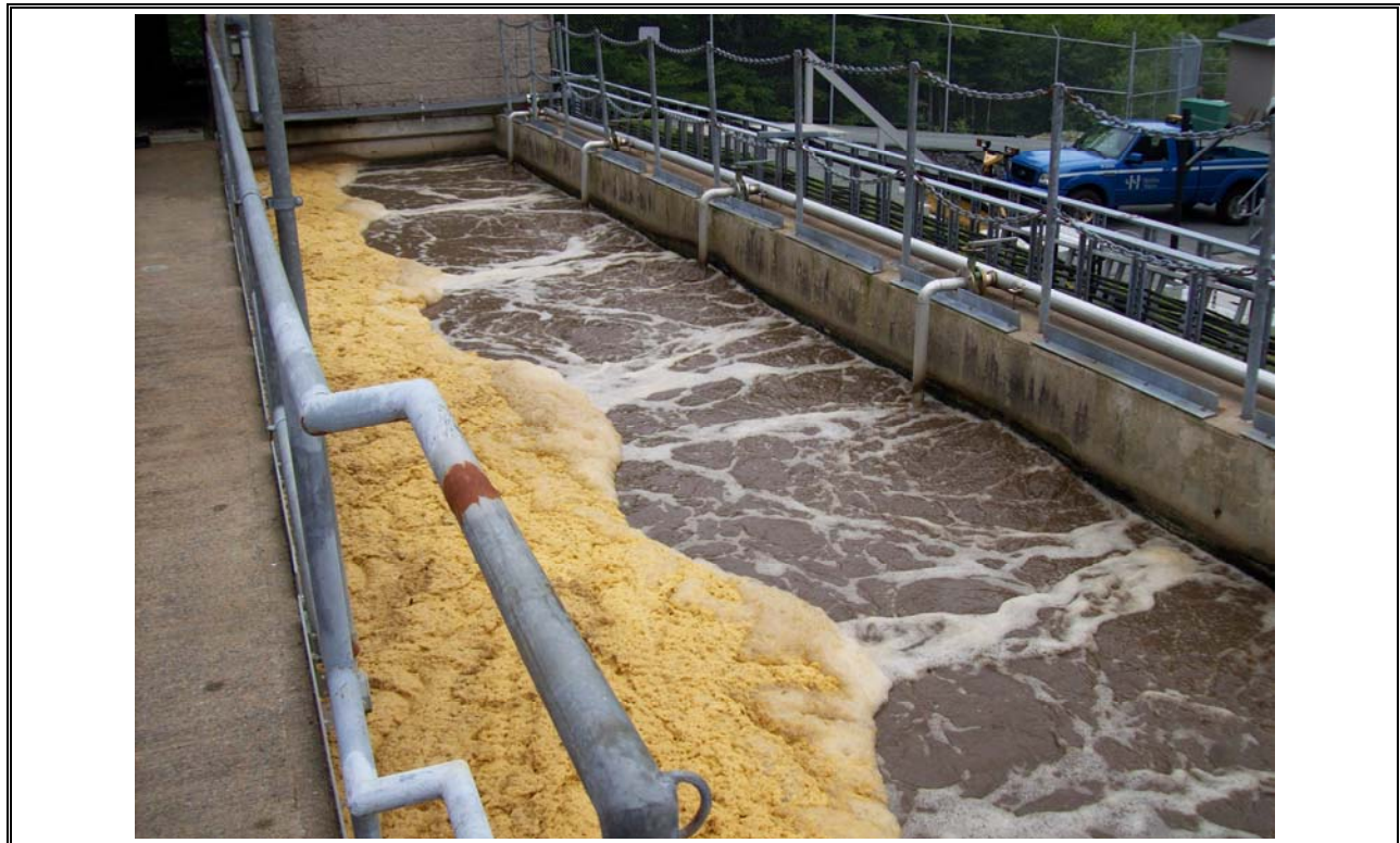
Photo 8 Lockview Aeration Tank
