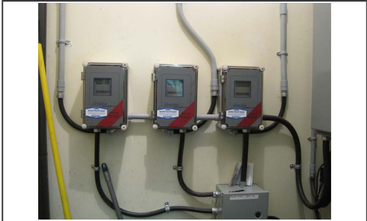
Photo 23 Flow Meters for Three Influent Forcemains
