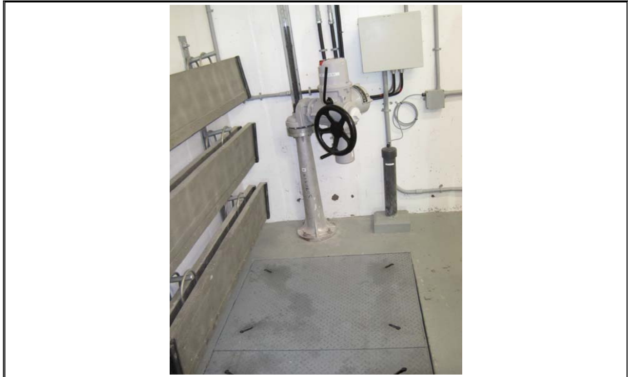
Photo 1 Herring Cove Inlet Chamber and Shut Off Valve
