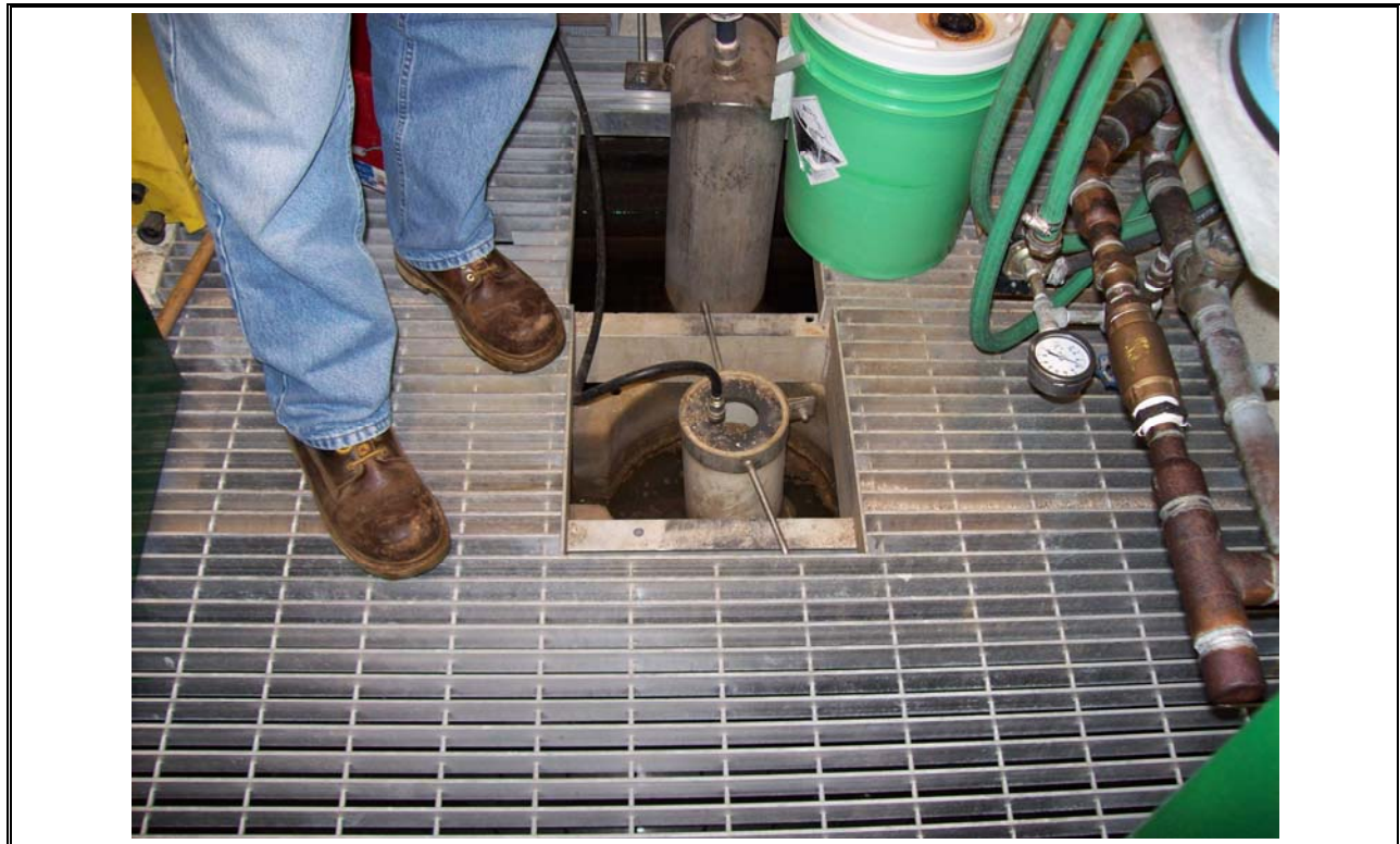
Photo 23 Lockview Tertiary Filter Below Grating
