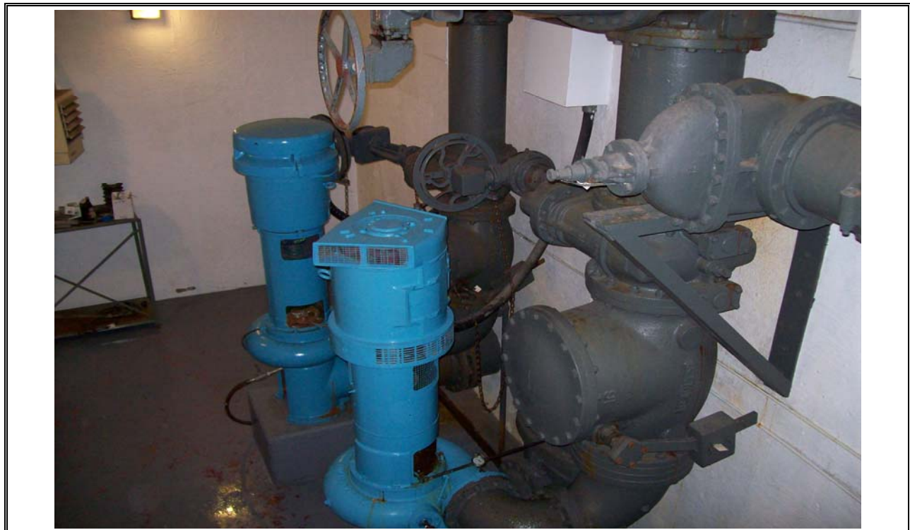
Photo 2 Raw Wastewater Pumps
