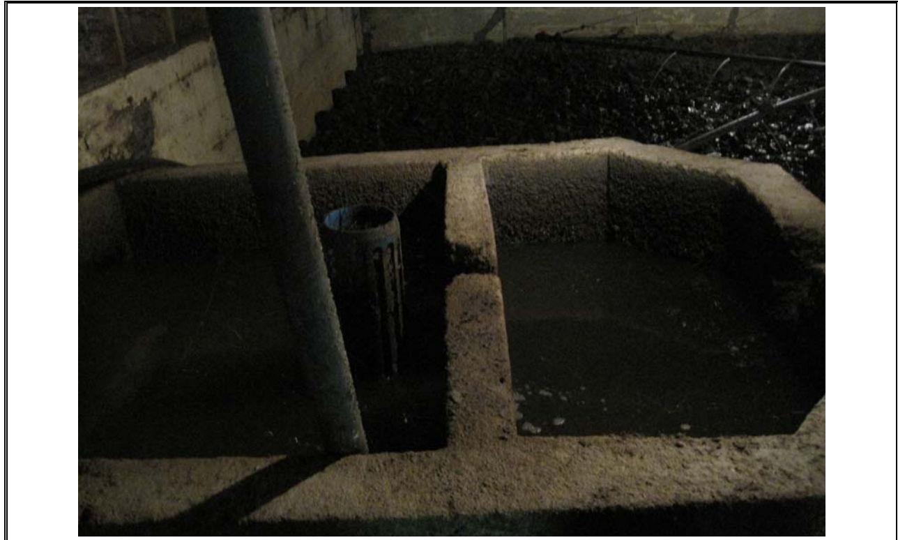
Photo 11 Uplands Park Cylindrical Screen & Secondary Clarifier Return
