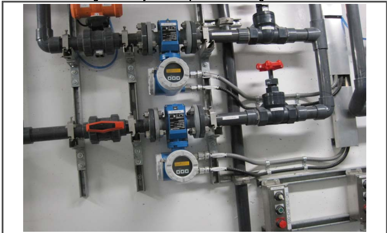
Photo 28 Herring Cove Polymer Pump Metering System
