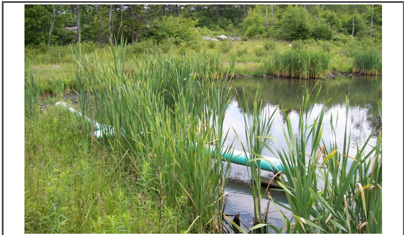
Photo 18 Engineered Wetland Cell No. 1 - Inlet
