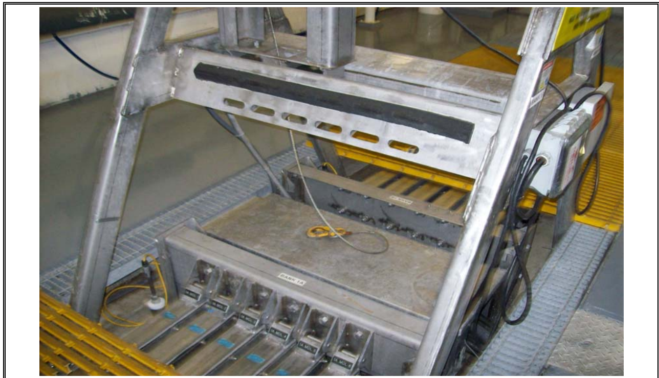
Photo 40 UV Disinfection System – UV Bulbs
