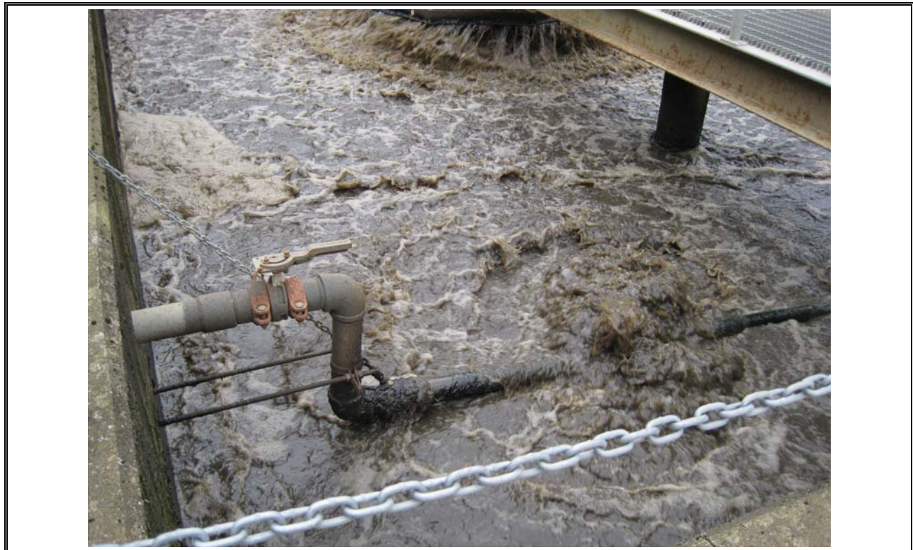
Photo 8 BioLac Aeration Aystem Piping
