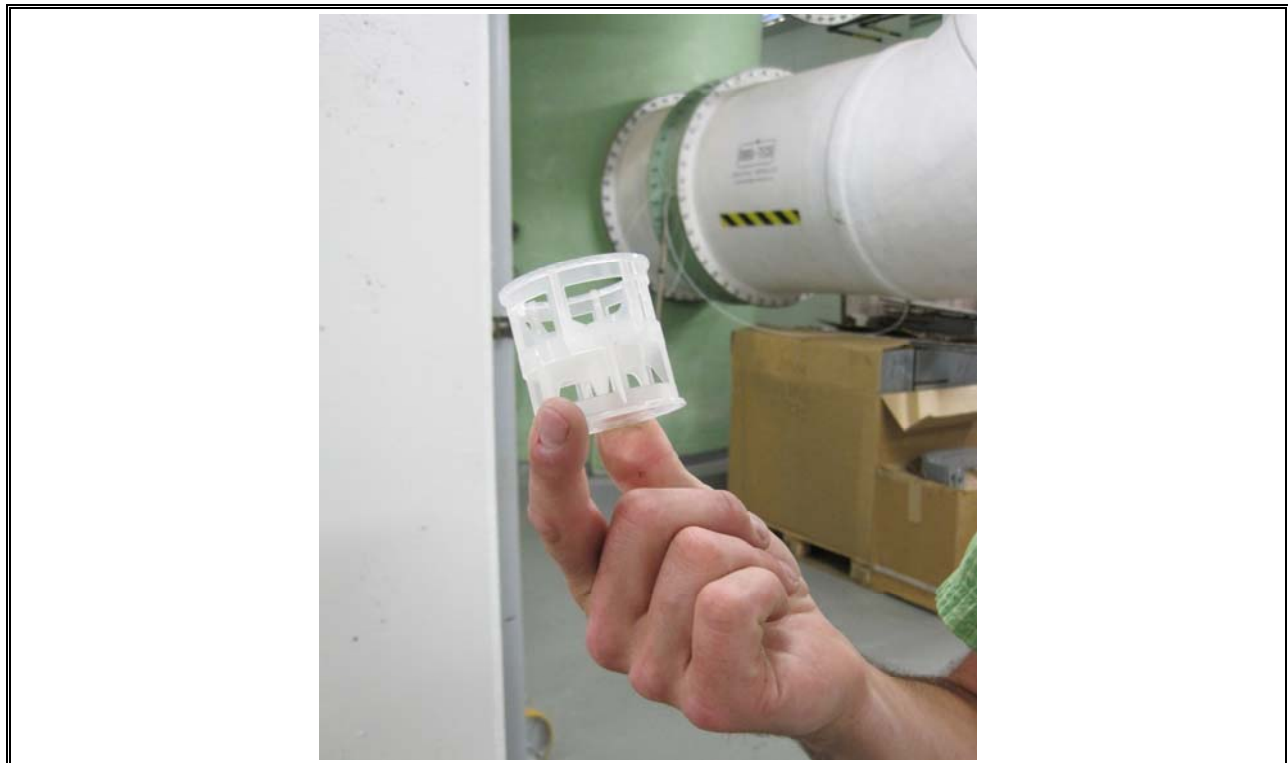
Photo 48 Herring Cove Odour Control Wet Scrubber Media
