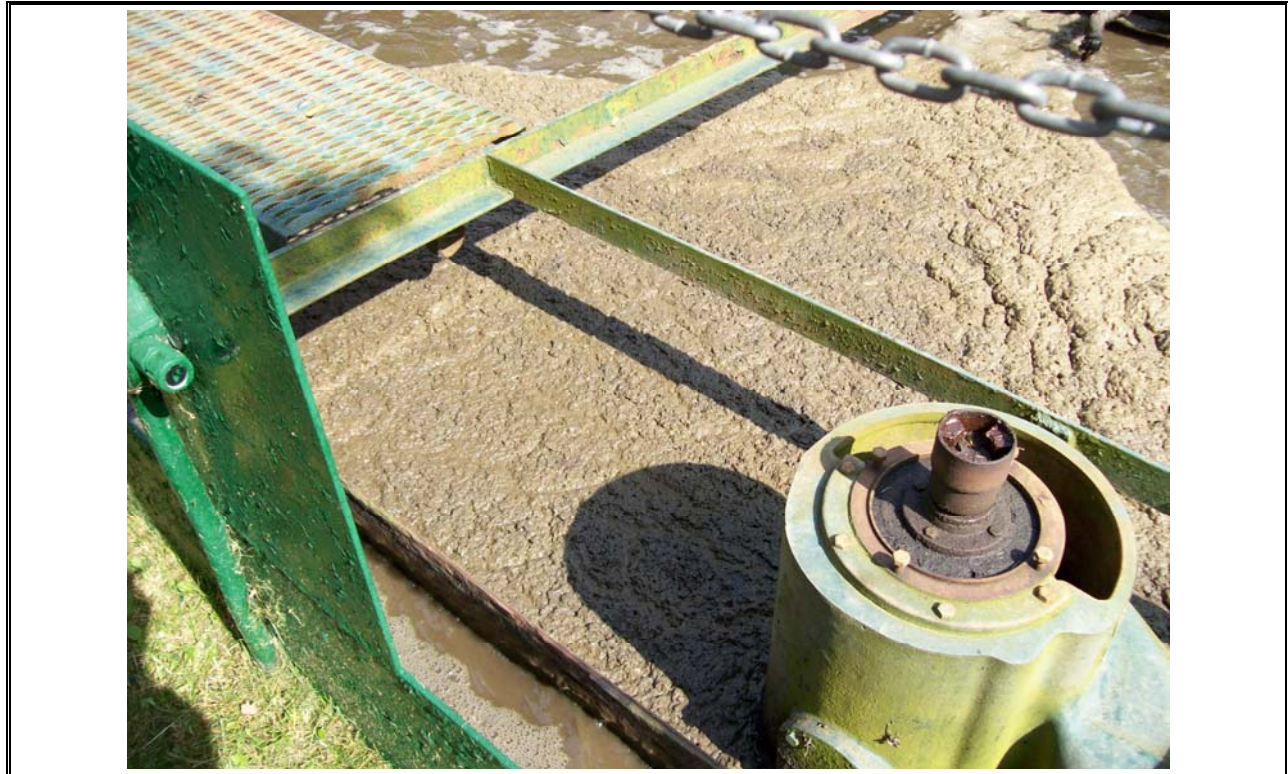
Photo 7 Wellington Foam on Bioreactor
