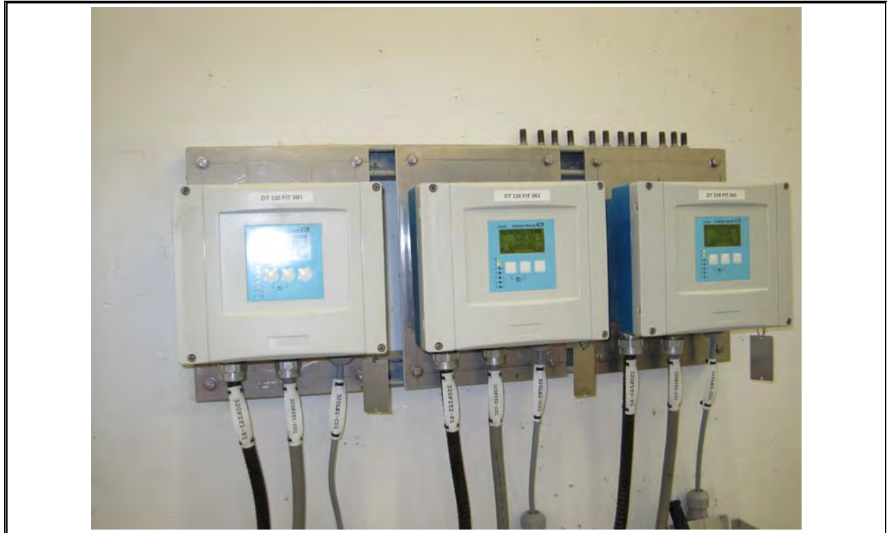
Photo 27 Dartmouth Flow Metering of Effluent
