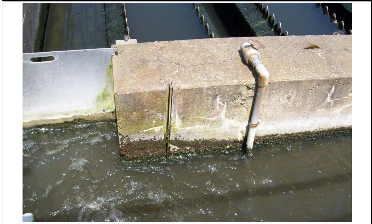
Photo 31 Bypass Slide Gate Around Secondary Clarification
