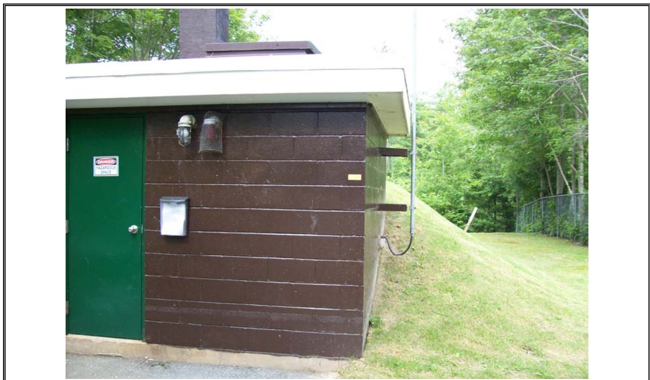
Photo 16 Wellington Blower Building
