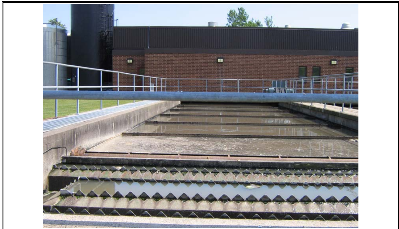
Photo 16 Primary Clarifier Effluent Weirs
