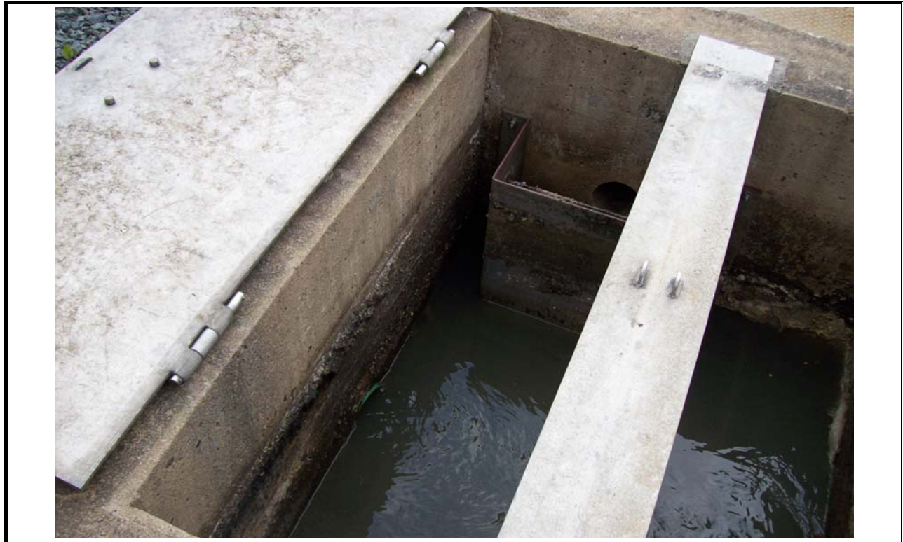
Photo 5 Grit Tank Overflow Weir
