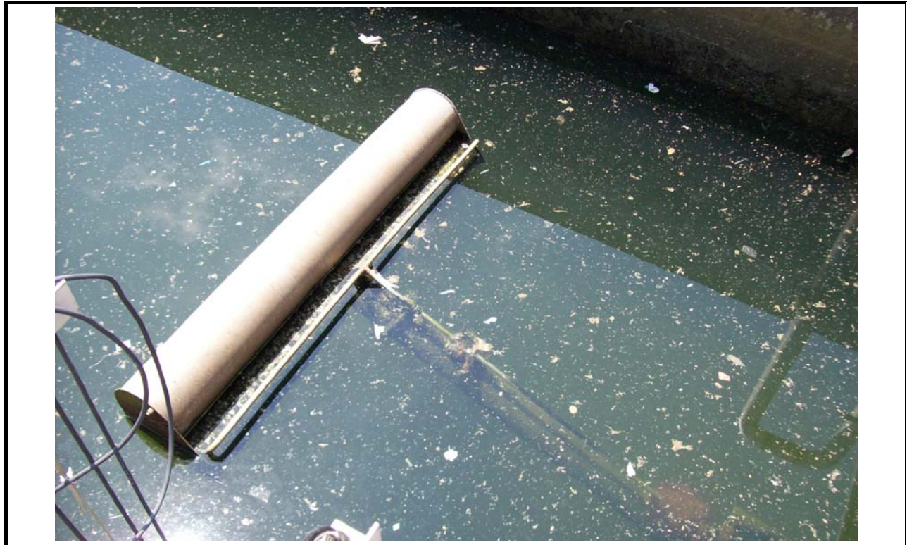
Photo 13 SBR Decant Mechanism (typ)
