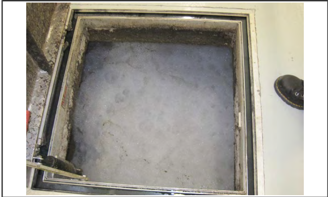
Photo 19 Dartmouth Densadeg Foam in Effluent Channel
