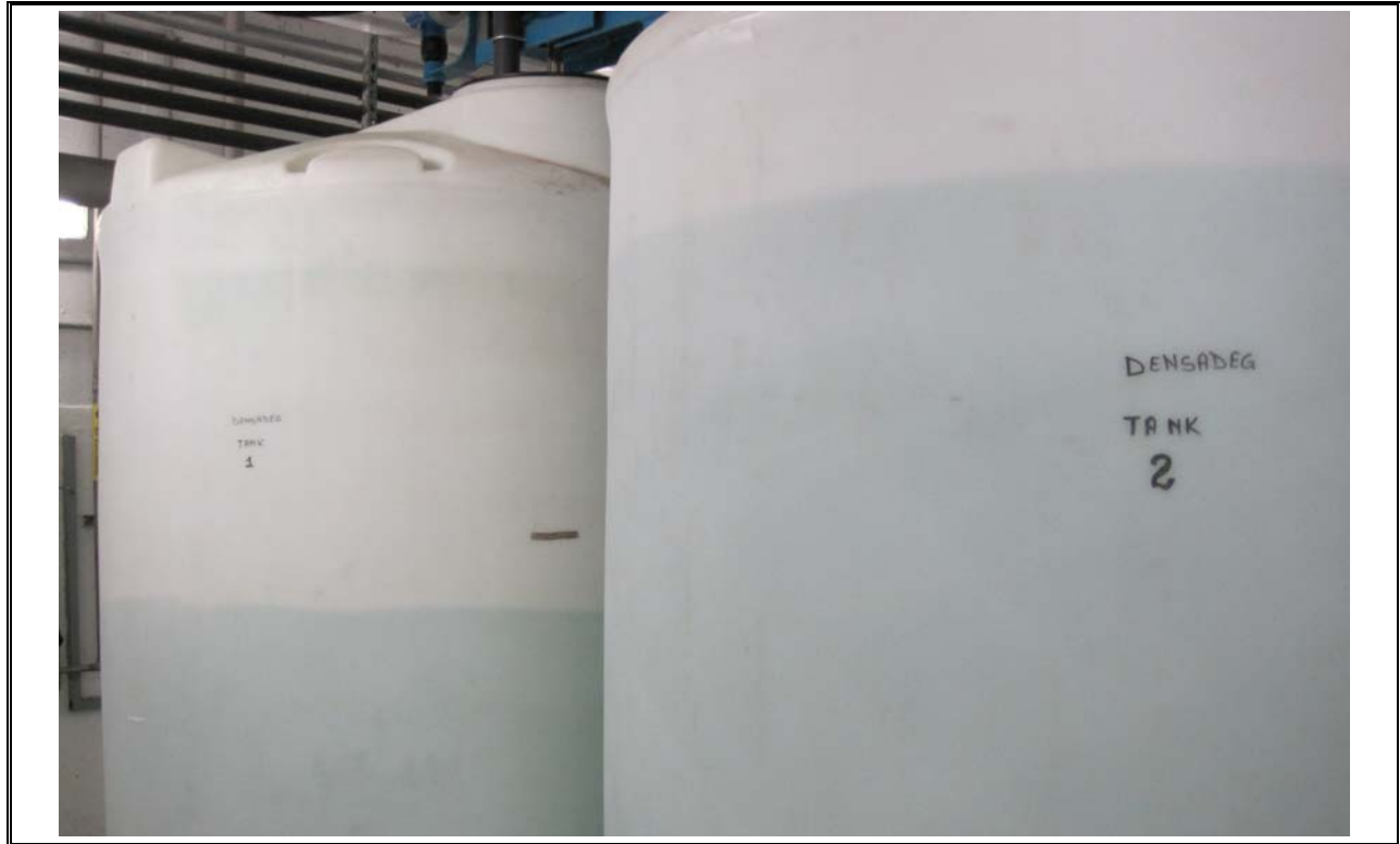
Photo 29 Herring Cove Polymer Storage Containers for Densadeg Polymer
