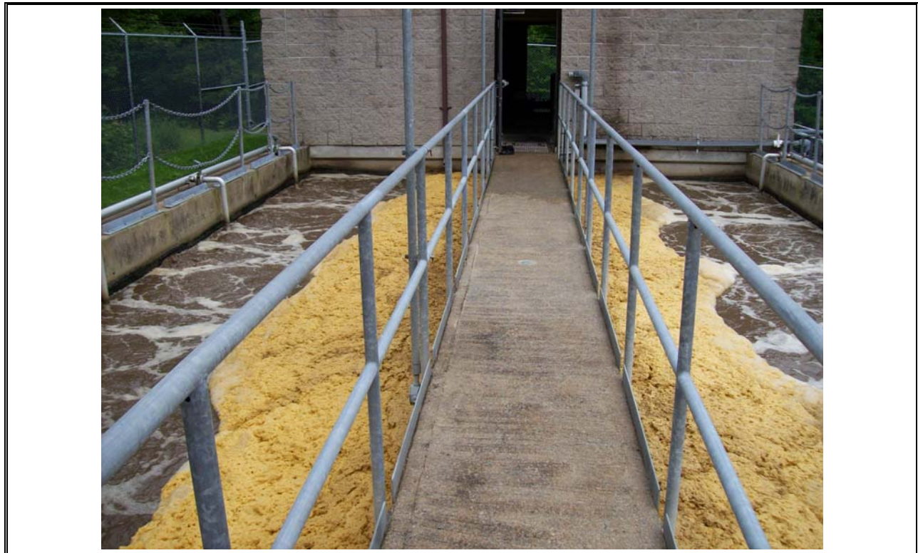
Photo 7 Lockview Aeration Tanks
