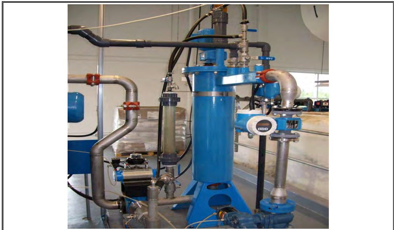
Photo 34 AeroTech Sludge Floc Tank
