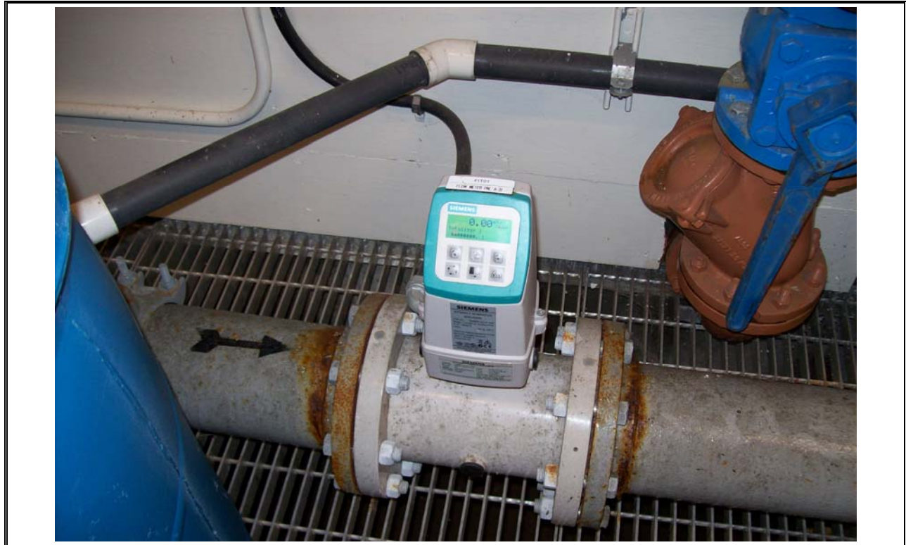
Photo 9 SBR Influent Flowmeter
