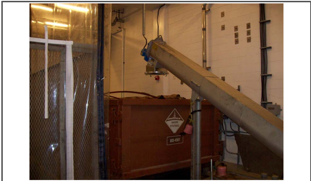
Photo 14 Halifax Grit Bin
