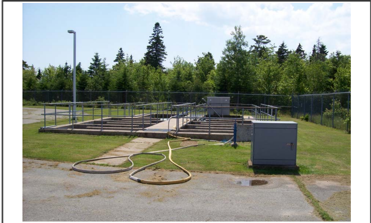
Photo 35 Chlorination/Post Aeration Tanks
