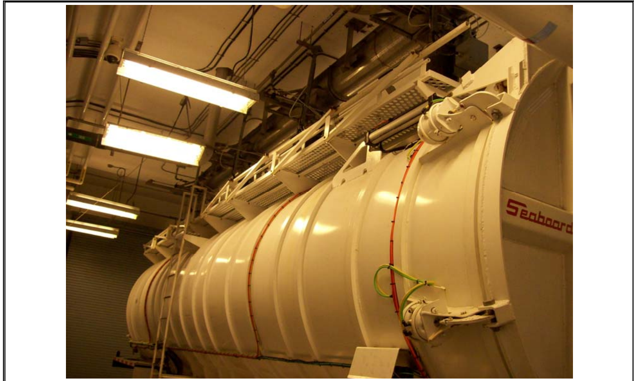
Photo 35 Halifax Sludge Cake Loading Bay and Truck
