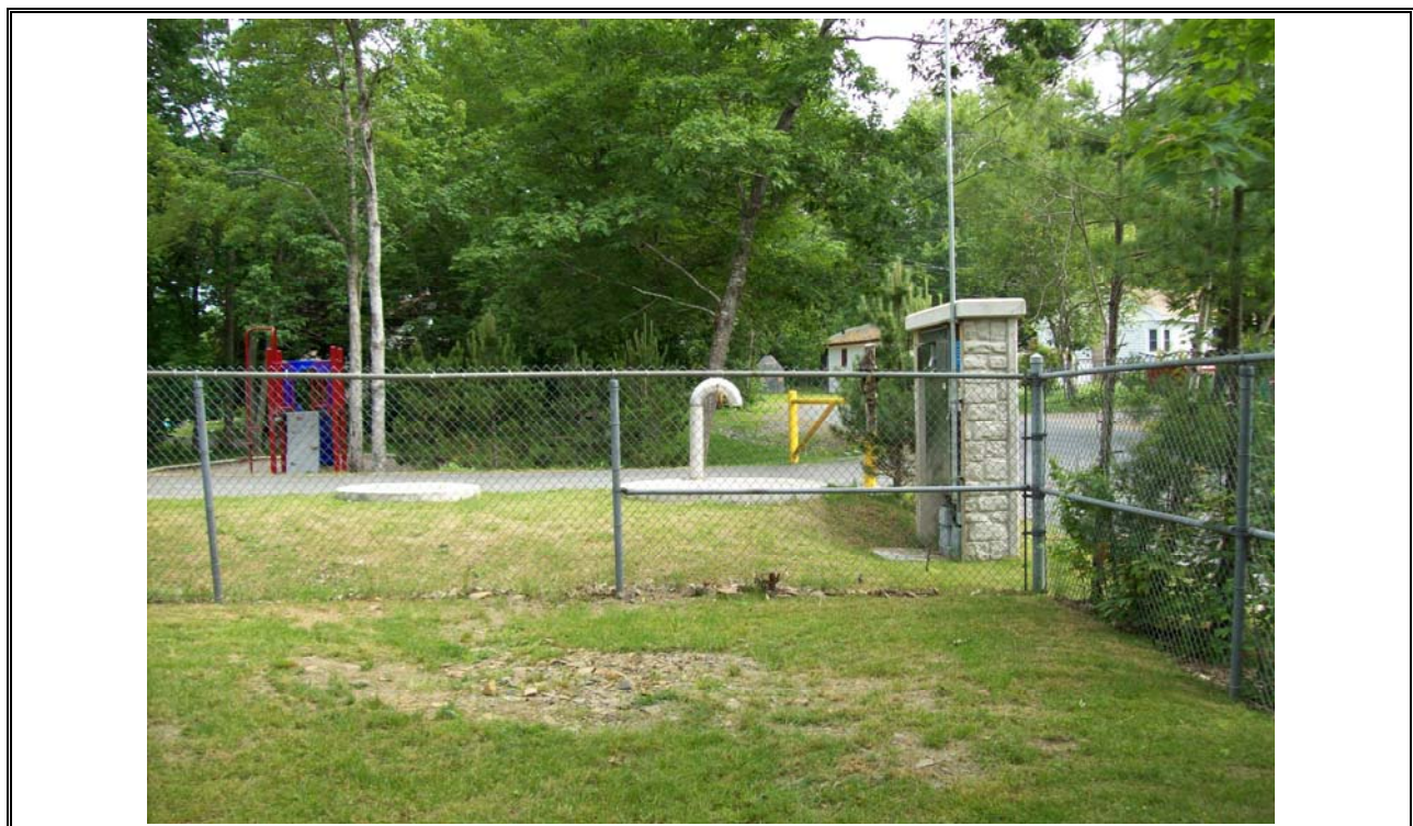
Photo 2 Wellington Influent Pumping Station & Site for New Facility
