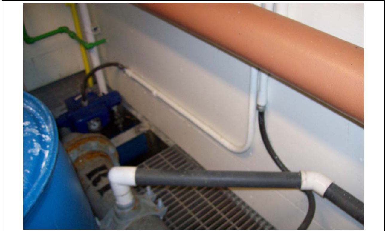
Photo 11 Lime Injection Point
