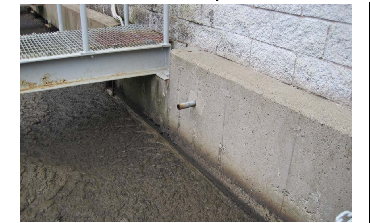
Photo 10 Supernatant Return Line from Waste Tank to Aeration Tank
