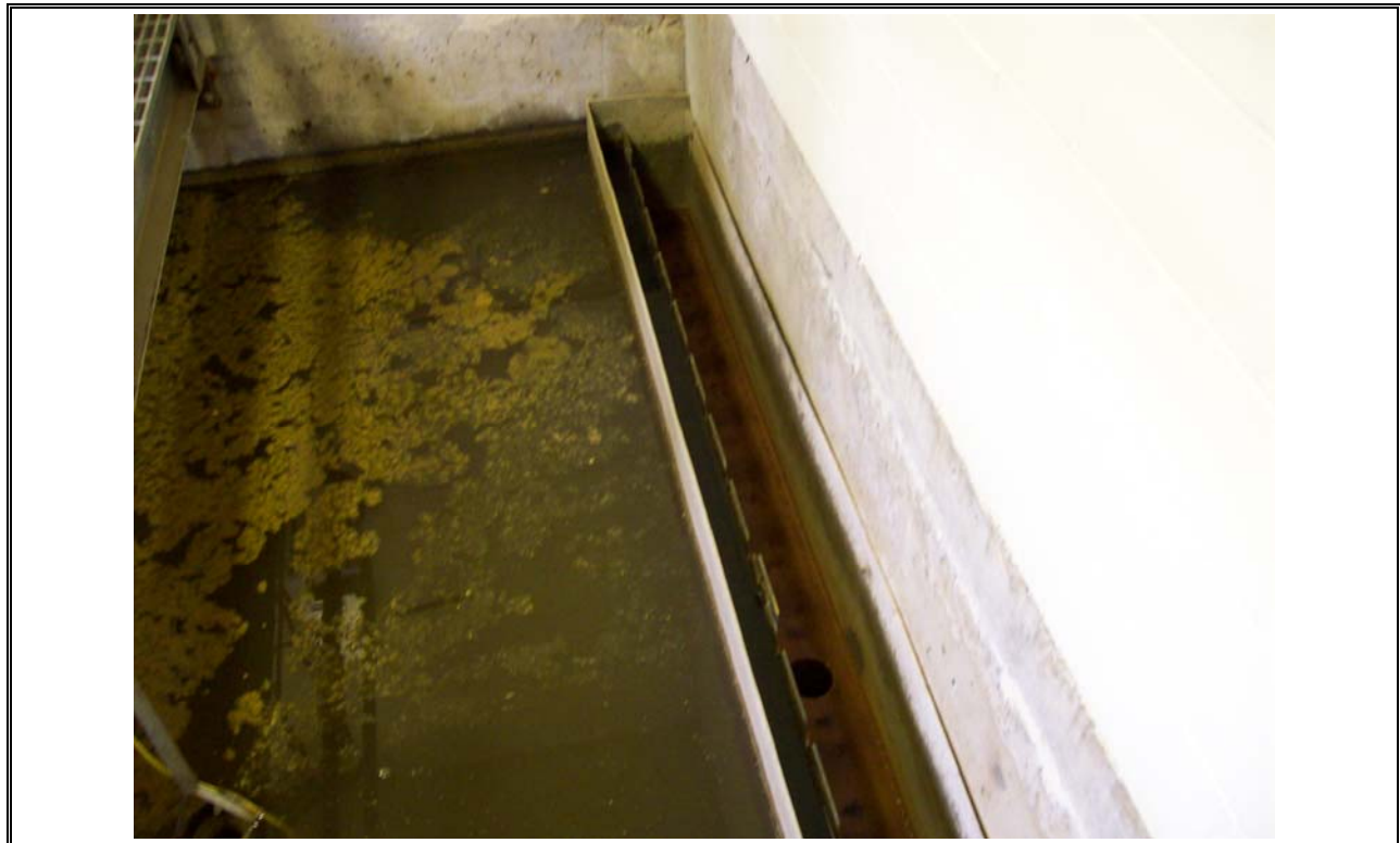
Photo 16 Lockview Clarifier Effluent Weir
