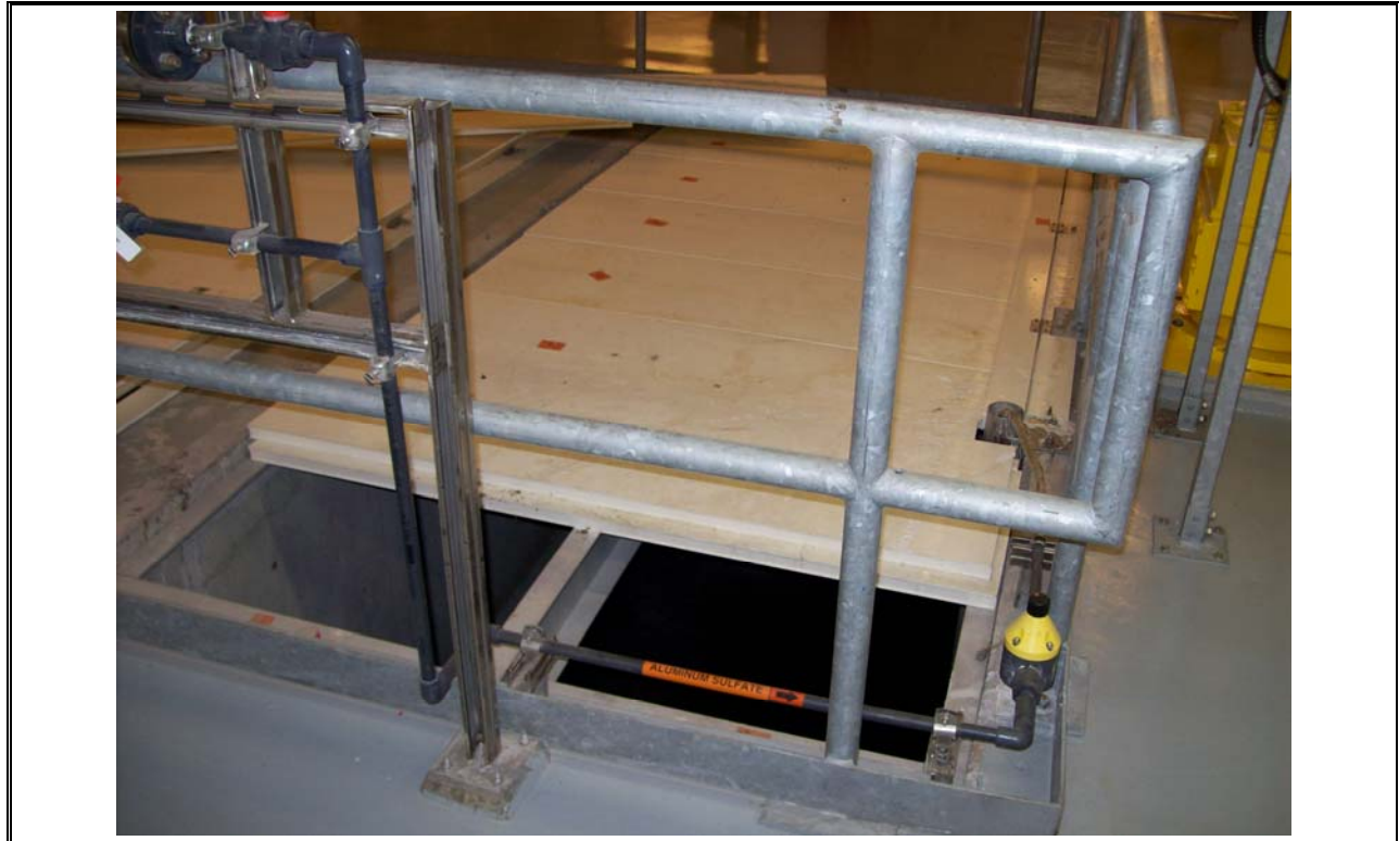
Photo 17 Halifax Densadeg Alum Dosing Line
