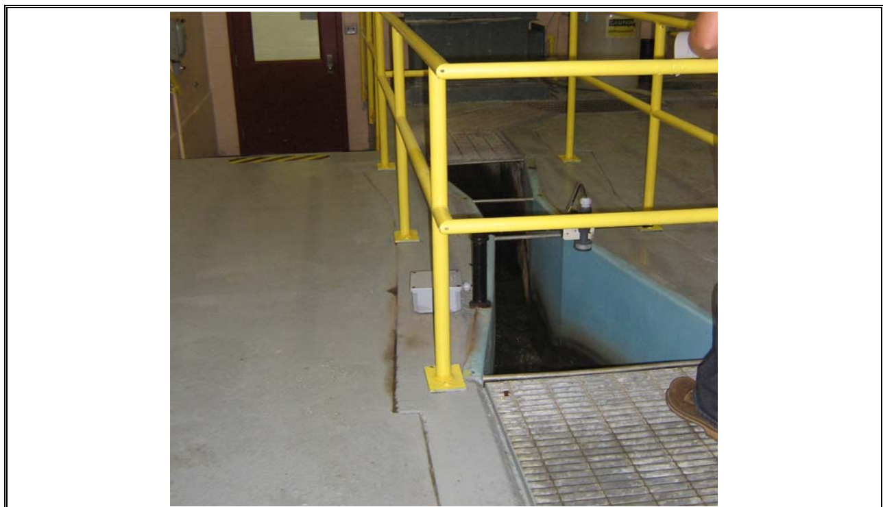
Photo 6 Parshall Flume Following Screens
