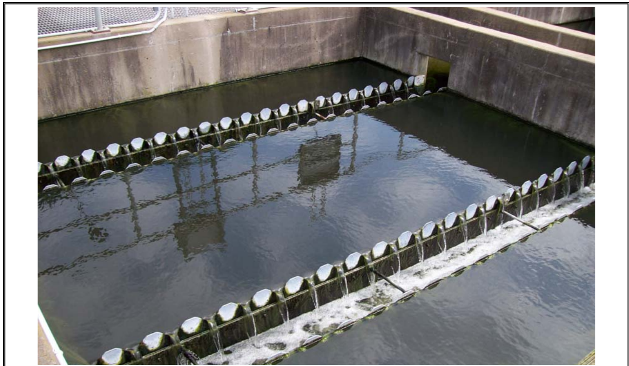
Photo 20 North Plant Secondary Effluent Trough
