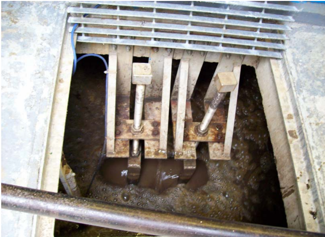
Photo 18 Lockview RAS Tank with WAS Valve Open
