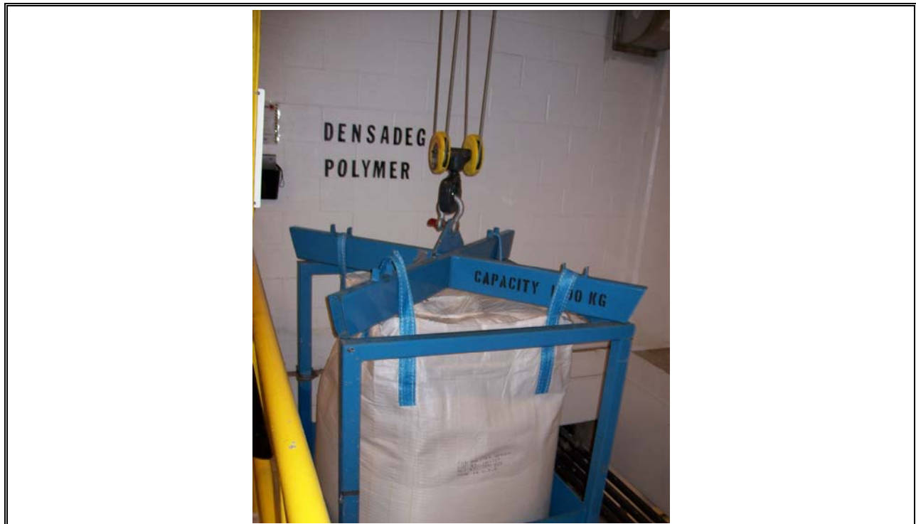
Photo 26 Halifax Densadeg Polymer Make-Up System
