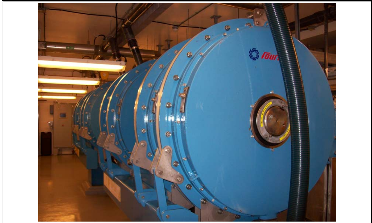
Photo 33 Halifax Fournier Rotary Presses
