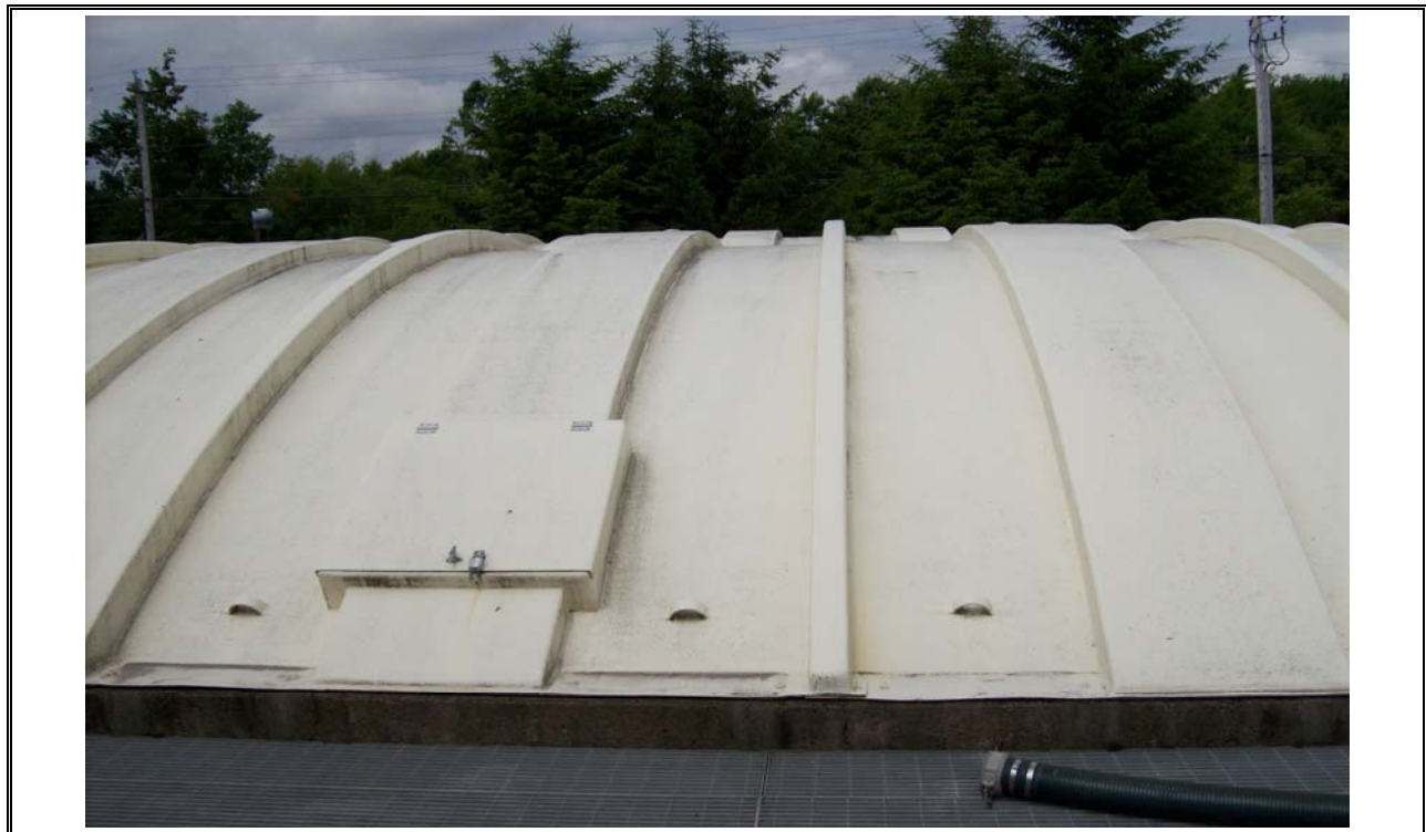
Photo 18 Primary Clarifier Cover
