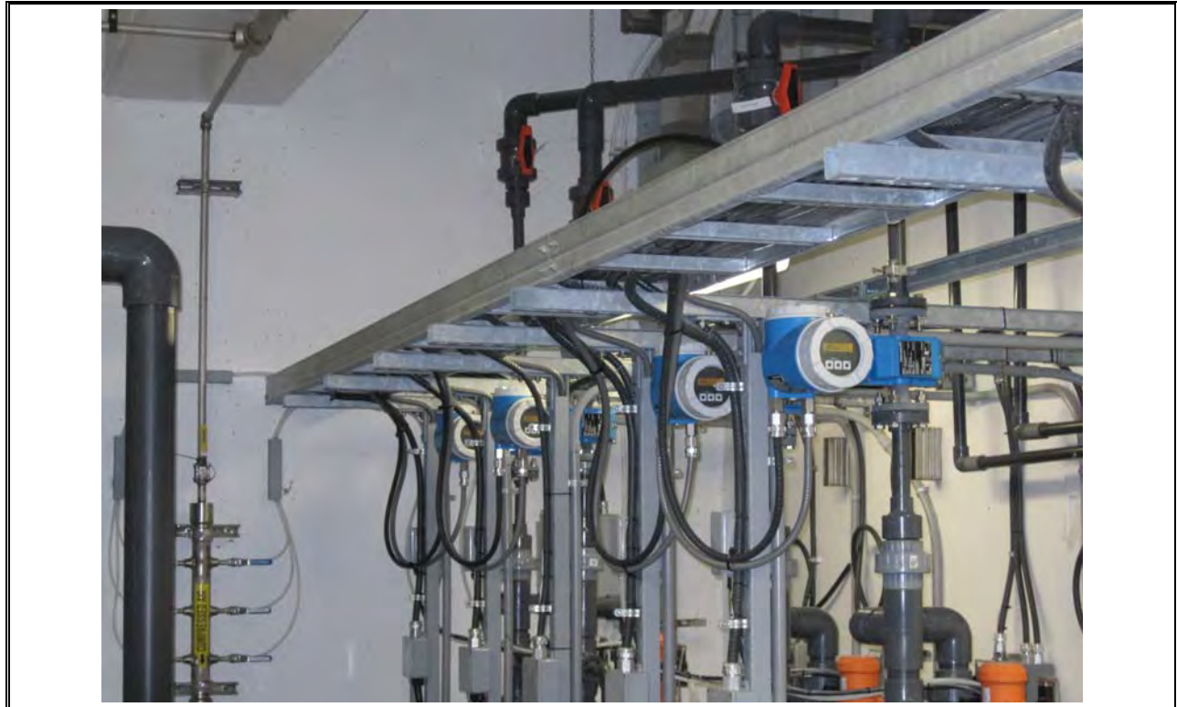
Photo 31 Dartmouth Chemical Flow Metering
