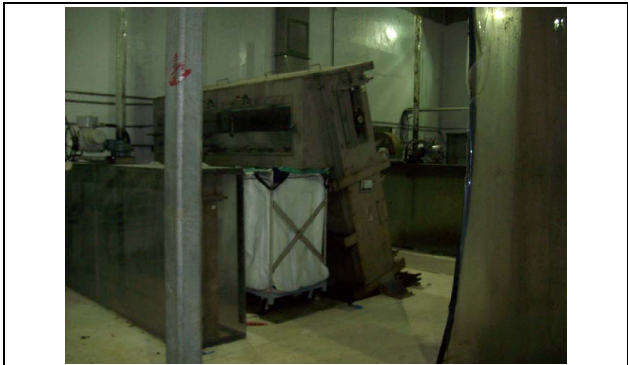
Photo 8 Halifax Back-Up Bar Screen Screenings Bin
