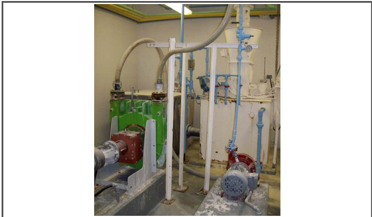
Photo 48 Lime Storage, Make-up Tank and Pumps
