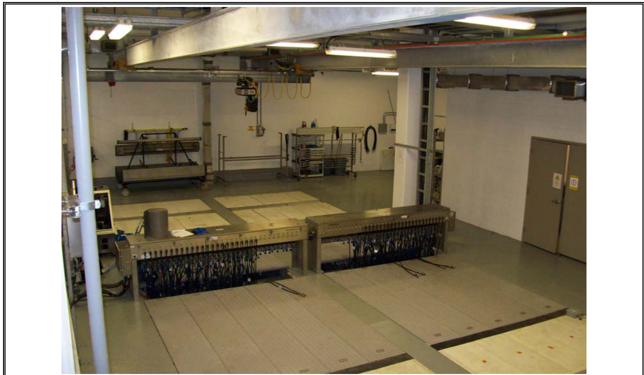
Photo 22 Halifax West UV Disinfection System
