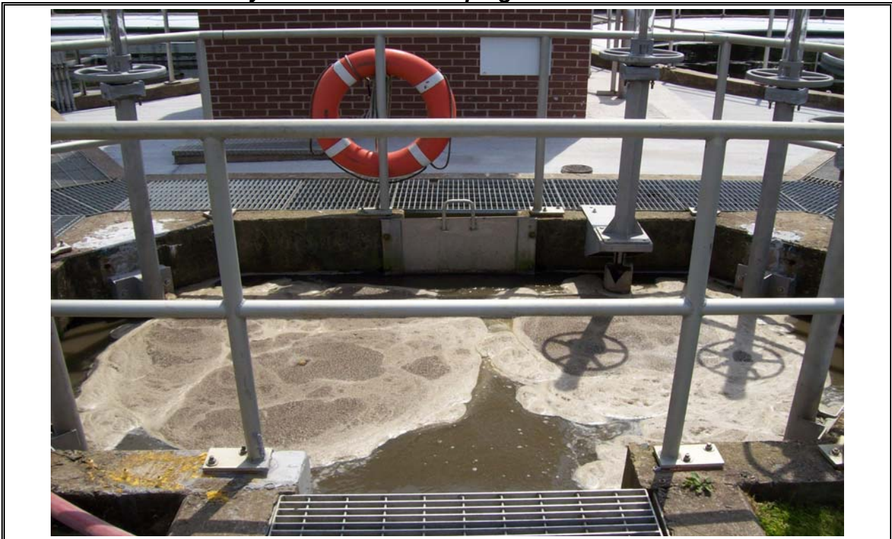
Photo 32 Secondary Clarifier Influent Flow Control
