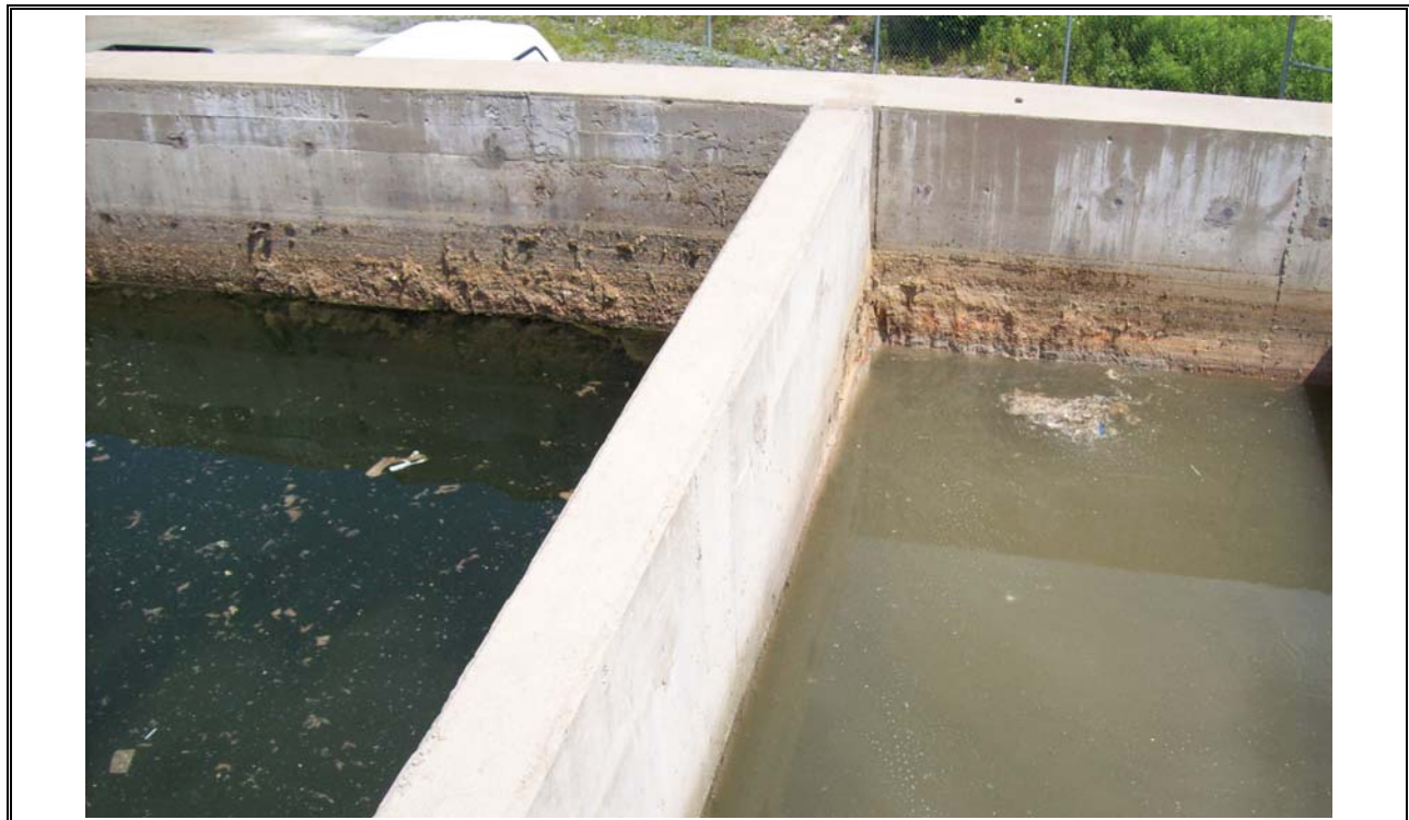
Photo 14 SBR Tanks in Decant Mode (left) and Fill Mode (right)
