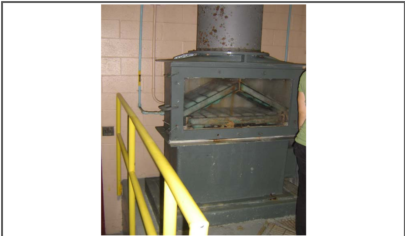
Photo 8 Odour Control System
