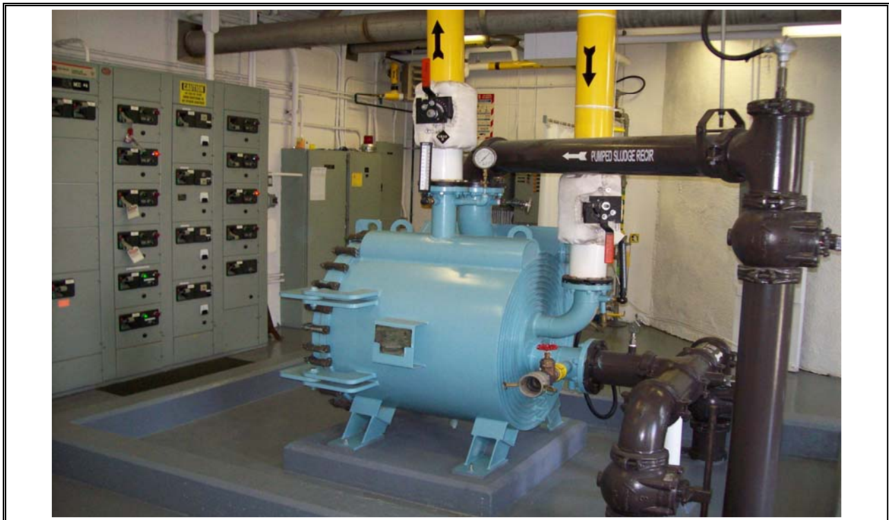
Photo 50 Heat Exchanger
